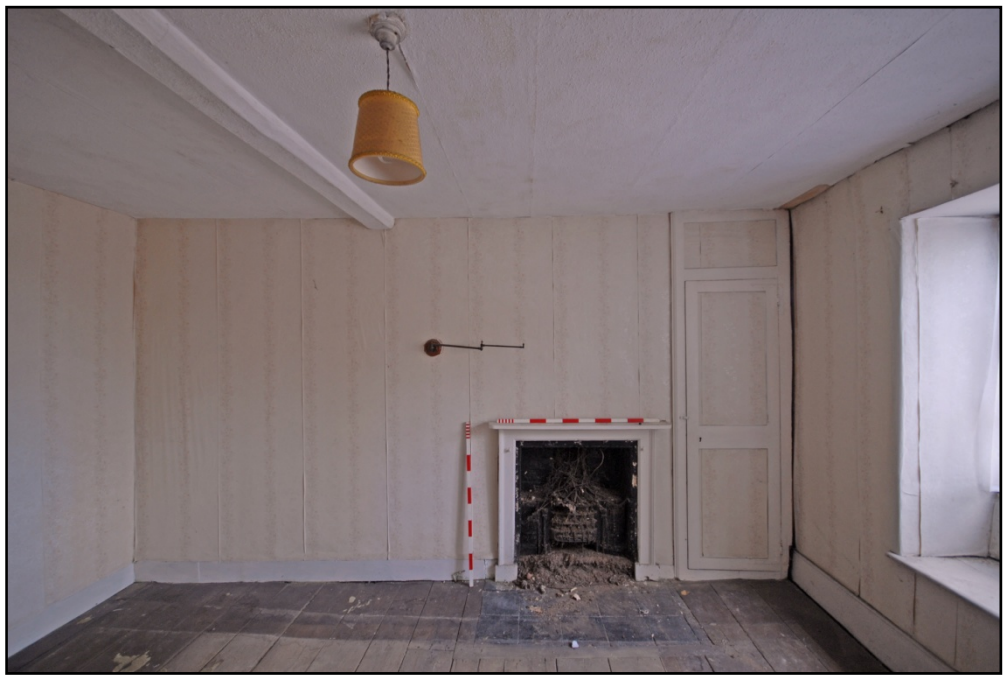
Room F2, looking north Fig 59
