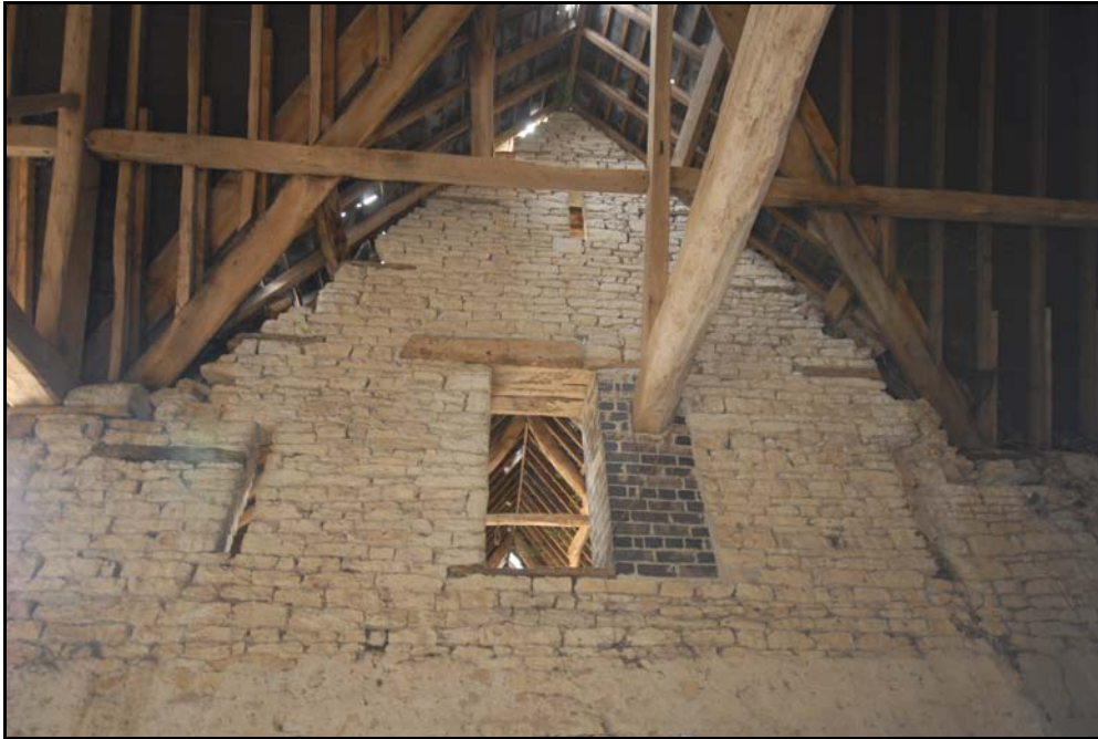
Barn 2, detail of blocked window Fig 101
