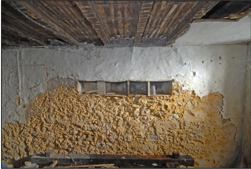
Alcoves in the north wall of the Cellar Fig 28
