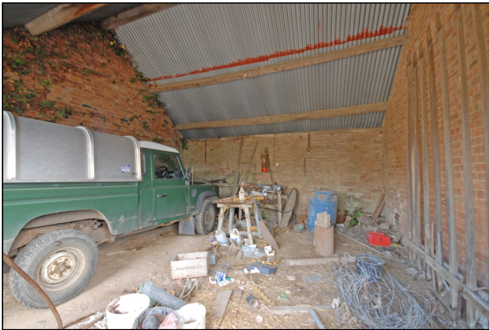
Garage 1, interior, looking north Fig 125
