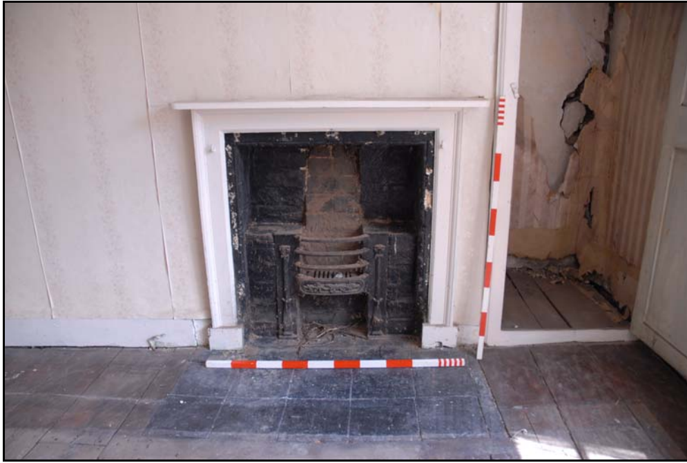
Room F2, detail of the fireplace Fig 60
