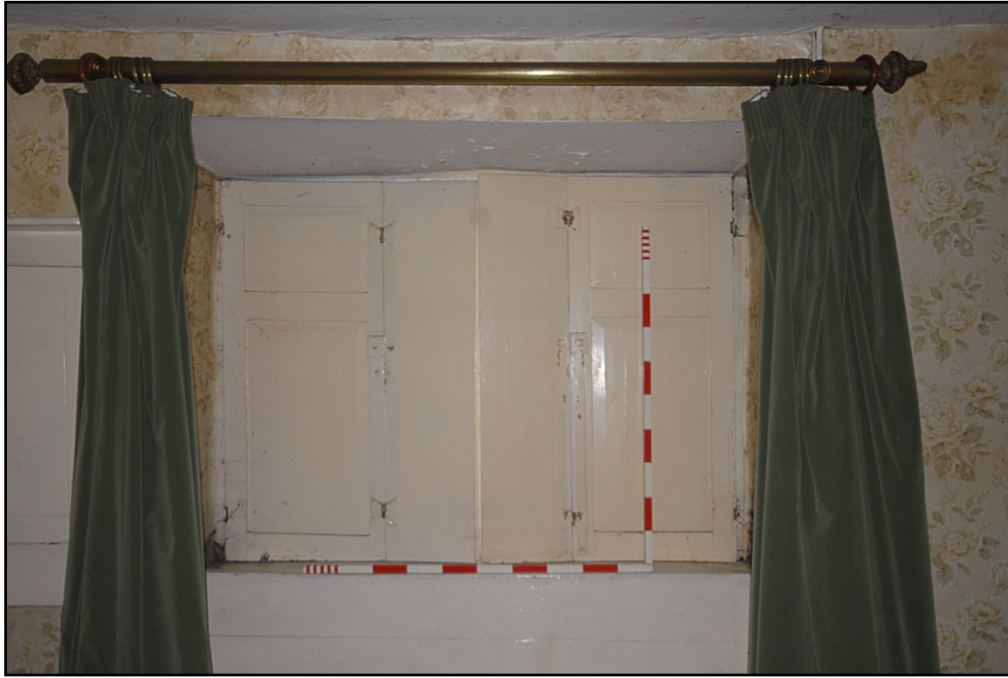
Detail of window shutters in Room G2 Fig 36
