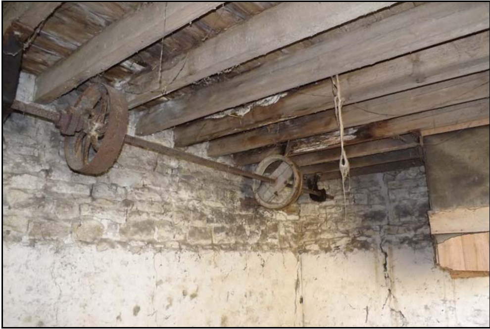
Barn 1, detail of drive shaft below Mezzanine Fig 93
