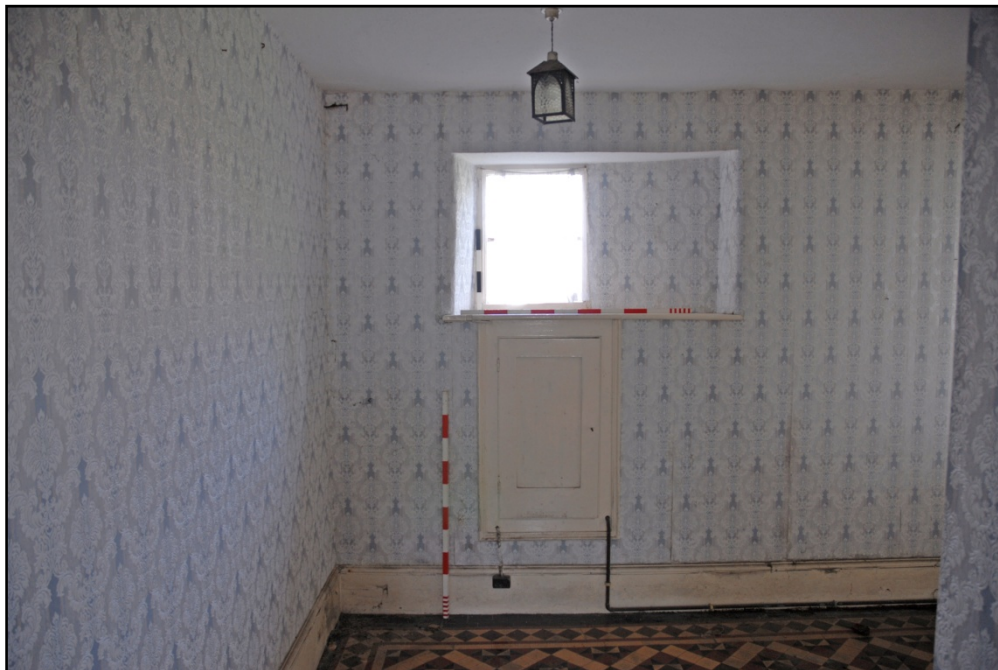
Blocked door with utility cupboard below Fig 31
