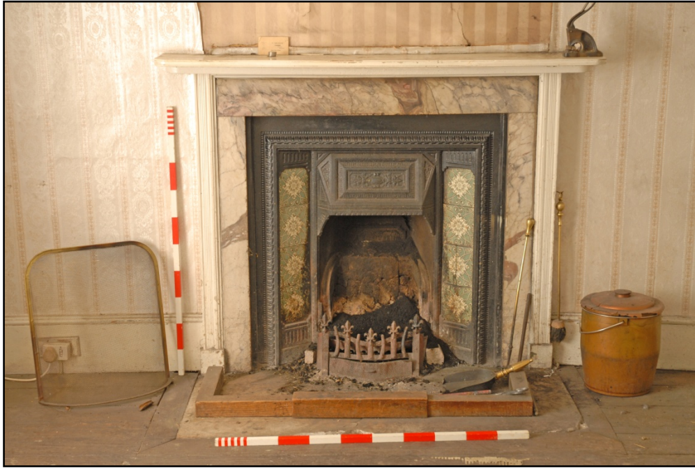
Detail of the fireplace in Room G3 Fig 38
