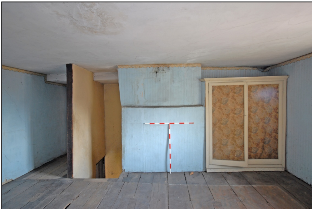
Room S2, looking east, showing chimney breast and stairs Fig 73
