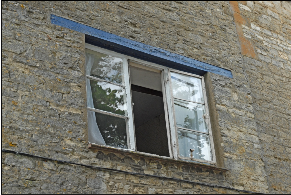
Detail of first floor window Fig 18
