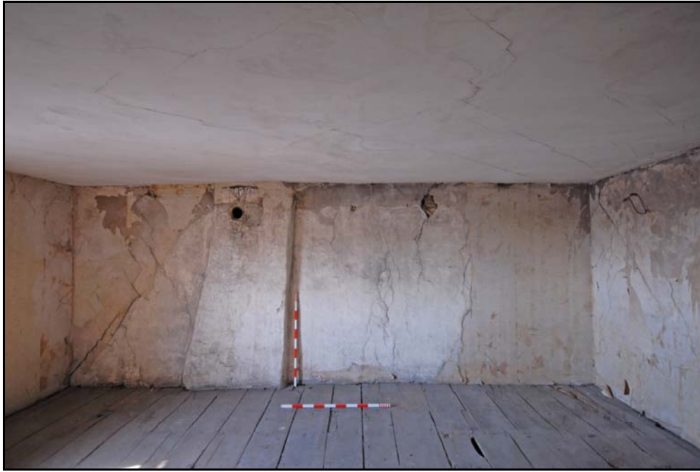
Room S1, looking south, showing chimney breast Fig 70
