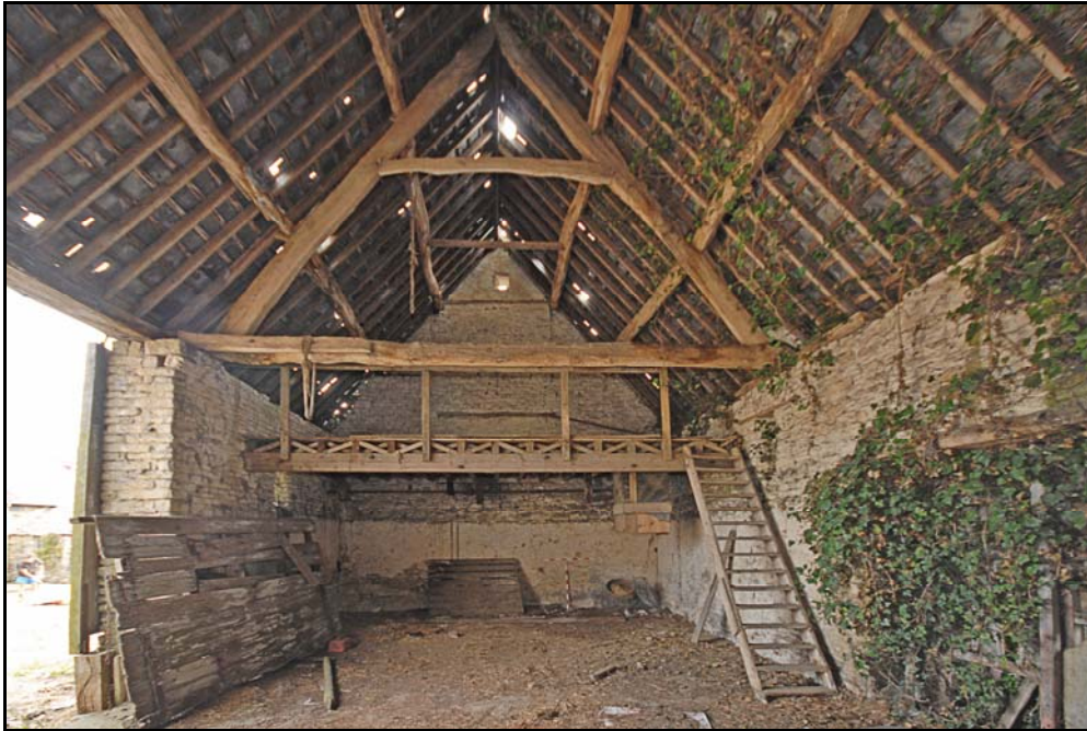
Barn 1, interior, looking east Fig 91
