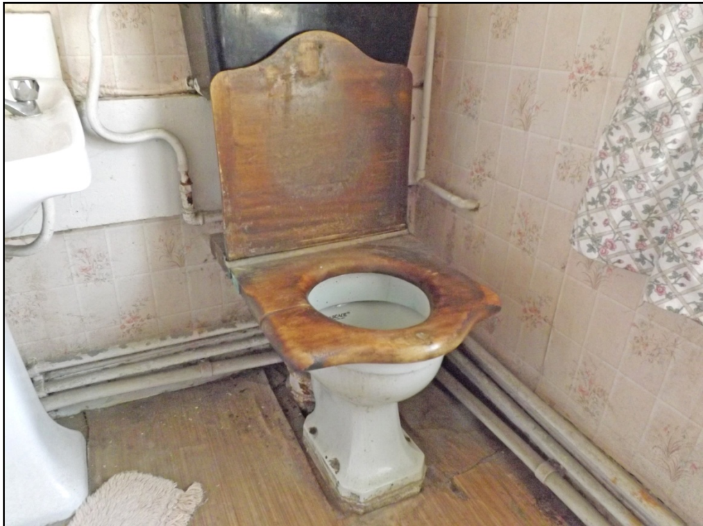
Bathroom, F5, Detail of "Cascade" toilet Fig 69
