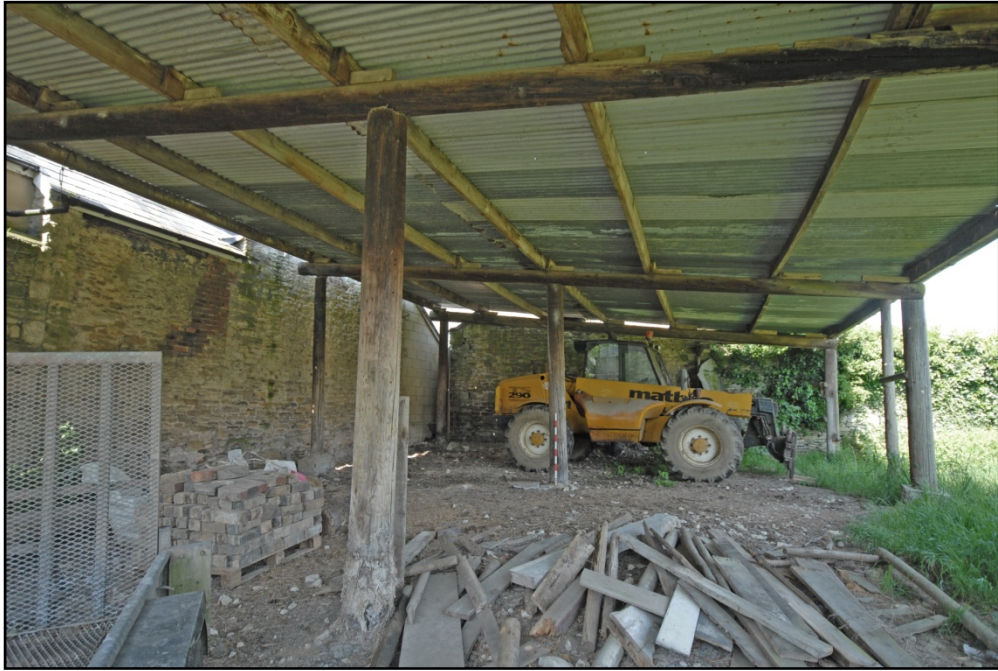
The Pole Barn, interior, looking west Fig 128
