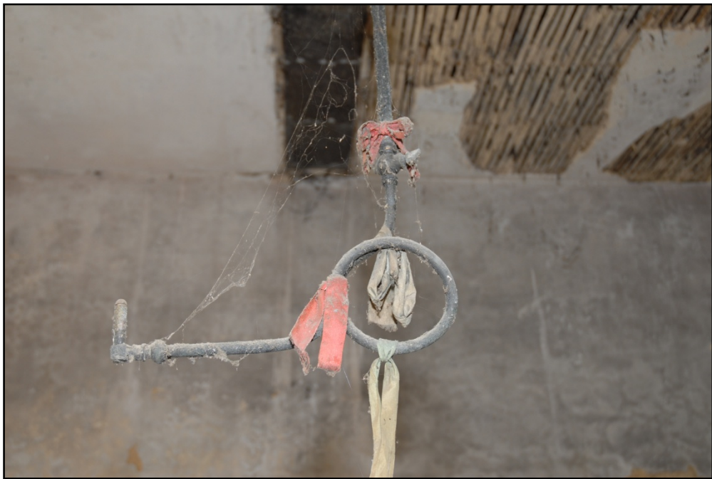
The Dairy, detail of gas light Fig 55
