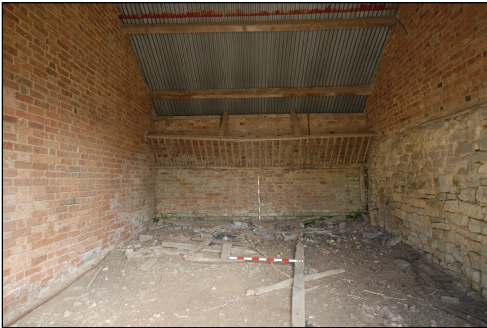
Stable 3, interior Fig 123
