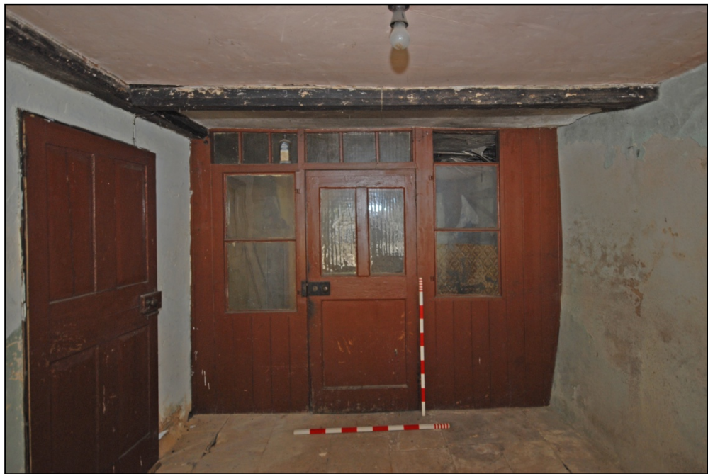
Room G4, looking west Fig 43
