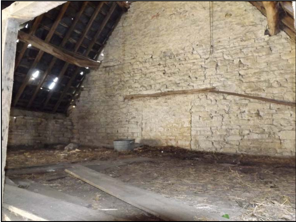
Barn 1, blocked window in the east elevation Fig 95
