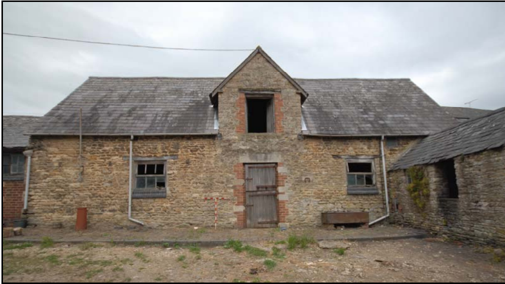
Stable 1, south elevation, looking north Fig 103
