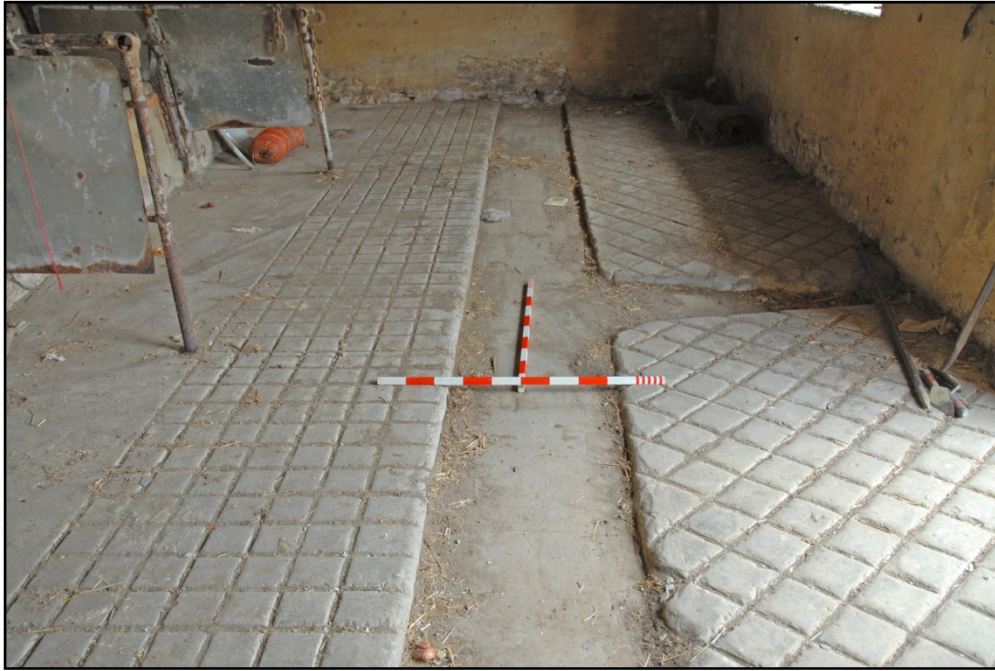
Milking Parlours, detail of concrete floors and drainage Fig 115
