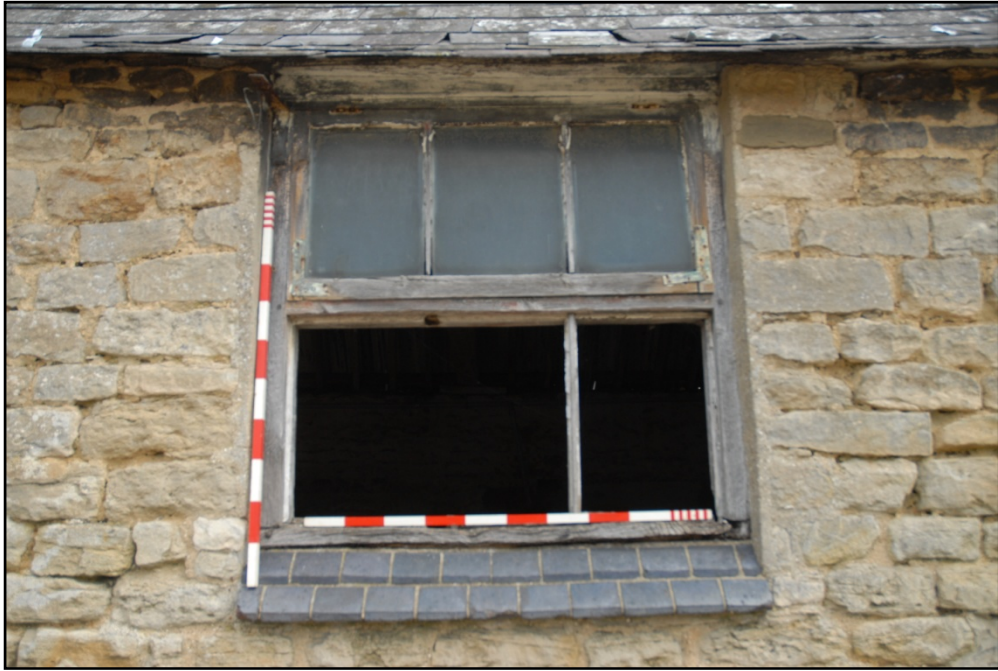
Stable 2, detail of window Fig 117
