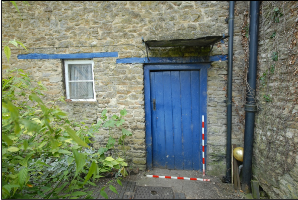
Exit from the passage with blocked door adjacent Fig 22
