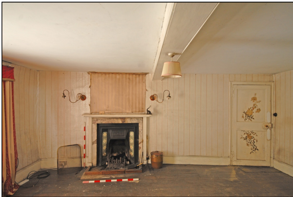
Room G3, looking south Fig 37
