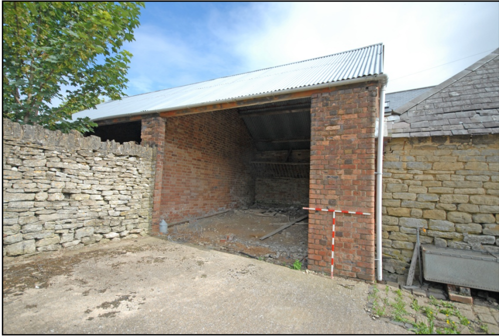
Stable 3, looking north Fig 122
