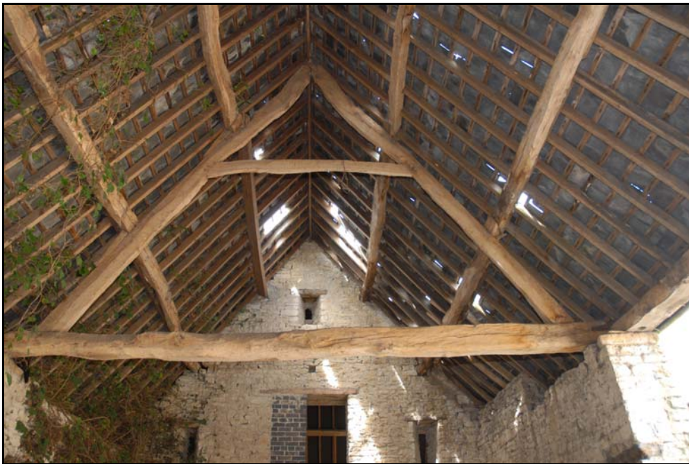
Barn 1, detail of truss Fig 94
