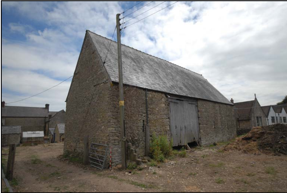
Barn 2, the west and north elevations, looking south - east Fig 97
