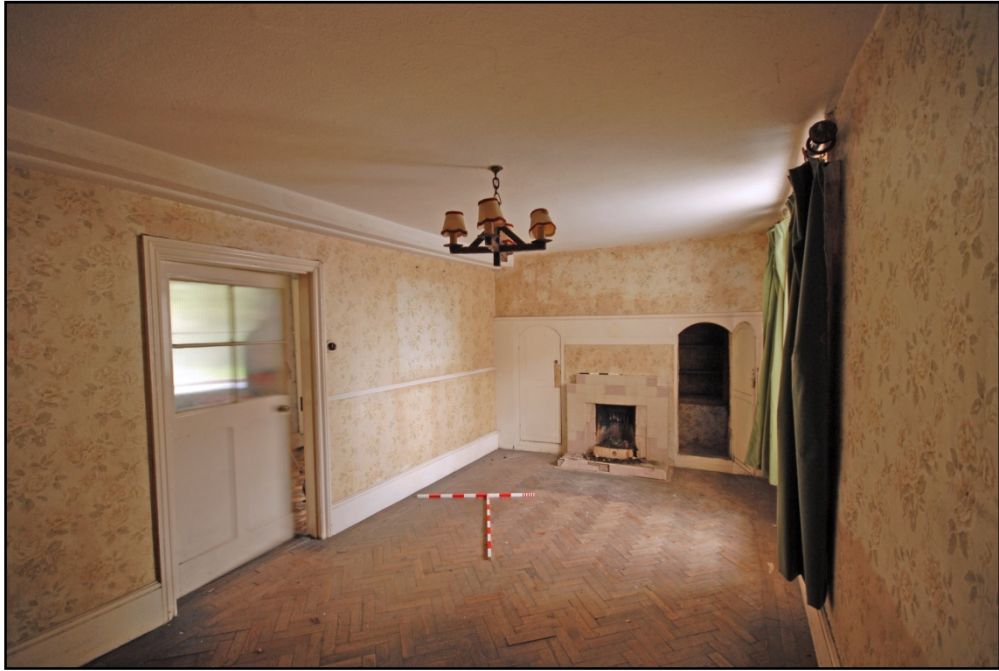
Room G2, looking north Fig 34
