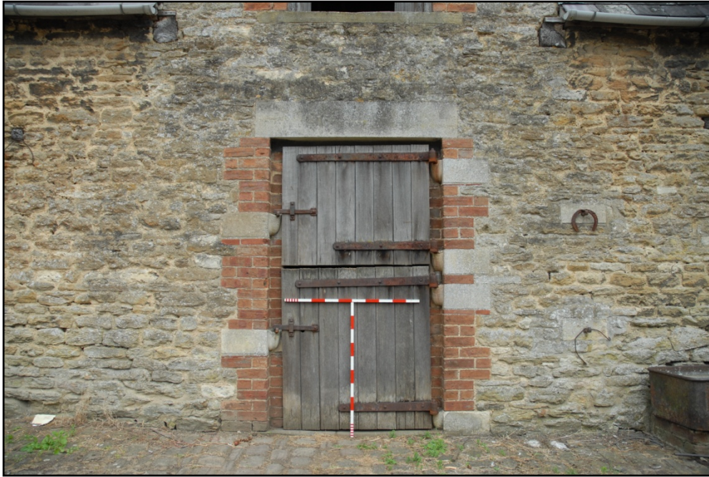
Stable 2, detail of door Fig 105
