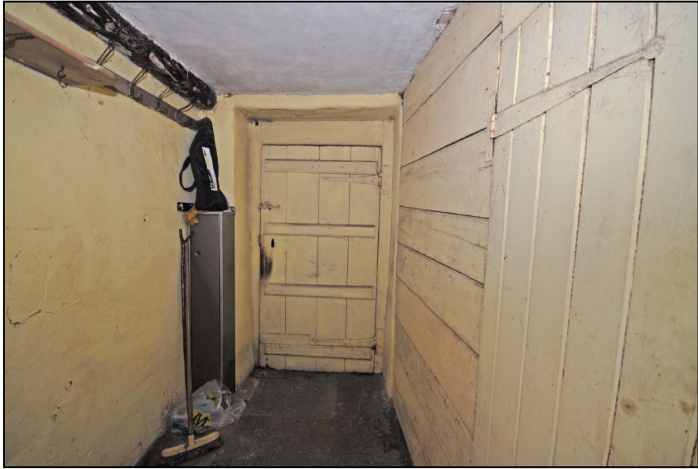
Room G5, looking west Fig 46
