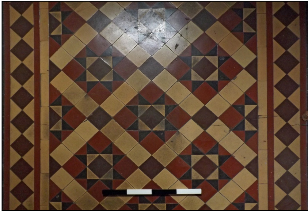
Detail of Victorian tiled floor, "Carron" pattern Fig 30
