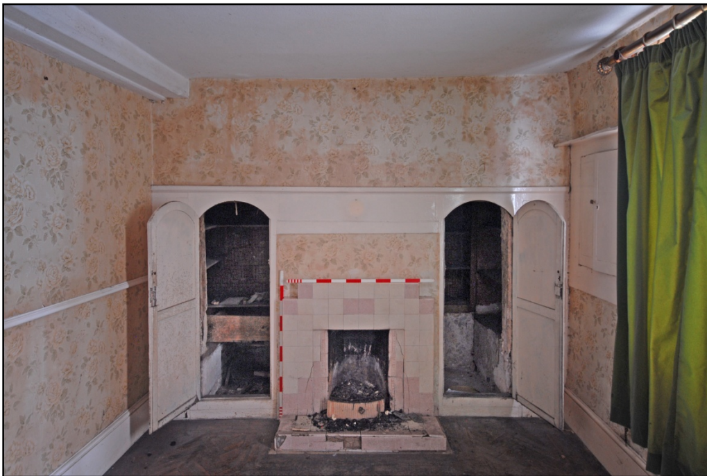
Former inglenook with 1930s fireplace Fig 35
