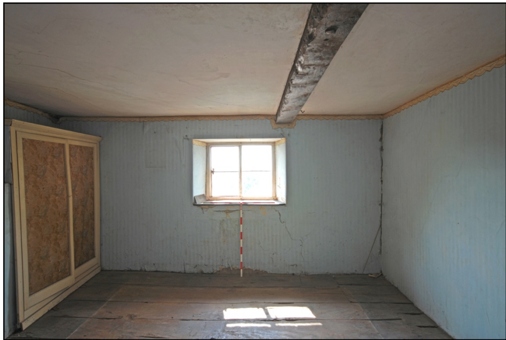
Room S2, looking east Fig 75
