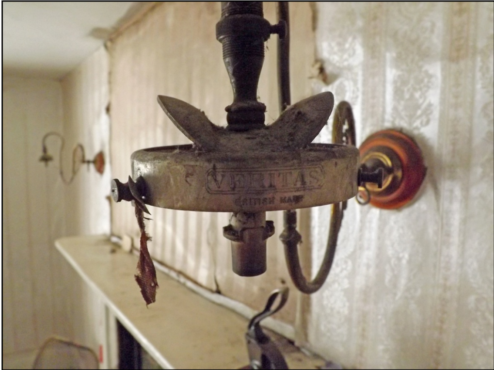
Detail of maker's mark "Veritas" on gas light bracket, Room G3 Fig 40
