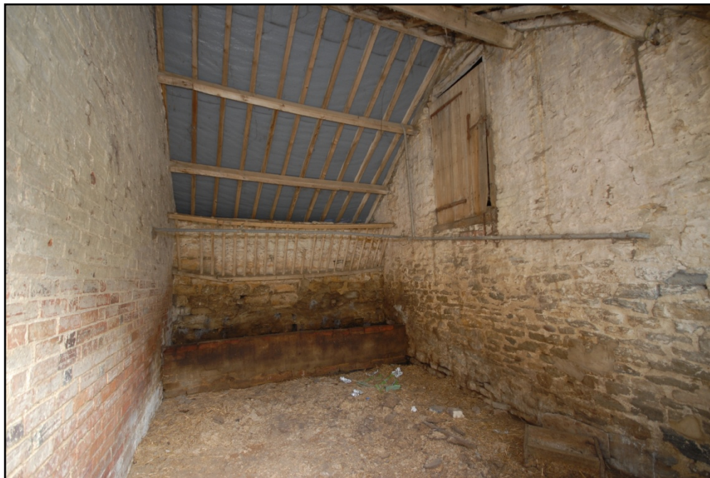
Milking Parlours, elevated door to Stable 1 Fig 112
