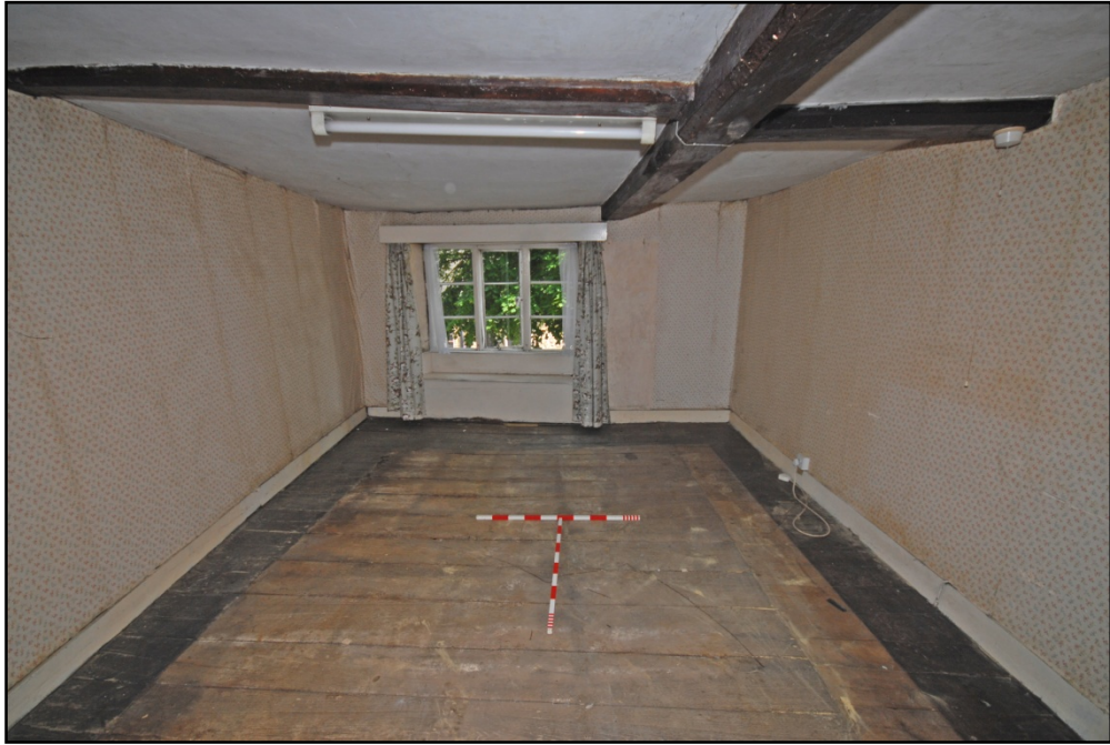
Room F4, looking east Fig 66
