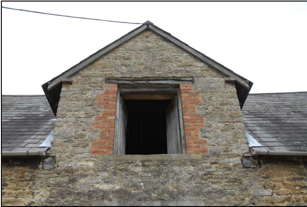
Stable 1, detail of dormer Fig 104
