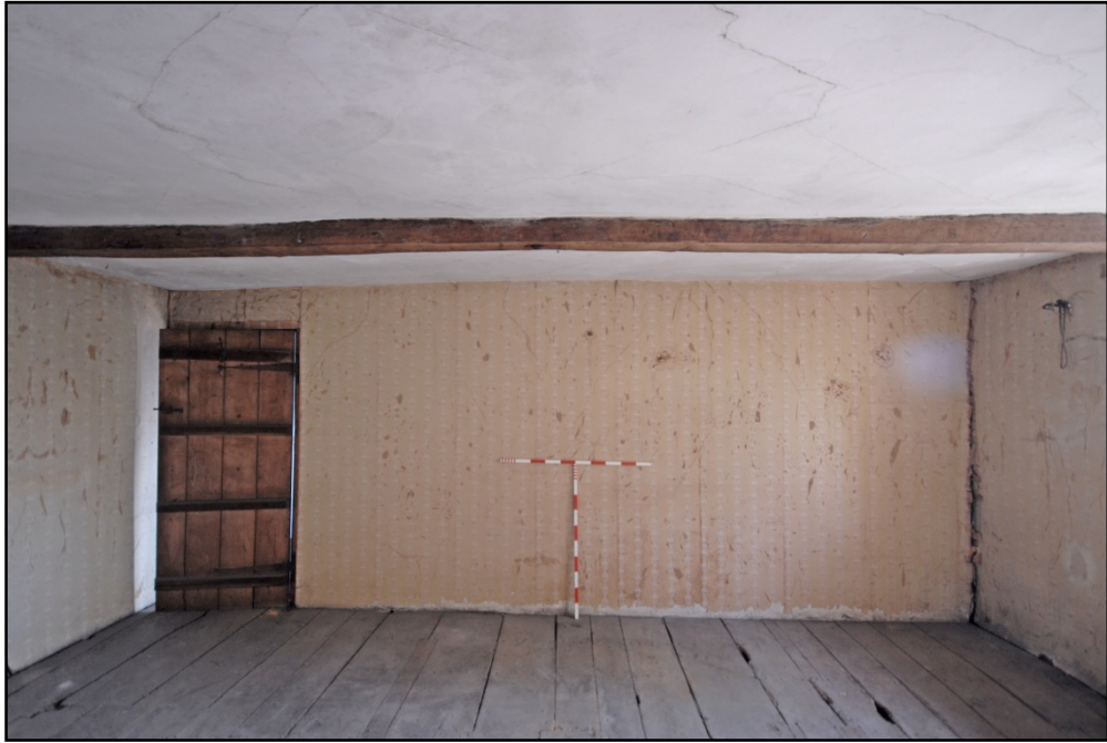
Room S1, looking north Fig 72
