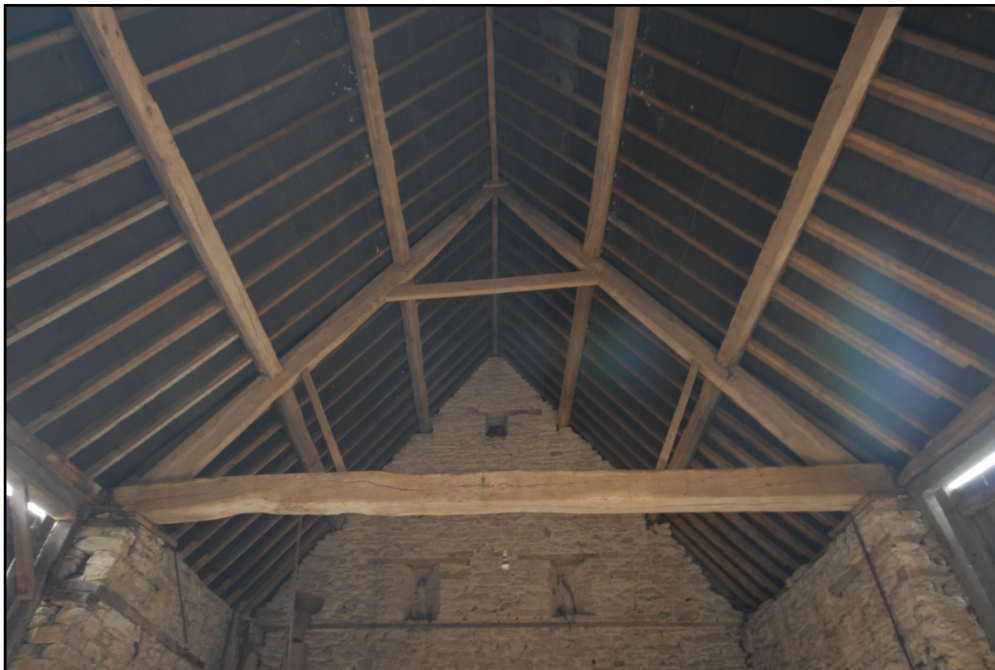
Barn 2, detail of truss Fig 102
