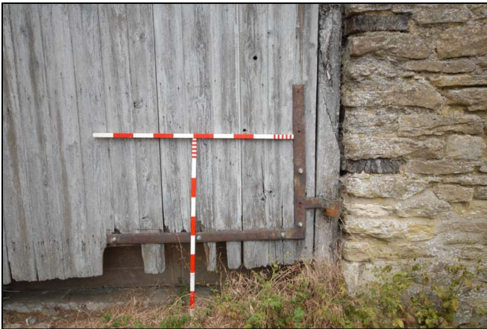
Barn 2, detail of L hinges on the east door Fig 98
