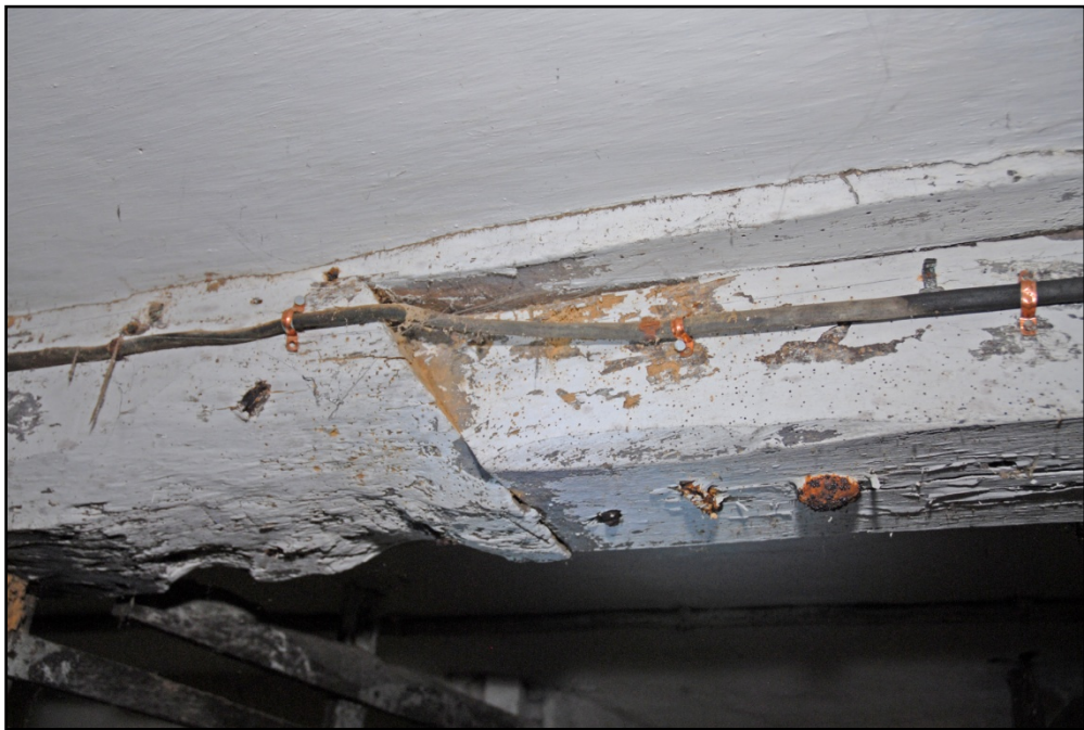
Detail of repair to the central beam Fig 25
