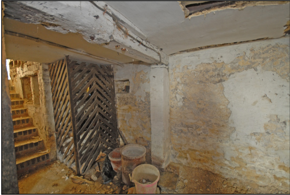
The Cellar, looking south Fig 24
