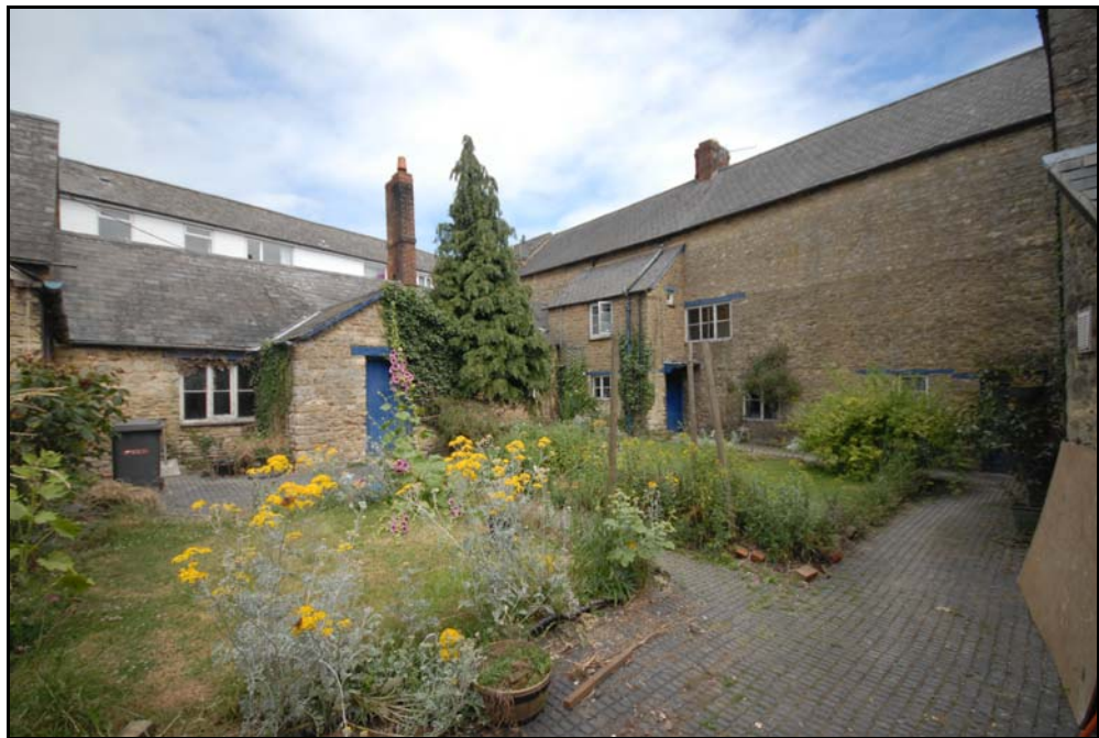
View towards the Kitchen and Dairy, looking north - east Fig 23
