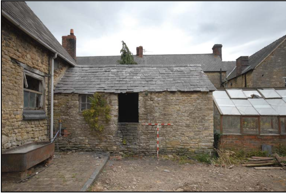
The Coal Shed and Privy, looking east Fig 85
