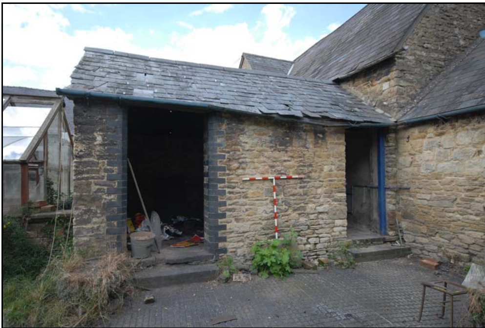
The Coal Shed and Privy, looking west Fig 84
