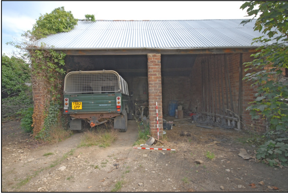
Garage 1, looking north Fig 124
