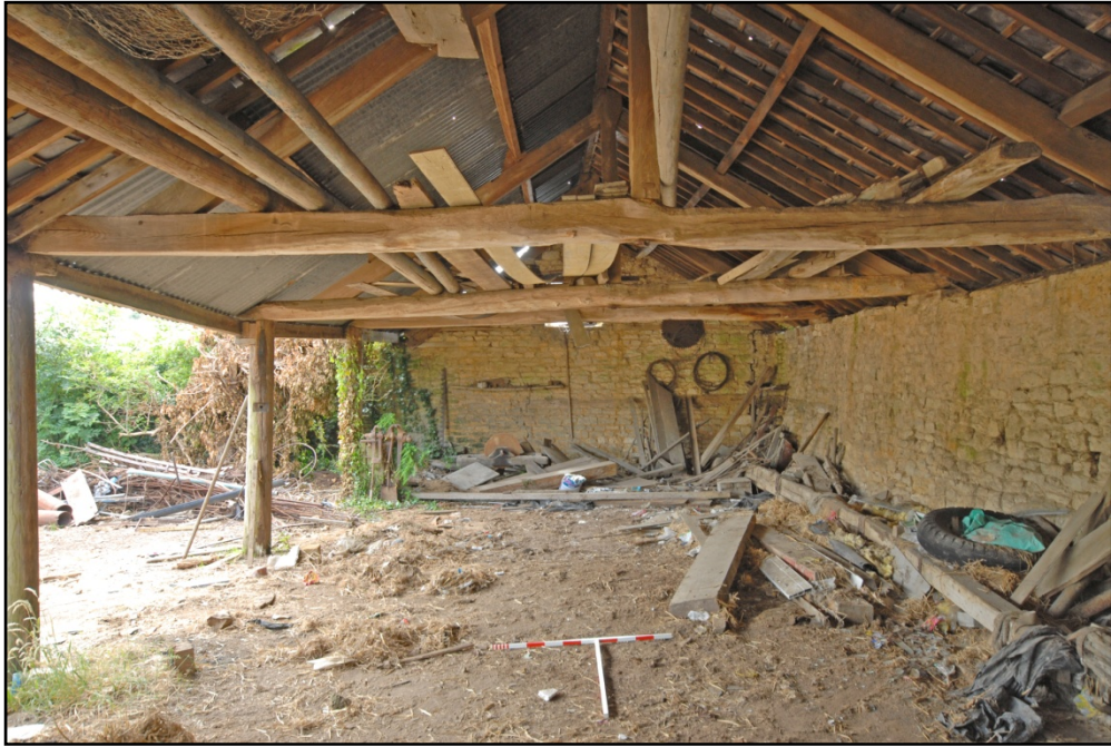
Cart Shed, looking east Fig 130
