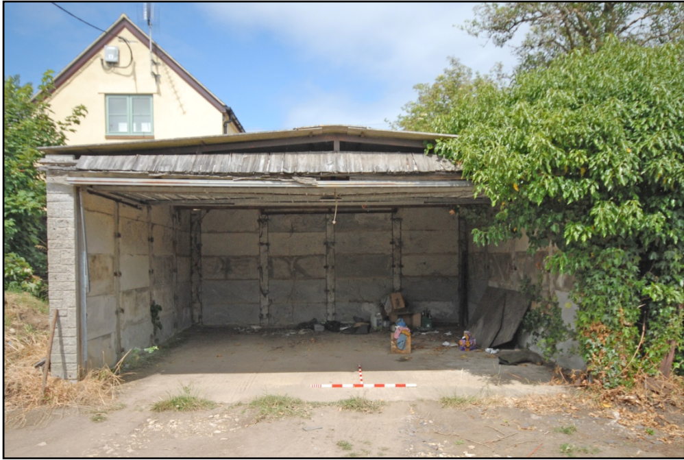
Garage 2, looking north Fig 126
