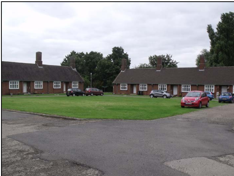
The site upon completion, looking south-west Fig 7
