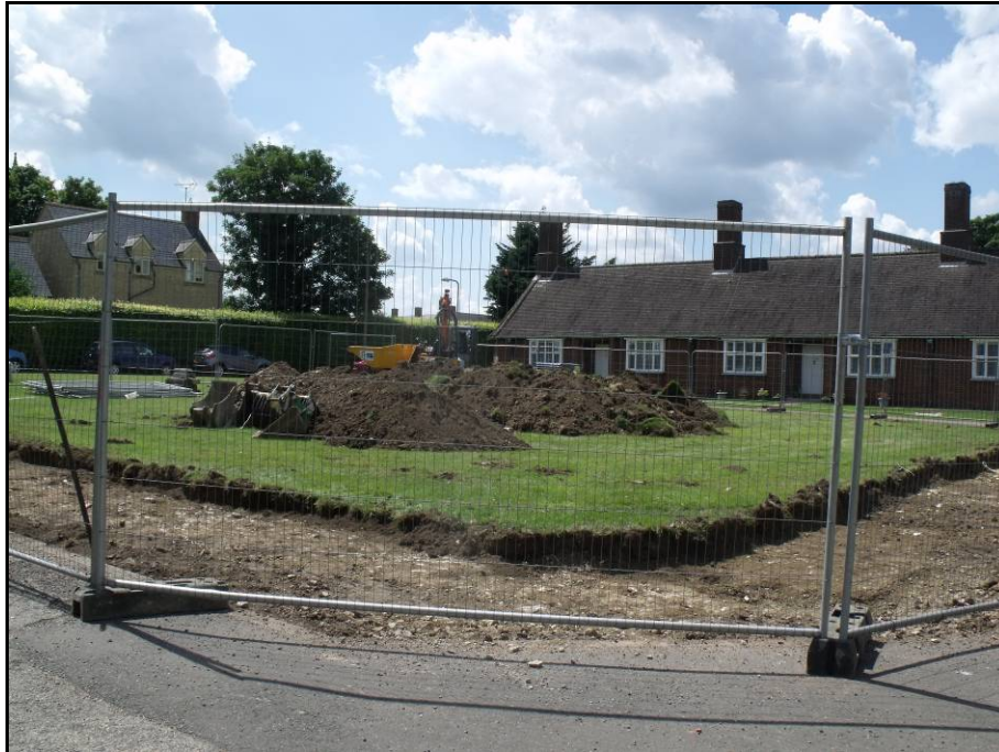
The excavated area, looking south-west Fig 4
