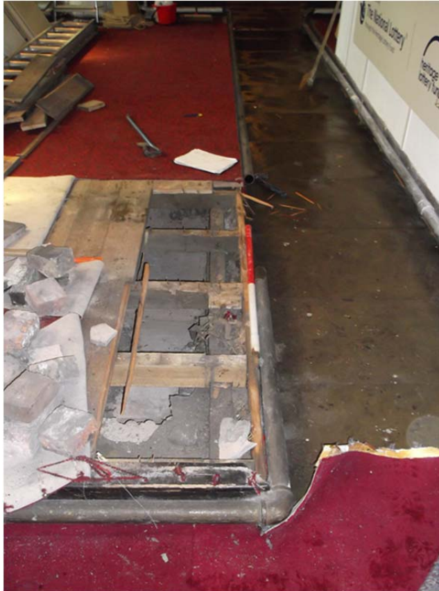
General view of test pit 1 Fig 4
