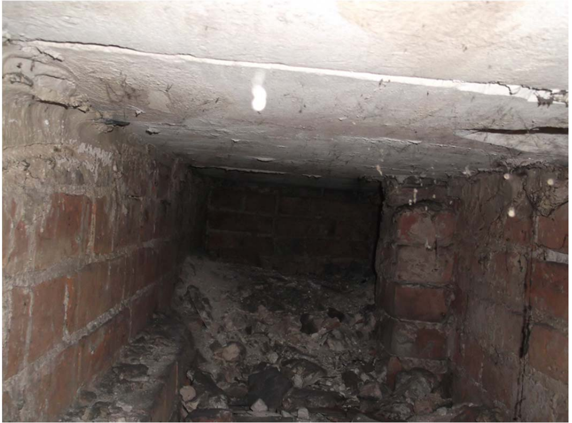
The void beneath the flag floor, test pit 1 Fig 5
