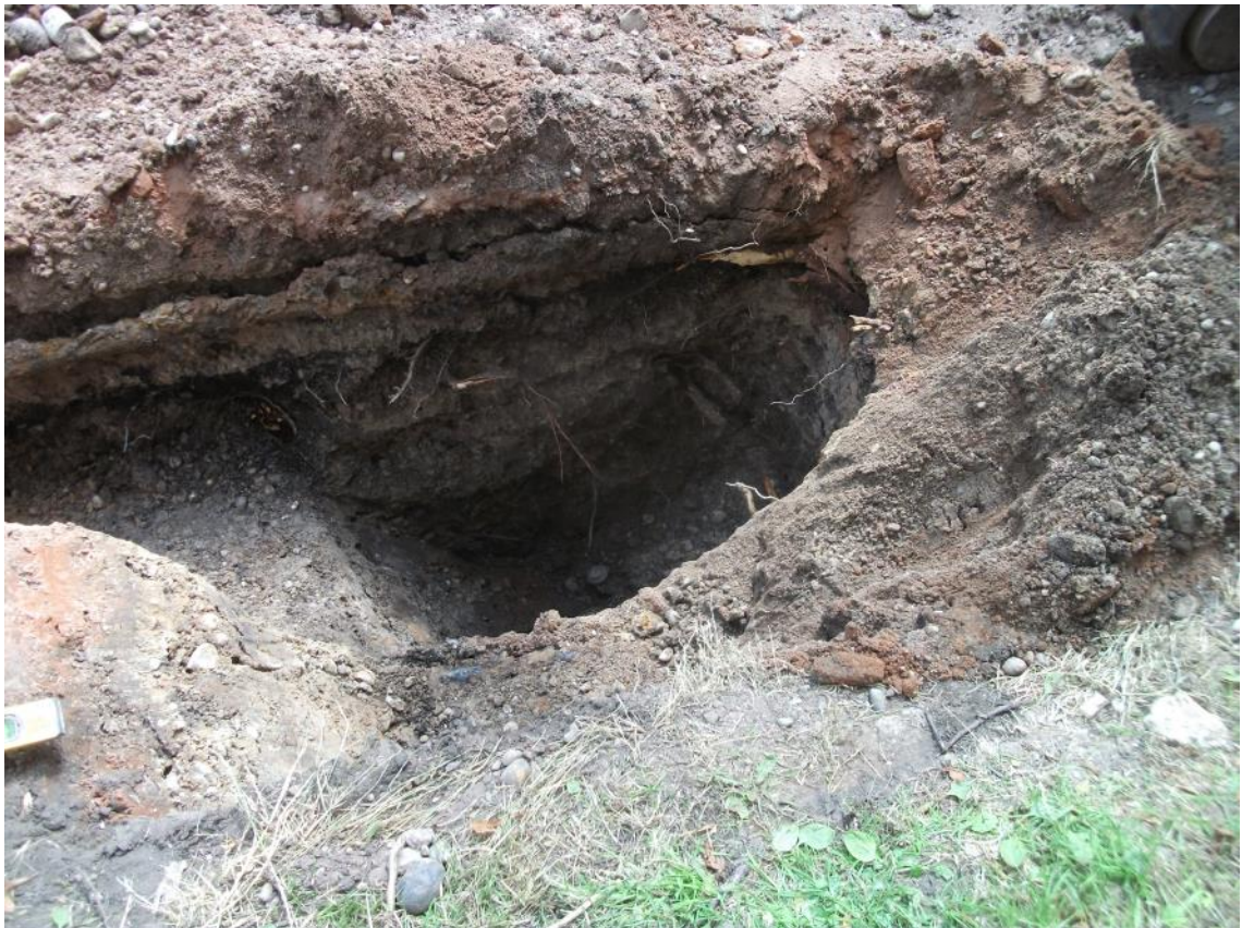
The new soak-away Fig 10
