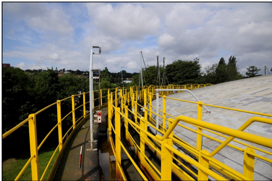
General view from the walkway of the static base Fig 24
