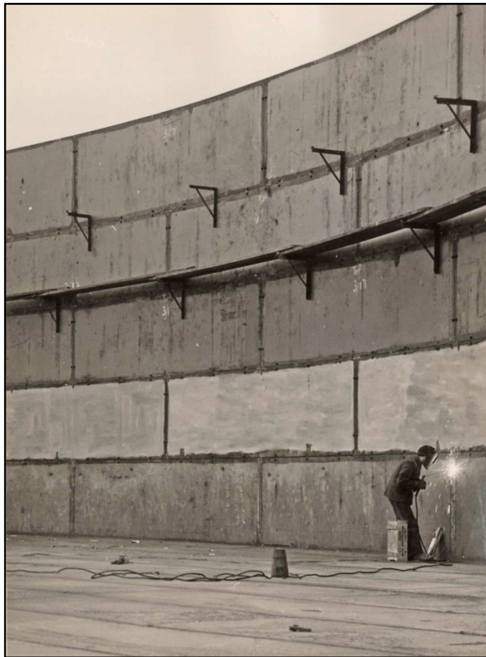
Gasholder 4 under construction (c.1950) Fig 11
