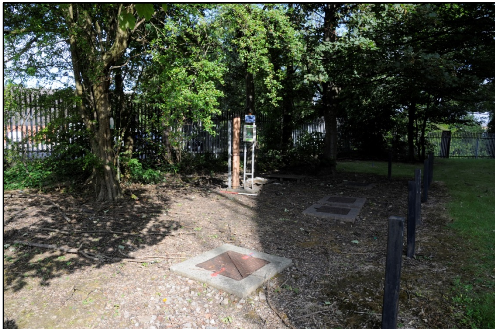
Manhole covers and separator alarm system Fig 31
