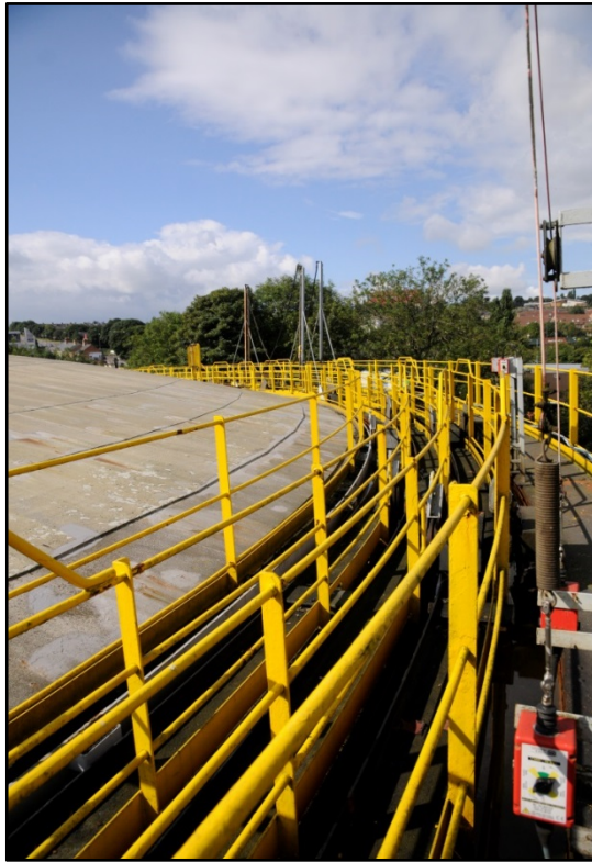
View of the static base tank, showing the safety railings of the four upper lift tanks Fig 19
