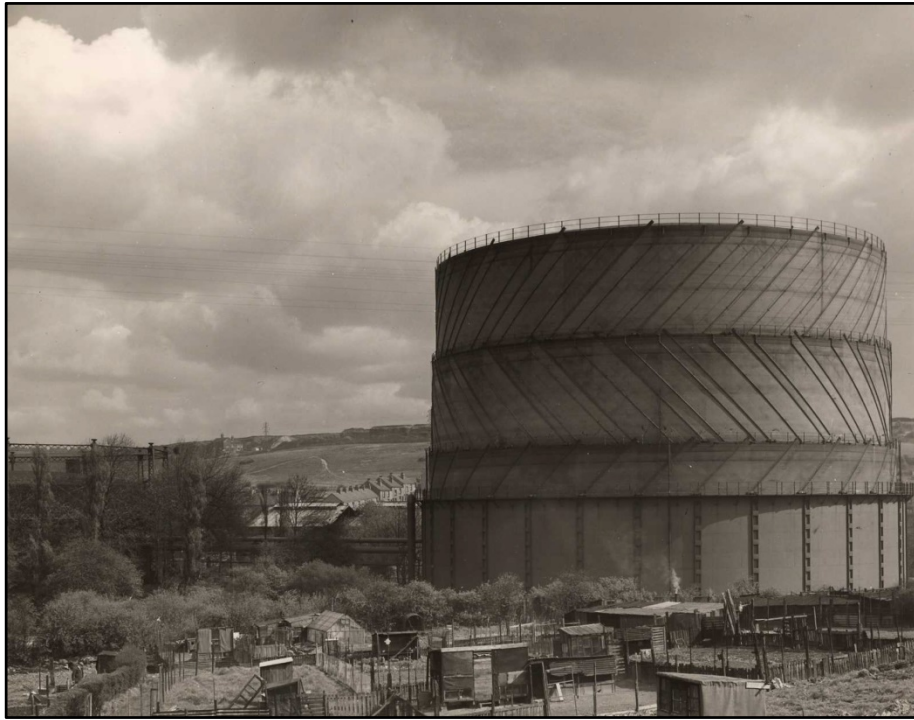
Gasholder 4, fully raised with allotments in the foreground (c.1960) Fig 12
