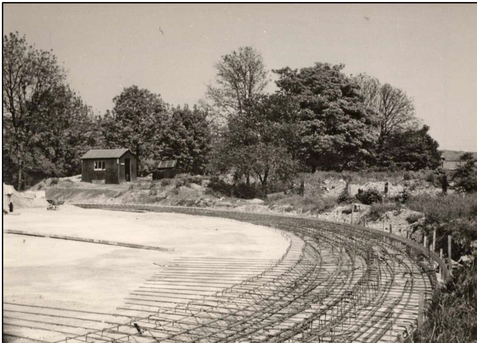
Construction of foundations for Gasholder 4 (c.1950) Fig 9
