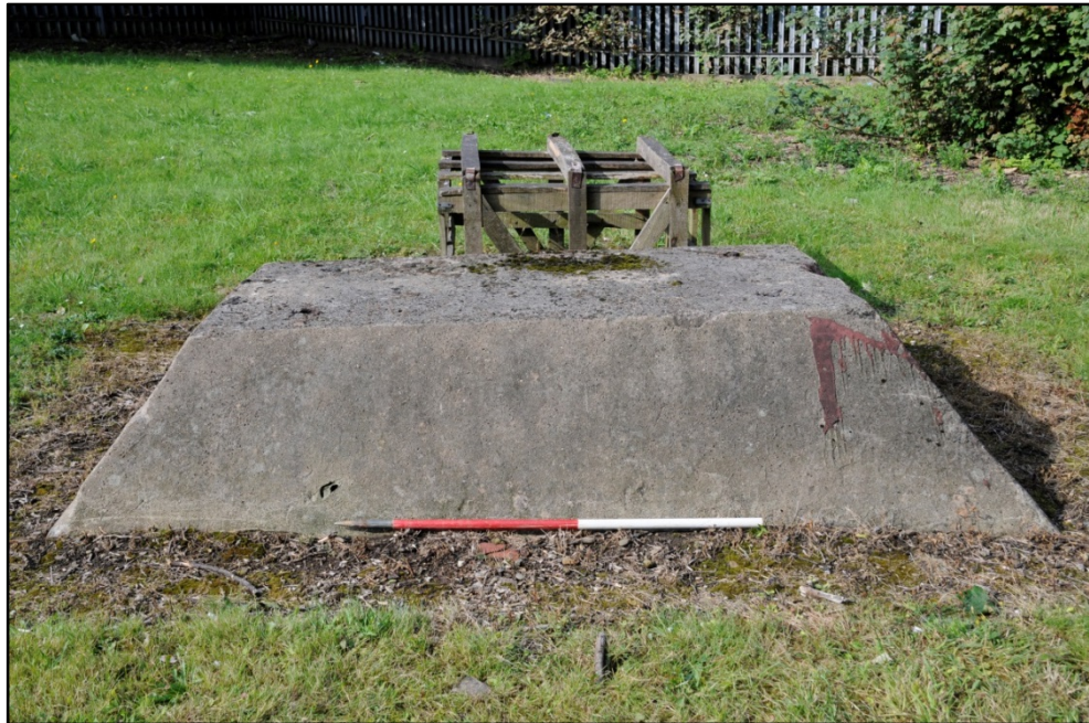
Concrete plinth Fig 30
