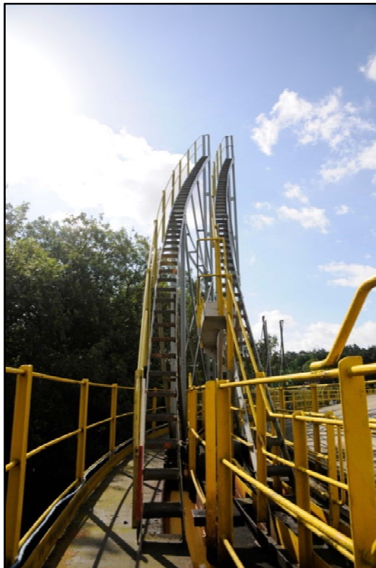
The eastern pair of staircases for the upper lift tanks Fig 22
