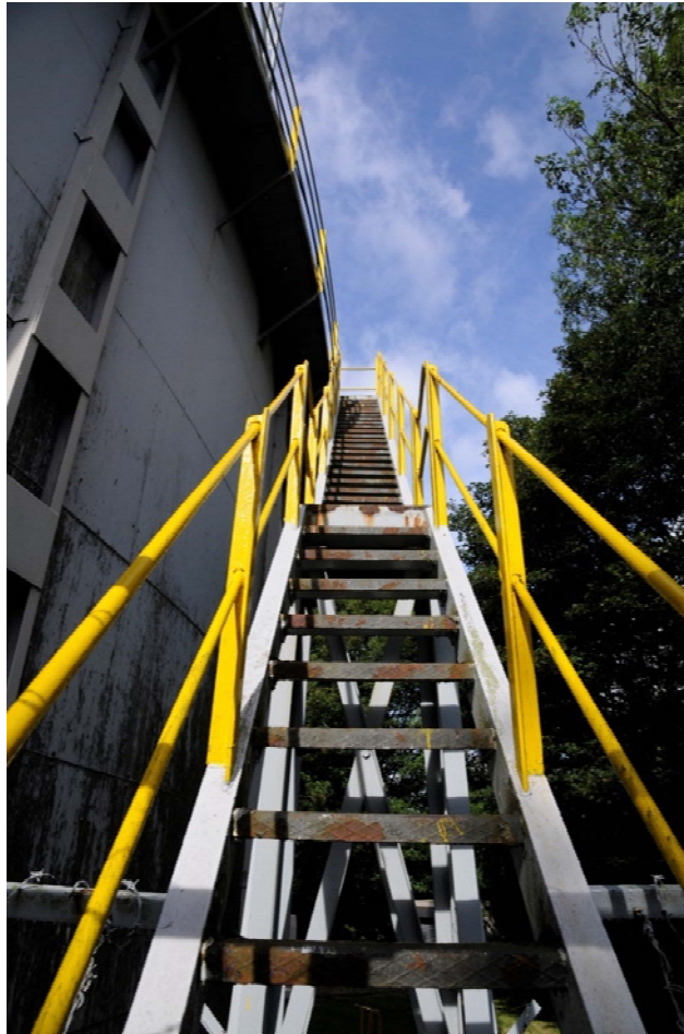
Upper section of external staircase Fig 17
