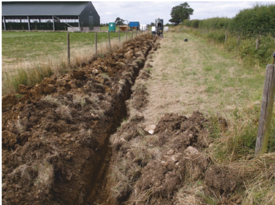
Excavation in progress of the service trenches, looking west Fig 7
