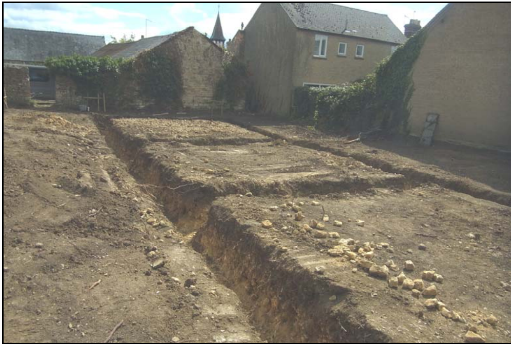
The footings trenches, looking south-east Fig 5
