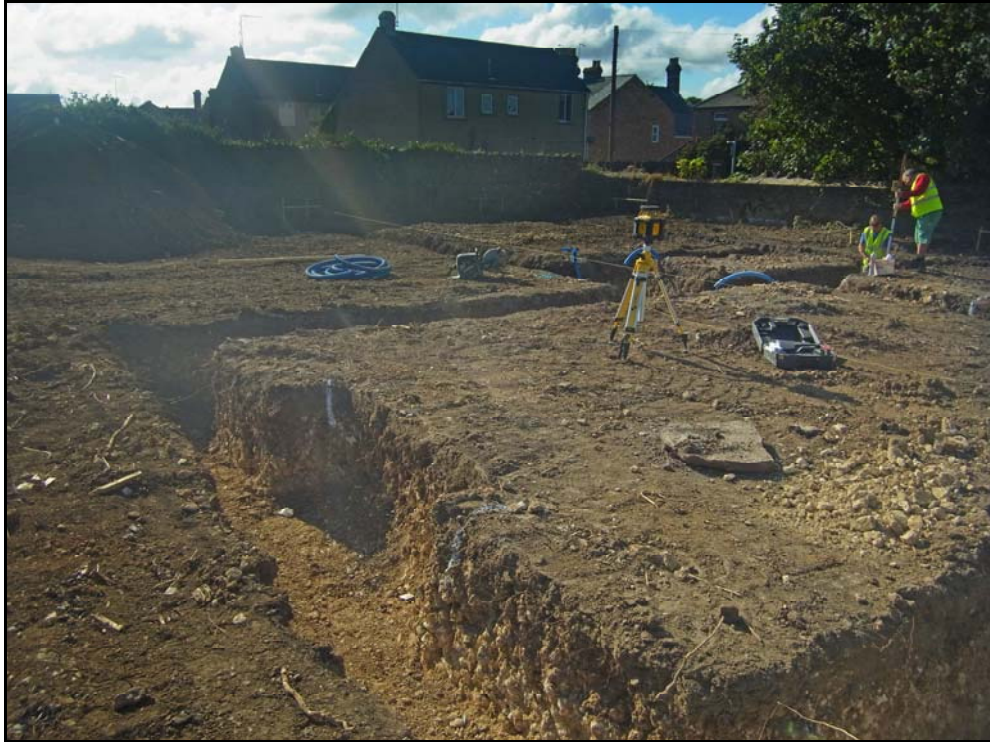
The footings trenches, looking south-west Fig 6
