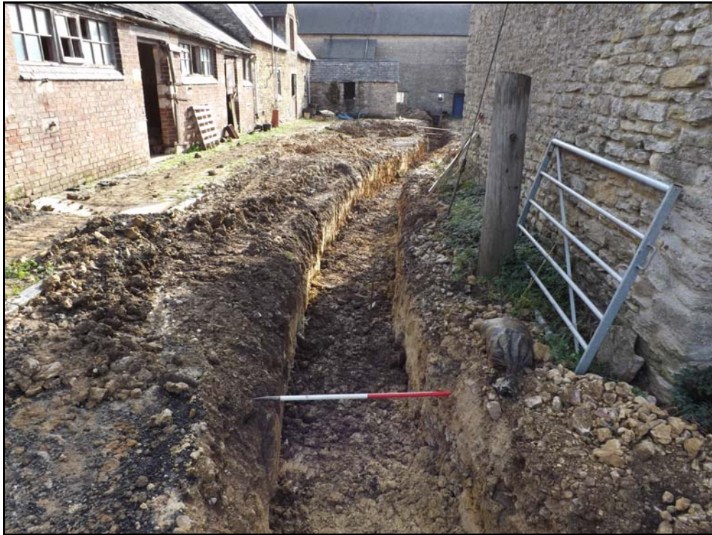
The service trench alongside the barns, looking east Fig 12
