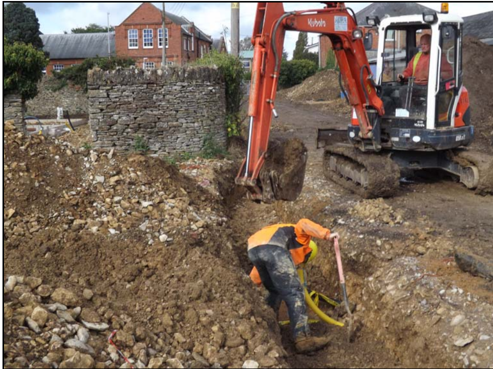
The excavation of the service trenches, looking west Fig 8
