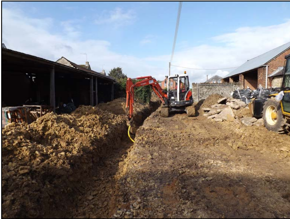
The excavation of service trenches across the former farmyard Fig 10
