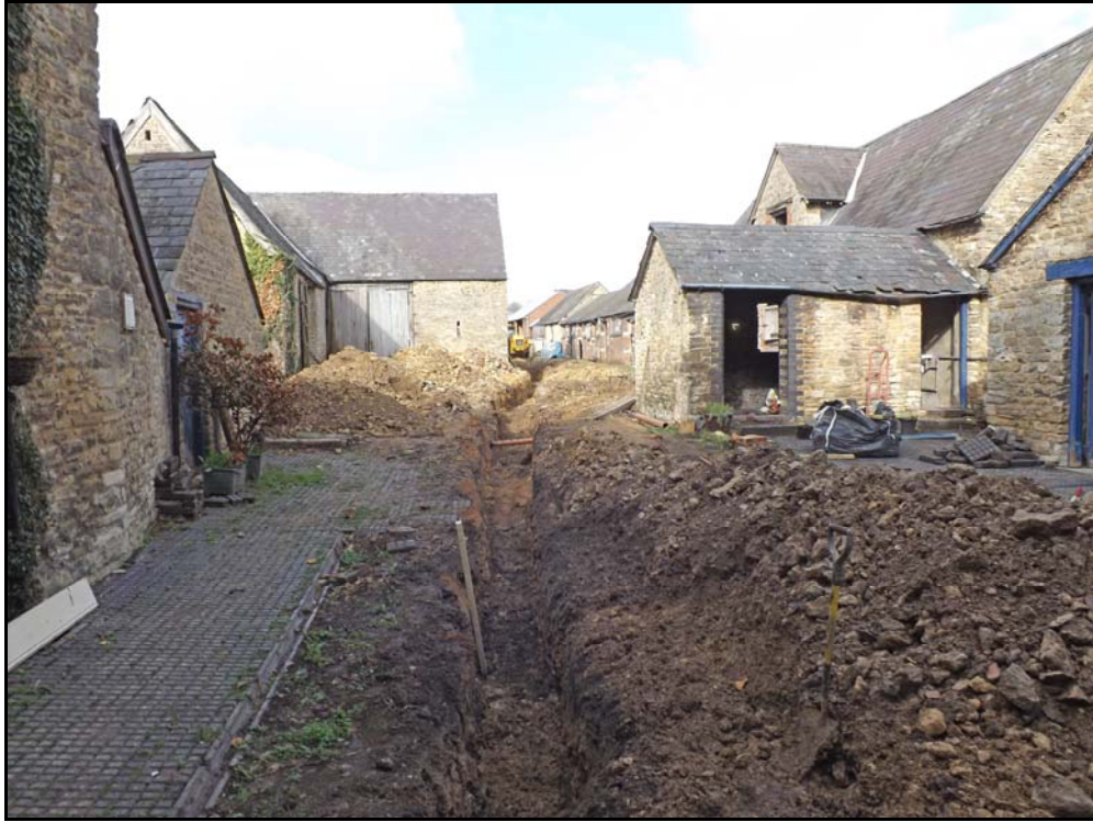
The service trenches, looking west from the farmhouse Fig 14
