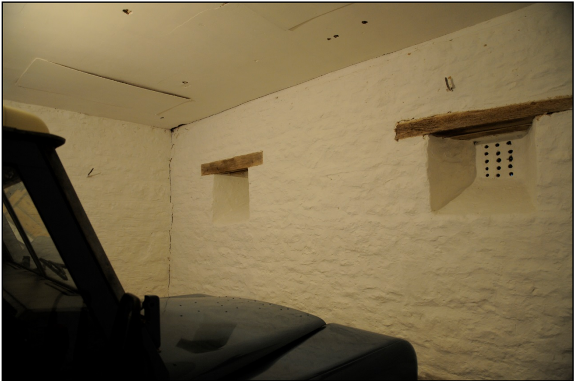
Room G2, detail of ventilation in south wall, looking south-east Fig 13
