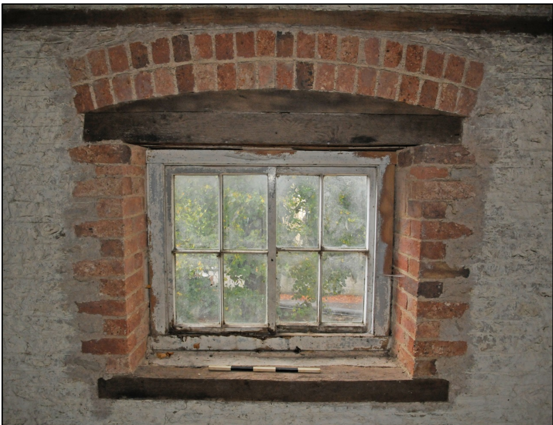
Room F2, detail of window with timber bonding course over Fig 22
