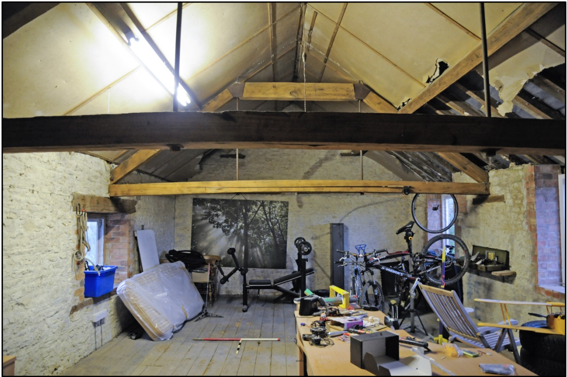
Room F1, looking east Fig 15
