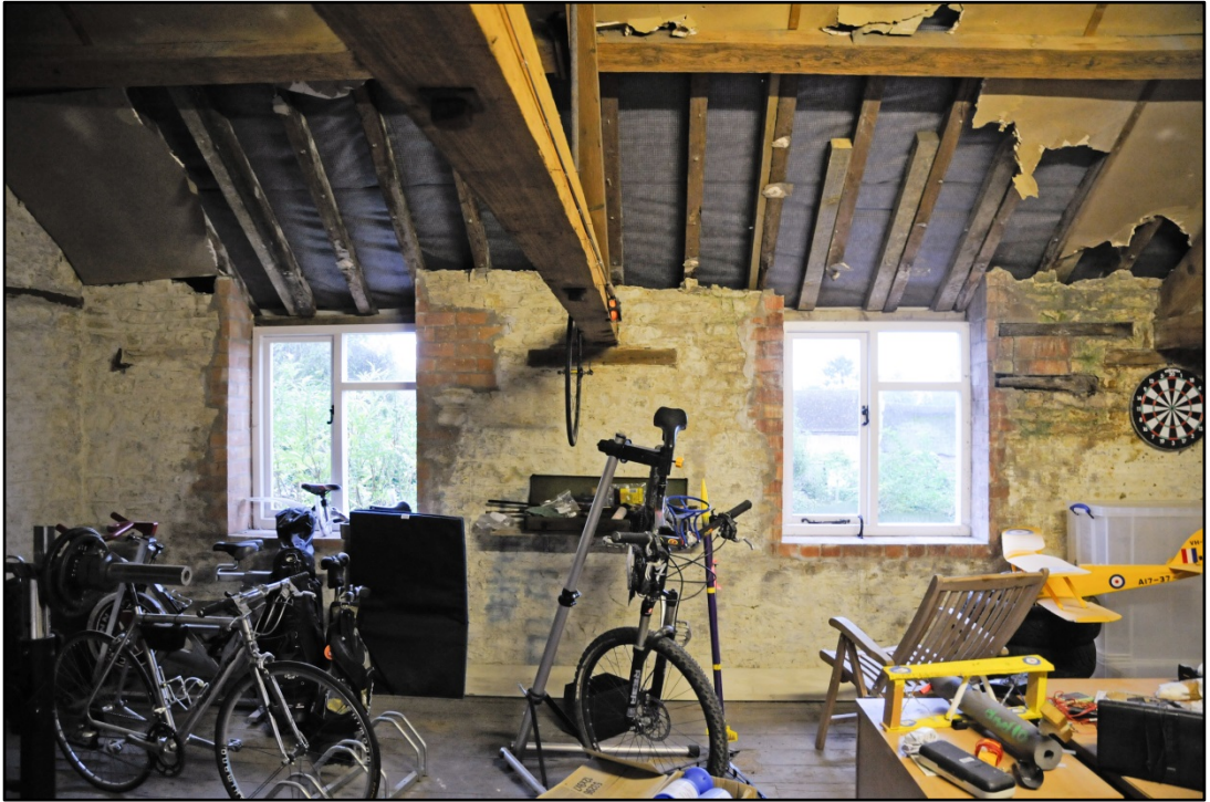
Room F1, modern windows inserted in the south wall Fig 17
