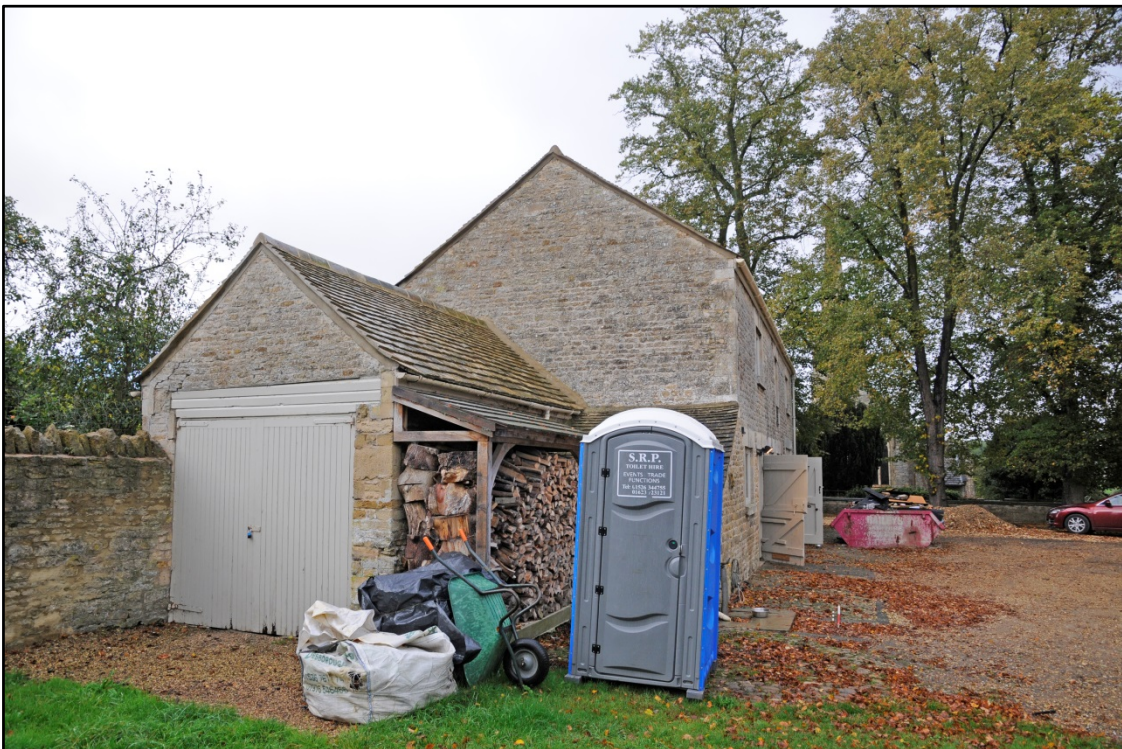
The east elevation and sheds, looking west Fig 8
