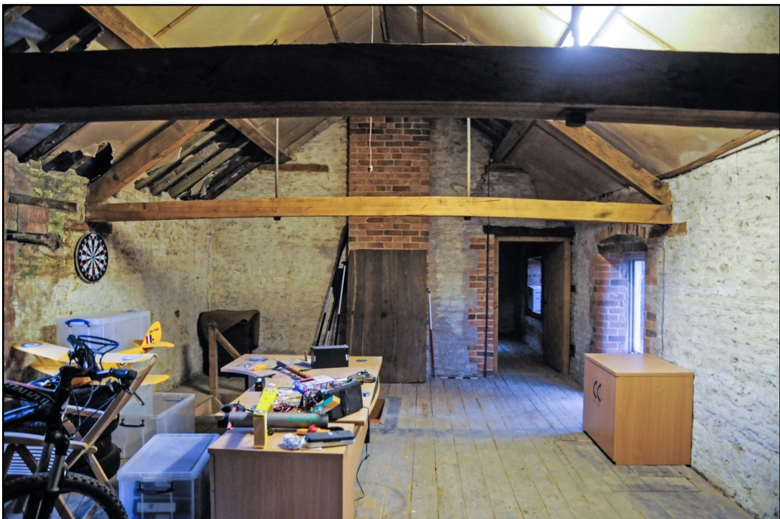
Room F1, looking west Fig 16
