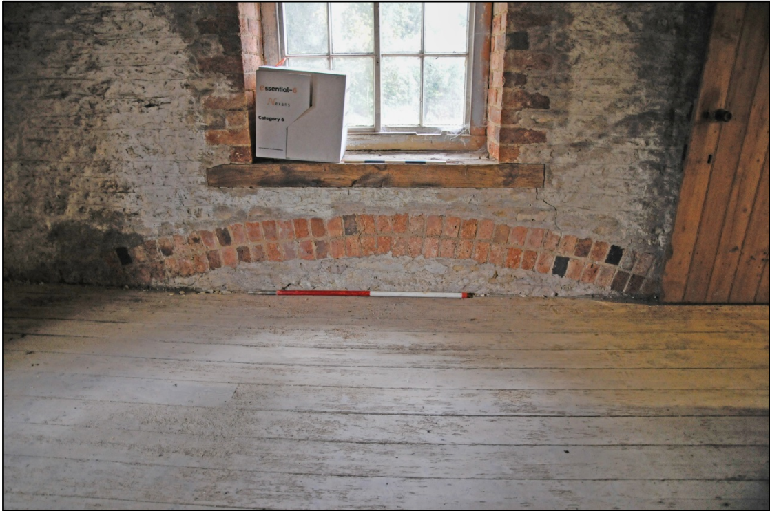
Room F2, brick relieving arch over the coach room door Fig 23
