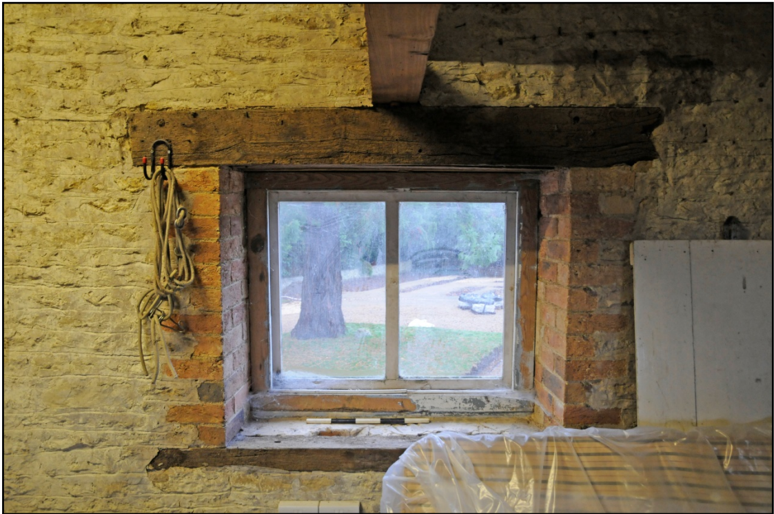
Room F1, detail of window with truss over Fig 19
