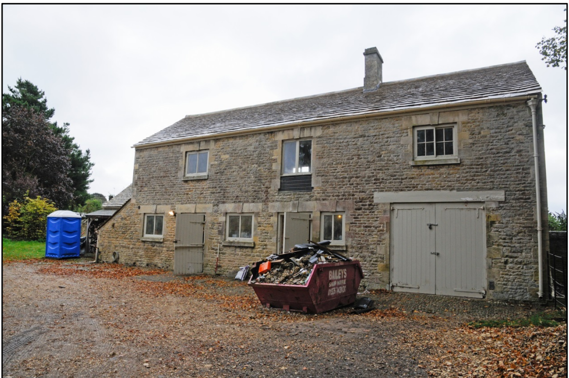
The north elevation, looking south-east Fig 6
