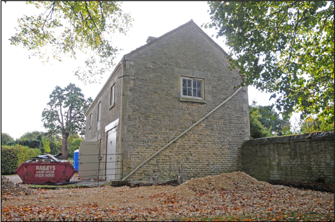
The west elevation, looking east Fig 7
