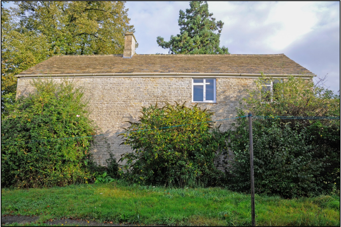
The south elevation, looking north Fig 9
