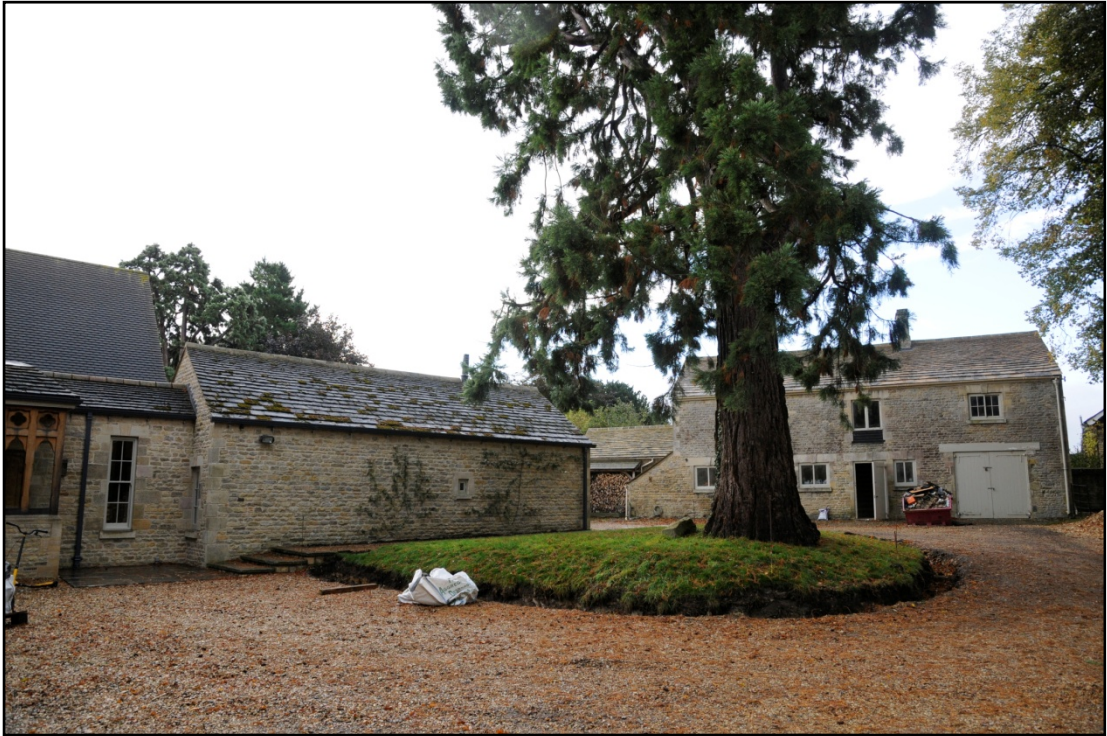
General view of the range in relation to the rectory, looking south Fig 5
