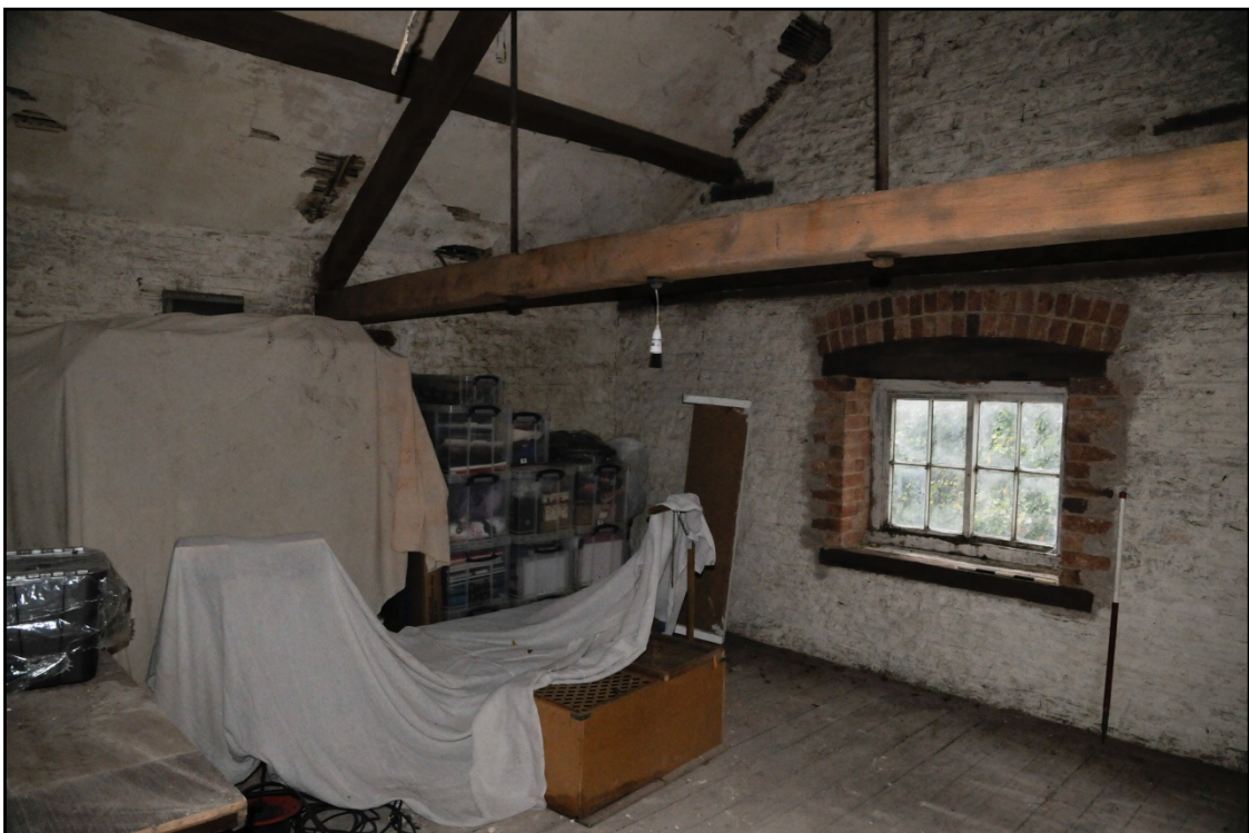
Room F2, looking south-west Fig 20
