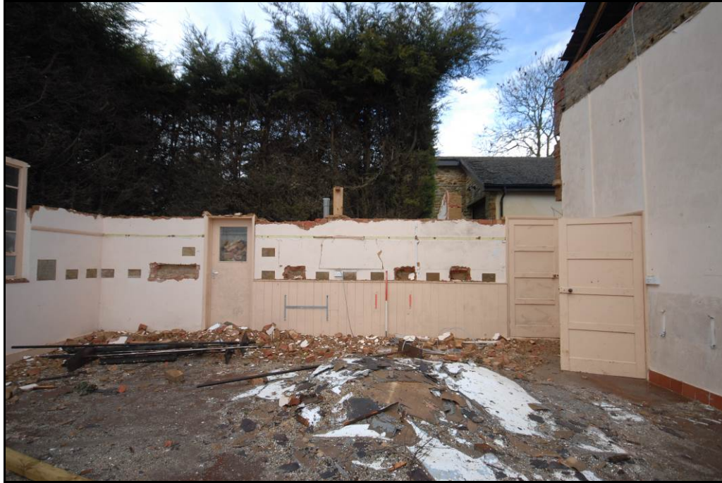
Schoolroom extension, looking north-west Fig 24
