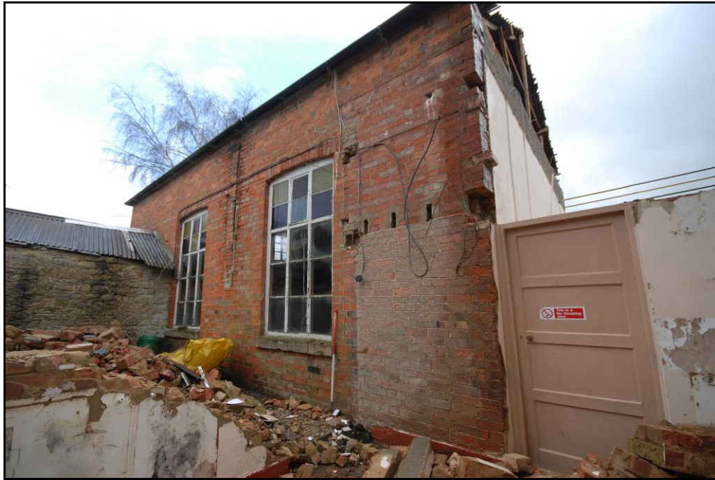
North-west elevation of original building Fig 8
