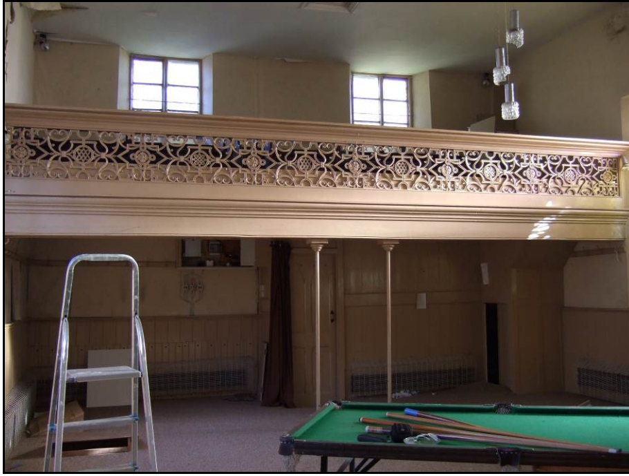
The gallery before removal (R Gulliver) Fig 21
