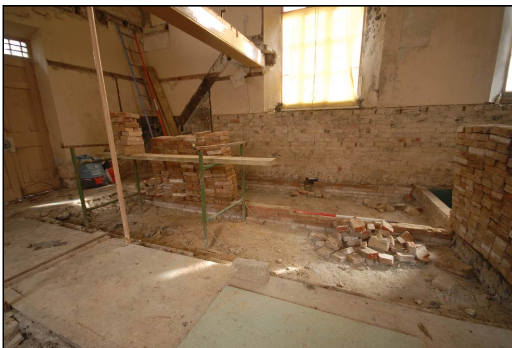
Remnants of original flooring structure Fig 16
