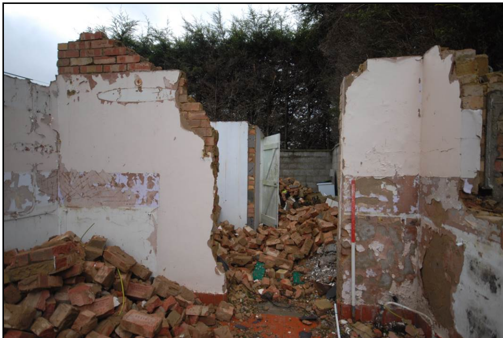
Extension with toilet, looking south-west Fig 27
