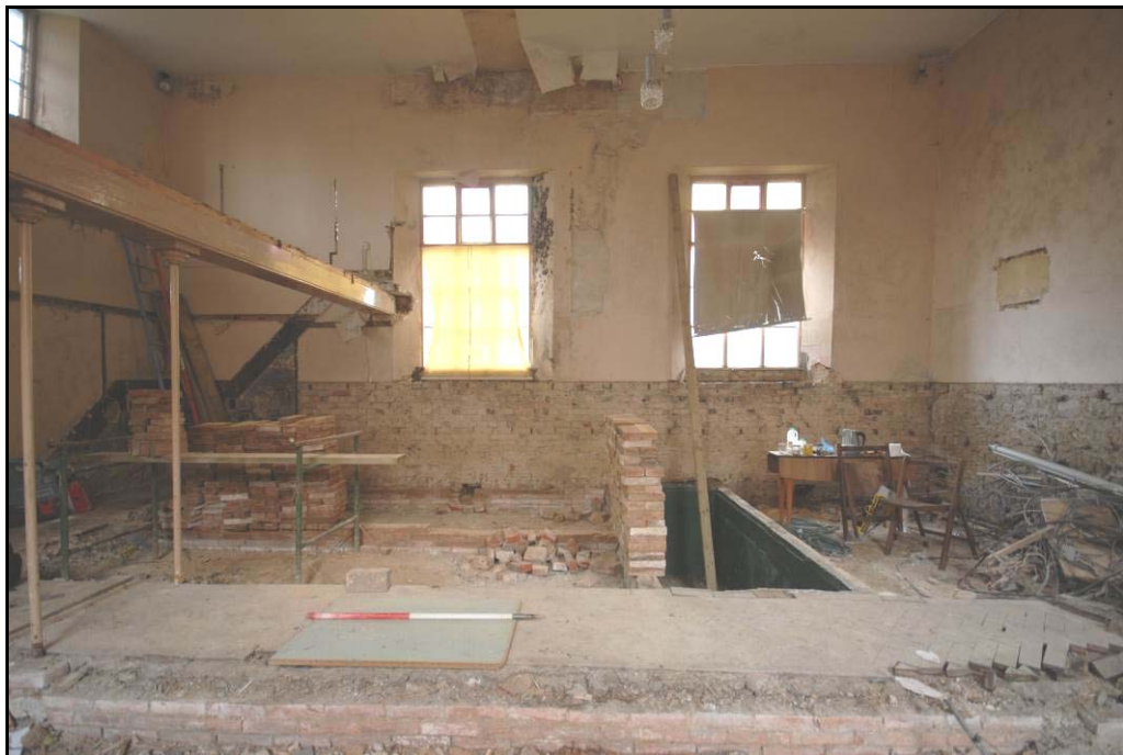
Interior south-east elevation Fig 12
