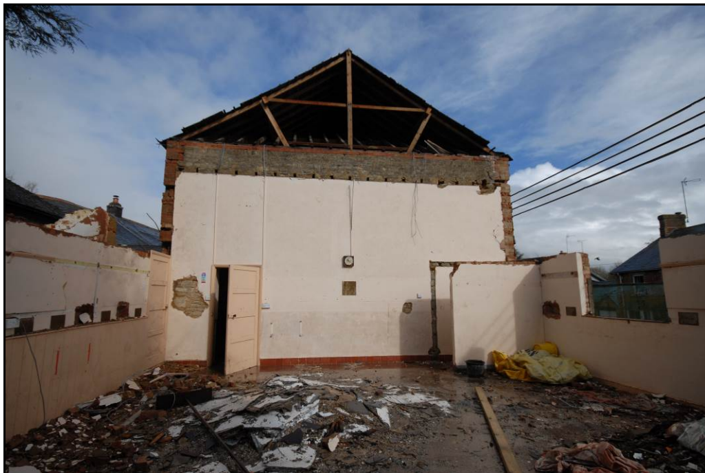
South-west elevation of original building Fig 9
