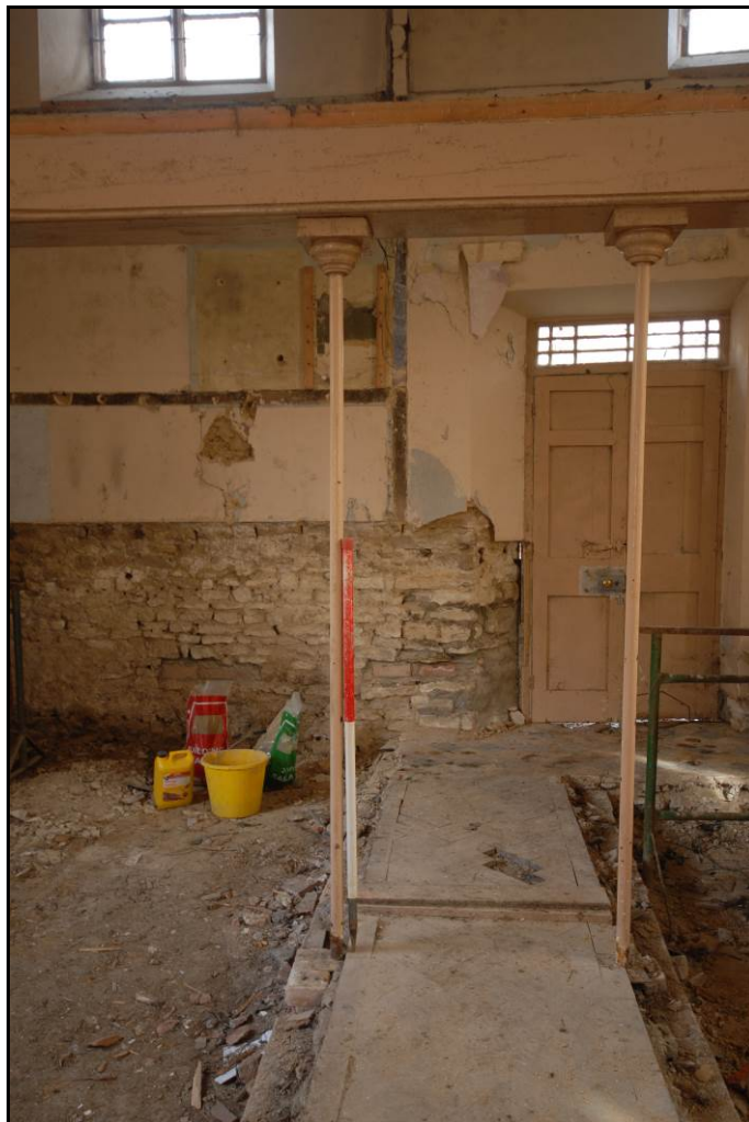
Metal poles supporting the gallery, looking north-east Fig 20
