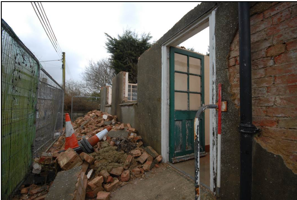
Southern elevation with door, looking north-west Fig 22
