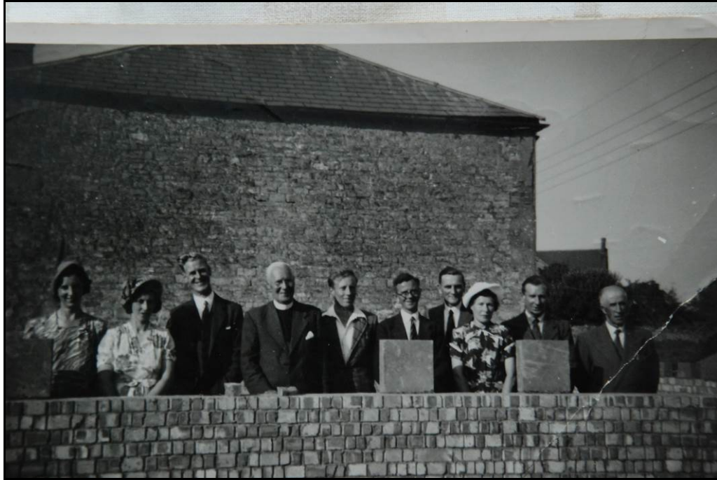
Laying of commemorative stones, 1952 (R Gulliver) Fig 26
