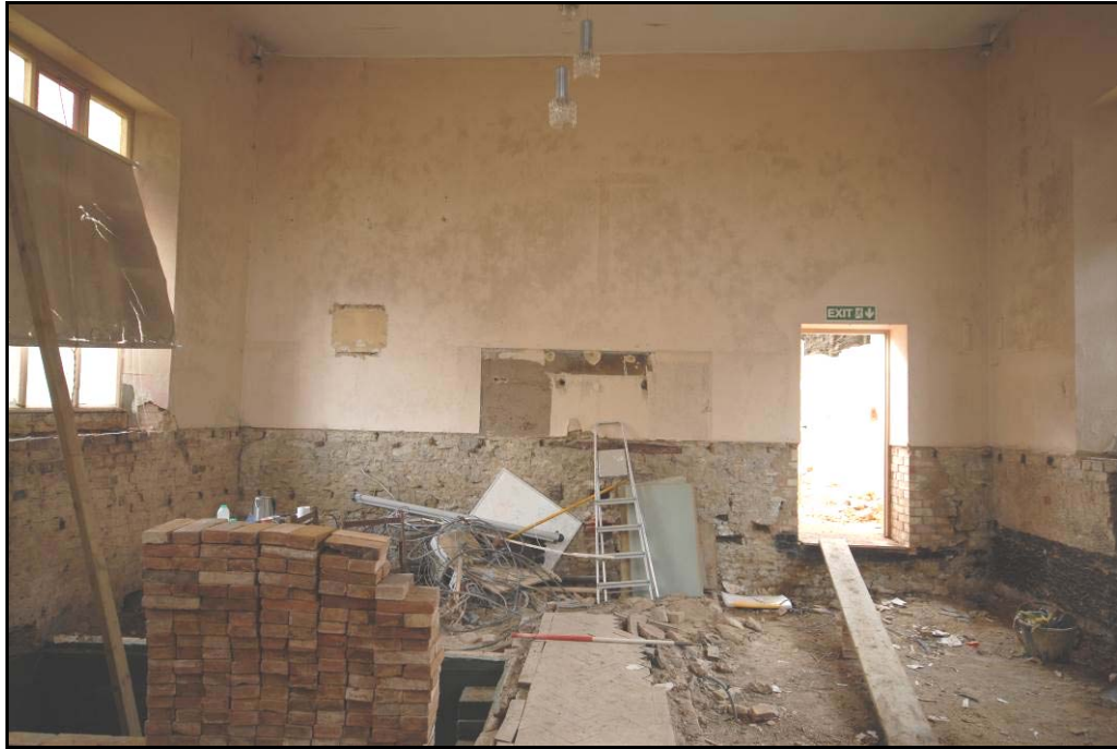
Interior south-west elevation Fig 11
