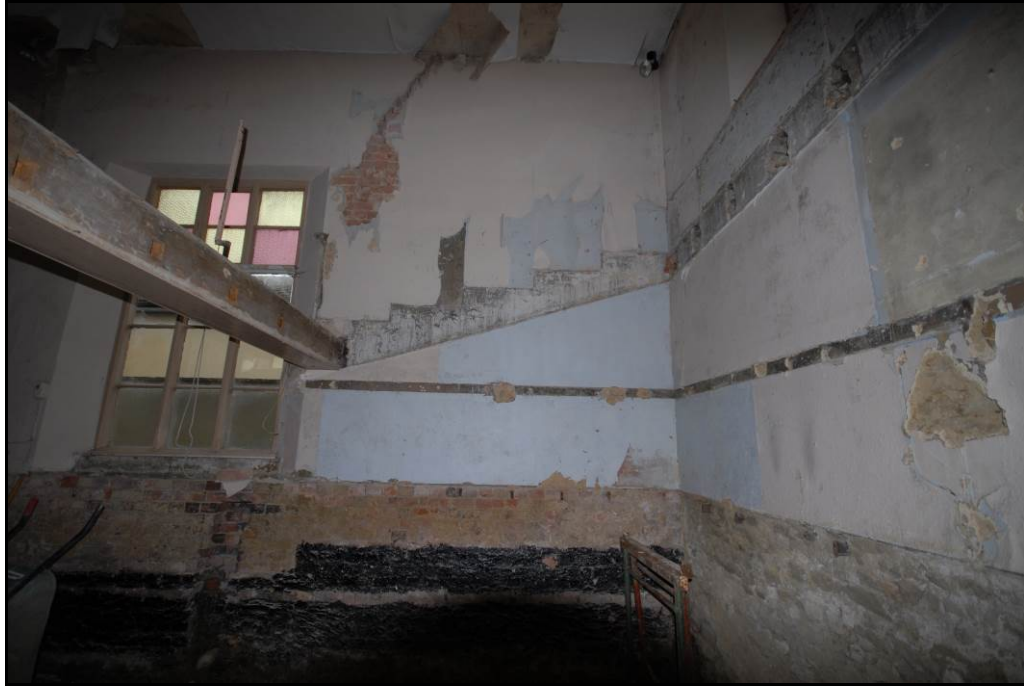
After removal of gallery, looking north Fig 19
