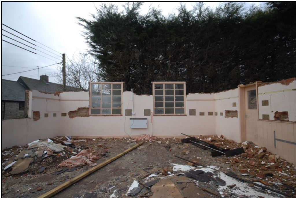
Schoolroom extension, looking south-west Fig 25
