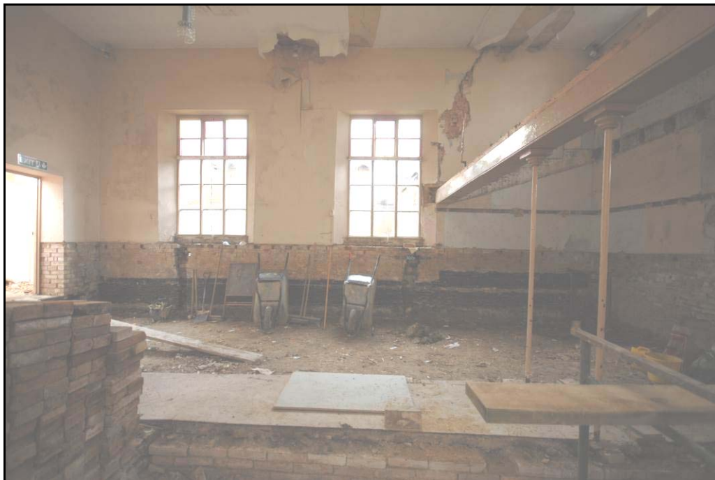
Interior north-west elevation Fig 14
