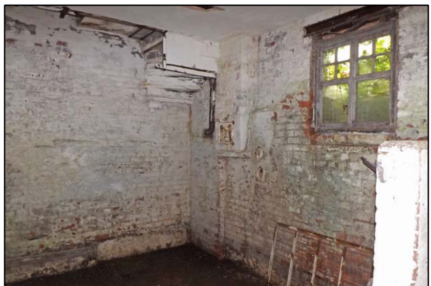
The Bothy cellar, looking west Fig 5.7.21
