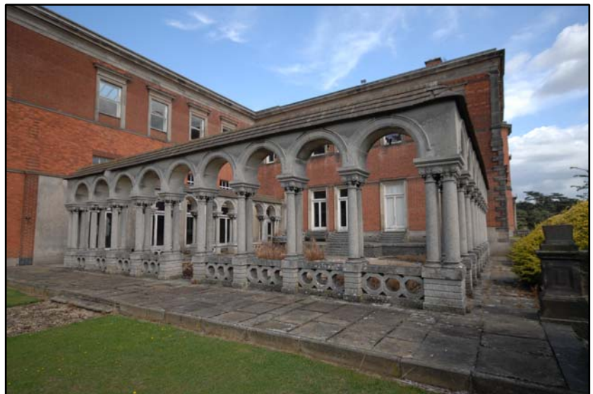
The 1930s arcade with decorative columns Fig 4.1.14
