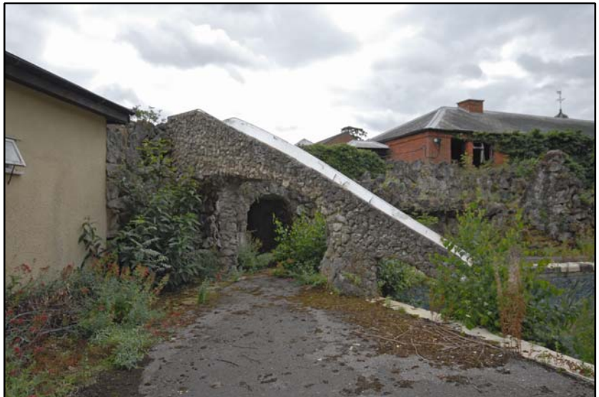
Water slide adjacent to the female changing rooms Fig 5.4.14
