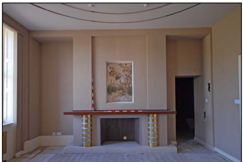
Room F7, the Deco style fireplace Fig 4.5.15
