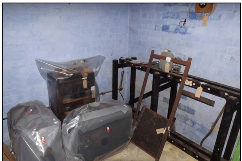
Store room, looking south-east Fig 4.4.32
