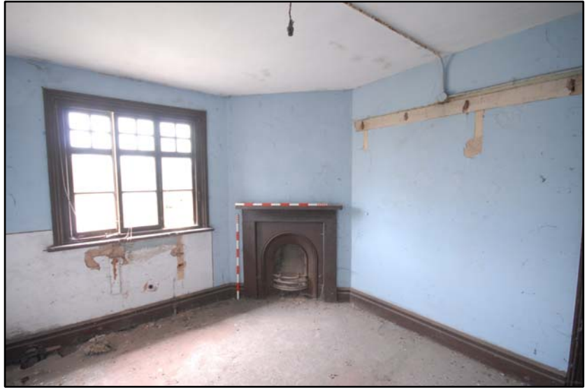
First floor room, looking north Fig 5.7.16
