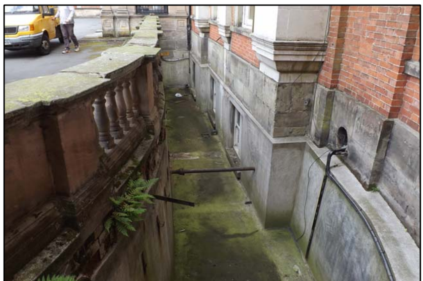
Cellar light wells to the north of the central facade Fig 4.1.9
