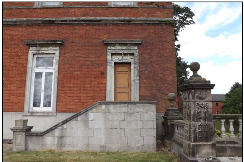
Stair leading to secondary exit of the theatre Fig 4.1.26
