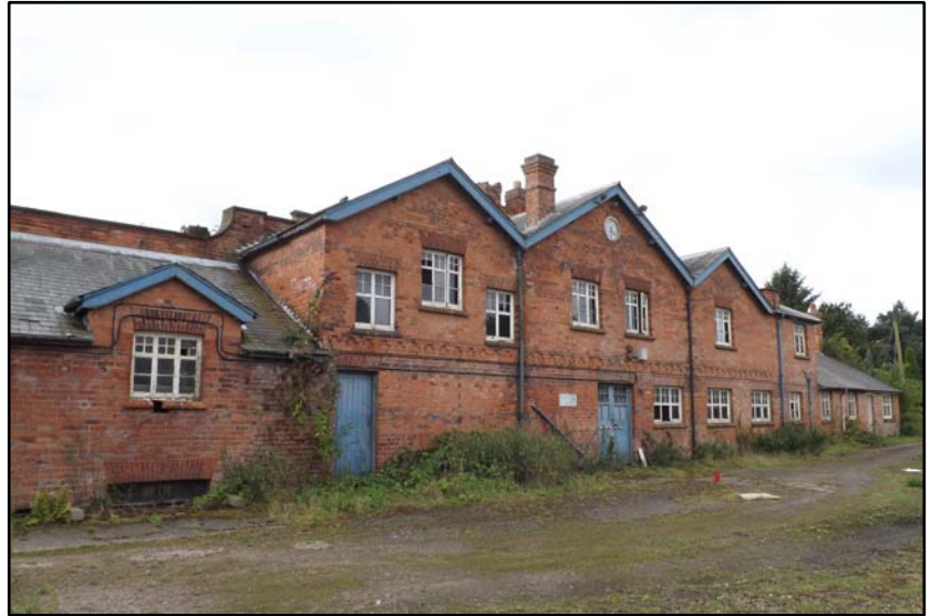
The north elevation of the Bothy, looking south-west Fig 5.7.1
