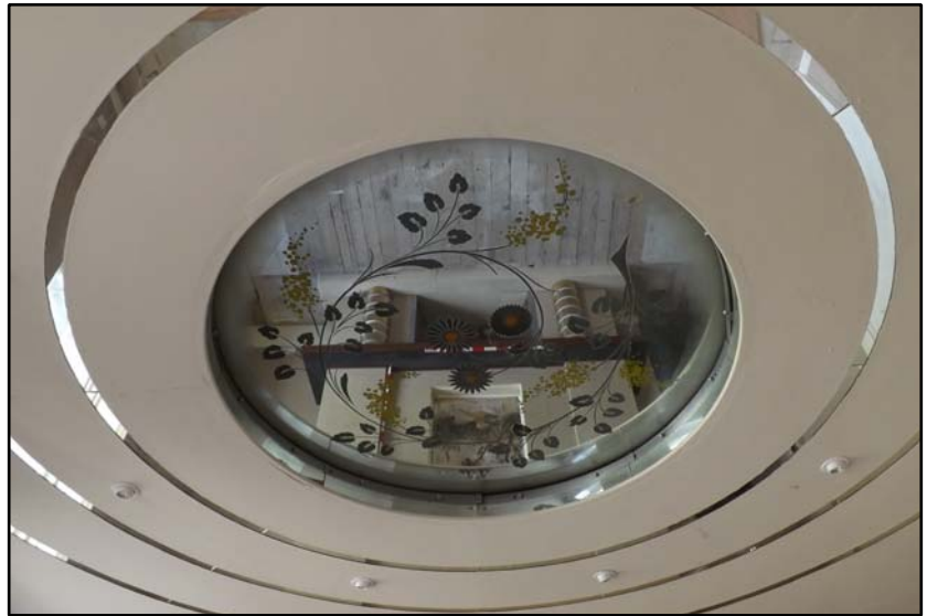
Room F7, detail of the ceiling mirrors Fig 4.5.16
