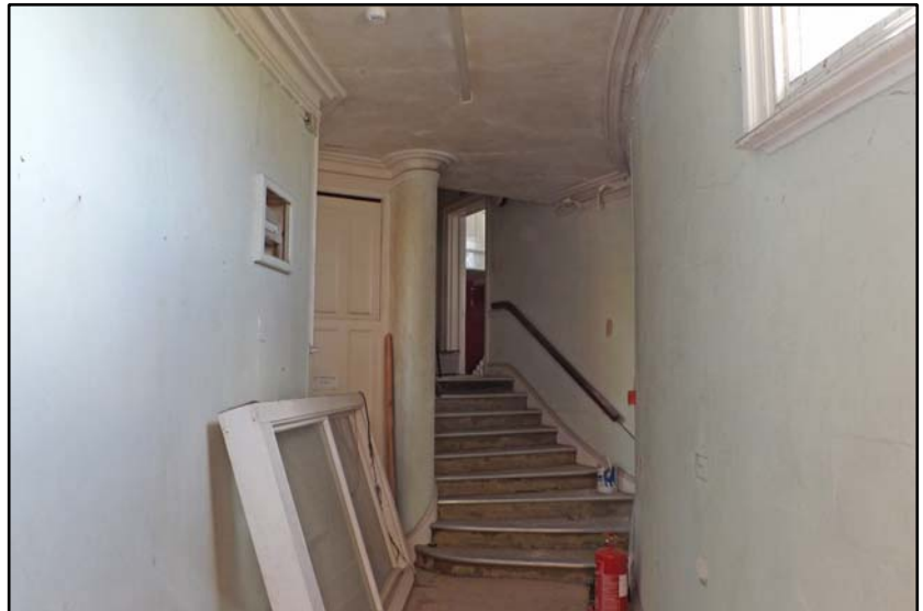
The corridor between the hall and the west wing, F15 Fig 4.5.48
