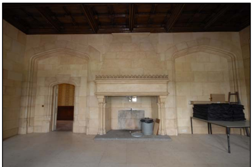
Room G8, the south elevation with central fireplace Fig 4.3.27
