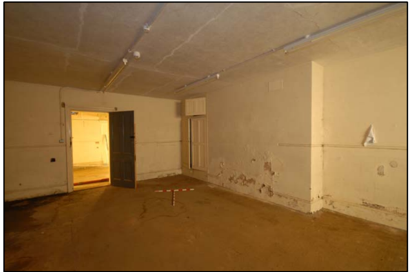
Large room adjacent to the former chapel Fig 4.2.10
