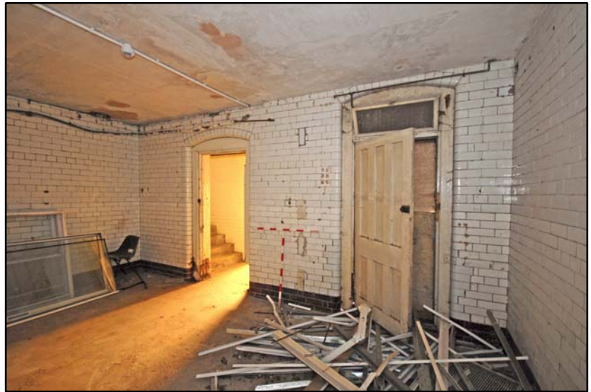
Cold storage room with stairs leading to the kitchens Fig 4.2.7
