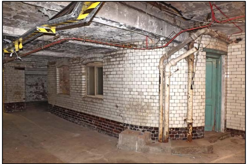
Workshop and store room Fig 4.2.19
