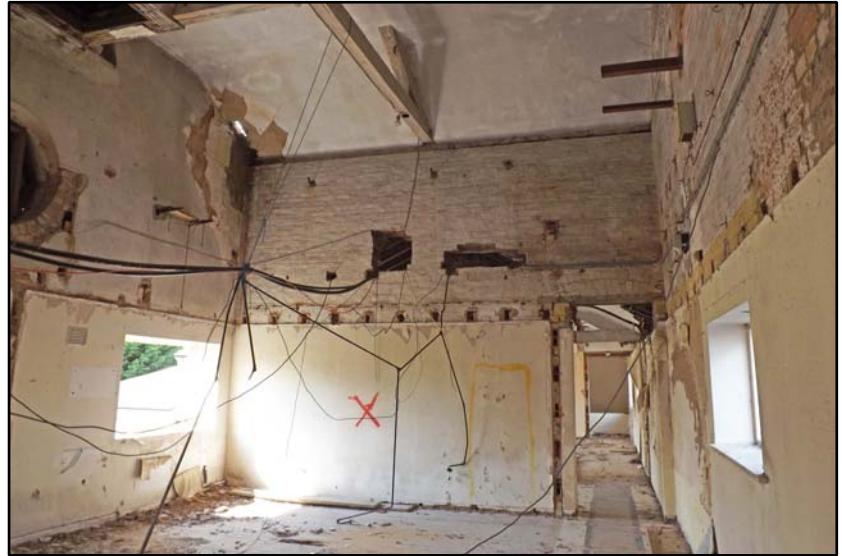
Former joist slots below the cupola Fig 5.1.16
