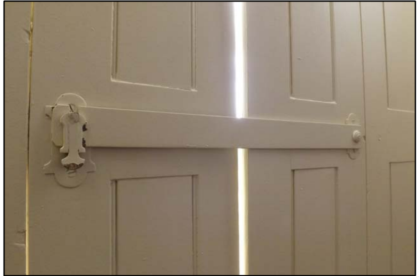
Detail of window shutter lock Fig 4.3.13
