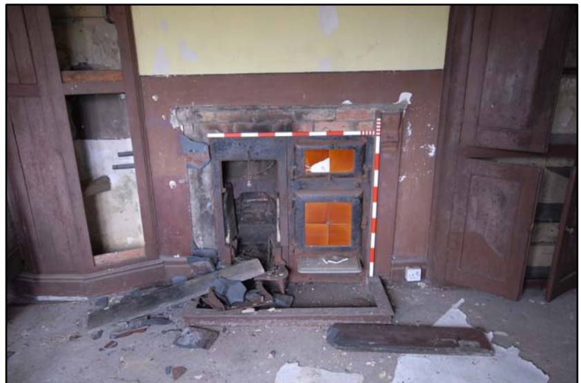
Detail of the kitchen range Fig 5.7.14
