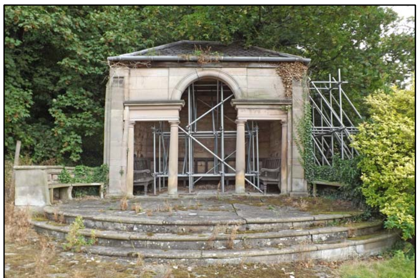
The main facade of the Pavilion, looking east Fig 5.5.3
