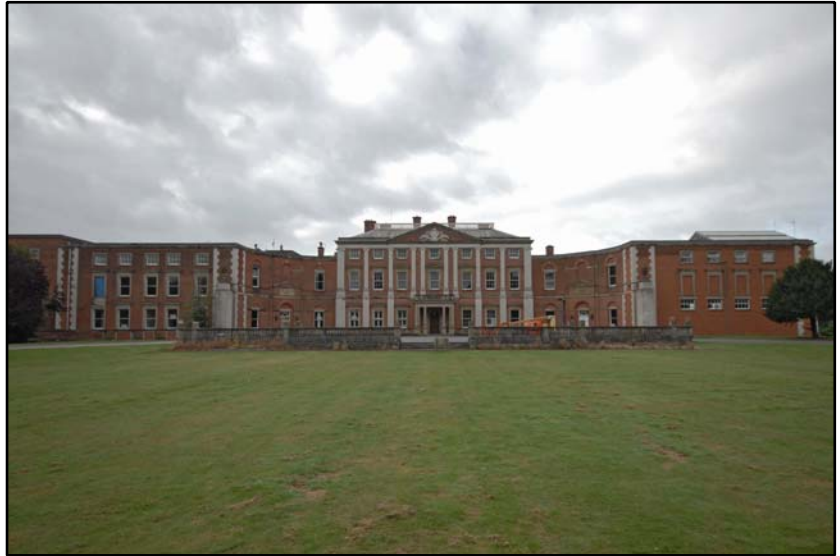
The exterior, looking south Fig 4.1.1
