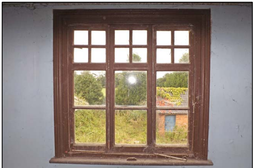
Detail of window at first floor Fig 5.7.18
