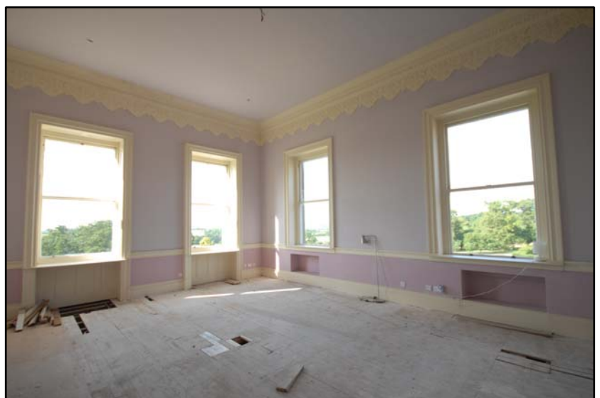
Room F3, looking south-west Fig 4.5.9
