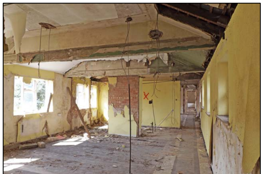
View of the first floor, looking north Fig 5.1.15
