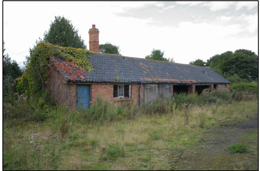
The Long Shed, looking north-west Fig 5.9.1
