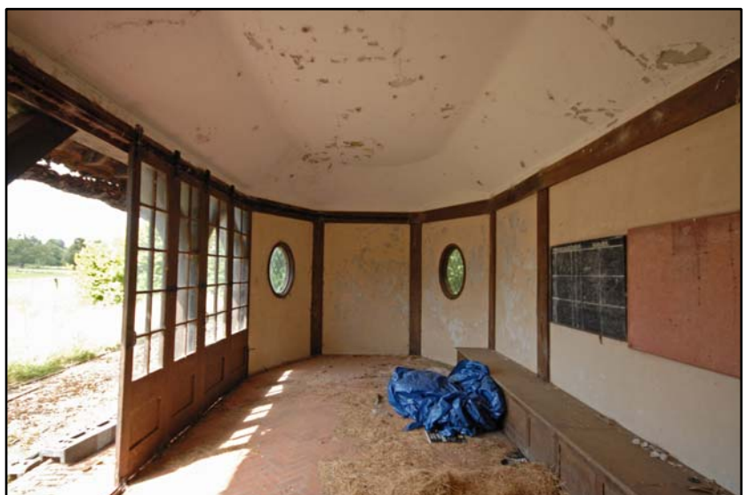
Interior of the pavilion, looking north Fig 5.2.6
