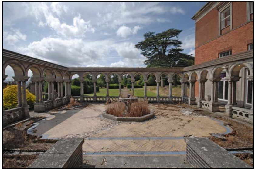
The arcade, looking west Fig 4.1.16
