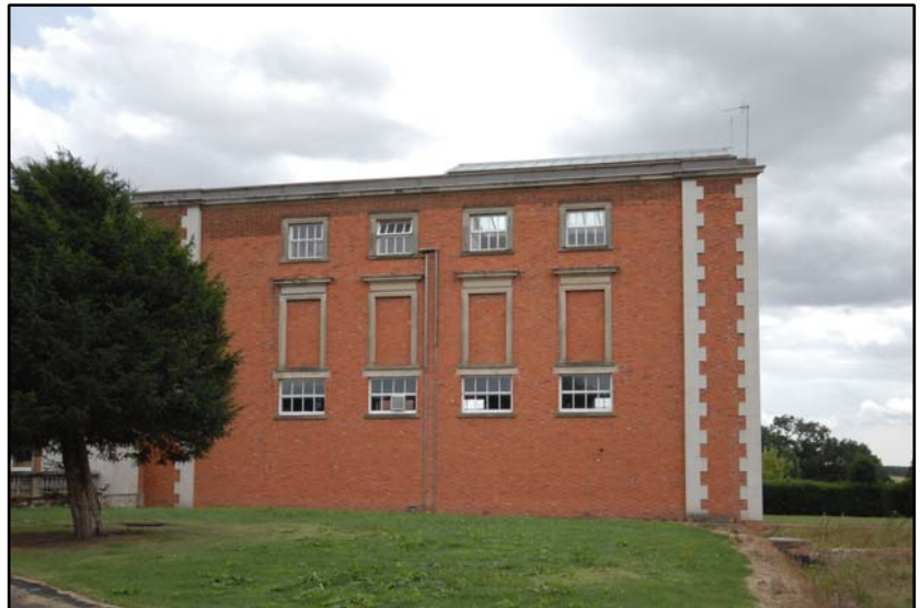
The east wing, looking south Fig 4.1.11
