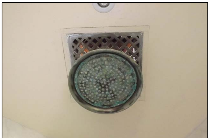
Room F14, detail of shower head Fig 4.5.44
