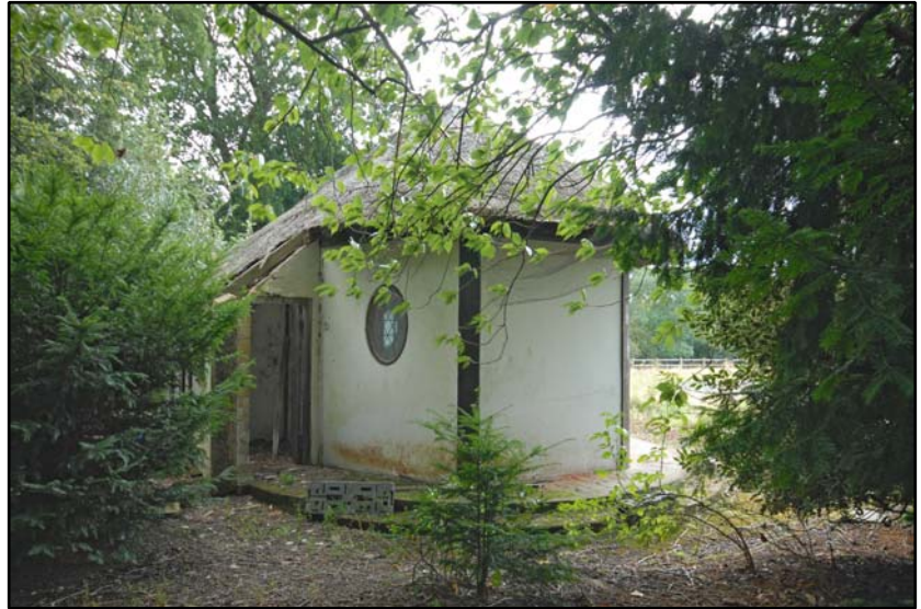
The north elevation with entrance to the rear toilet Fig 5.2.4
