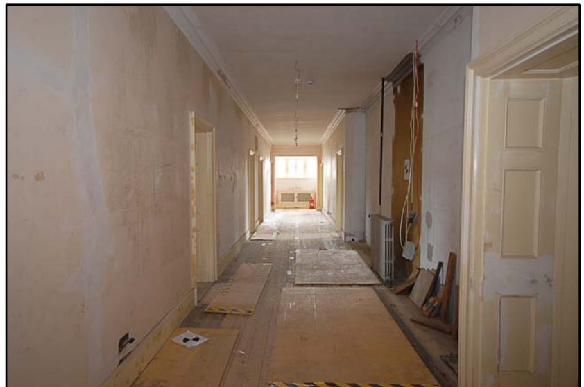
The central corridor, looking east Fig 4.6.2
