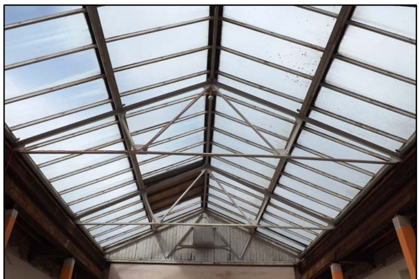
Room F1, detail of the steel frame roof Fig 4.5.3
