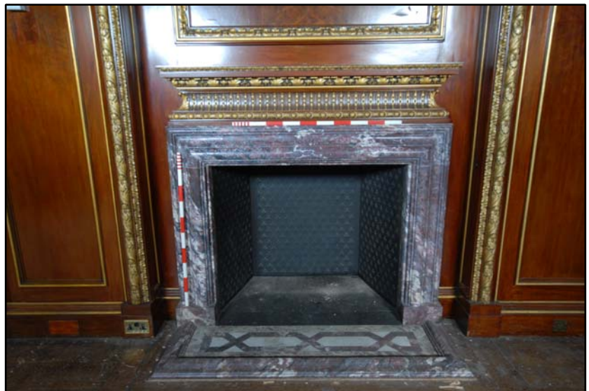
Room G4, detail of the fireplace Fig 4.3.17
