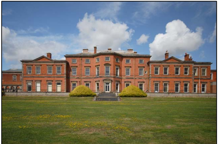
The central elements of the southern elevation, looking north Fig 4.1.20
