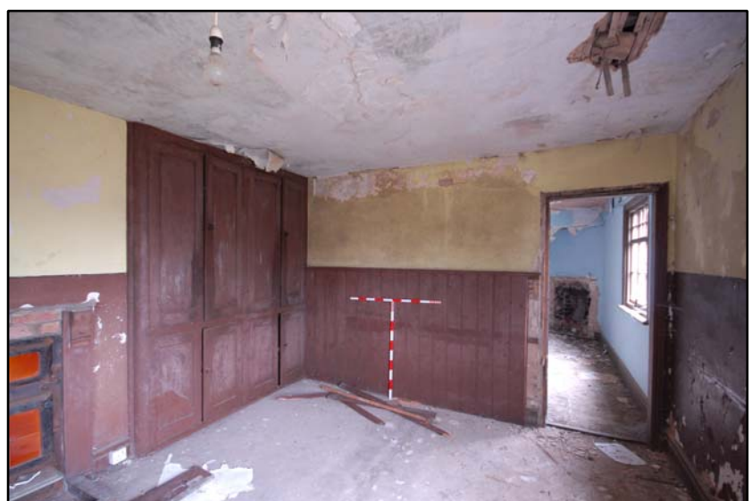
First floor head gardeners' kitchen, looking west Fig 5.7.15
