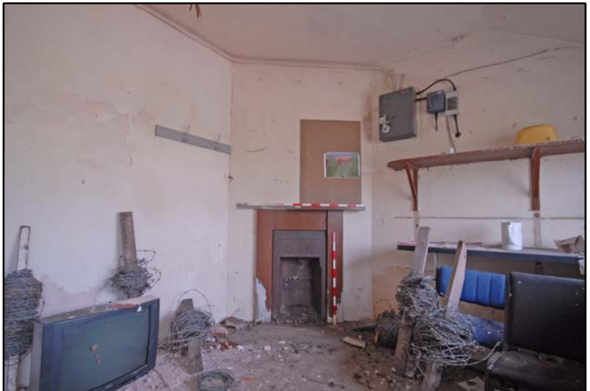
Interior of the western extension Fig 5.7.8
