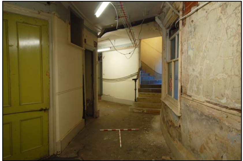
The cellar landing with stairs up Fig 4.2.1
