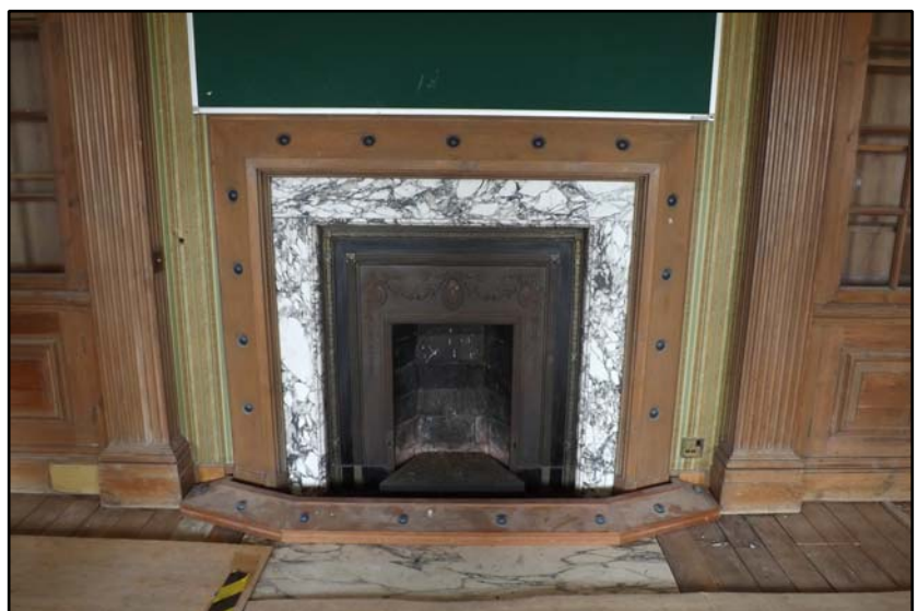
Room S2, detail of the fireplace Fig 4.6.9
