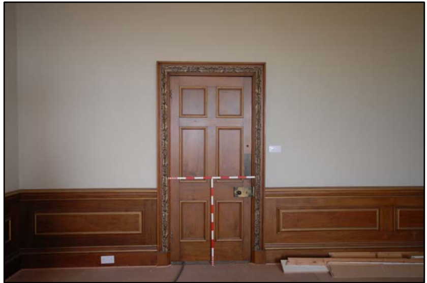
Room F12, detail of the door, looking north Fig 4.5.36
