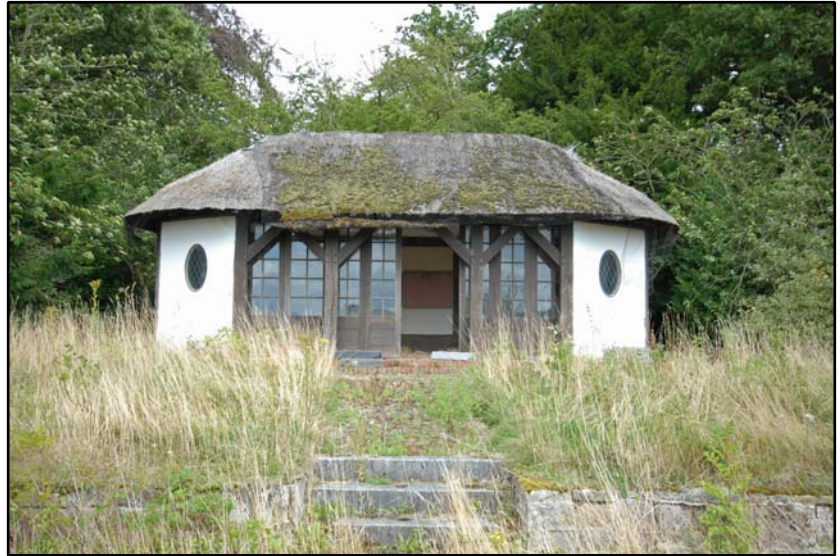
The main, west elevation of the tennis pavilion Fig 5.2.1
