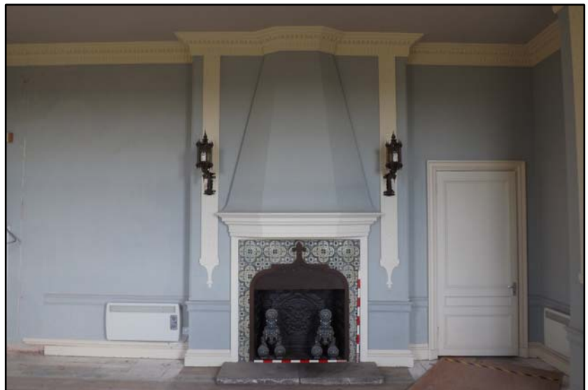
Room F11, the north elevation Fig 4.5.31
