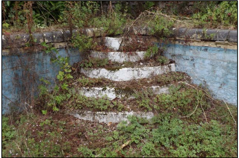
Concentric steps in the western shallow end of the pool Fig 5.4.13
