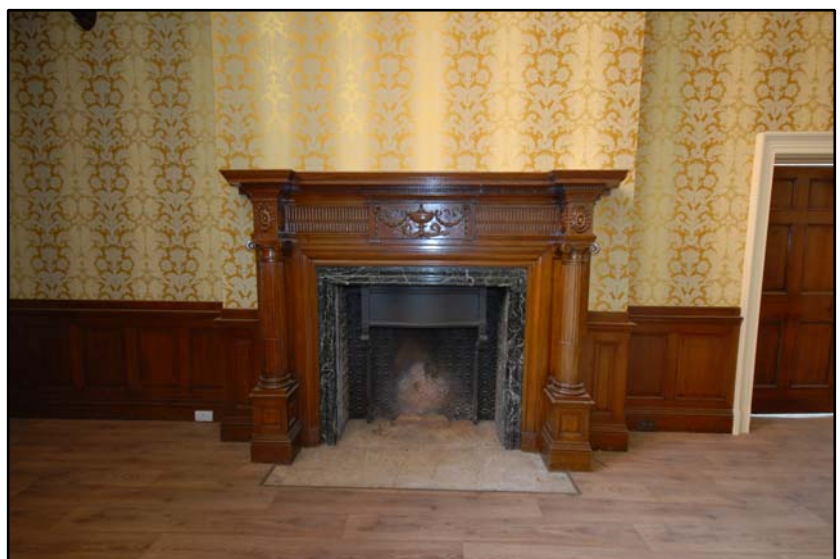
Fireplace adjacent to the stair landing and room G10 Fig 4.3.44
