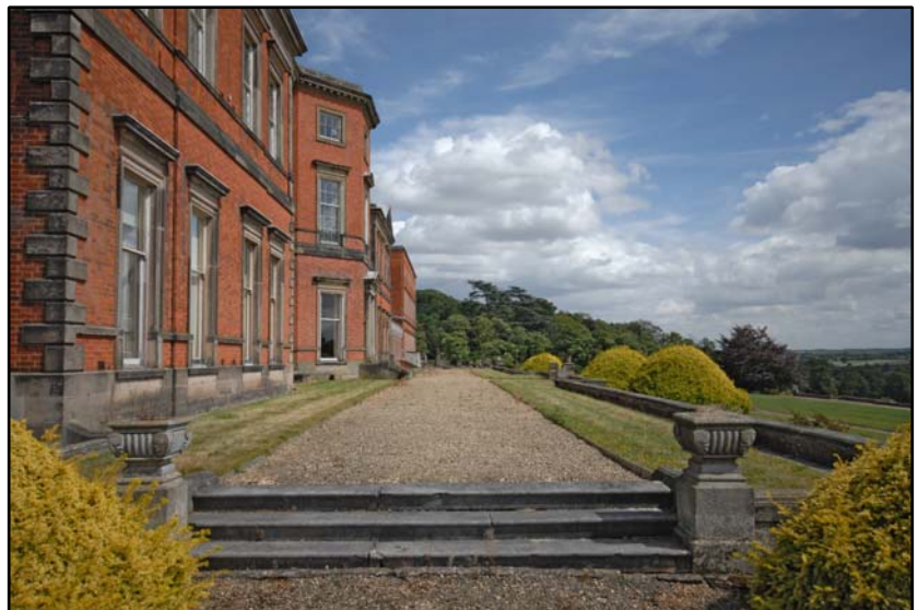
View along the southern path, looking north-east Fig 4.1.17
