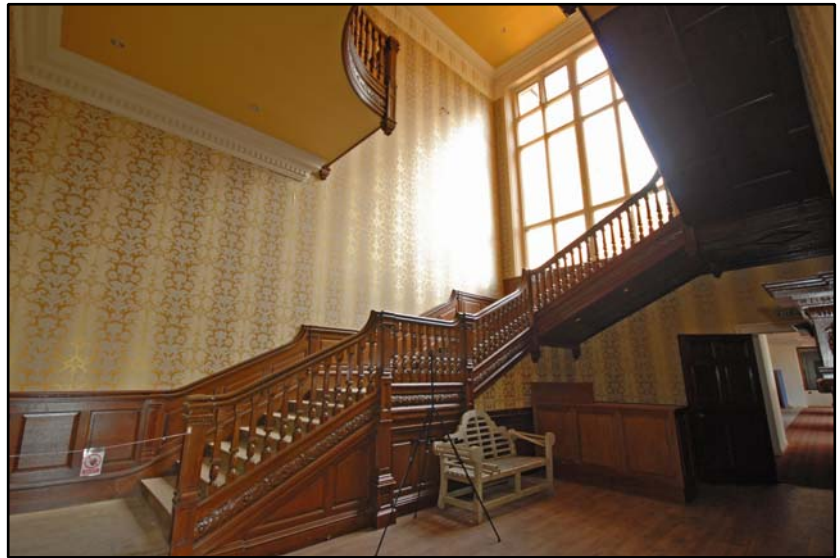
The main stair, ground floor landing Fig 4.3.42
