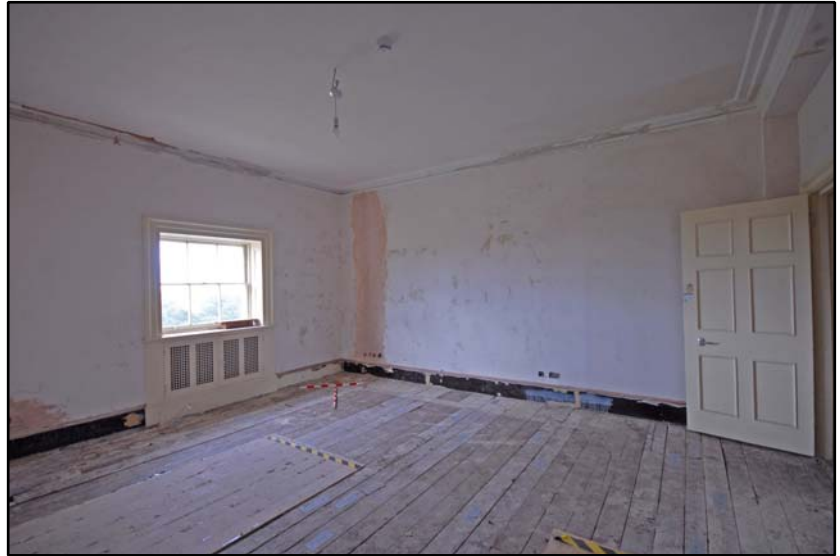
Room S3, looking south-west Fig 4.6.10
