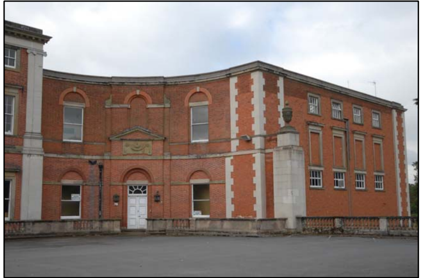
The west wing, looking south-west Fig 4.1.10
