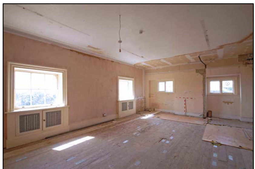
Room S2, looking south-west Fig 4.6.3
