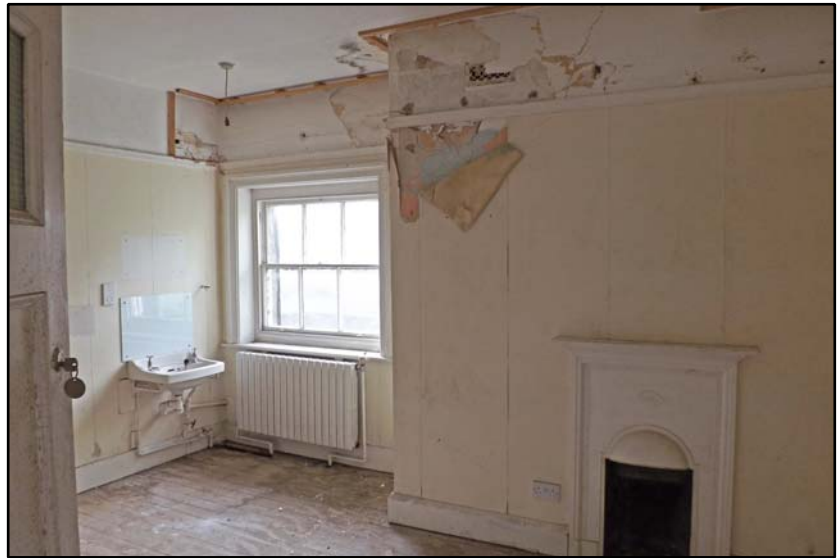
Example of the rooms in S11 Fig 4.6.22
