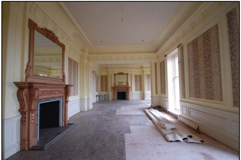
Room G9, looking east Fig 4.3.32
