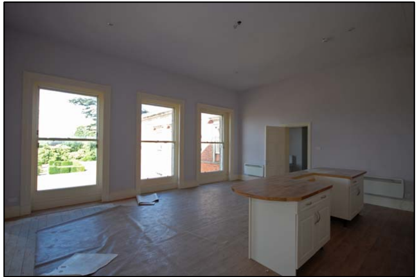
Room F2, looking north-west Fig 4.5.4
