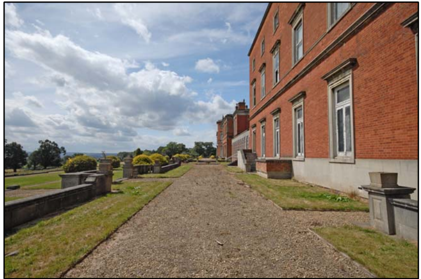
View along the southern path, looking south-west Fig 4.1.25
