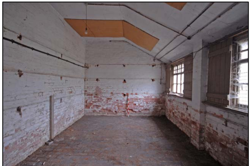
Interior of the potting shed, looking west Fig 5.7.11
