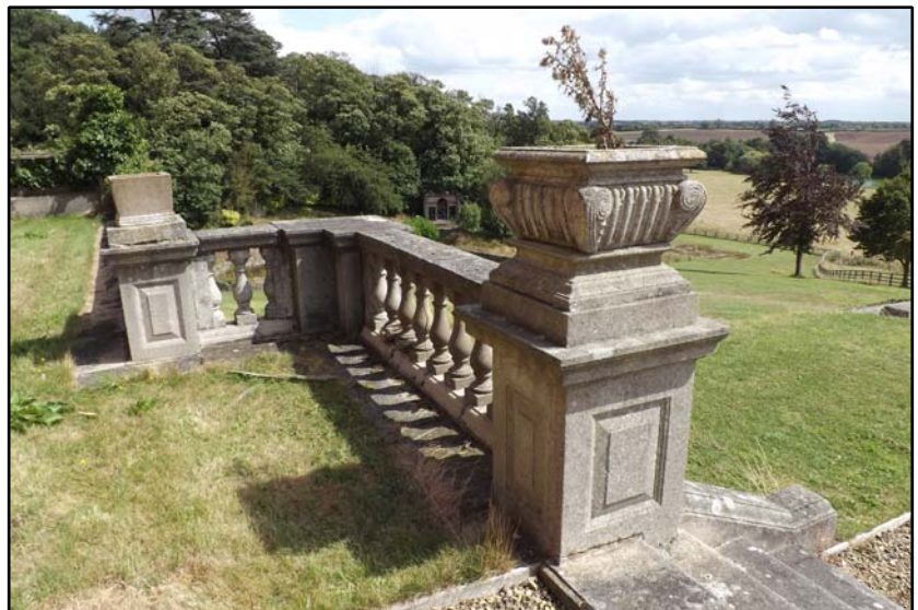
The decorative elements of the southern garden wall Fig 4.1.29
