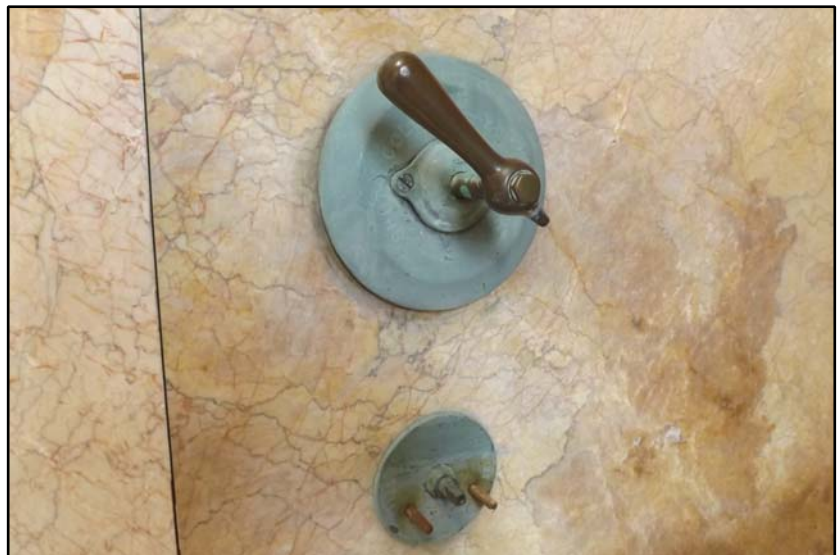
Room F14, detail of original tap fittings Fig 4.5.43
