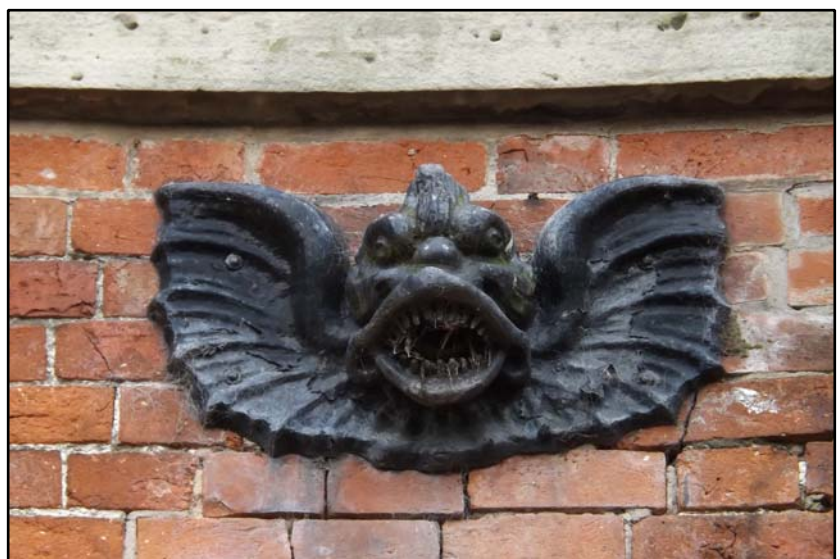
Gargoyle on the north face of the east wing Fig 4.1.6
