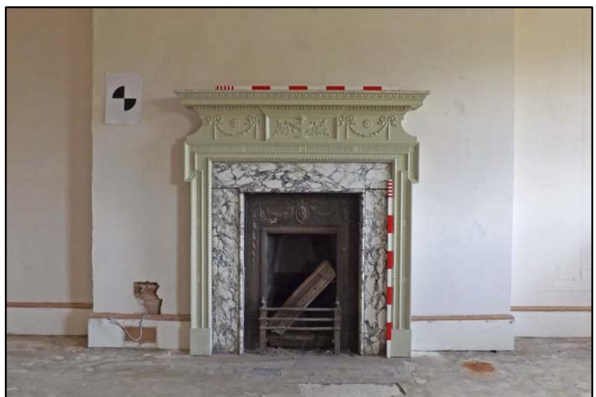
Room S8, detail of the fireplace Fig 4.6.18
