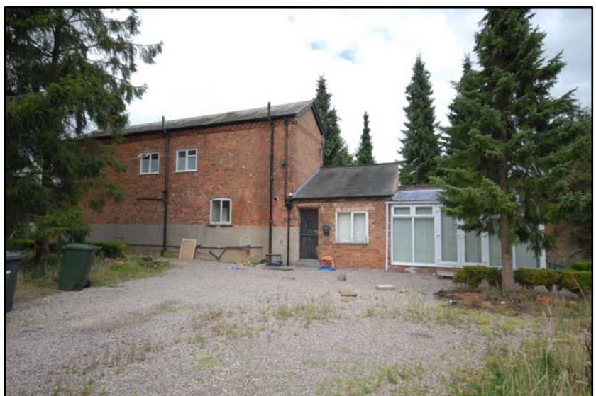
The west elevation of the cottage, looking east Fig 5.6.12
