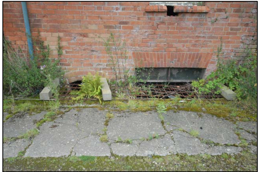
Light wells and former stair to Bothy cellar Fig 5.7.19
