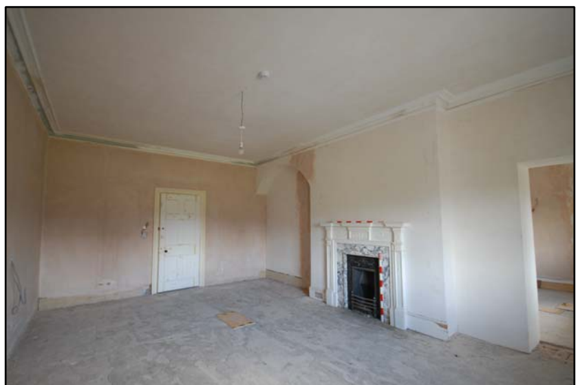
Room S7, looking south-west Fig 4.6.15
