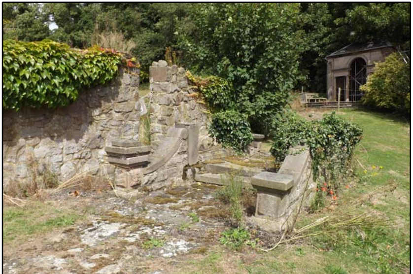
The footbridge south of the sea lion pool Fig 5.5.8
