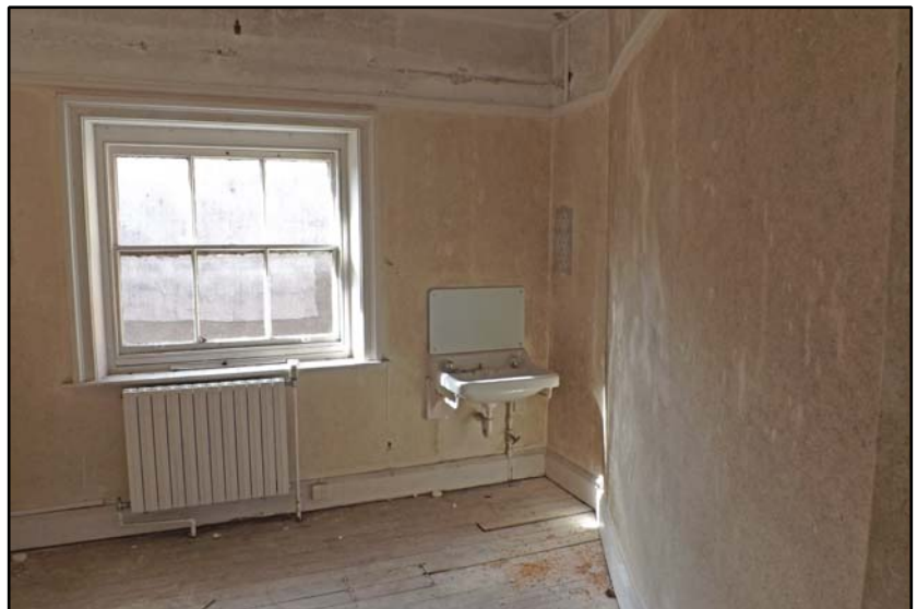
Example of the rooms in S11 Fig 4.6.23
