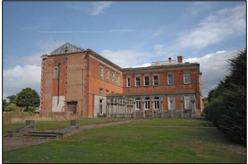
The east wing and arcade, looking north-east Fig 4.1.13
