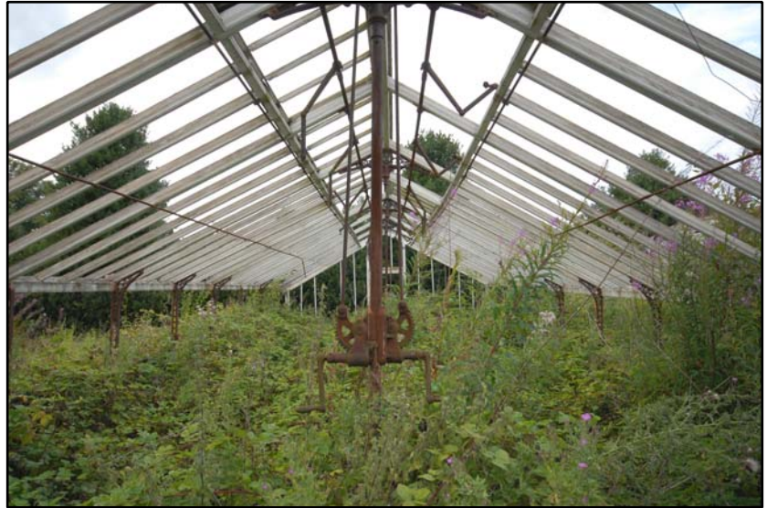
The interior of Greenhouse 1 Fig 5.8.4
