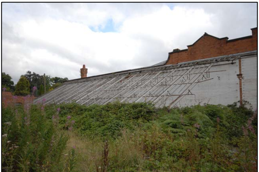
The former peach house, looking north-west Fig 5.6.6
