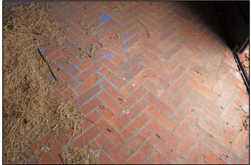
Detail of the brick, herringbone pattern floor Fig 5.2.10
