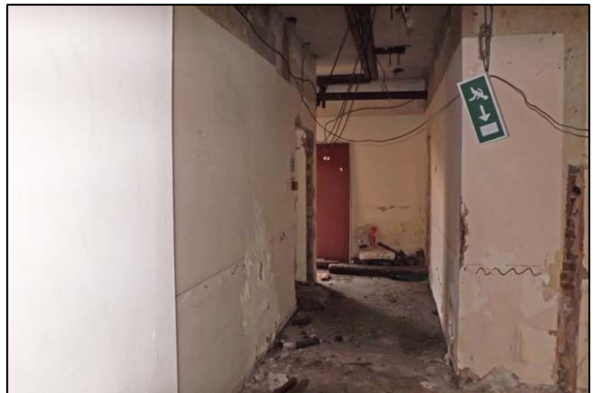
Interior of the south wing Fig 5.1.14
