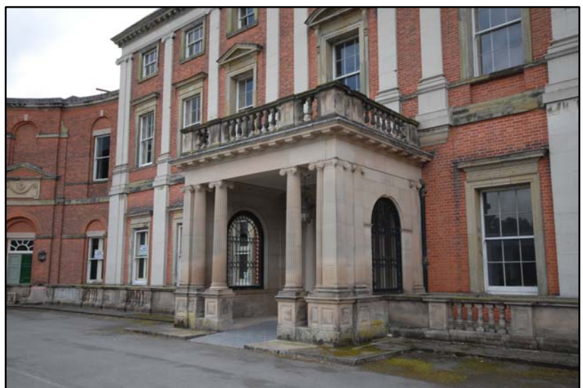
The north porch Fig 4.1.3
