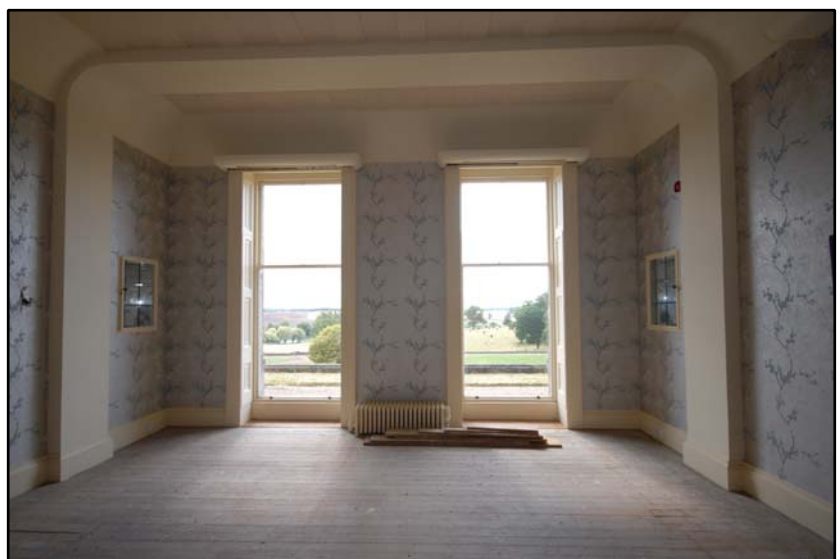
Room G10, looking south Fig 4.3.36
