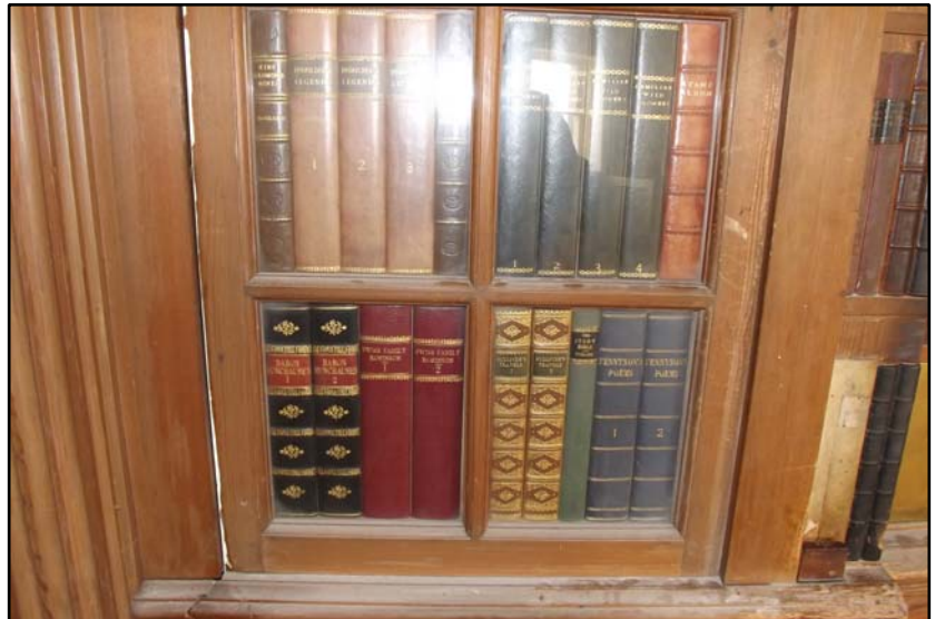
Room S2, detail of fake books with concealed door latch at bottom right Fig 4.6.7
