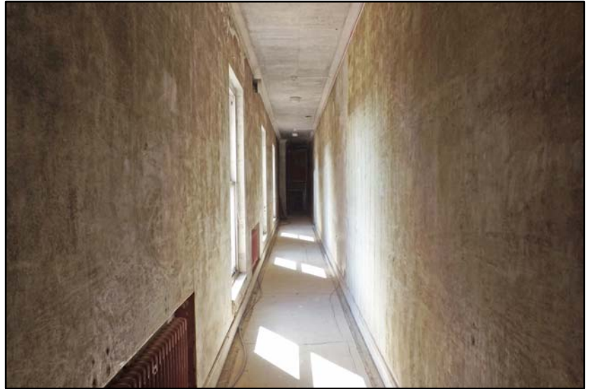
The access corridor between the Hall and Projector Suite, F16 Fig 4.4.27
