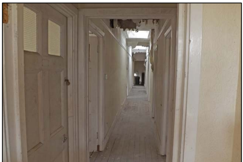
The central corridor of S11, looking east Fig 4.6.21
