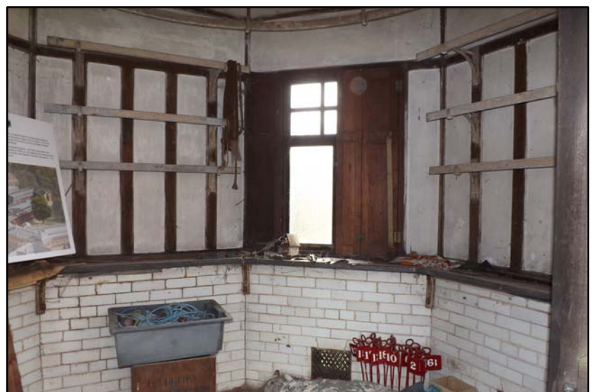
The interior, looking north-east Fig 5.3.3
