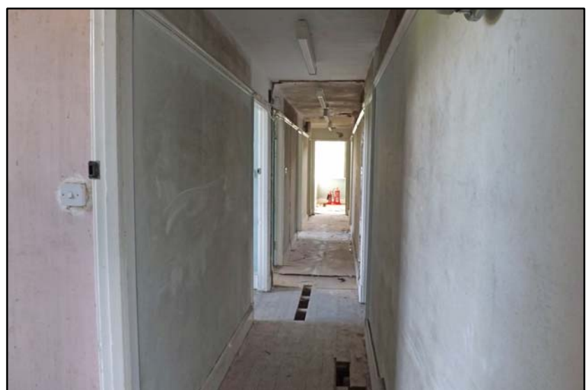
The central corridor of the west wing, F15, looking east Fig 4.5.50
