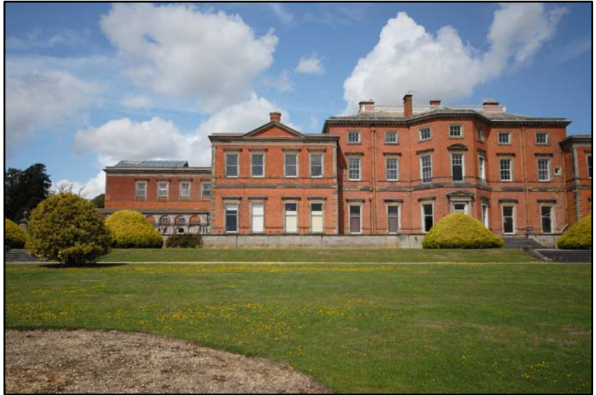
The eastern extent of the south elevation, looking north Fig 4.1.19
