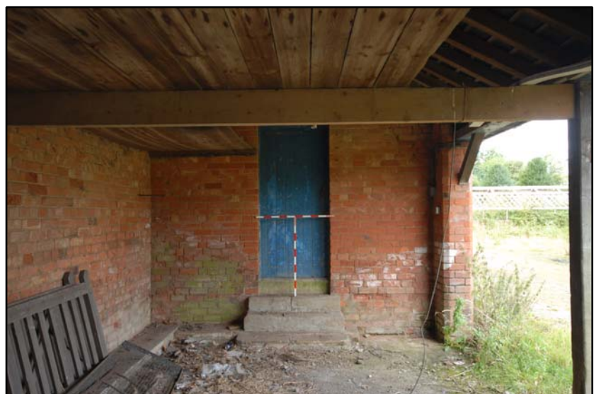
The eastern shed, looking west Fig 5.7.6
