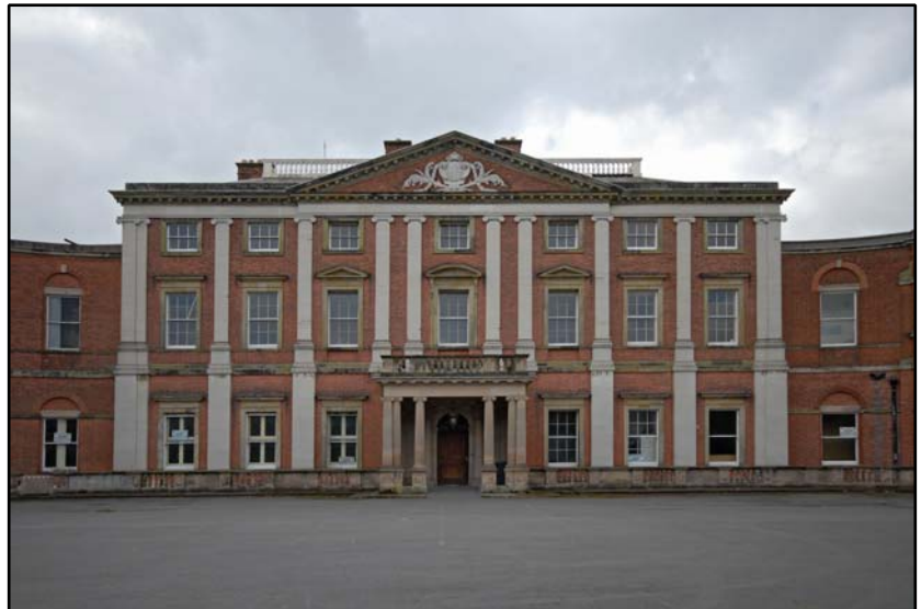
The central facade, looking south Fig 4.1.2
