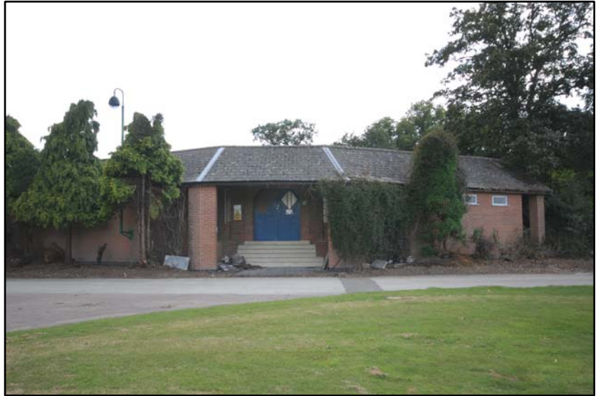
The main frontage of the Lido, looking south-west Fig 5.4.1
