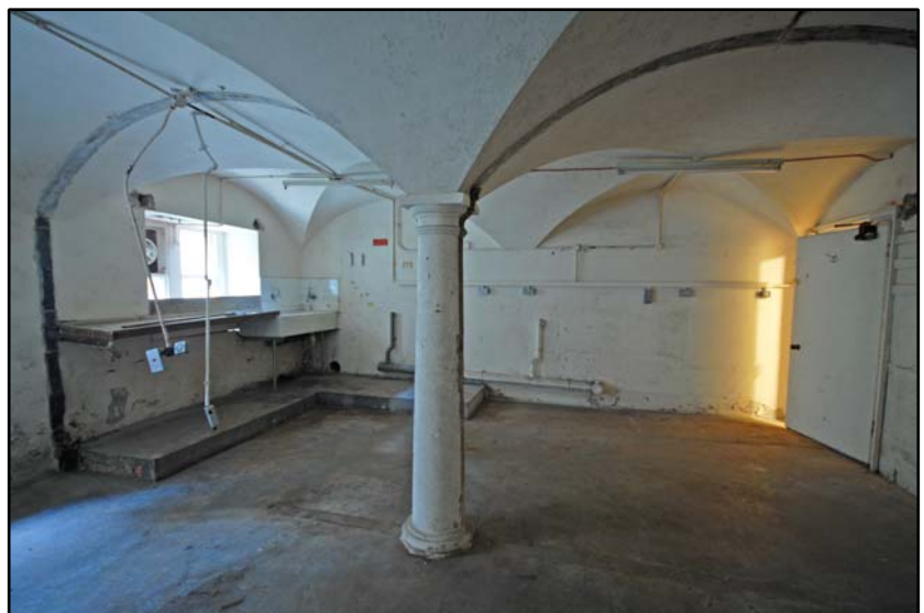
The cellar washroom Fig 4.2.14
