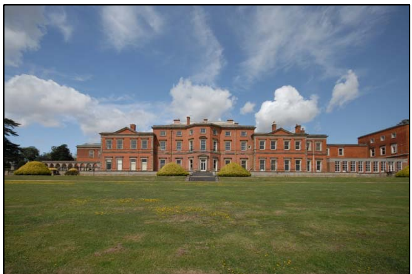
View of the south facing elevation, looking north Fig 4.1.18
