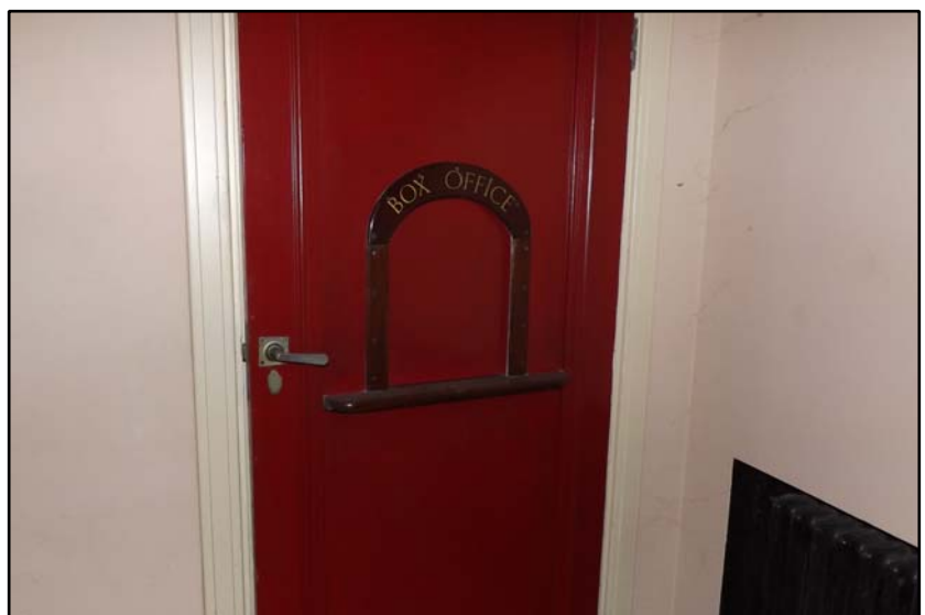
Former box office door Fig 4.4.26
