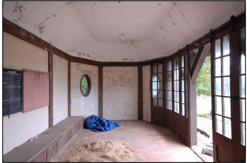
Interior of the pavilion, looking south Fig 5.2.7
