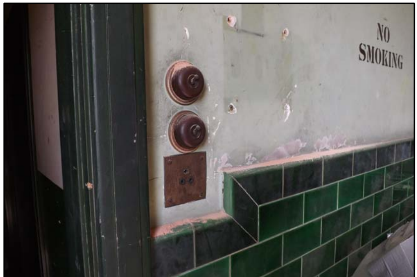
Detail of tiling and bakelite switches Fig 4.4.34
