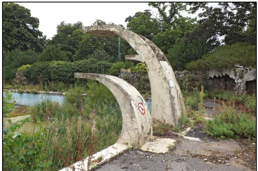
The concrete diving boards, looking north-west Fig 5.4.8
