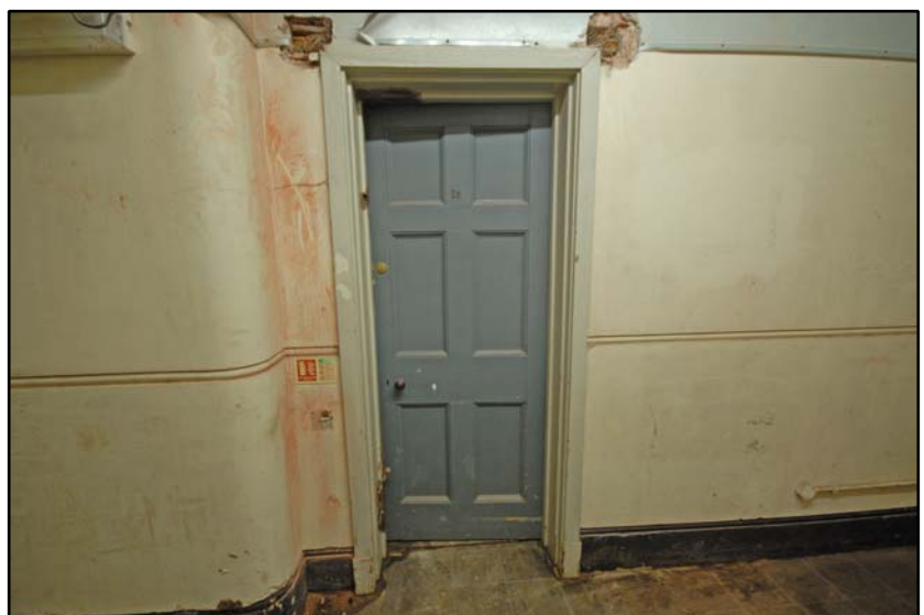
Example of panelled door to the staff rooms Fig 4.2.6
