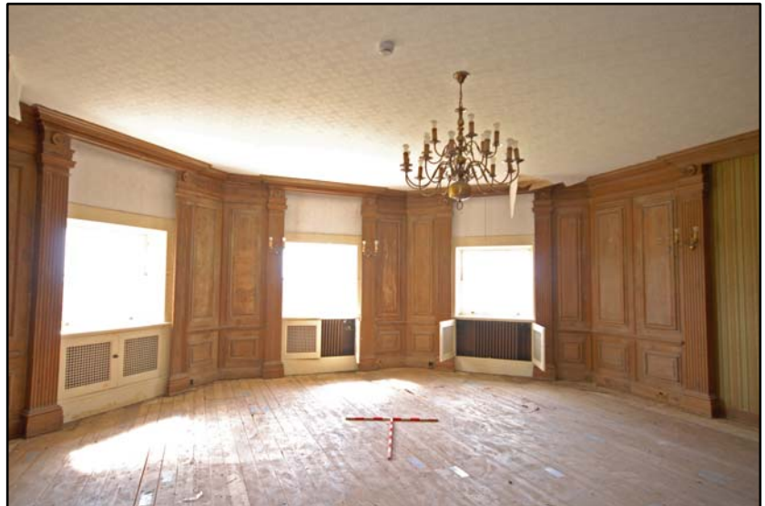
Room S2, looking south-west Fig 4.6.4
