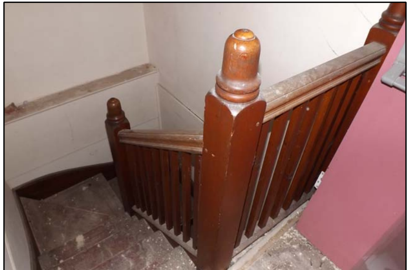
Stair between the Theatre and Projector Suite, F16 Fig 4.4.28
