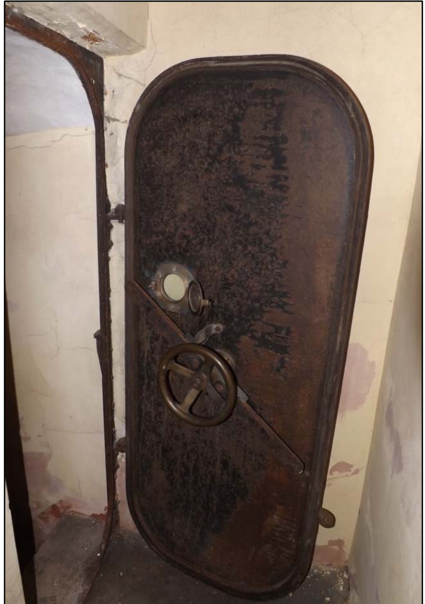
Entrance to the air raid shelter Fig 4.4.36
