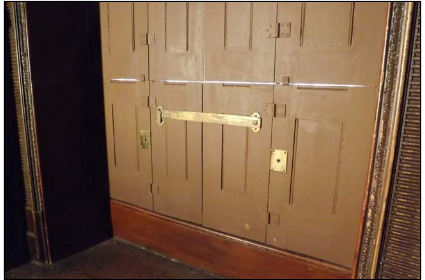
Detail of shutter hinges and lock Fig 4.3.19
