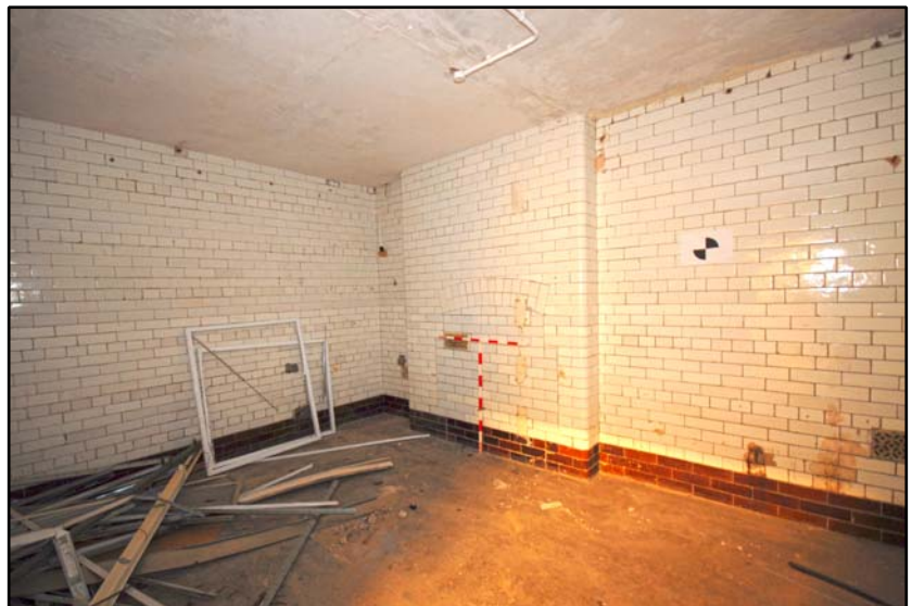
Blocked opening in the cold storage room Fig 4.2.8
