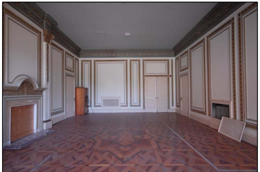
Room G2, looking east Fig 4.3.5
