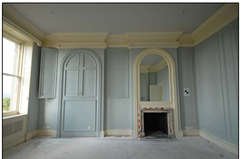
Room F4, the west elevation Fig 4.5.12
