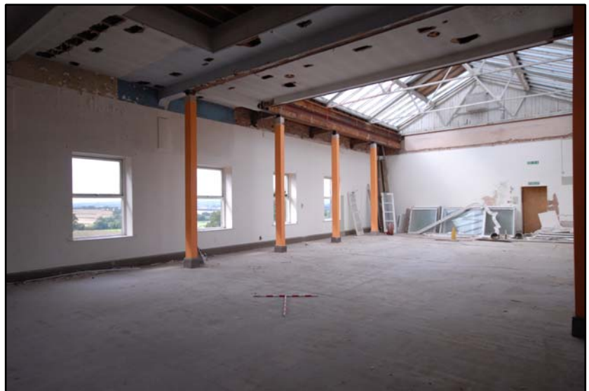
Room F1, looking south-west Fig 4.5.2
