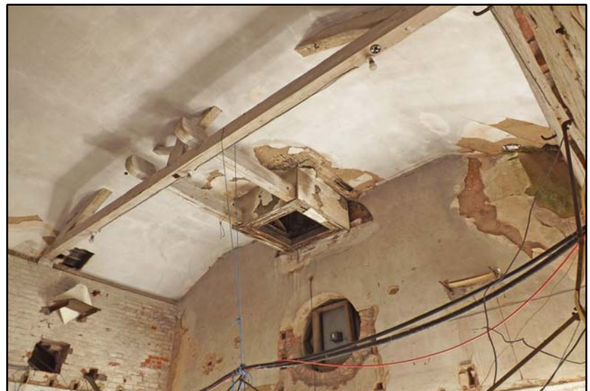
The structural supporting beams of the cupola Fig 5.1.17
