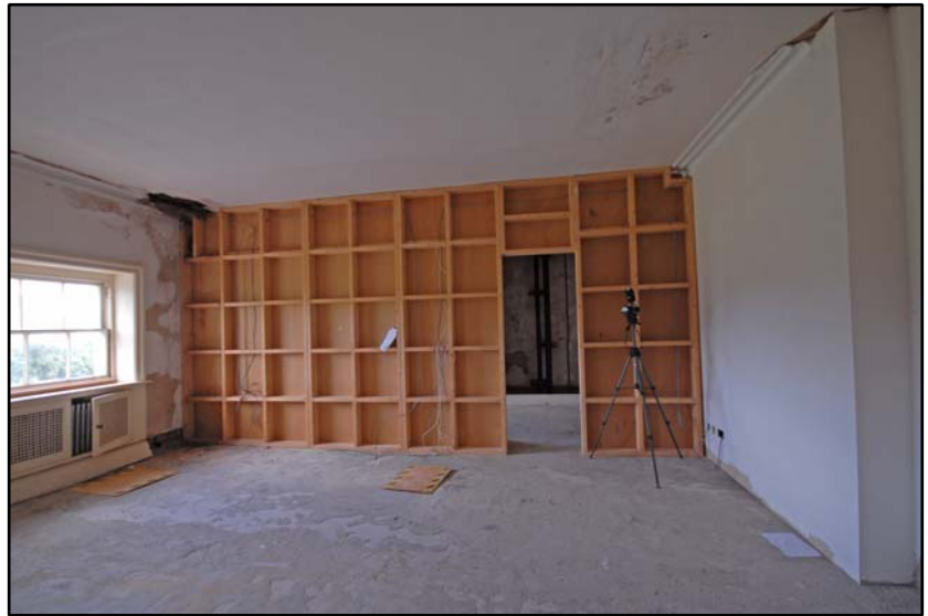
Room S8, looking east toward the modern partition Fig 4.6.19
