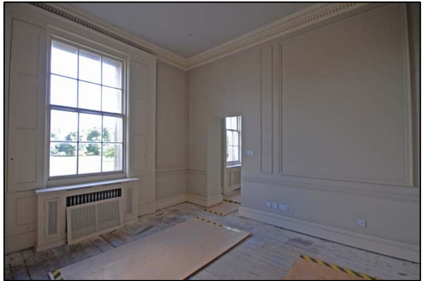
Room F8, looking north-east Fig 4.5.18
