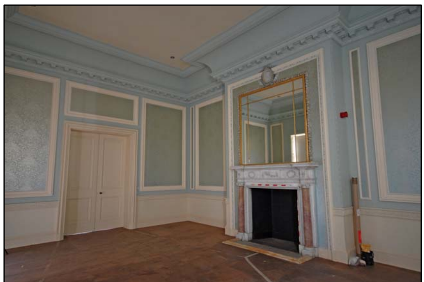
Room G3, looking north-east Fig 4.3.9
