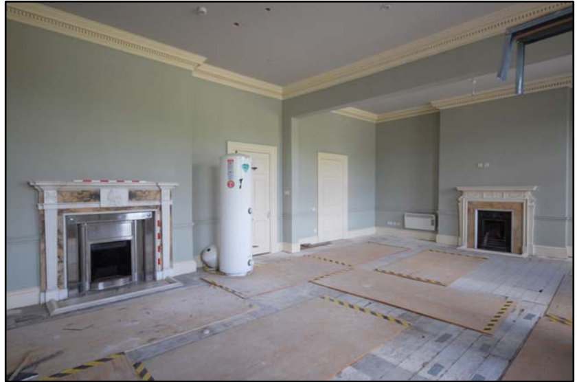
Room F9, looking south-west Fig 4.5.21
