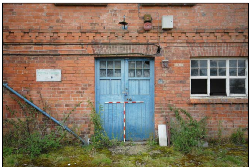
Detail of the main, central door to the Bothy Fig 5.7.3
