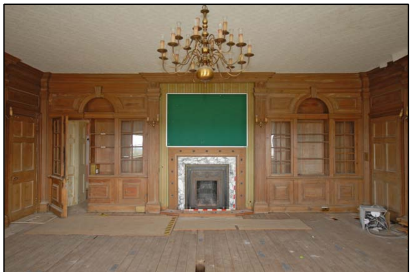
Room S2, looking north with concealed door open Fig 4.6.5
