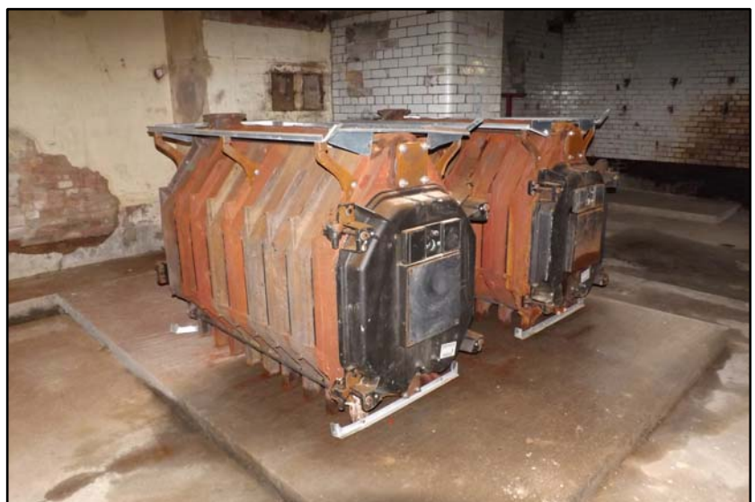
Boilers surviving in-situ Fig 4.2.21
