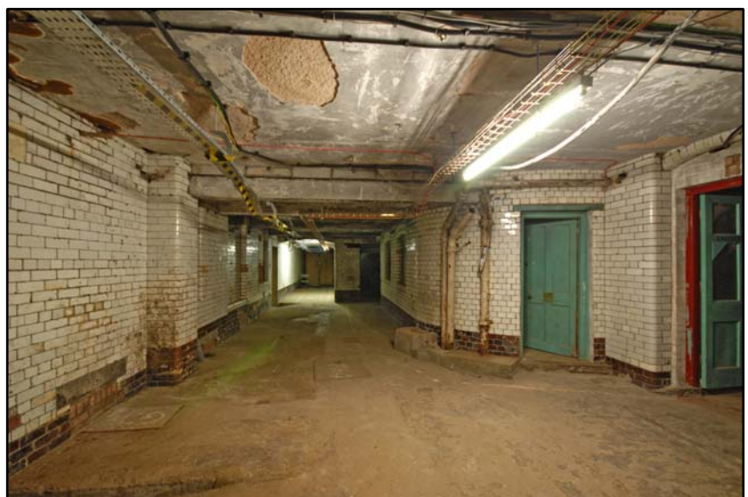
The southern workshop and boiler areas Fig 4.2.18
