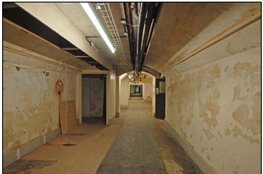
The south corridor, looking west Fig 4.2.17
