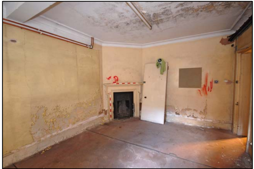
Staff room in the northern extent of the cellars Fig 4.2.4
