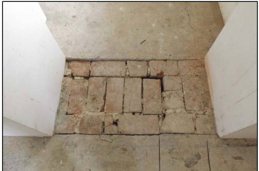
Modern door insertion between rooms S6 and S7 Fig 4.6.14
