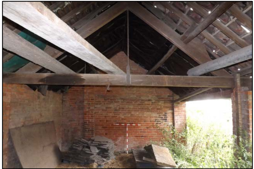
The central shed, looking east Fig 5.9.4
