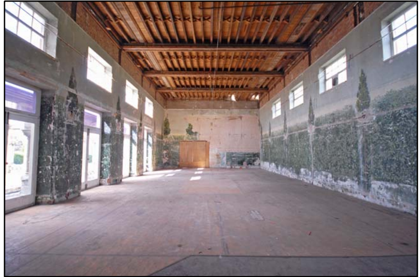
The badminton court, G1, looking west Fig 4.3.1
