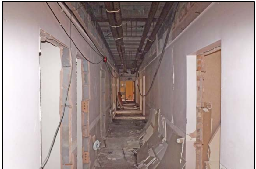
The central corridor of the 1980's extension Fig 5.1.23
