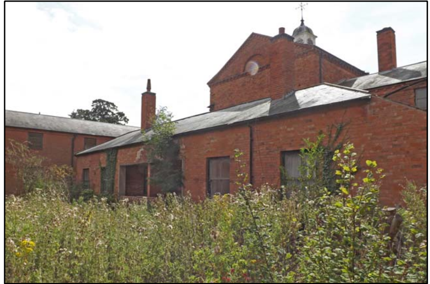
The 1950's extension to the rear of the Mews Fig 5.1.19
