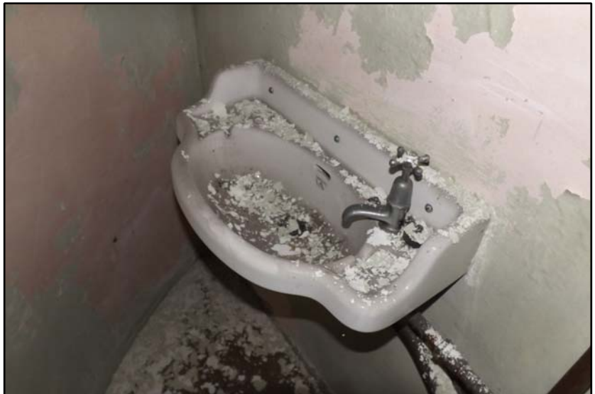
Sink within the air raid shelter Fig 4.4.39
