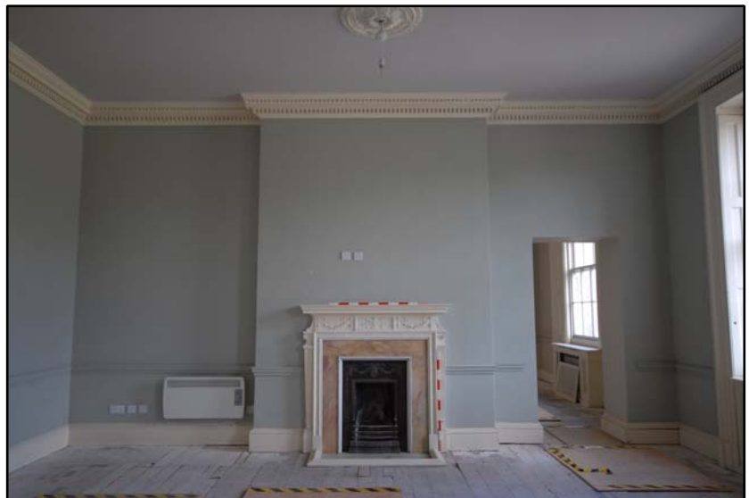
Room F9, the west elevation Fig 4.5.22
