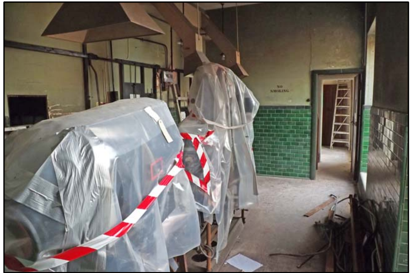
The projector room, F16, looking south Fig 4.4.30
