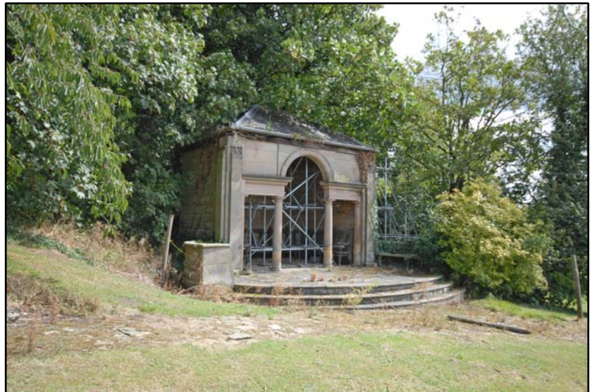
The Grotto, looking south-east Fig 5.5.2
