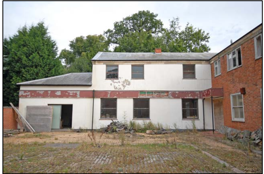
The south elevation of the north wing Fig 5.1.4
