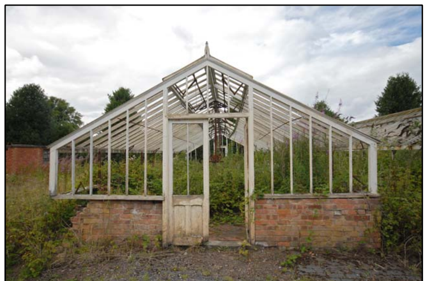
The south elevation of Greenhouse 1 Fig 5.8.3
