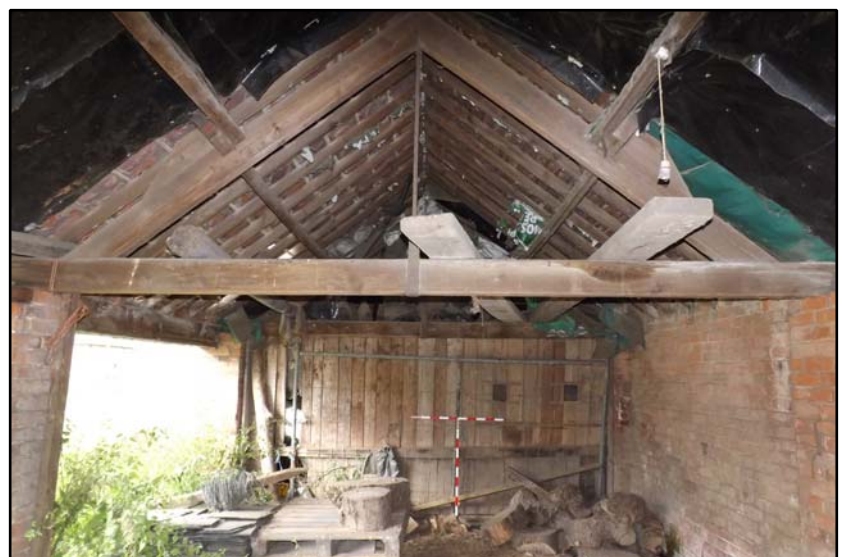
The central shed, looking west Fig 5.9.3
