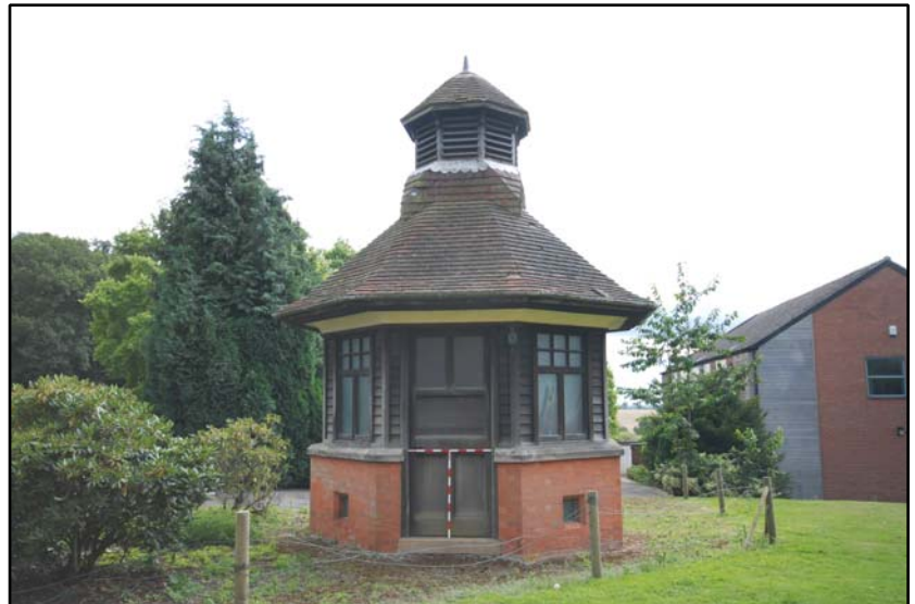
The north-west elevation, looking south-east Fig 5.3.2
