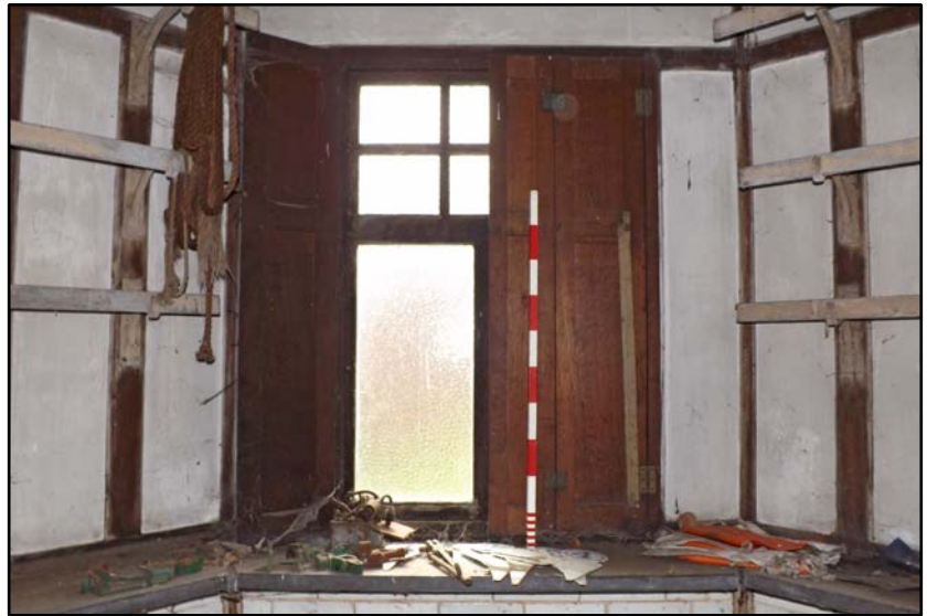
Detail of the windows and hanging rails Fig 5.3.4
