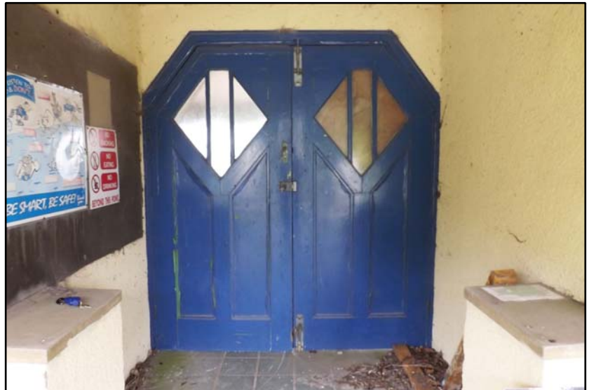
Interior view of the original entrance doors Fig 5.4.4
