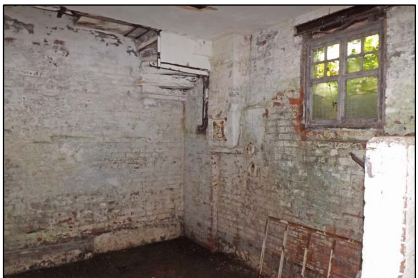
The Bothy cellar, looking west Fig 5.7.21
