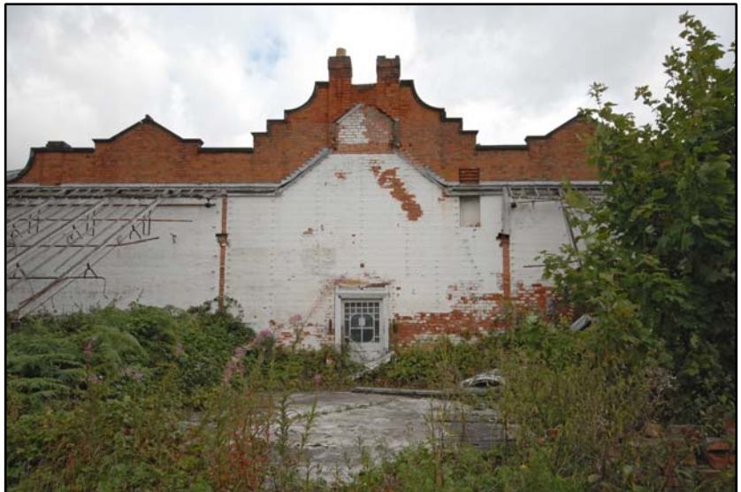
The former peach house to the rear of the bothy Fig 5.6.5
