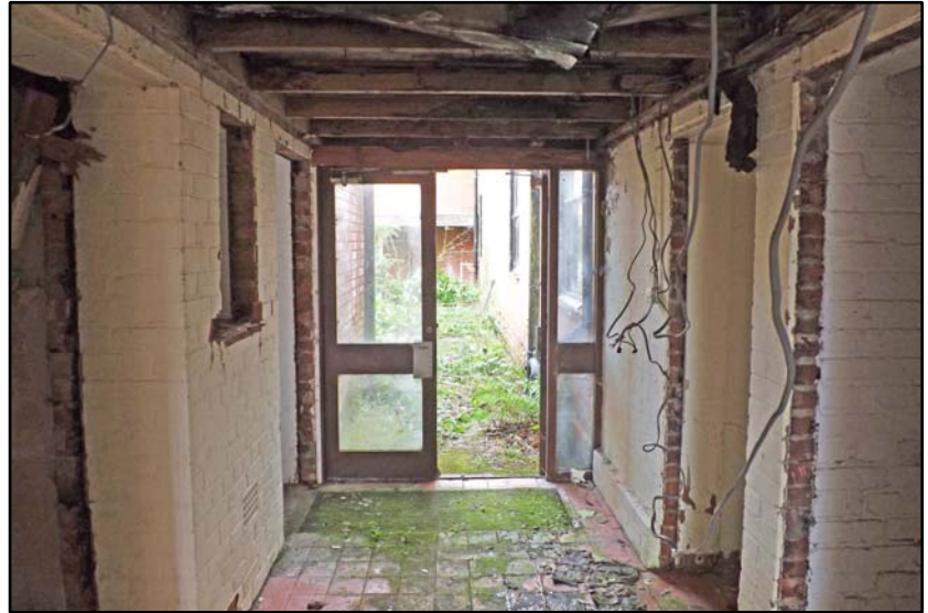
Entrance Hall of the central block, leading to the garden Fig 5.1.10
