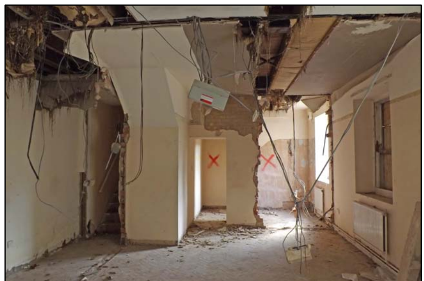
Interior of the central block Fig 5.1.12
