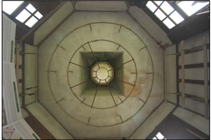
The ceiling hanging rails Fig 5.3.7
