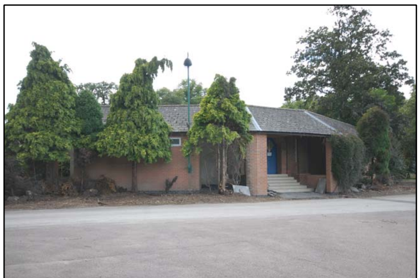
The south-east elevation Fig 5.4.3
