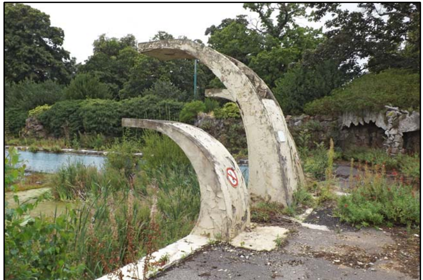
The concrete diving boards, looking north-west Fig 5.4.8
