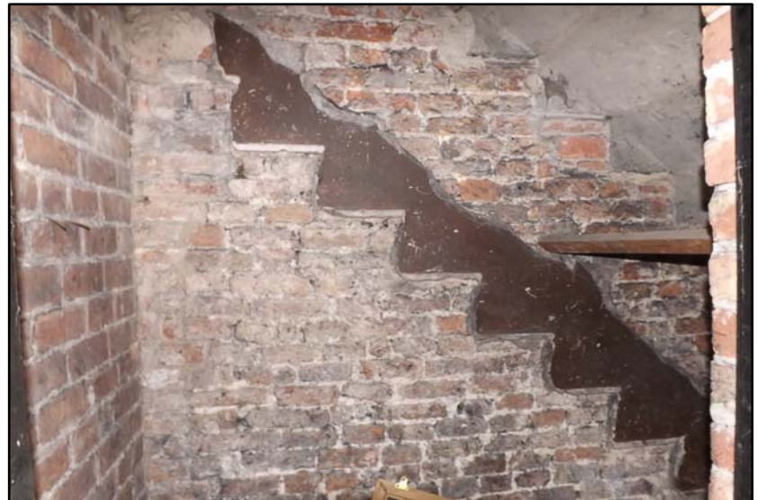
Remains of former stair Fig 5.1.11
