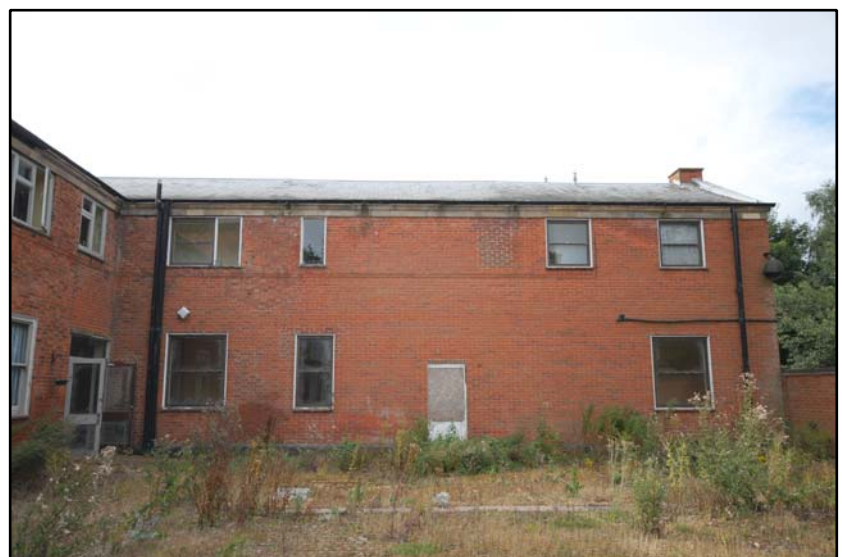
The north elevation of the south wing Fig 5.1.3
