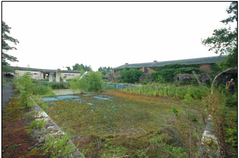
View of the swimming pool, looking west Fig 5.4.11
