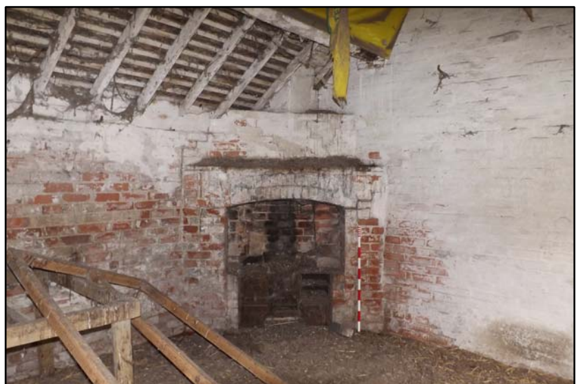
The mess, with fireplace and cast iron wood burner Fig 5.9.6
