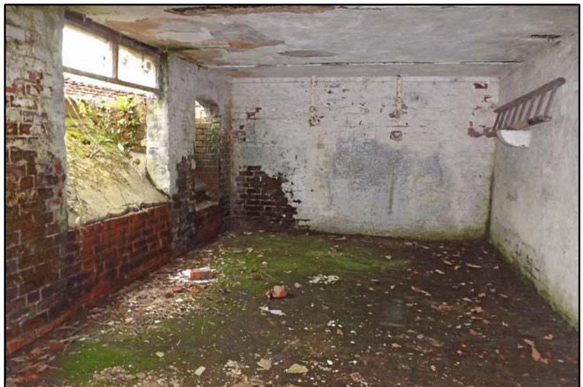
The Bothy cellar, looking east Fig 5.7.20
