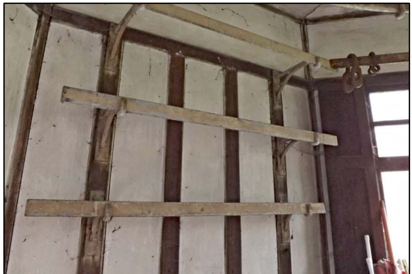
Detail of the hanging rail brackets Fig 5.3.5
