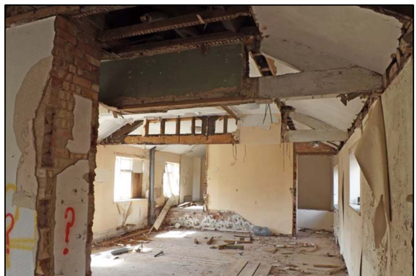
View of the first floor, looking north Fig 5.1.18
