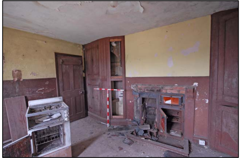
First floor head gardeners' kitchen, looking east Fig 5.7.13
