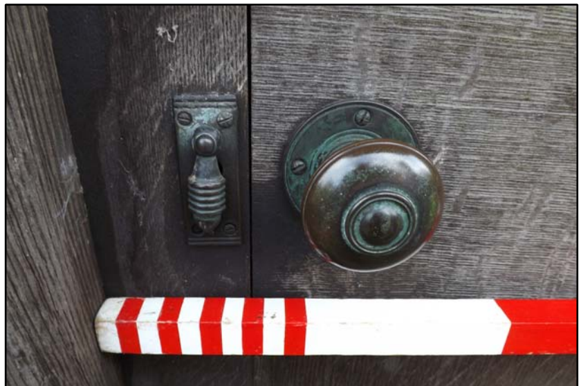
Detail of the door furniture Fig 5.3.8
