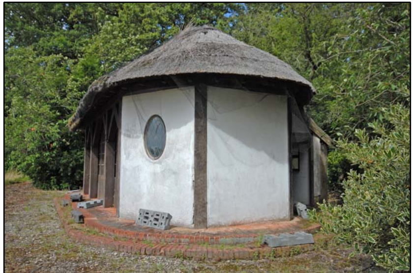
The south elevation of the tennis pavilion Fig 5.2.2
