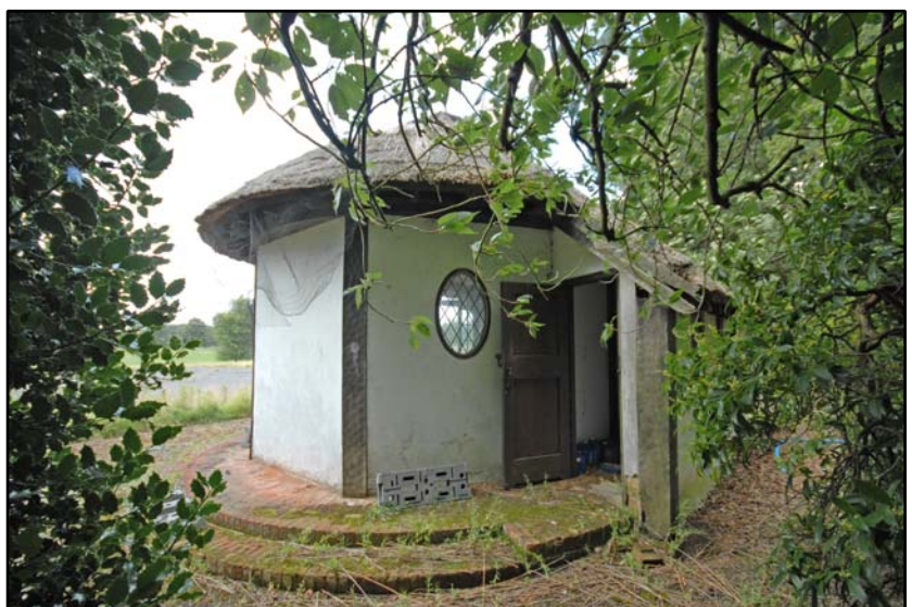
The south elevation of the tennis pavilion Fig 5.2.3
