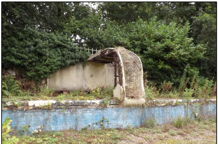
The concrete waterfall at the west end of the pool Fig 5.4.15
