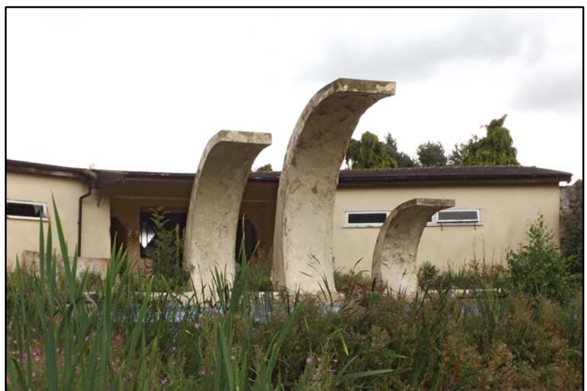
The underside of the diving boards Fig 5.4.9
