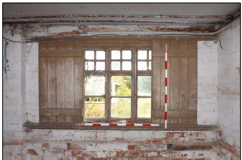
Detail of ground floor window with wooden sliding shutters Fig 5.7.12
