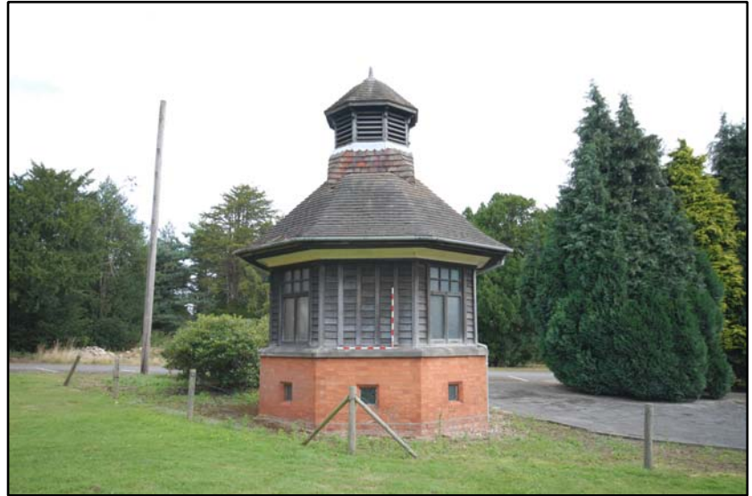
The south-west elevation, looking north-east Fig 5.3.1
