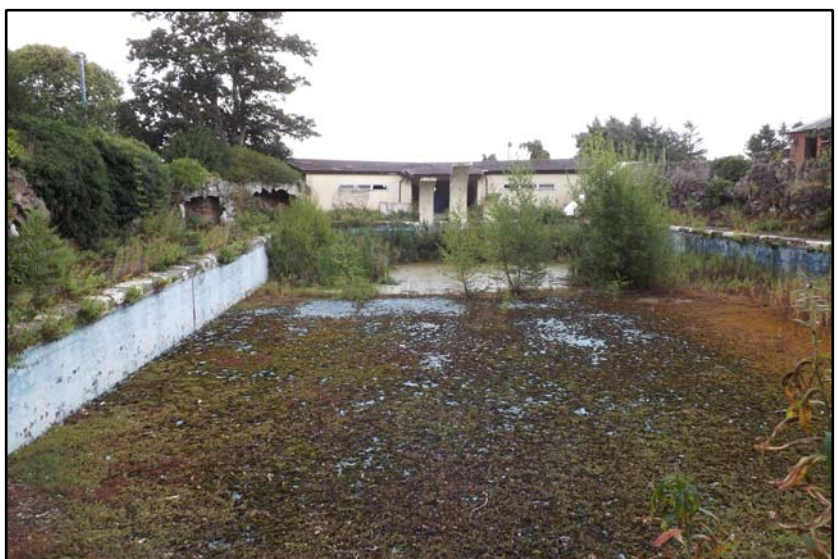
View of the swimming pool, looking north-east Fig 5.4.12
