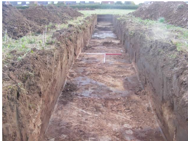
Trench 3, looking east Fig 7
