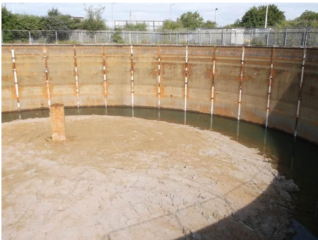
Gasholder 5 interior, looking north-west Fig 14
