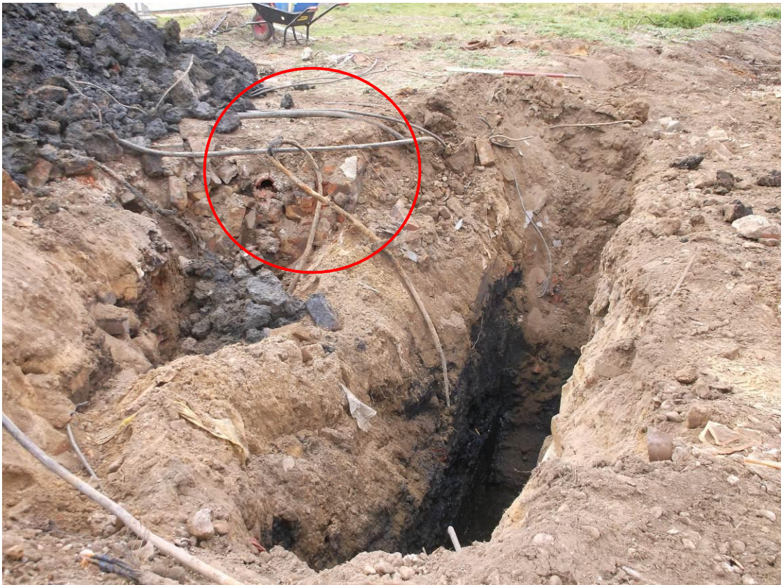
TP5, a brick corner foundation, looking west Fig 11
