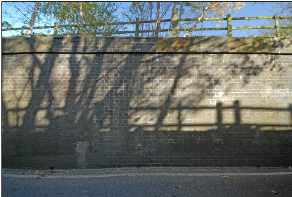
The central portion of the north abutment with sandstone padstones at the top Fig 9
