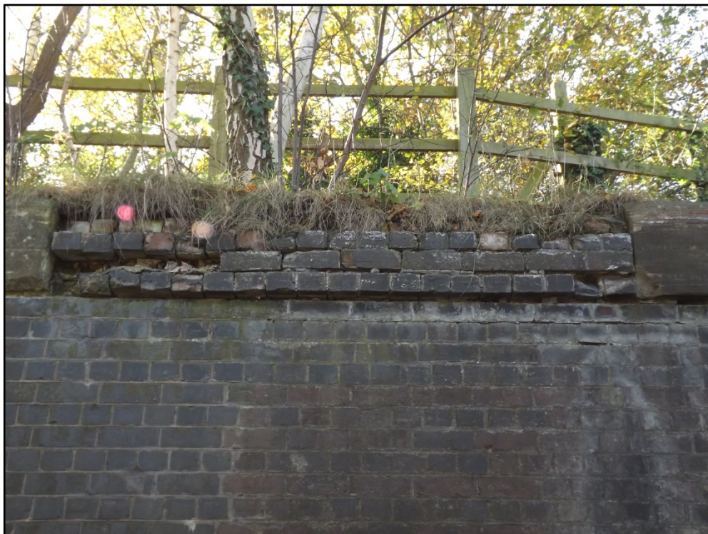
The southern abutment, detail of the damaged coping bricks Fig 13
