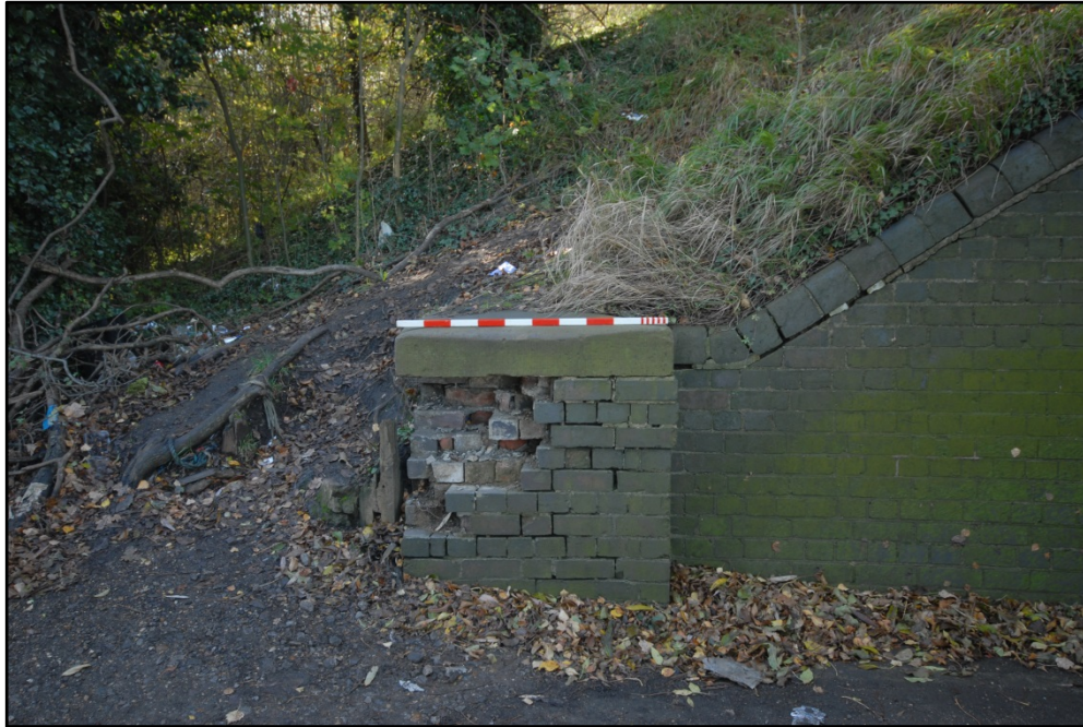
The south abutment, detail of the damaged brick pier Fig 12
