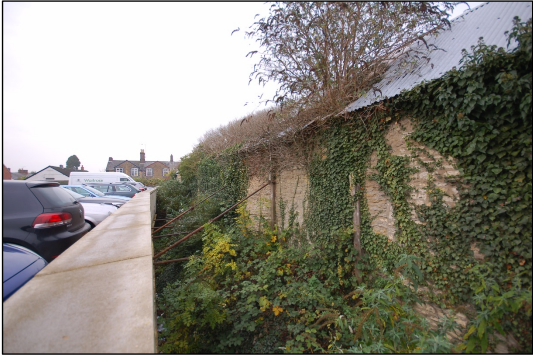
The rear of the linear range, showing modern steel props and the damage caused by vegetation Fig 18
