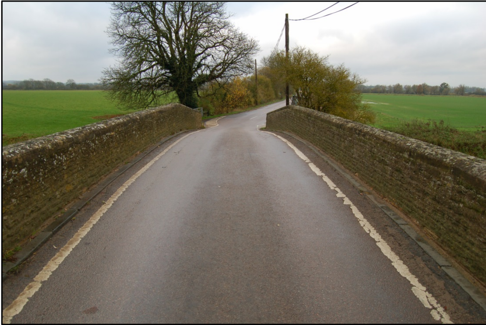
The bridge prior to excavation, looking south Fig 4
