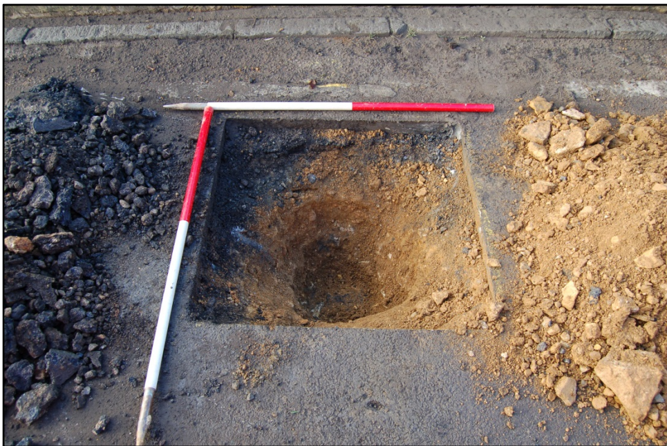
Test pit 2, looking west Fig 7
