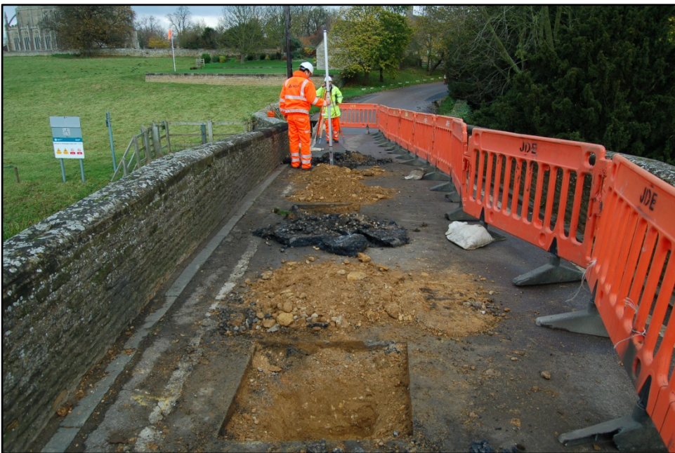
Test pits 1-3 upon completion of excavations, looking north Fig 9
