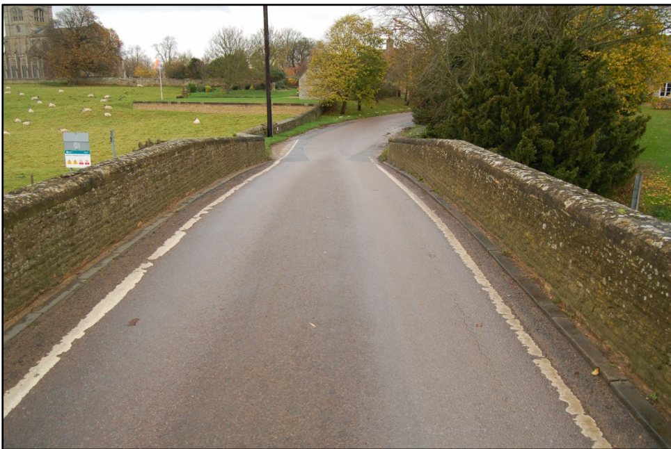
The bridge prior to excavation, looking north Fig 5
