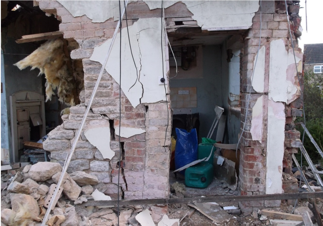
Squirrel Cottage, showing bull-nosed bricks on former doorway, looking east Fig 10
