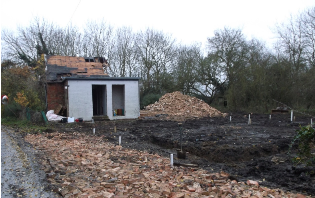
The site, with the partly-demolished Squirrel Cottage looking south Fig 5
