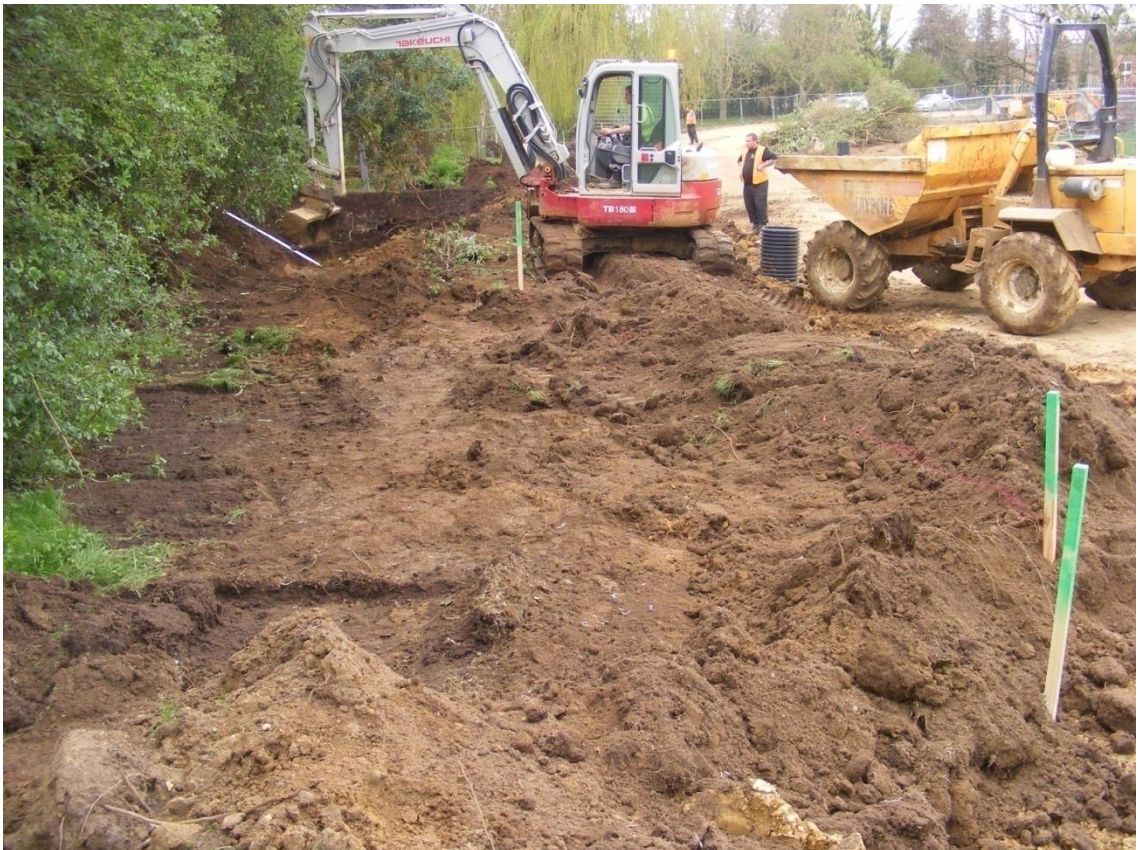
The groundworks in progress Fig 4
