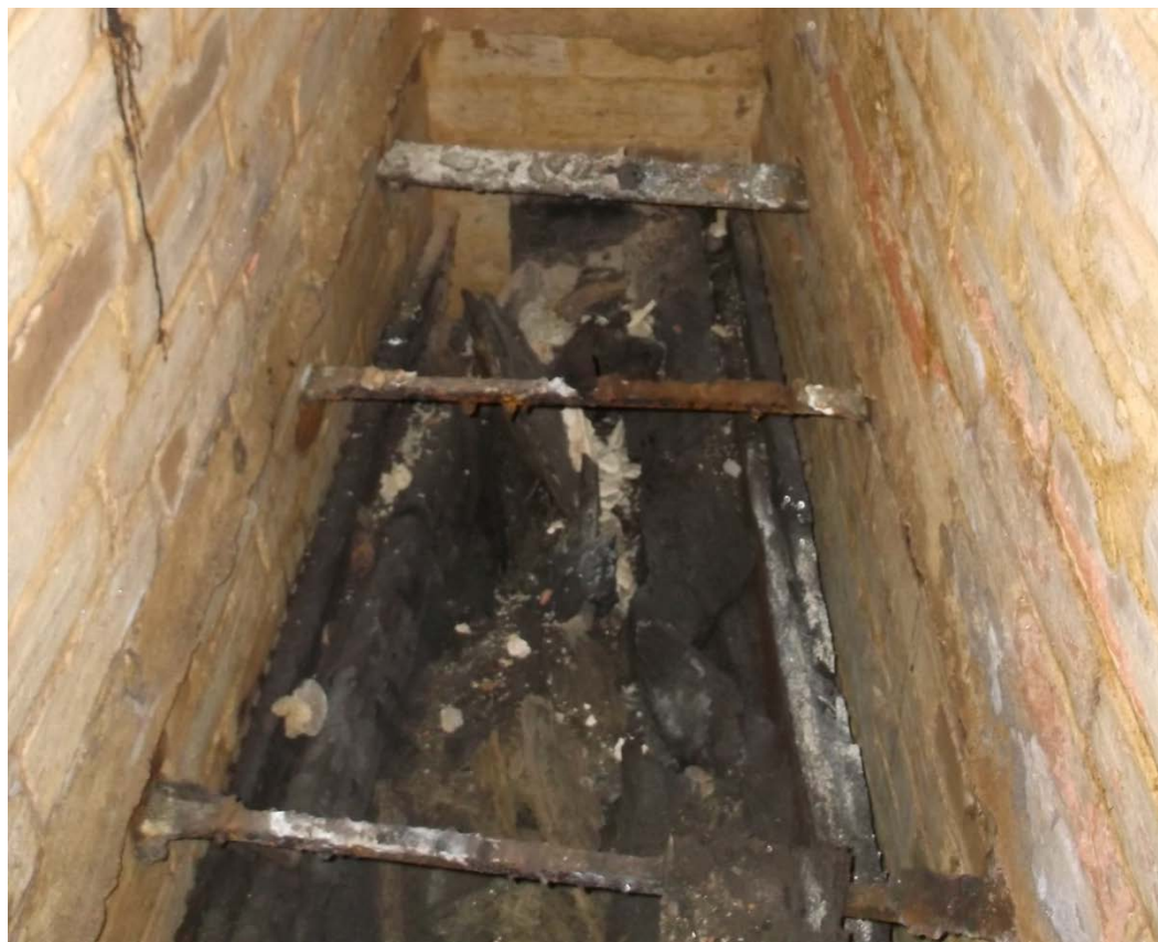
Vault (303), interior looking towards east end of vault Fig 9
