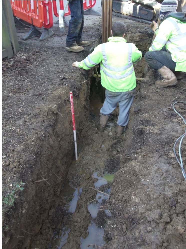
The groundworks in progress Fig 4
