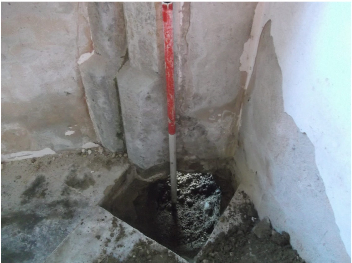
The connection pit inside the church Fig 6
