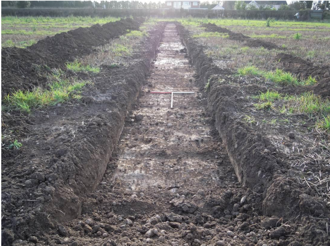
Trench 8, general view, looking south-west Fig 15
