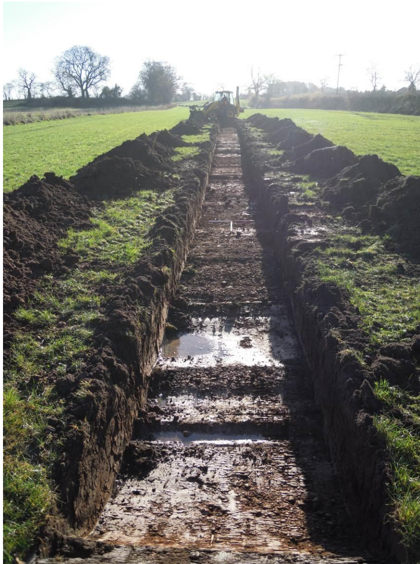
Trench 1, general view, looking south Fig 8
