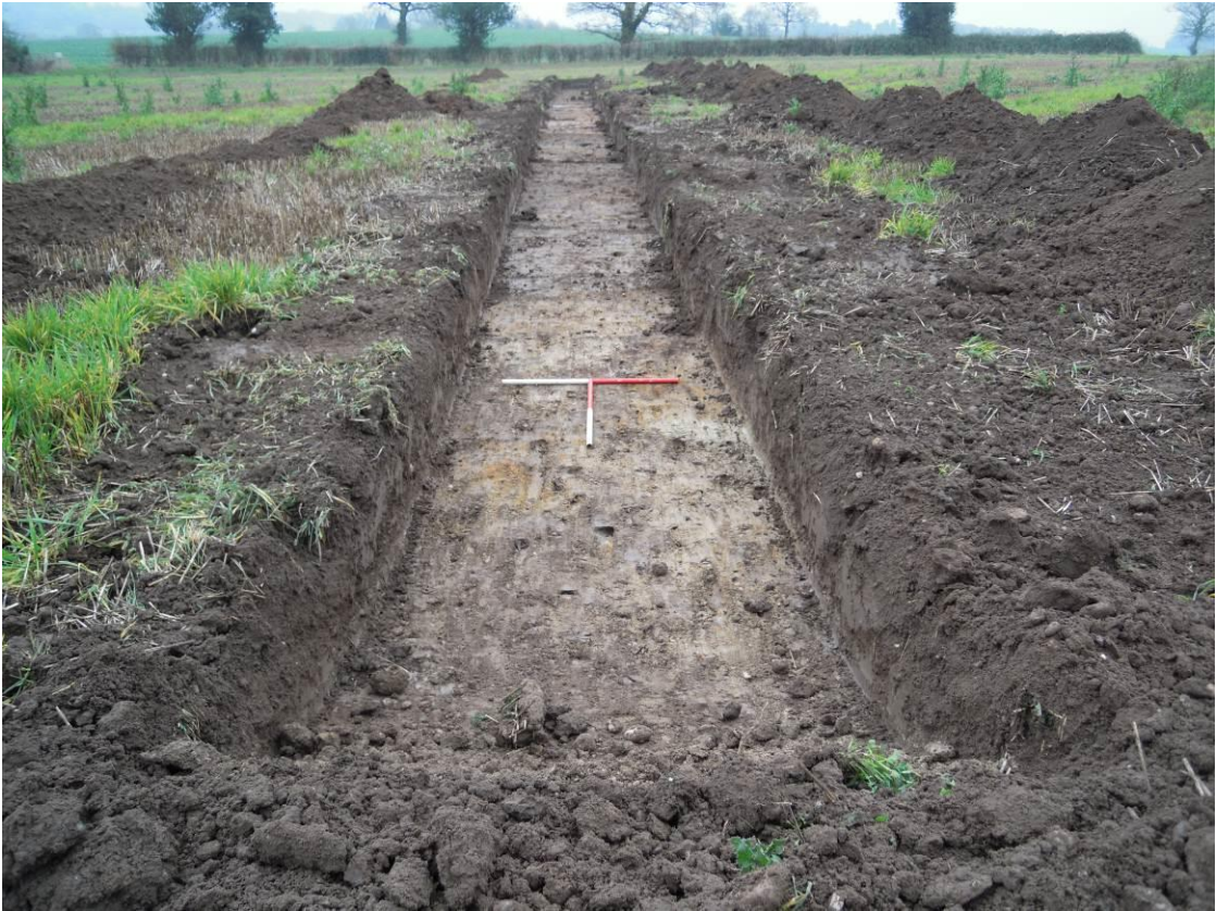
Trench 9, general view, looking east Fig 16
