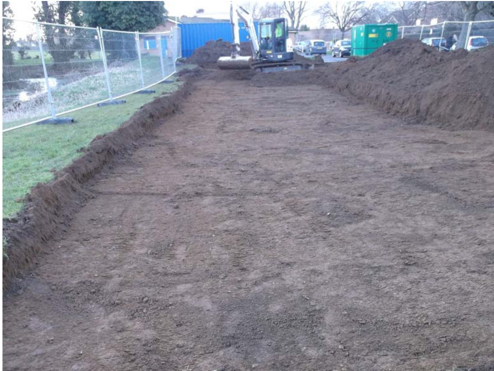
Trench 1, general view looking west Fig 3
