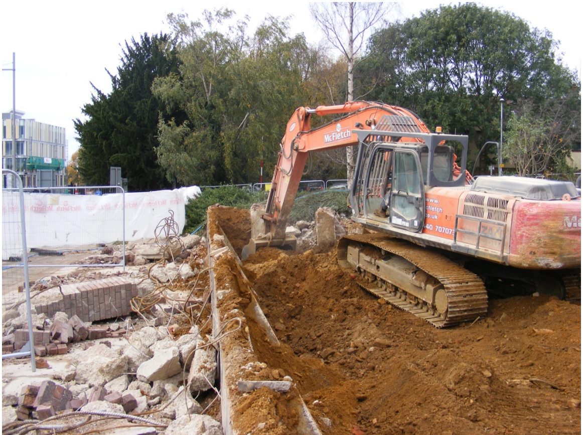
The groundworks in progress, looking west Fig 6
