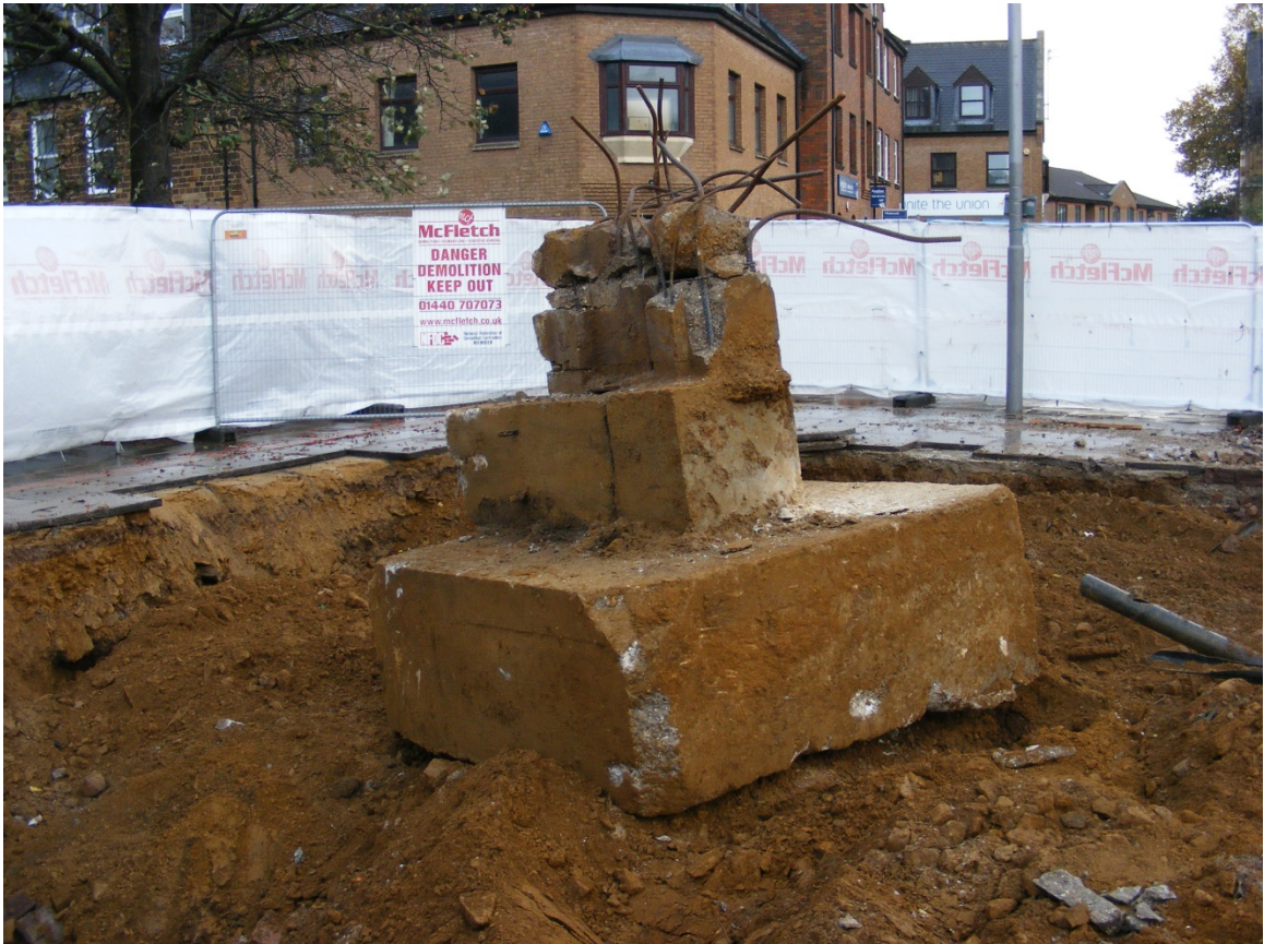
One of the column foundations after removal Fig 4
