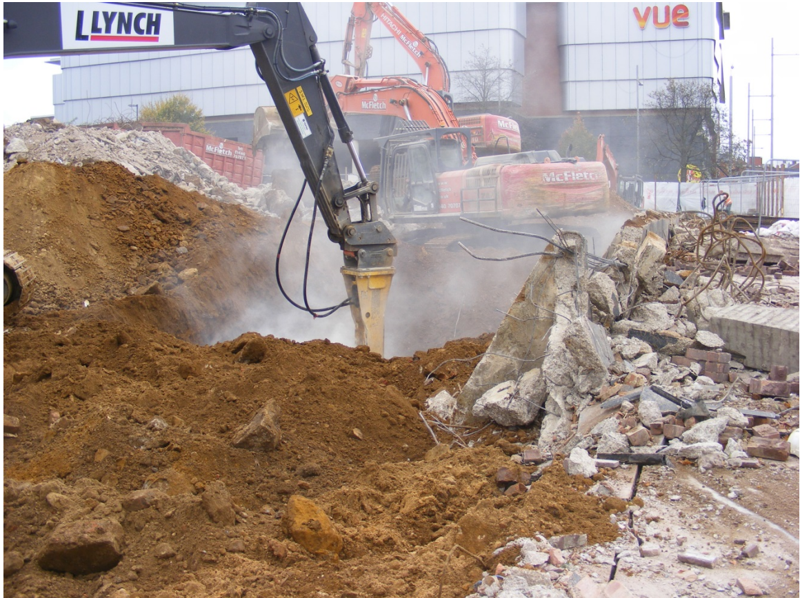
The groundworks in progress, looking east Fig 5
