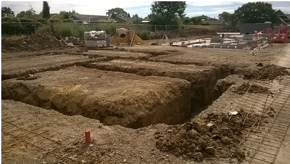
The groundworks in progress, looking west Fig 4
