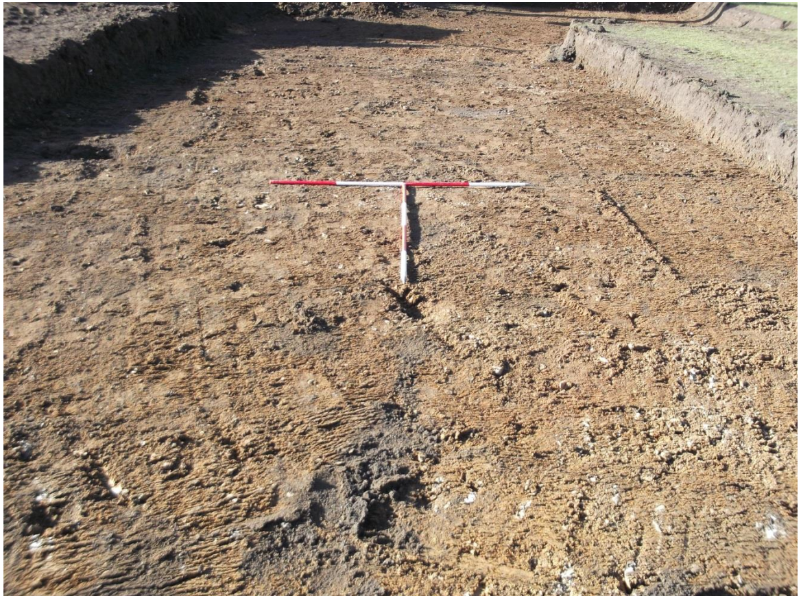
Overview of stripped area, looking north-west Fig 7
