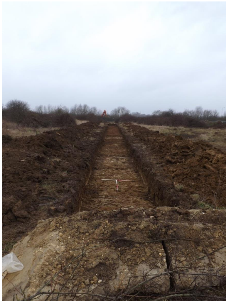
Trench 12 overview, looking north-west Fig 19
