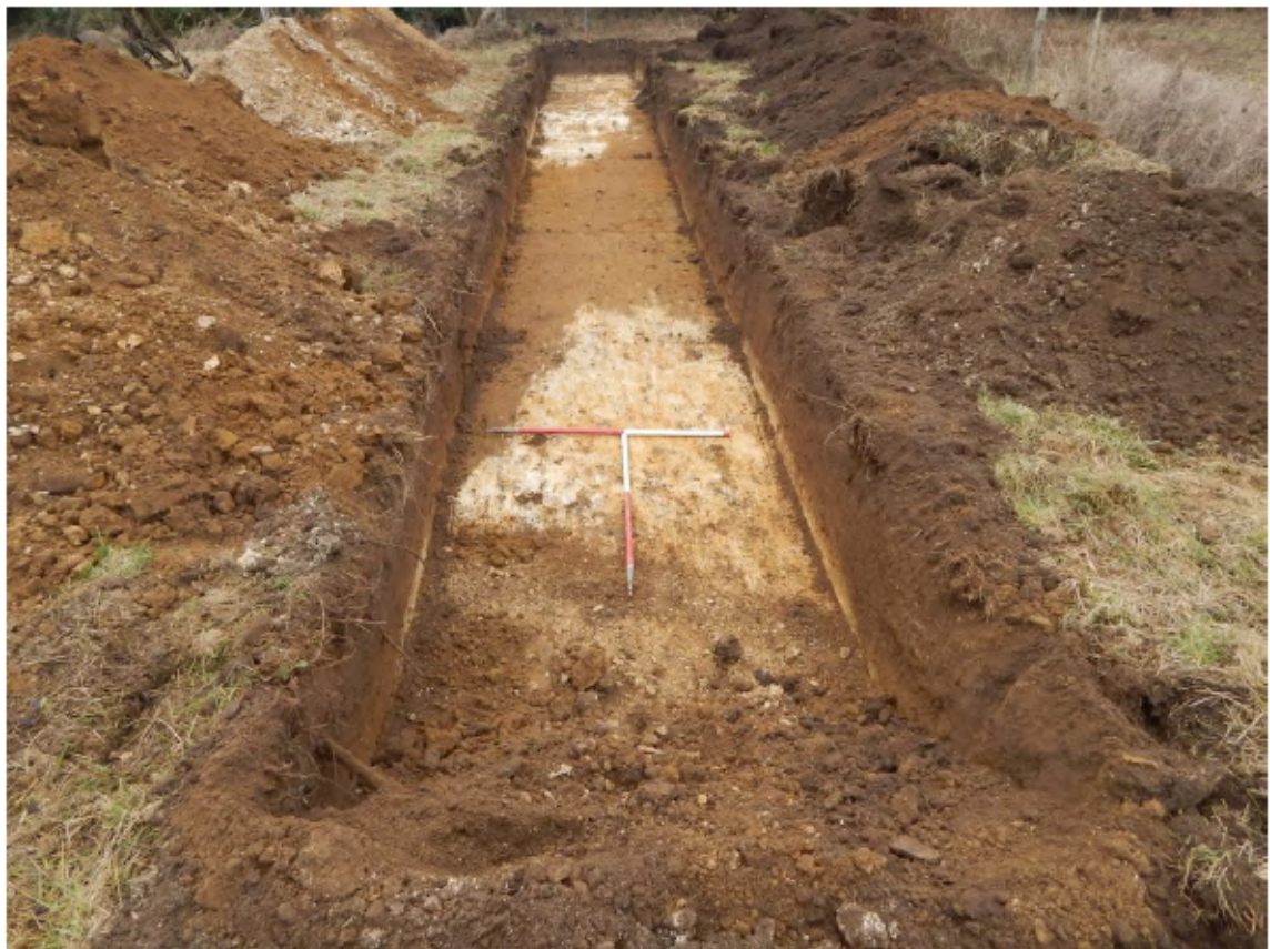
Overview of trench 11, looking north Fig 19
