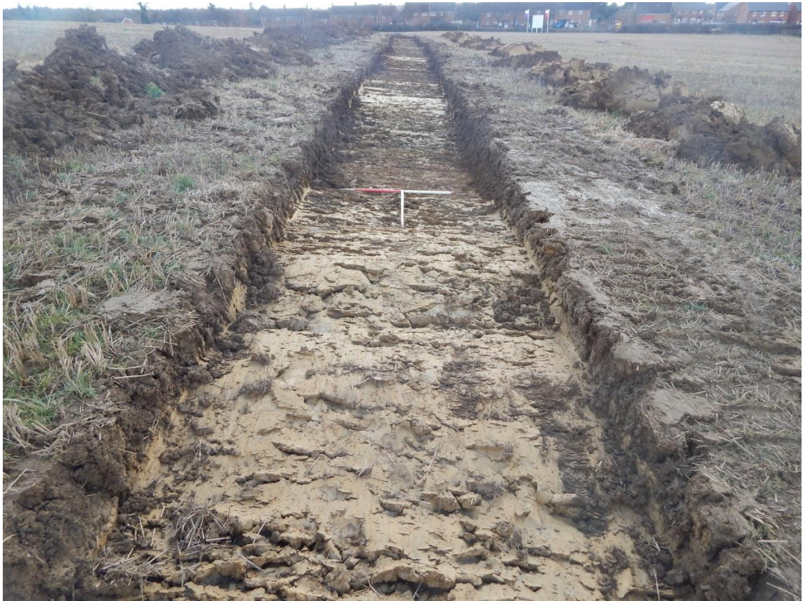
Overview of trench 15, looking south Fig 22
