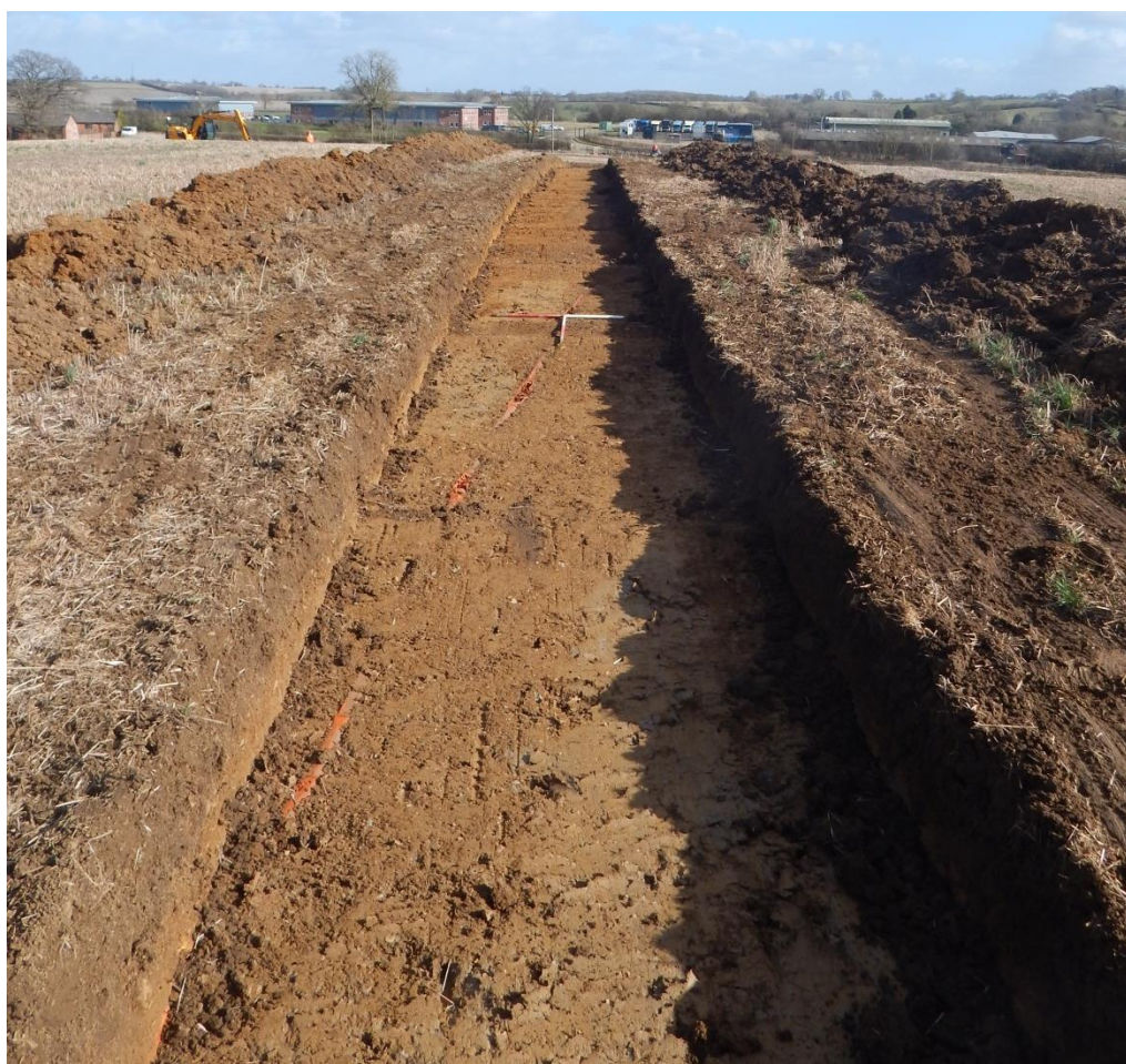
Overview of trench 13, looking east Fig 20
