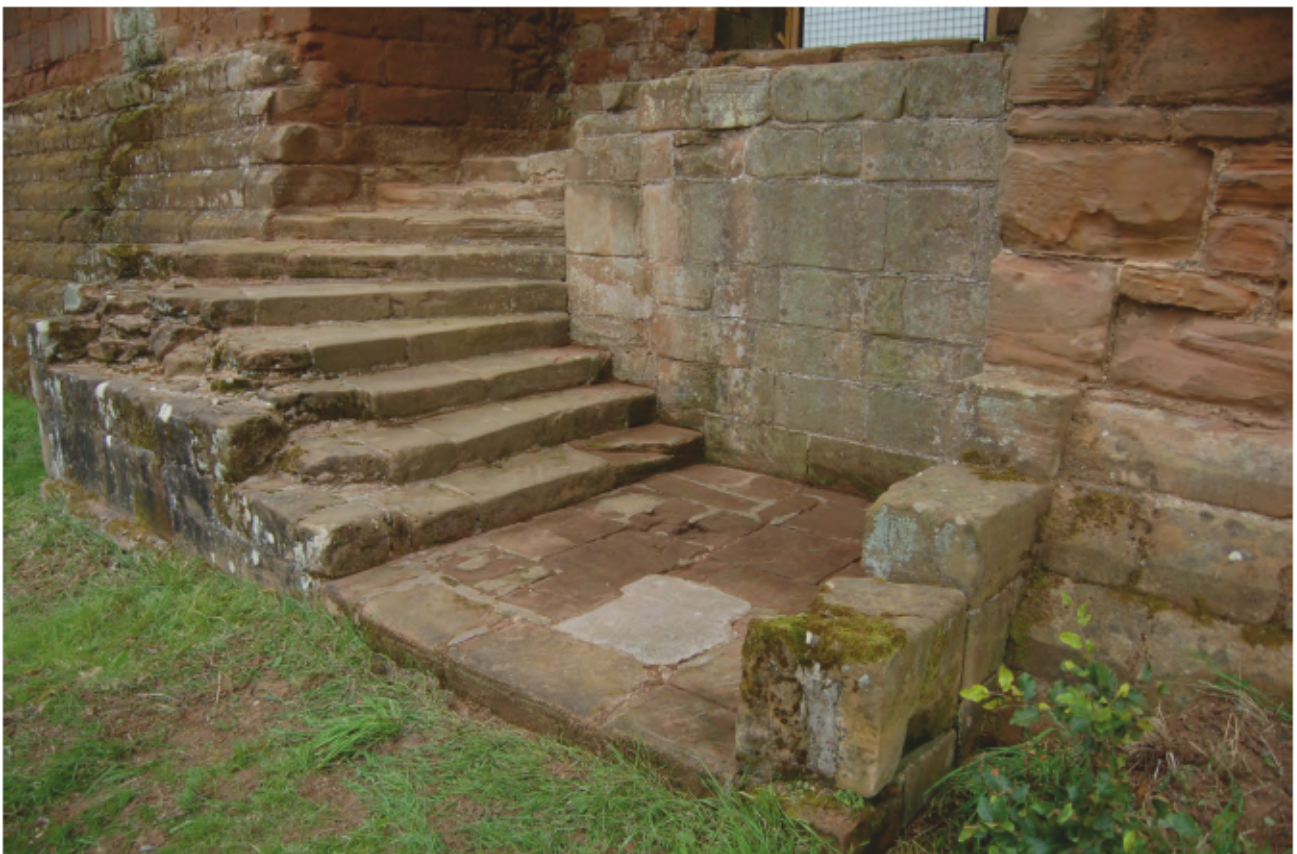
Sandstone stairs and platforms leading from the forebuilding arch Fig 38
