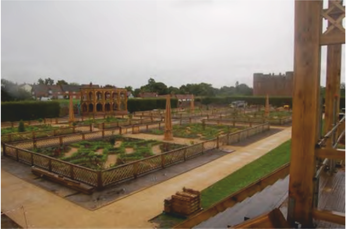
The 2009 garden under construction, looking north-east from the terrace Fig 11
