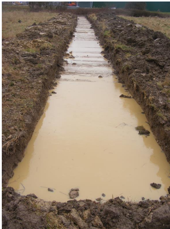
Trench 12, looking north-west Fig 3
