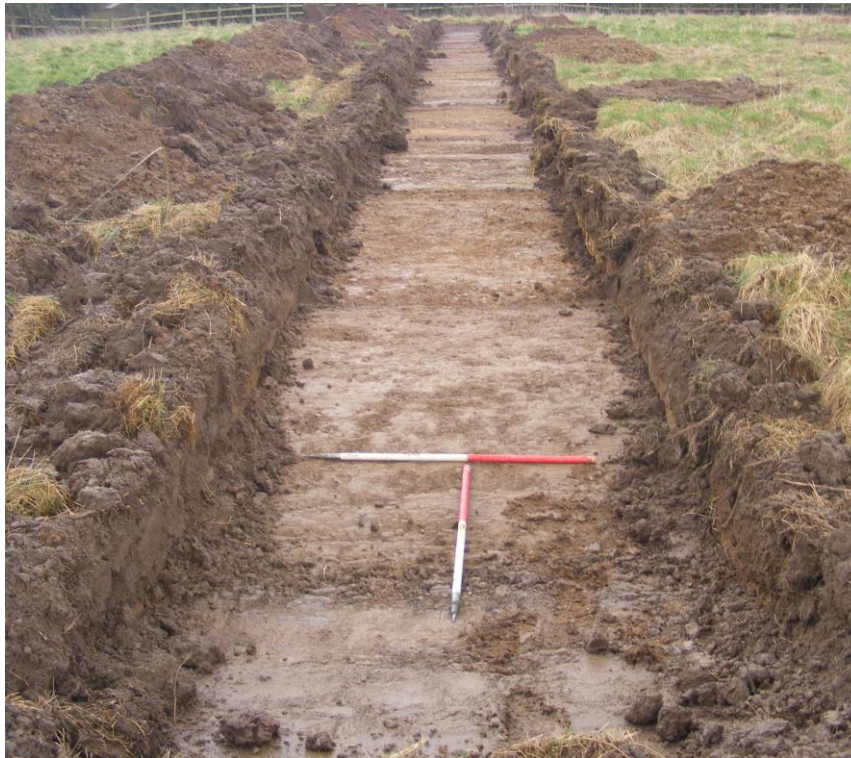
Trench 17, looking west-south-west
