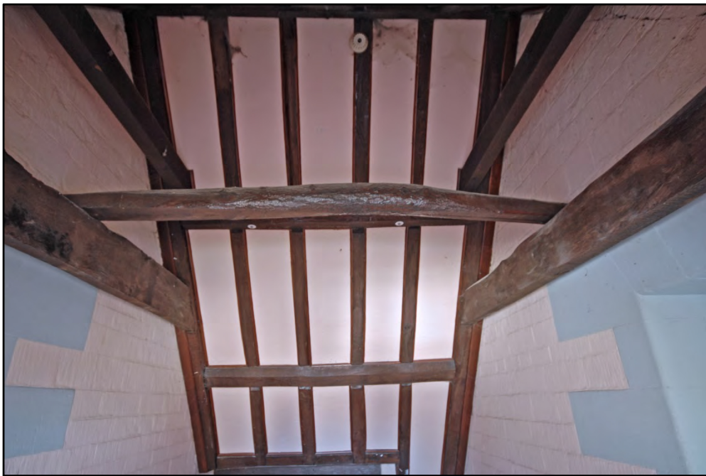
Detail of the roof structure over the north landing Fig 52
