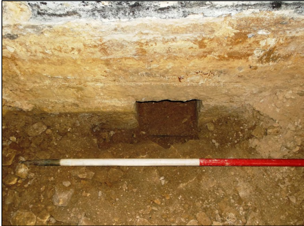
Trench 1, possible weep hole in foundations of east wall. Fig 59
