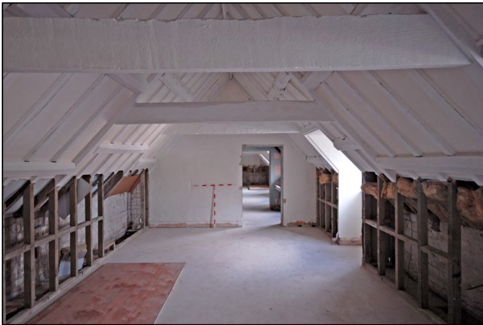
Room F3, looking west Fig 54
