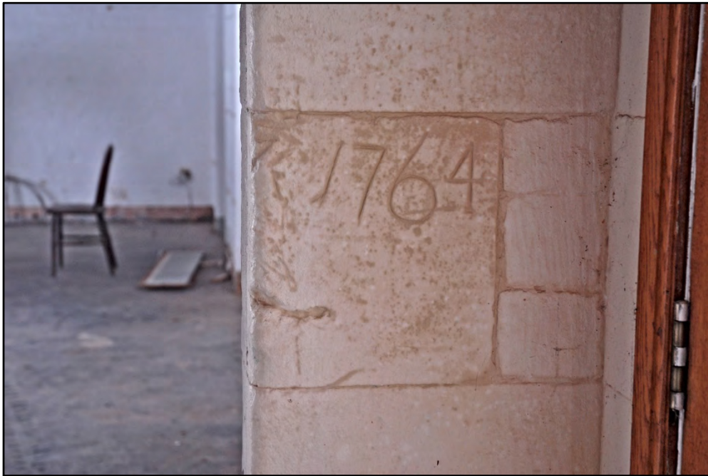
Detail of date stone, 1764, adjacent to the main entrance Fig 15
