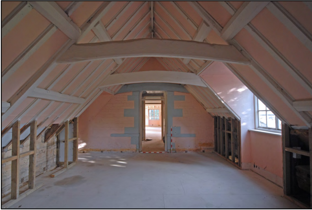
Room F2, looking east Fig 47
