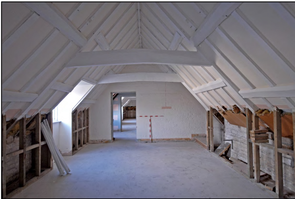
Room F4, looking east Fig 56
