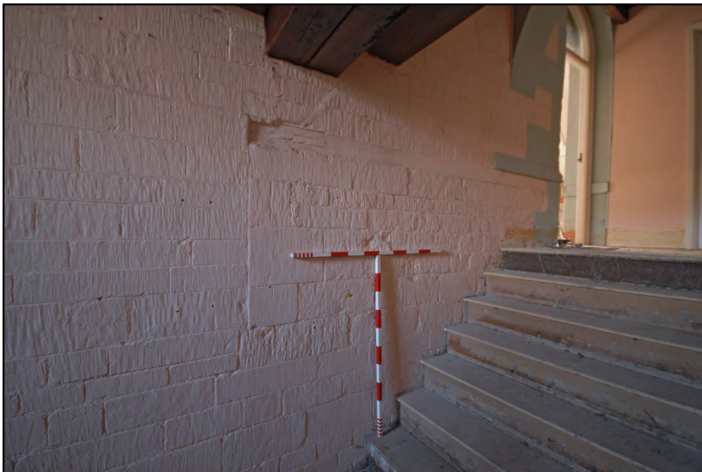
The intermediate landing, showing former quoin stones in line with the central dividing wall, looking south-east Fig 32
