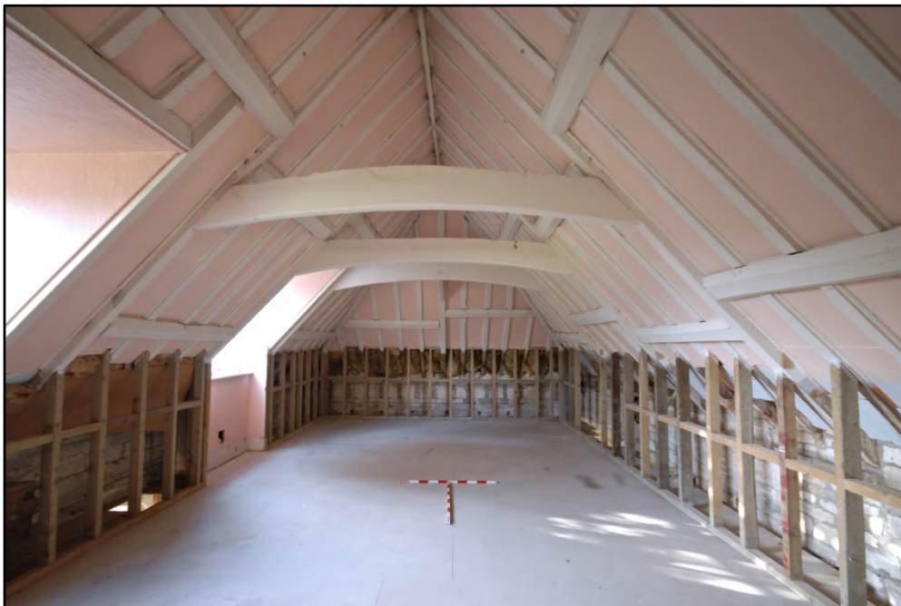
Room F2, looking west Fig 46
