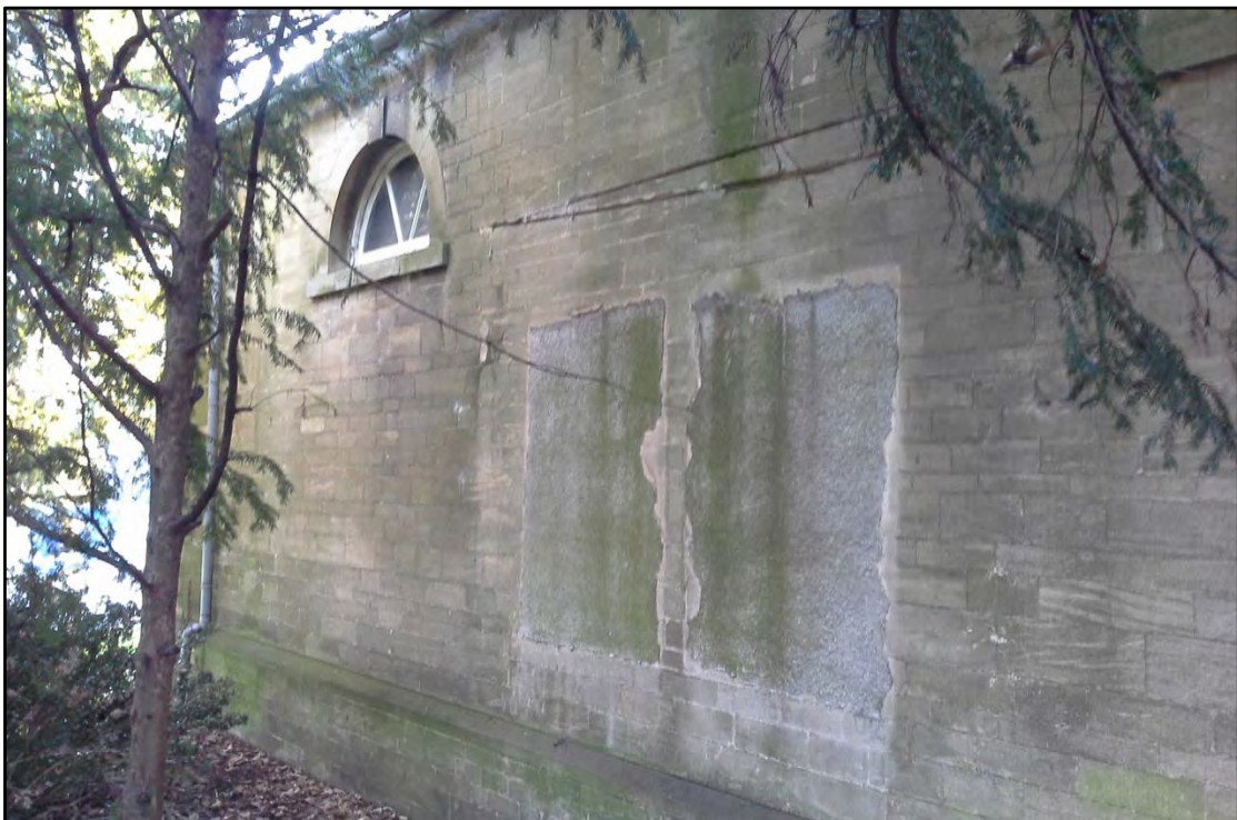
The east elevation, showing the rectangular blockings, looking south-west Fig 7
