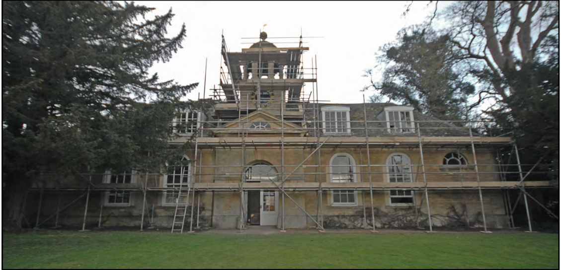
The south elevation, looking north Fig 2
