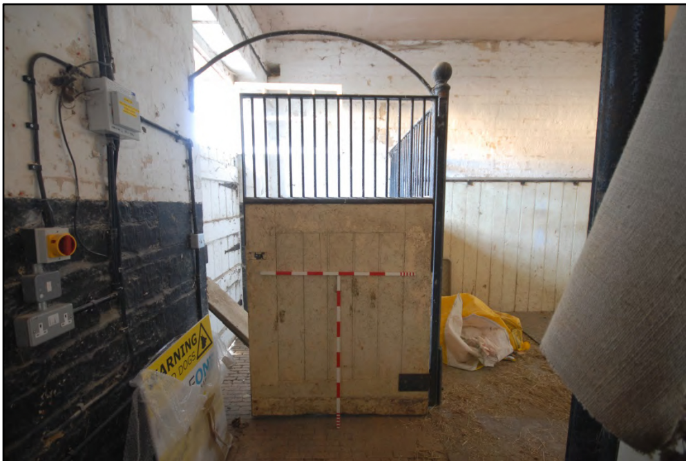
Detail of the stall doors Fig 26
