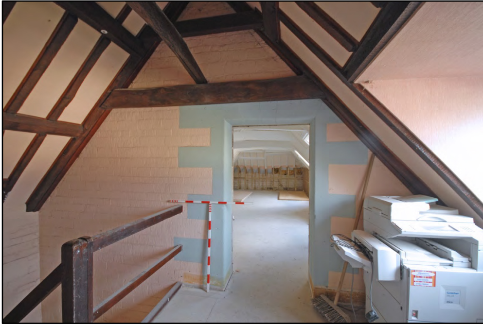
The north landing, looking west Fig 51
