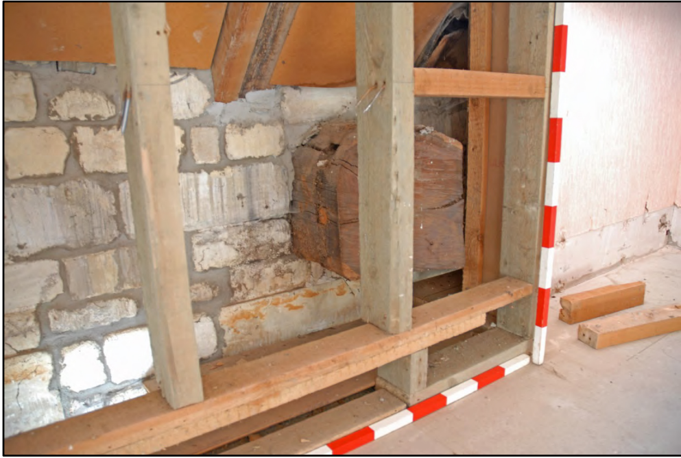
Detail of former tie beam with square peg holes Fig 43
