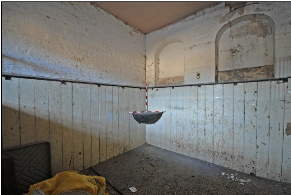
The eastern stall, showing the corner feeder, looking south-east Fig 24
