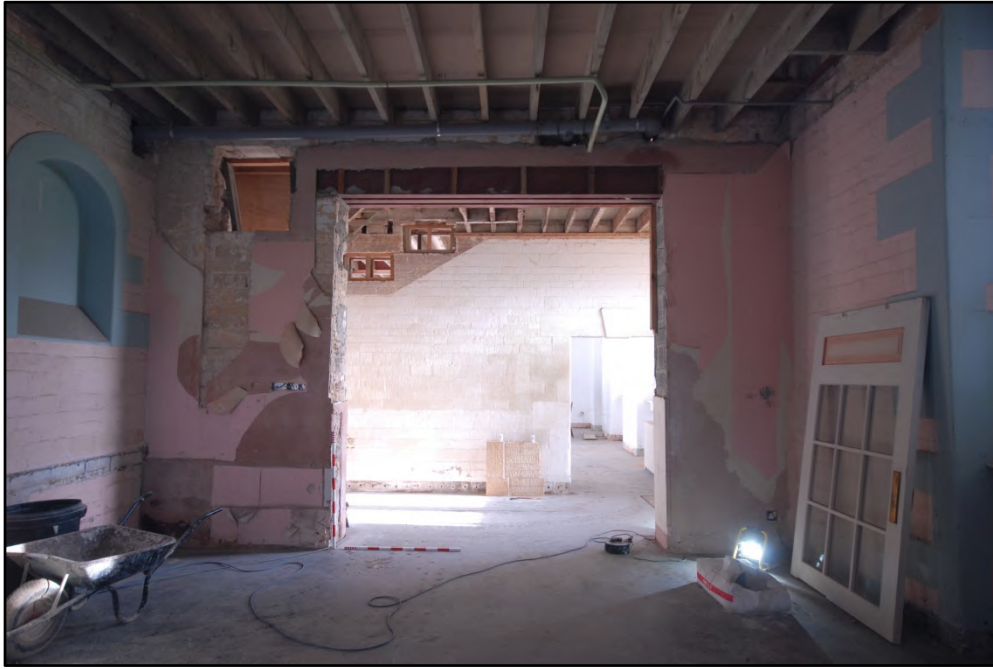
Room G2, showing the modern door opening, looking east Fig 19
