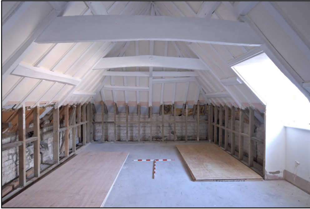
Room F4, looking west Fig 55
