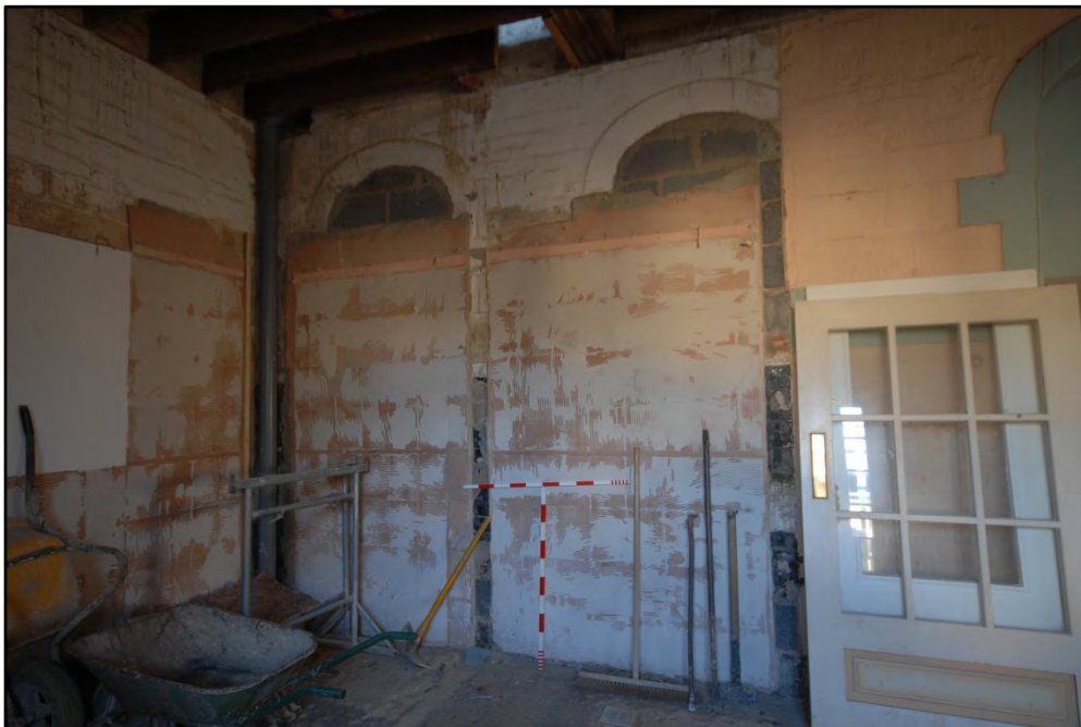
Room G4, detail of the blocked arched recesses Fig 30
