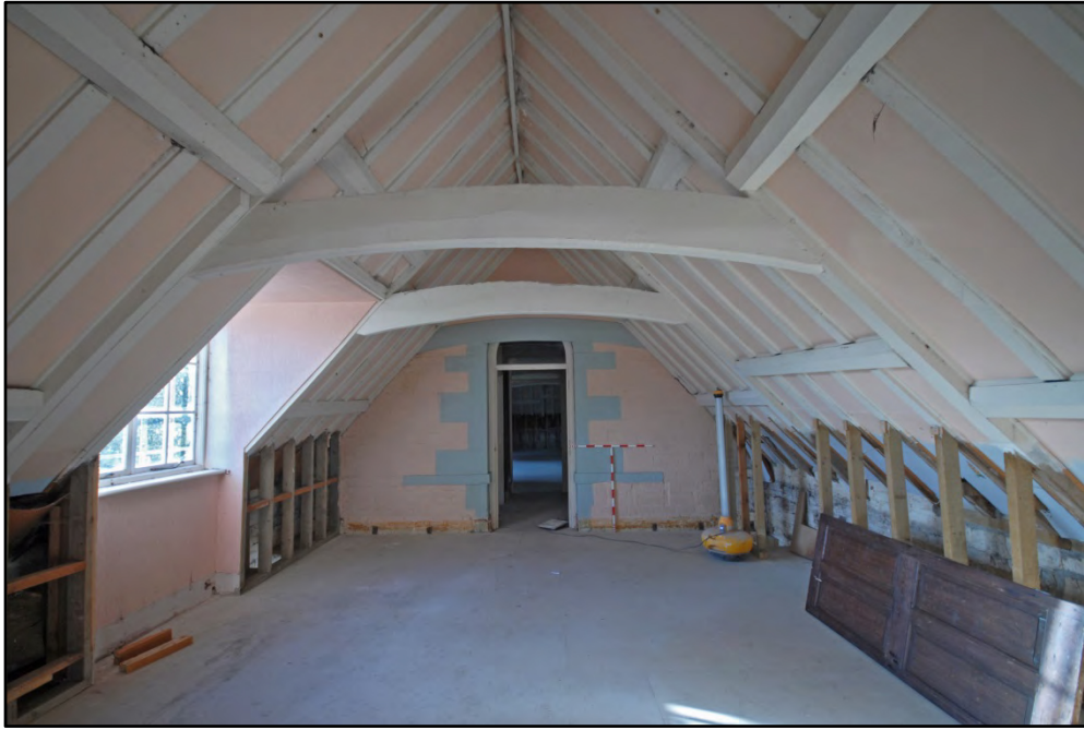
Room F1, looking west Fig 41
