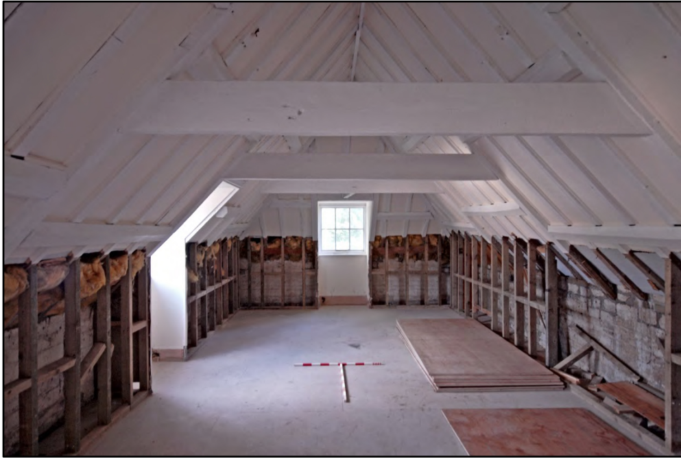
Room F3, looking east Fig 53
