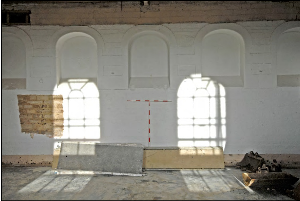
The north wall of room G1, showing the arched recesses Fig 17
