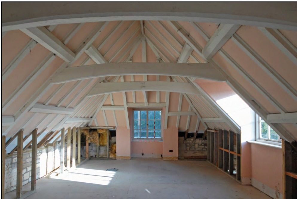
Room F1, looking east Fig 40
