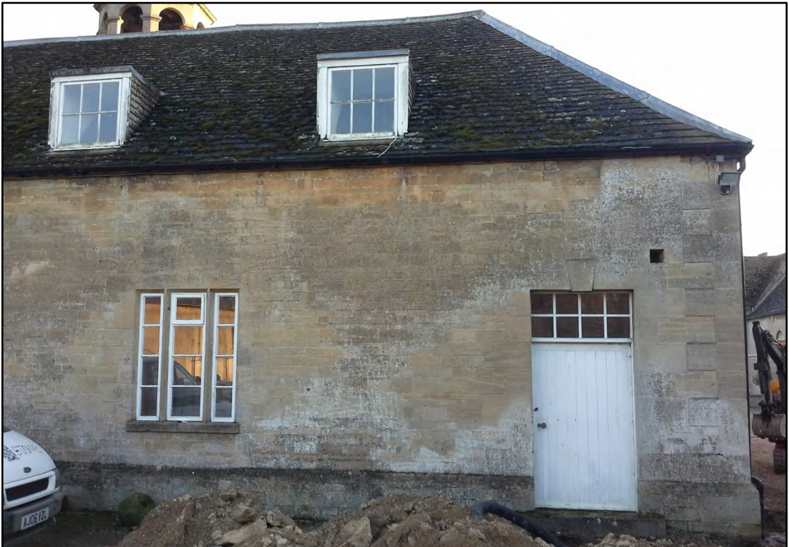
Detail of the north elevation Fig 5
