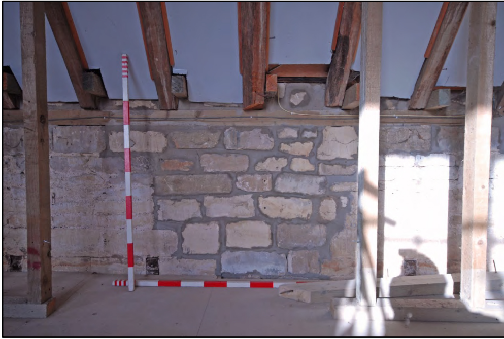
Detail of blocking opposite the easternmost tie beam Fig 45
