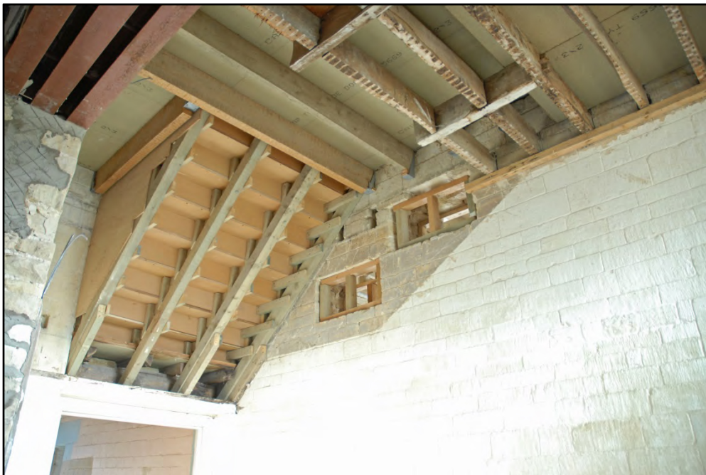
The underside of the stair, looking north-east Fig 12
