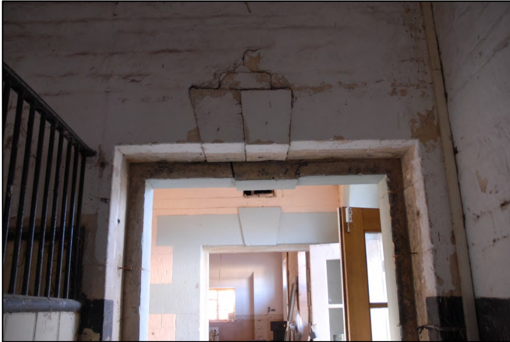
Detail of door header styles and keystones at ground floor Fig 13
