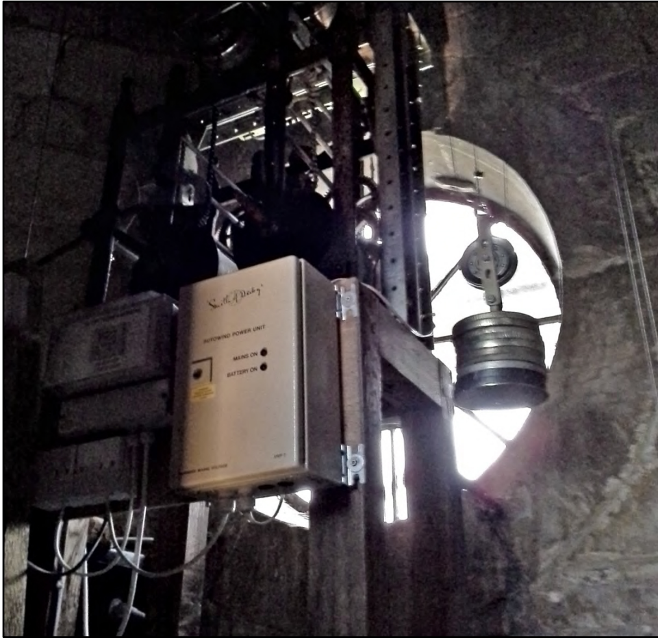
The clock mechanism, prior to removal Fig 37
