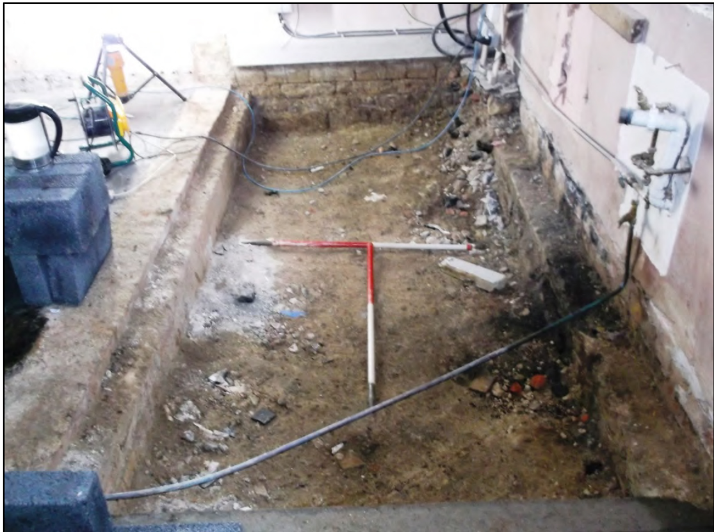
Trench 2, looking south. Fig 64
