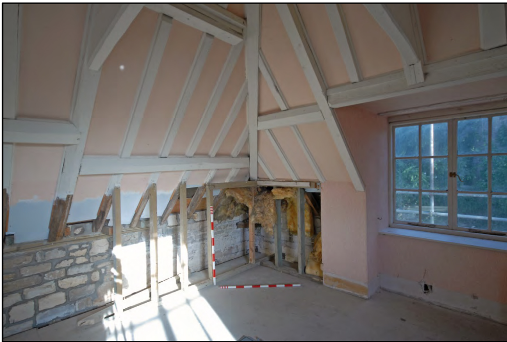
Room F1, detail of the joinery around the east hip, looking north-east Fig 42
