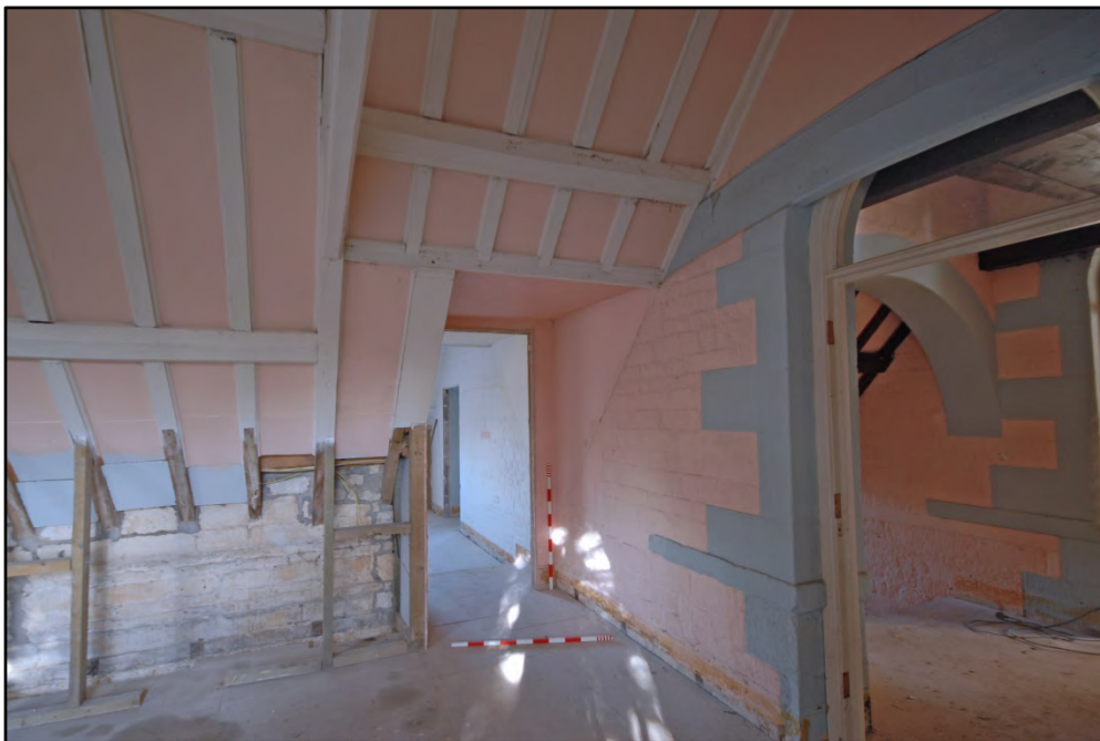
The doorway between rooms F2 and F4, looking north Fig 50
