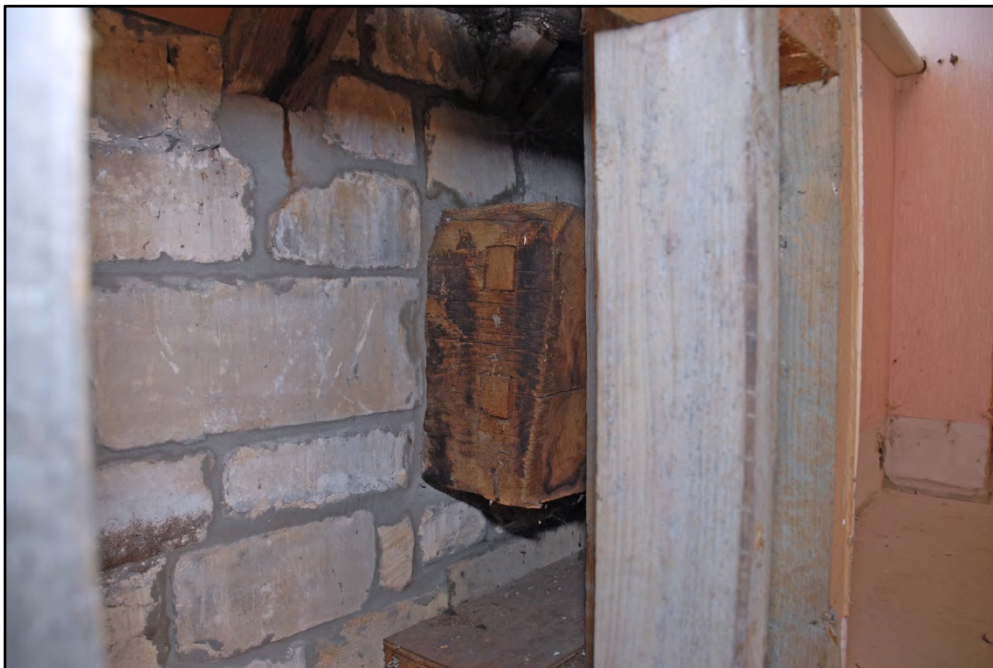
Detail of former tie beam with square pegs Fig 44
