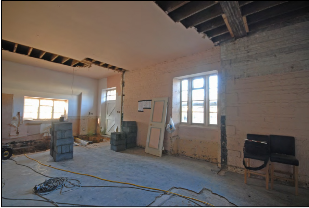
Room G4, looking north-west Fig 31
