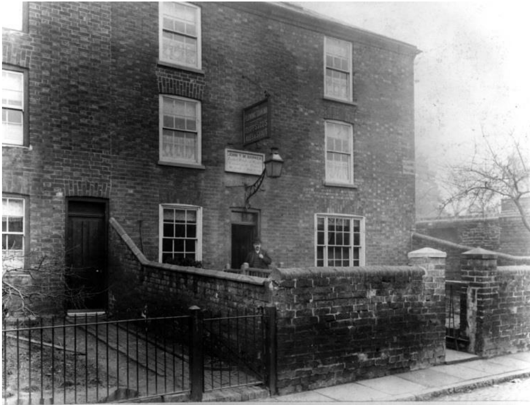
The Flowing Tankard , St John's Terrace in 1894, looking north-east Fig 5
