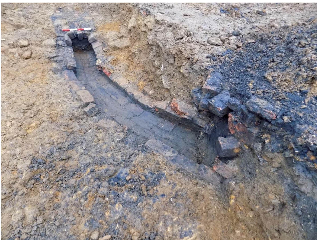
Brick culvert 148, looking west Fig 31
