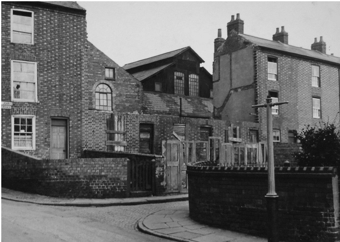
St John's Terrace in 1935, with the foundry behind, looking north-east Fig 4
