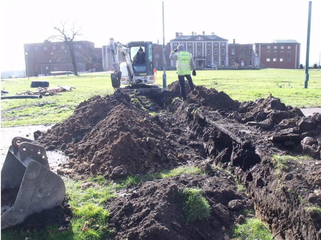
Trench 7 looking south Fig 9
