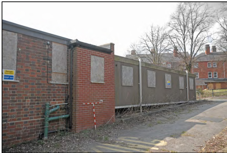
Ward Block 12, brick extension and pre-fabricated unit, looking north-west Fig 34
