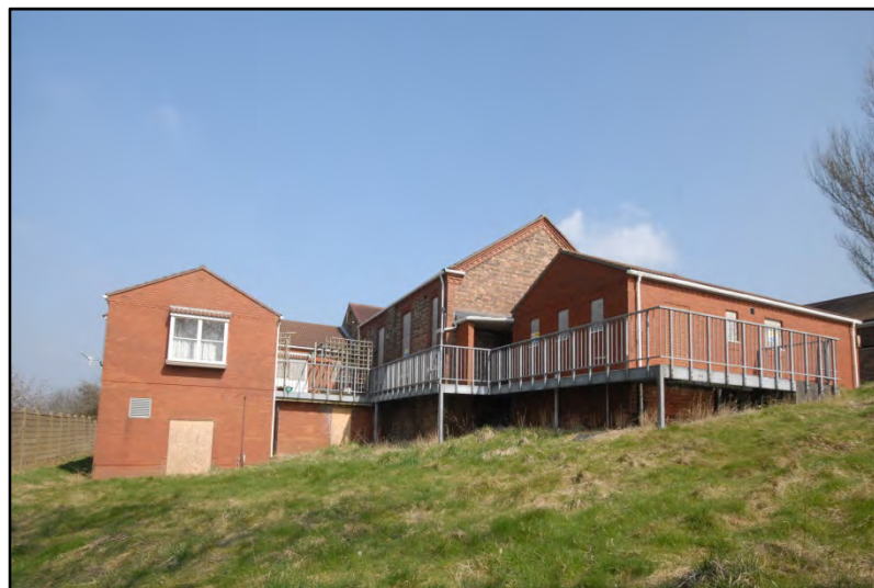
Ward Block 4, the south and west extensions, looking north-east Fig 17
