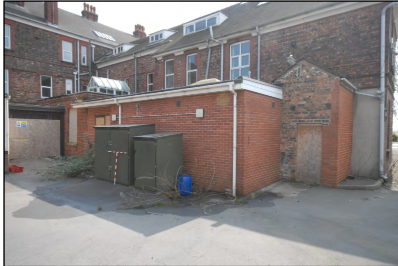
Administration, WC extension, looking south-east Fig 3
