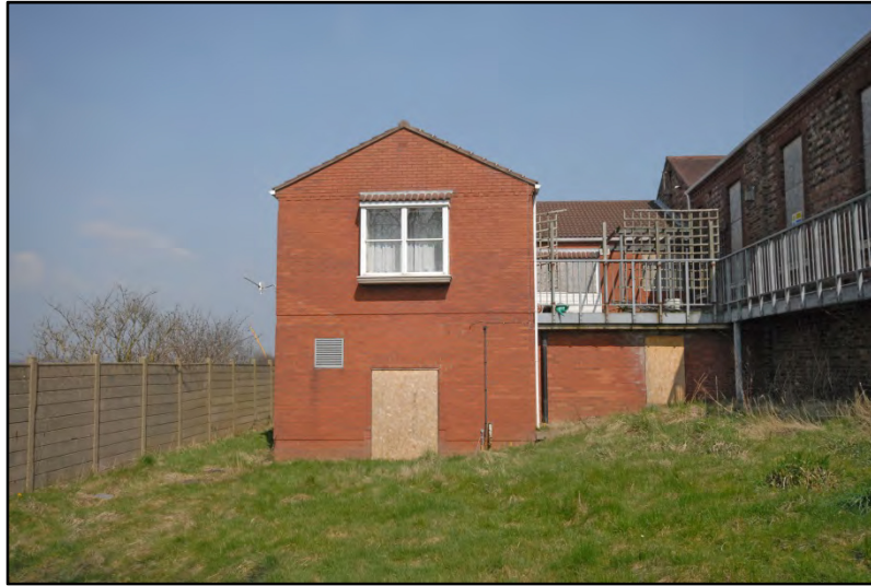
Ward Block 4, the west extension, looking north Fig 18
