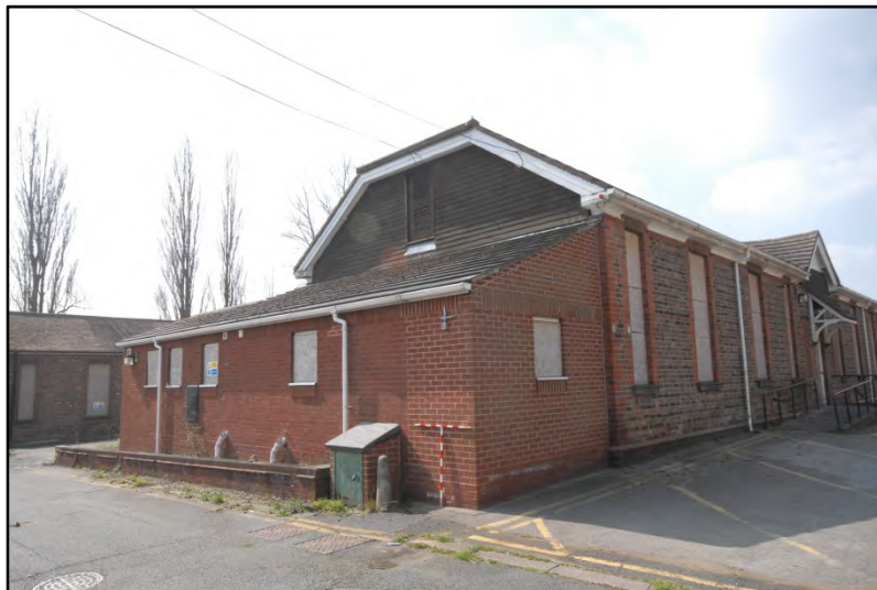
Ward Block 3, east extension, looking south-west Fig 8
