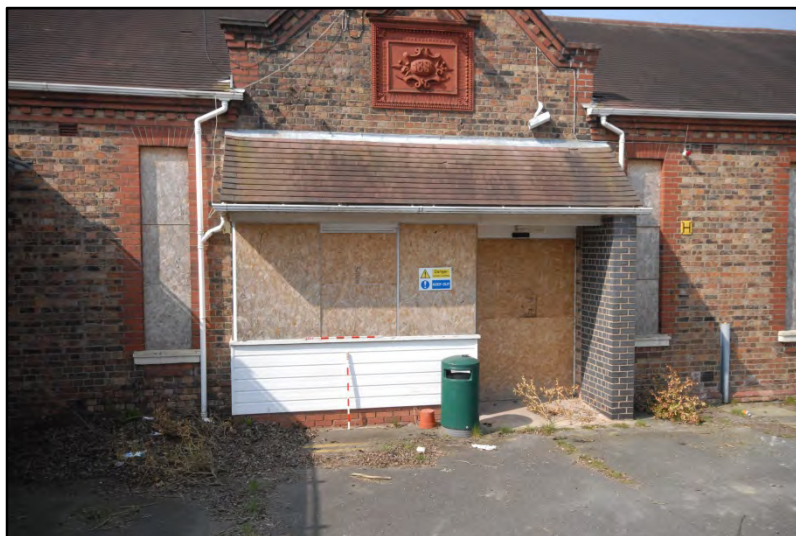
Ward Block 4, 1980s entrance, looking west Fig 14
