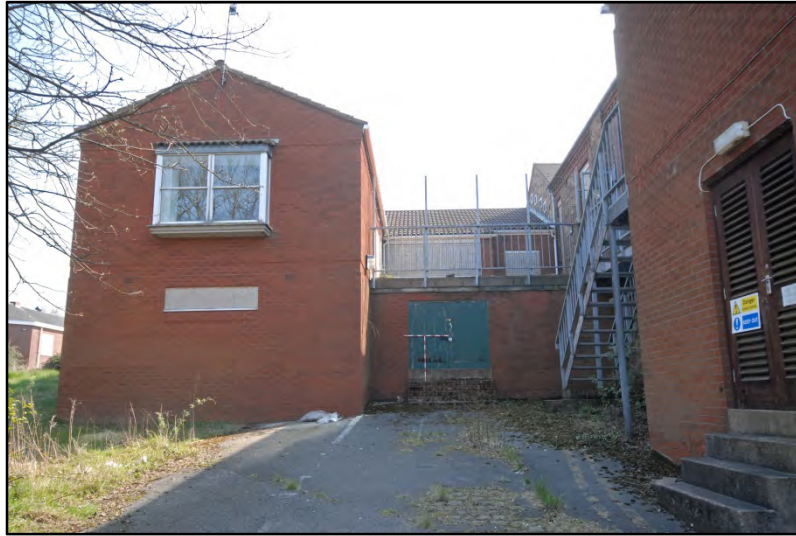
Ward Block 6, the north and west extensions, looking east Fig 27
