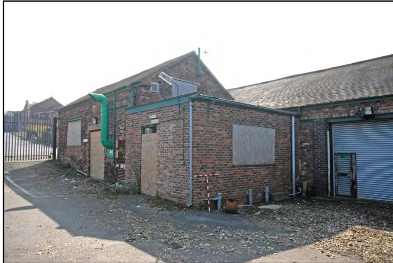
Workshops, north WC extension, looking south-east Fig 39
