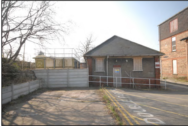
Garage, looking south Fig 45
