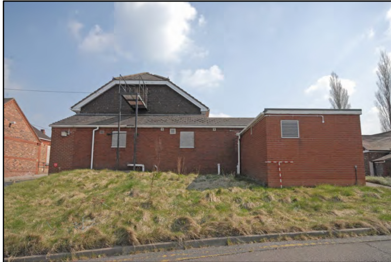
Ward Block 3, the west extension, looking east Fig 12
