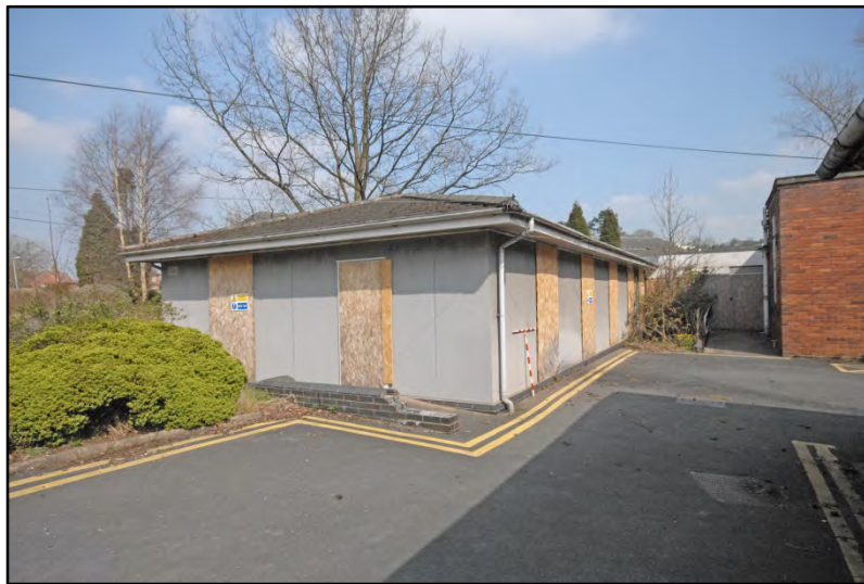
Ward Block 19, west wing of north extension, looking north-east Fig 37
