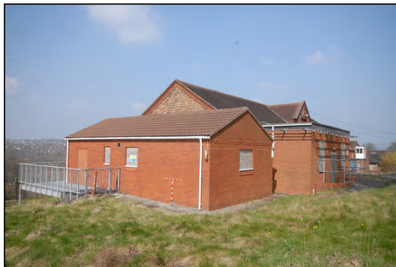
Ward Block 4, south extension, looking north-west Fig 16
