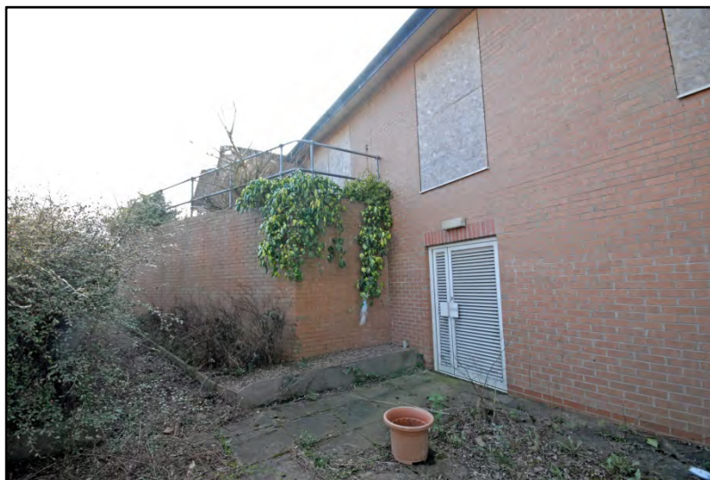
Wards 10 & 11, the north extension, looking south-east Fig 32
