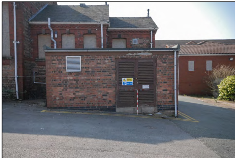
Ward Block 7, north boiler house, looking south Fig 29
