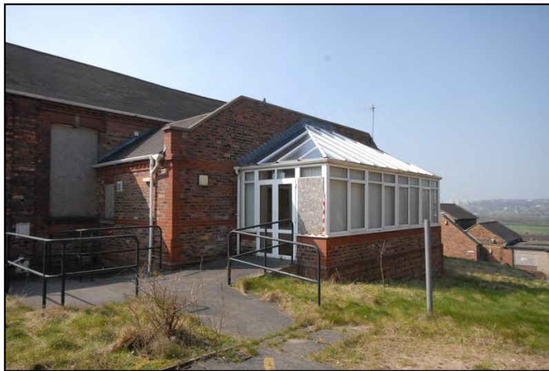
Ward Block 5, the north extension and conservatory, looking south-west Fig 19
