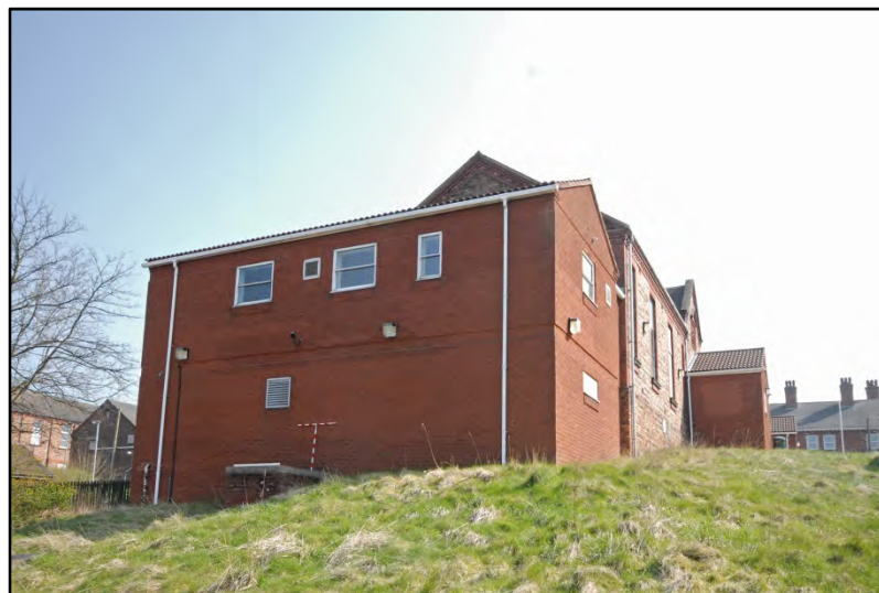
Ward Block 6, the west extension, looking east Fig 26
