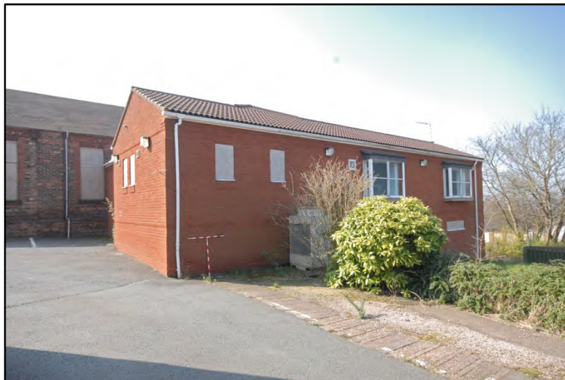
Ward Block 6, the north extension, looking south-west Fig 23
