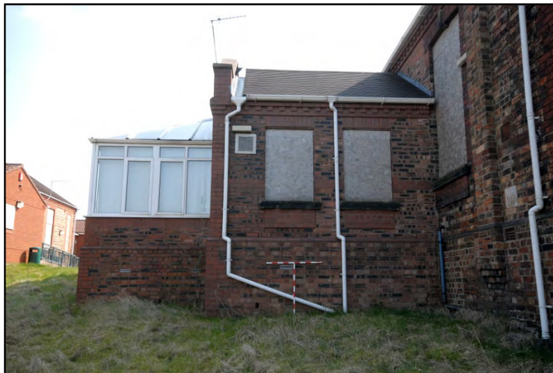
Ward Block 5, the north extension and conservatory, looking east Fig 20
