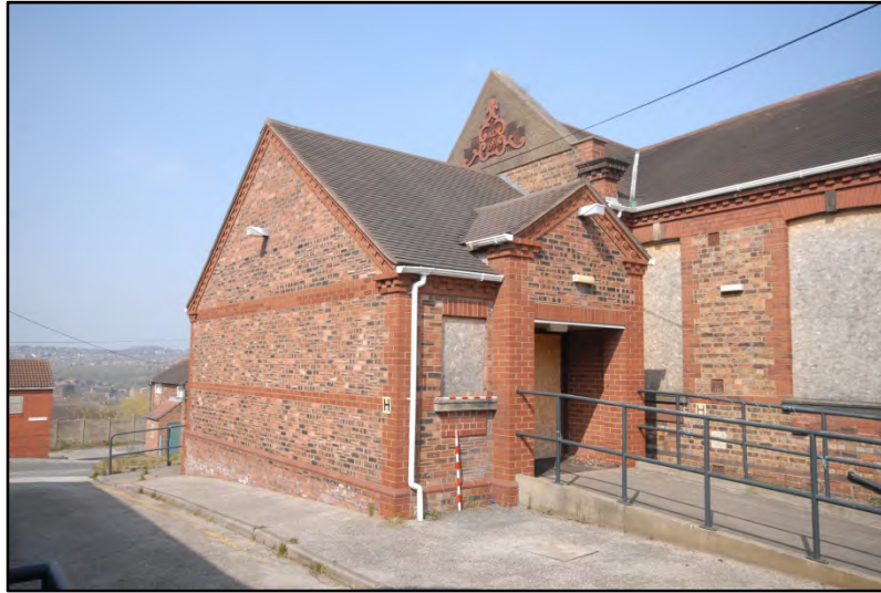
Ward Block 5, the south entrance, looking north-west Fig 21
