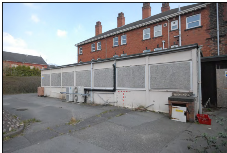
Administration, Kitchen extension, looking north-east Fig 4
