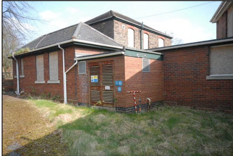
Ward Block 2, boiler house, looking north-east Fig 6
