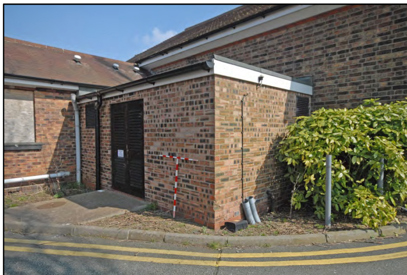
Laundry, the east boiler house, looking north-east Fig 38
