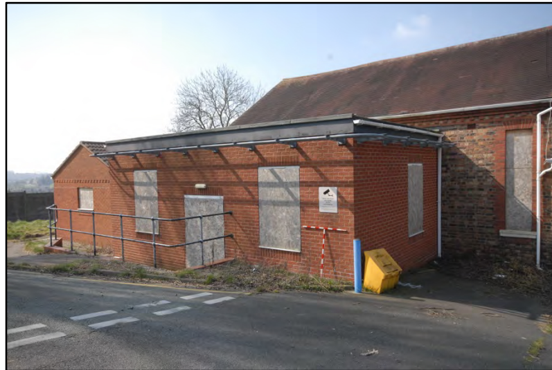
Ward Block 4, east extension, looking south-west Fig 15
