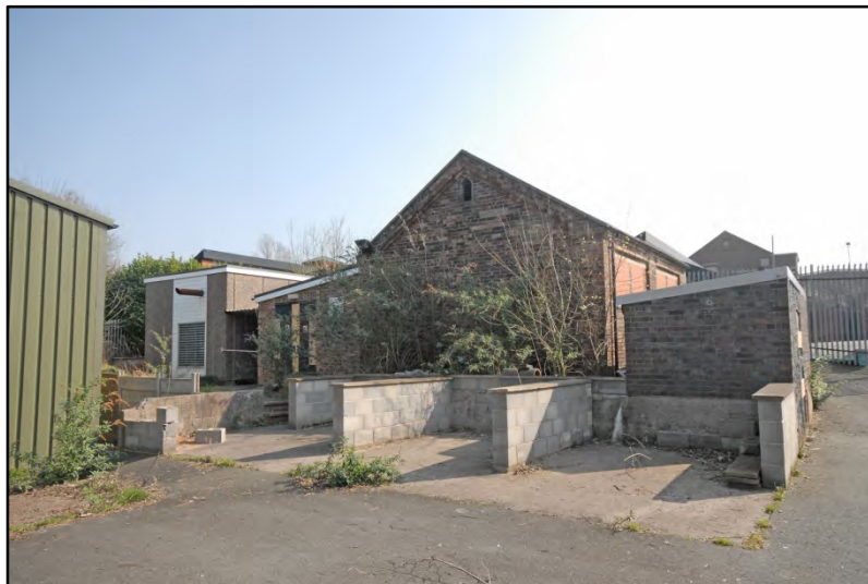
Breeze block bays, looking north-east Fig 52
