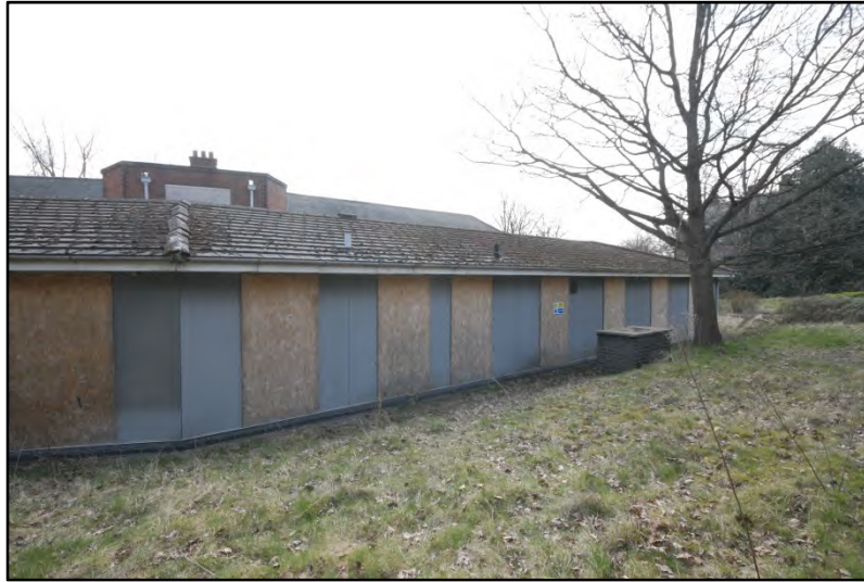
Ward Block 19, west wing of north extension, looking south-west Fig 36
