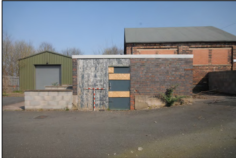
Store room and Shed, looking north Fig 51
