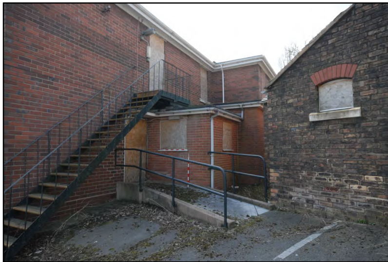
Ward Block 2, extension, looking south-west Fig 7
