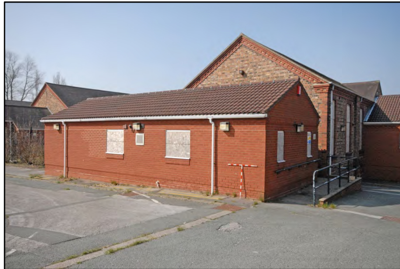
Ward Block 6, the east extension, looking west Fig 24
