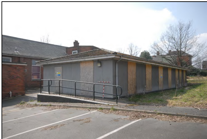
Ward Block 19, east wing of north extension, looking south-west Fig 35
