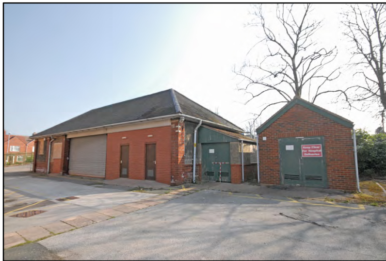
Garage and stores, looking north-east Fig 46
