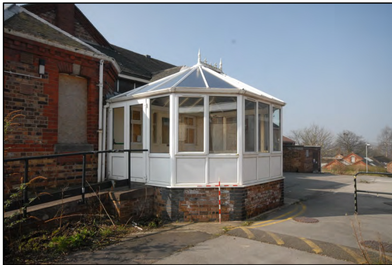
Ward Block 7, the north conservatory entrance, looking south-west Fig 28
