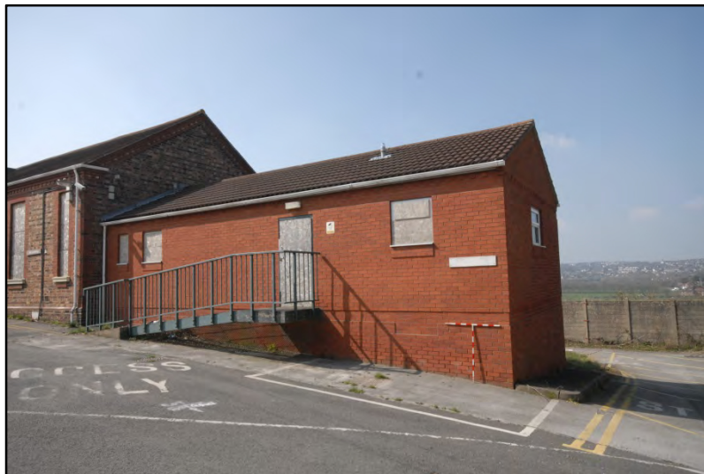
Ward Block 4, the north extension, looking west Fig 13
