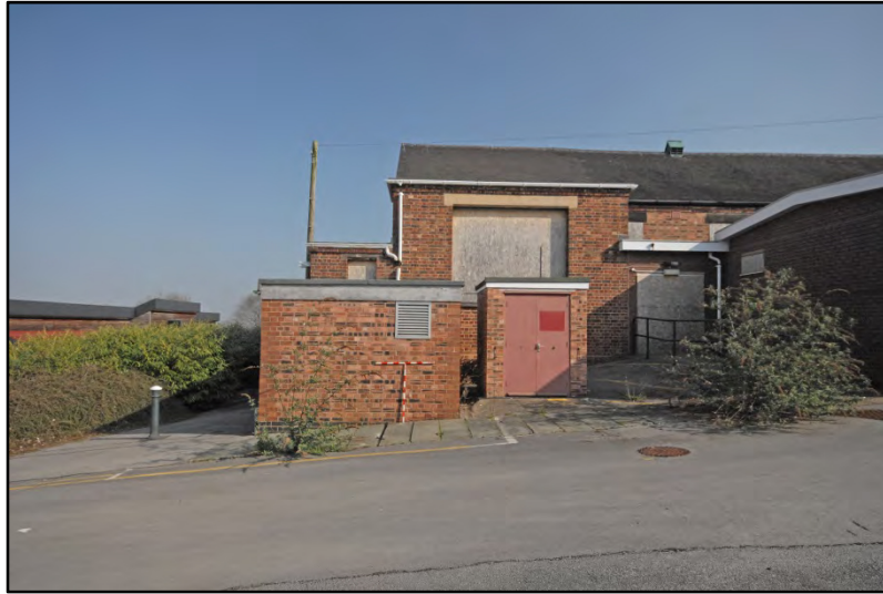
Day Hospital, boiler house and electrical room, looking north Fig 42
