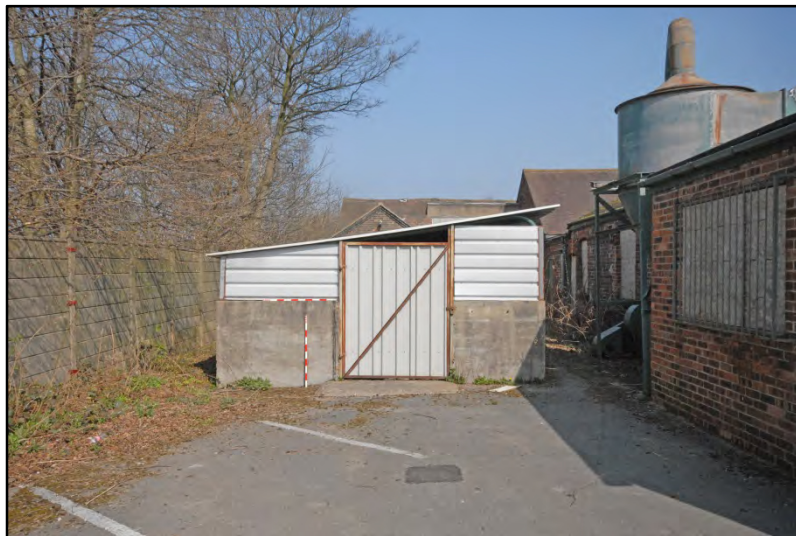
Workshops, detached garage/shed, looking north Fig 40
