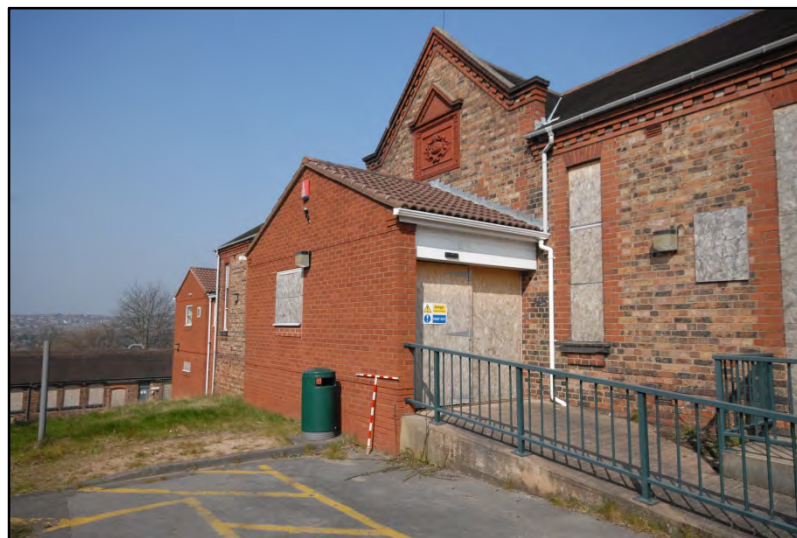
Ward Block 6, south entrance, looking north-west Fig 25
