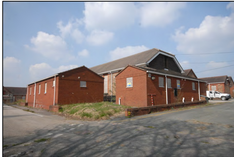
Ward Block 3, the east and south extensions, looking north-west Fig 9
