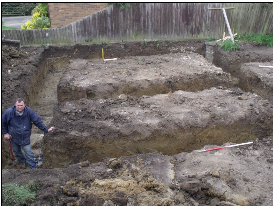
The southern trench foundations, looking south-west Fig 10
