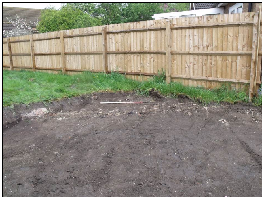
Rubble-filled trench, looking north Fig 6
