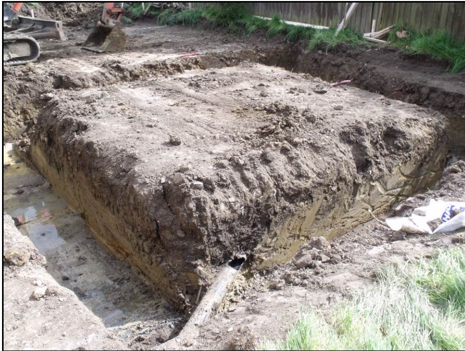
The north-western foundation trenches, looking south Fig 9
