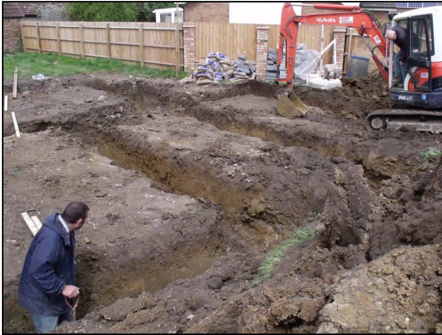
The north-eastern trench foundations, looking north Fig 11
