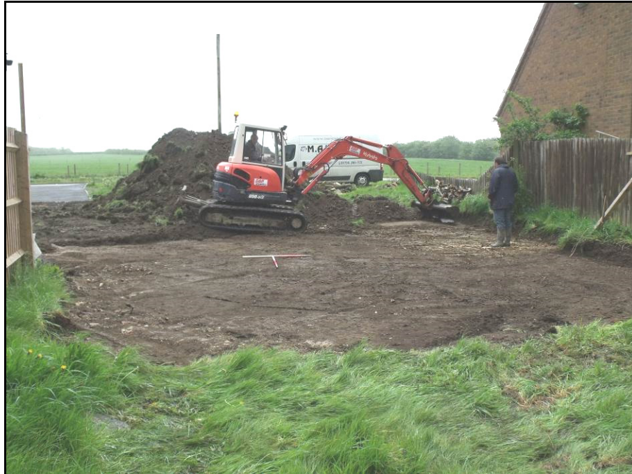
Footprint of house stripped, looking south-east Fig 5
