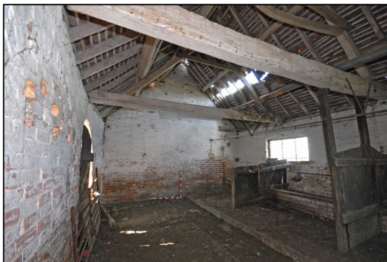
Stable 1, west range, looking south-west Fig 12
