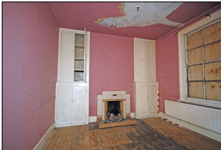
The Farmhouse, ground floor, room G1 Fig 24
