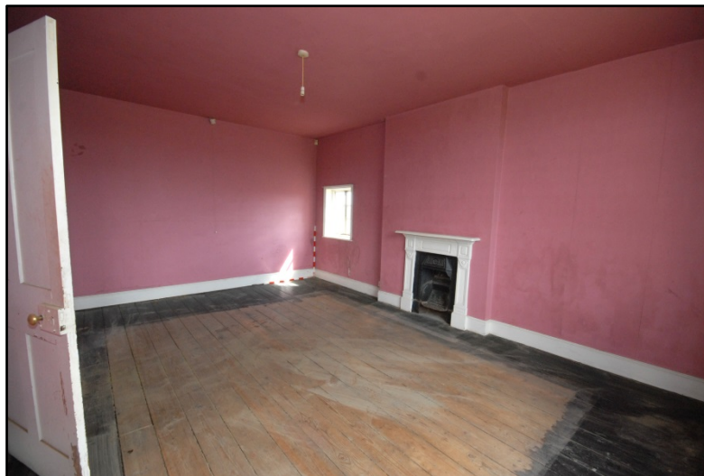
The Farmhouse, first floor, room F1 Fig 27
