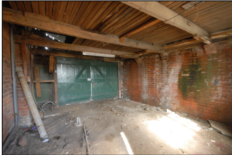
Garage 2, interior, looking north-east Fig 31
