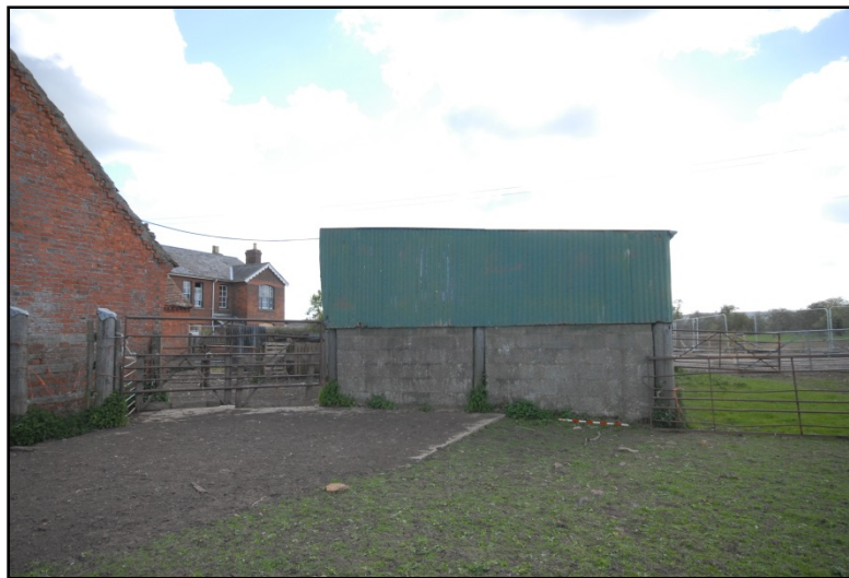
Cow Shed, looking south-east Fig 8
