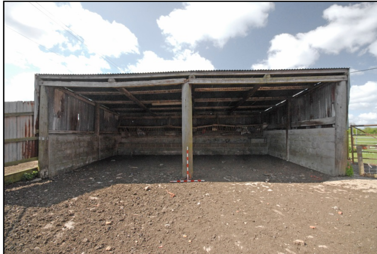
Cow Shed, looking north-west Fig 7
