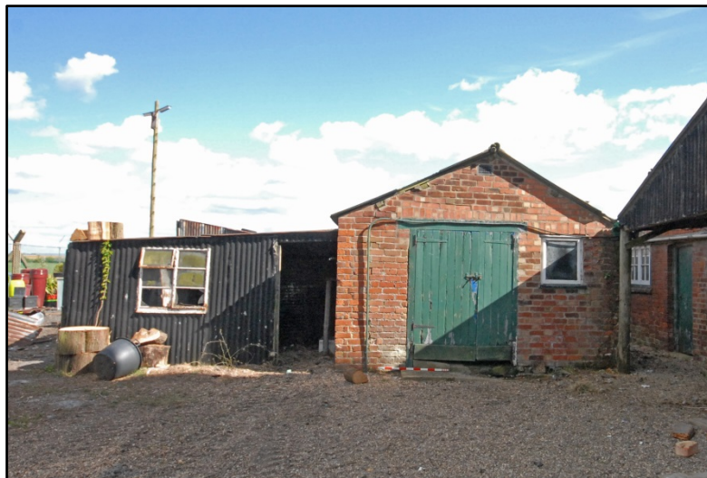
Stable 3 and Chicken Sheds, looking south-east Fig 36
