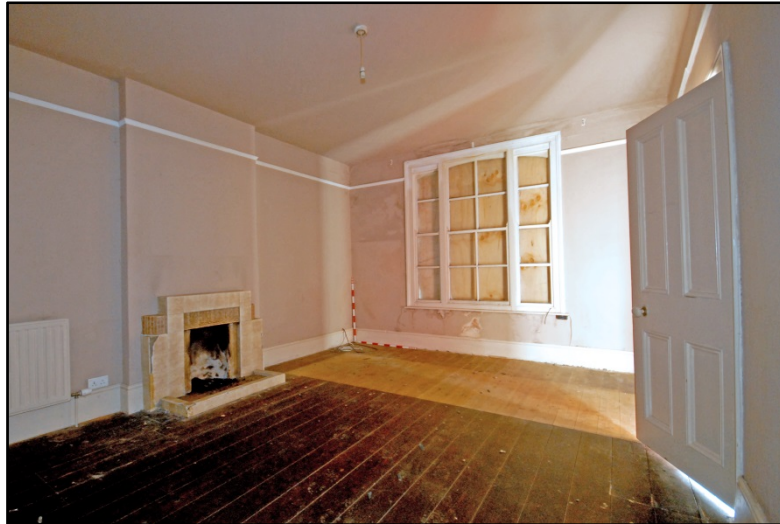
The Farmhouse, ground floor, room G3 Fig 25
