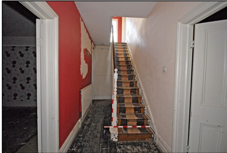
The Farmhouse, ground floor landing Fig 22
