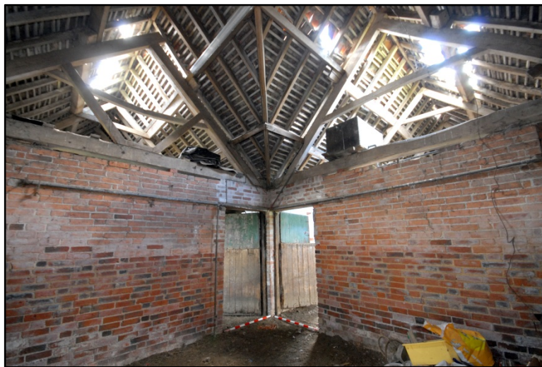
Stable 1, central barn, looking south Fig 14
