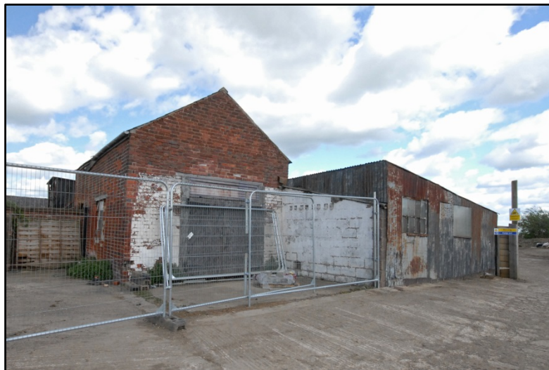
East Barn and Sheds, southern extent, looking east Fig 42
