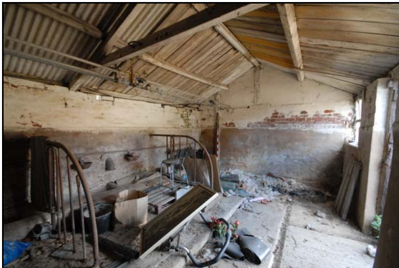
Stable 2, southern room, looking north-east Fig 33
