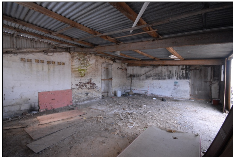
East Barn and Sheds, interior of southern shed, looking north-east Fig 45
