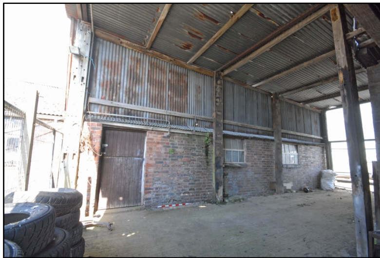
East Barn and Sheds, north shed, looking north toward Stable 3 Fig 47
