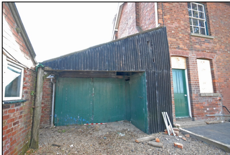
Garage 2, looking south-west Fig 30
