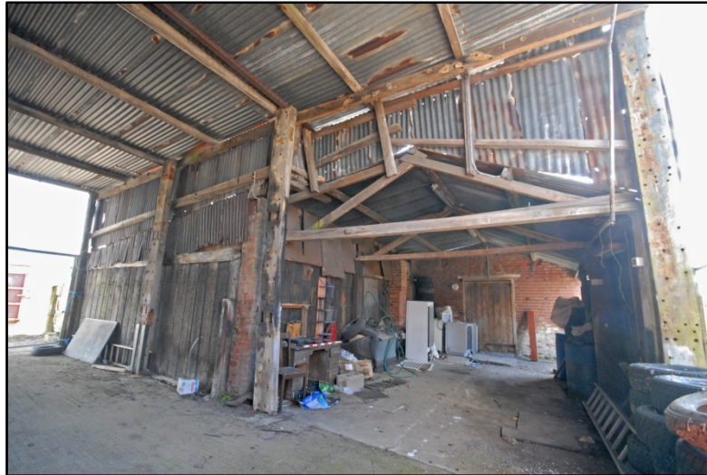
East Barn and Sheds, interior of north shed, looking south Fig 46
