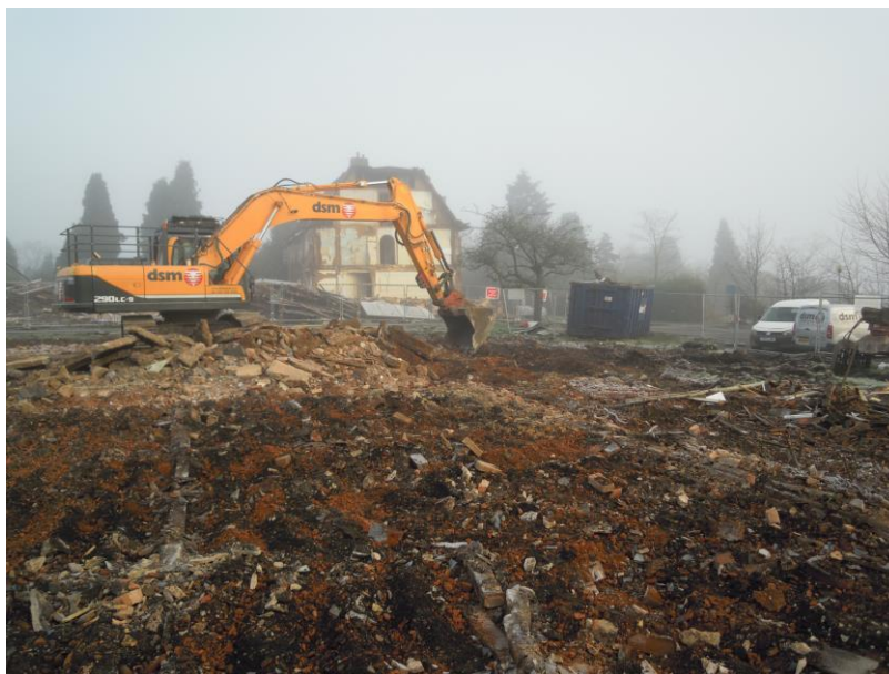
Area of watching brief, pre excavation
