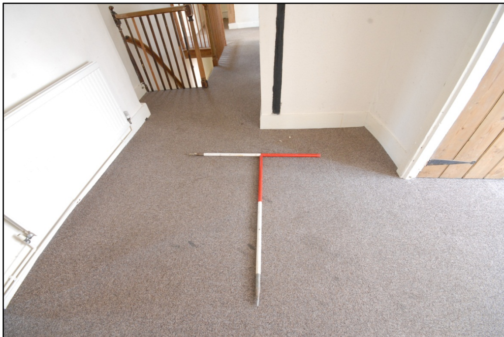
The floor at the investigation area Fig 9
