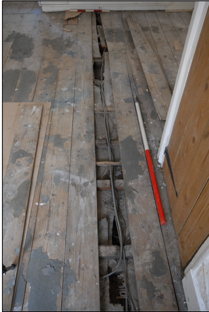
Joists and floorboards underneath the current floorboards, looking west Fig 14
