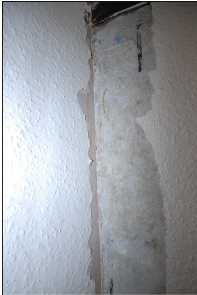
Older plaster under modern woodchip wallpaper Fig 12
