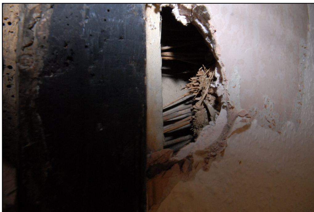
Detail of the straw and daub below the plasterboard Fig 11
