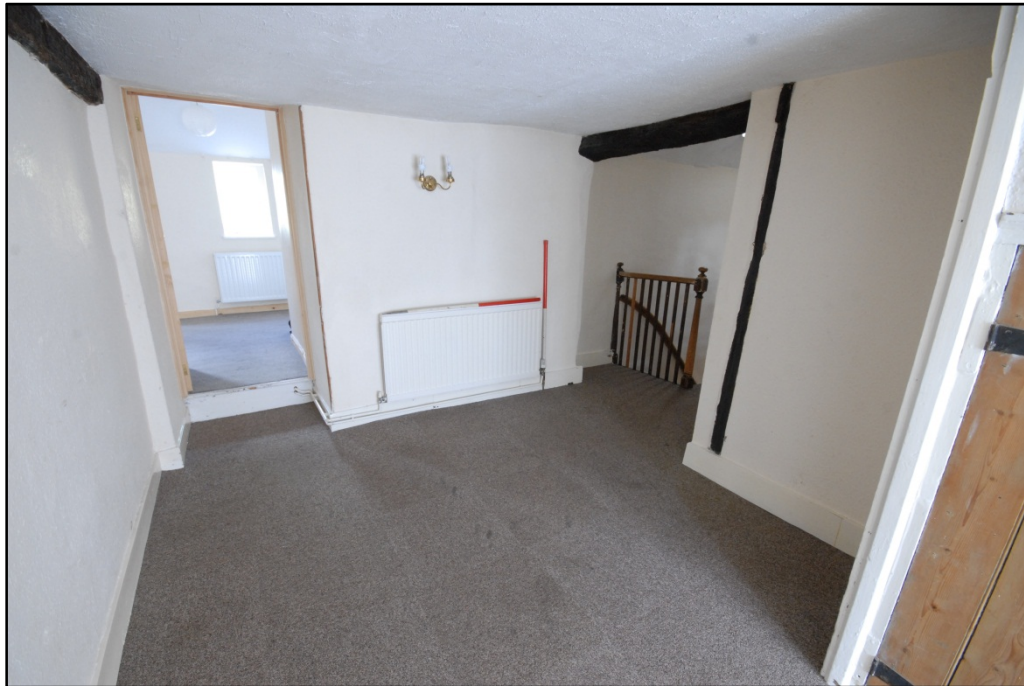
The investigation area, looking north-west Fig 7
