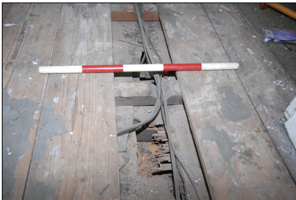
Older joist below 1st set of floor boards, looking west Fig 18
