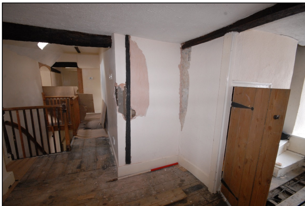
The investigation area after exposure of the fabric, looking north-east Fig 10
