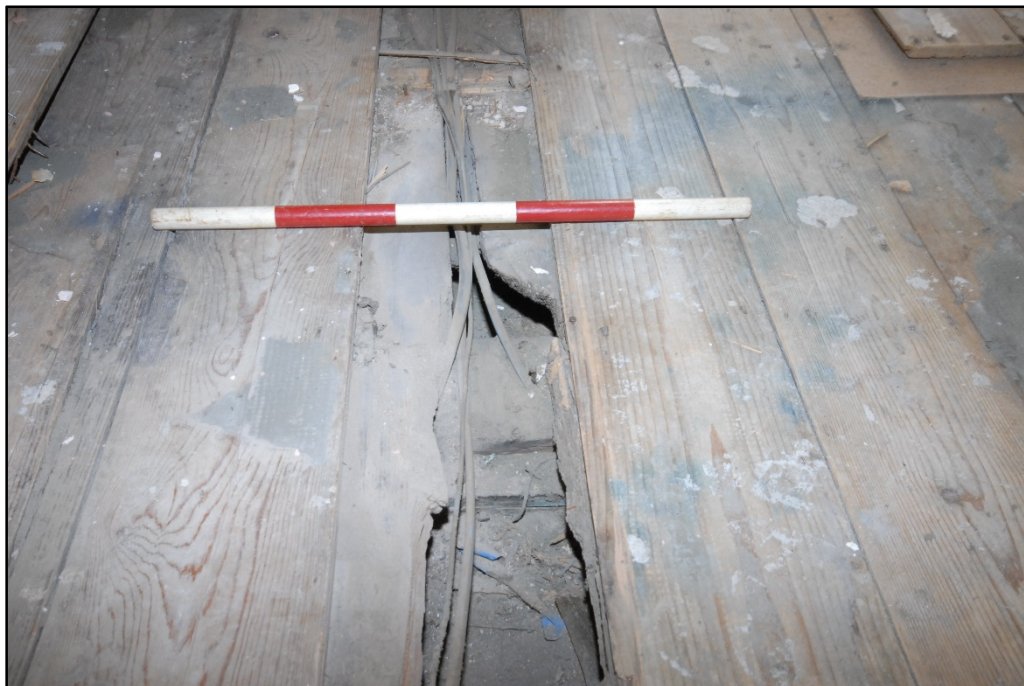
Older joist below 1st set of floor boards, looking east Fig 17
