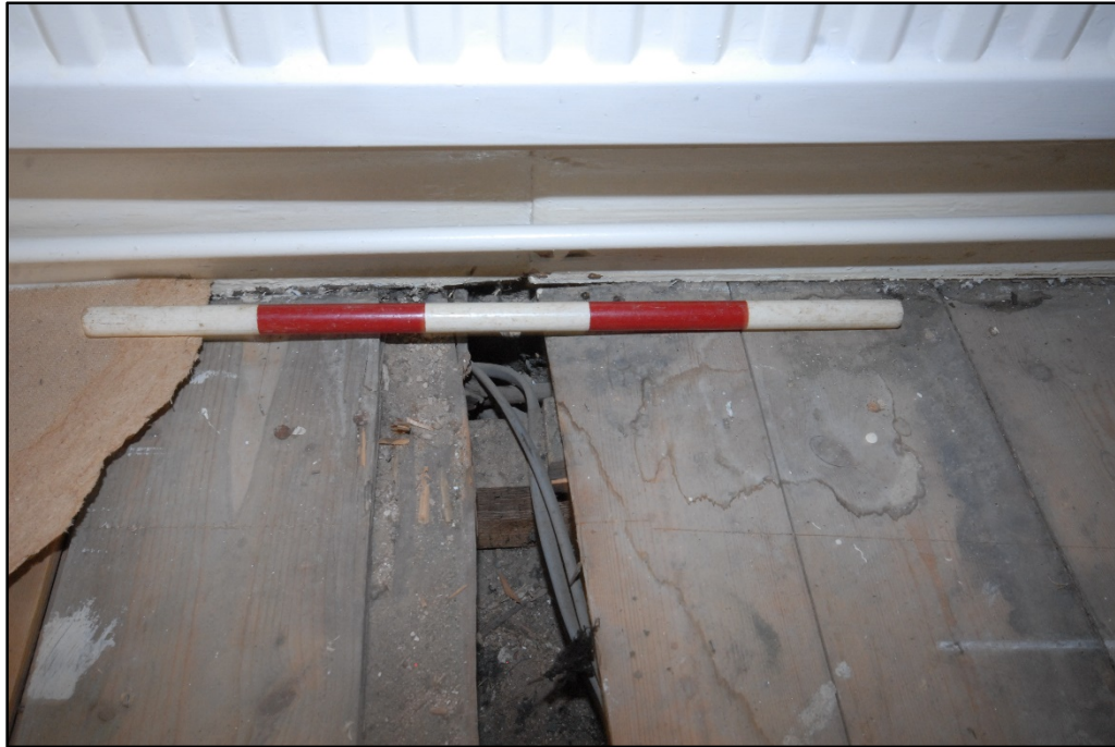
Newer joist, looking west Fig 16
