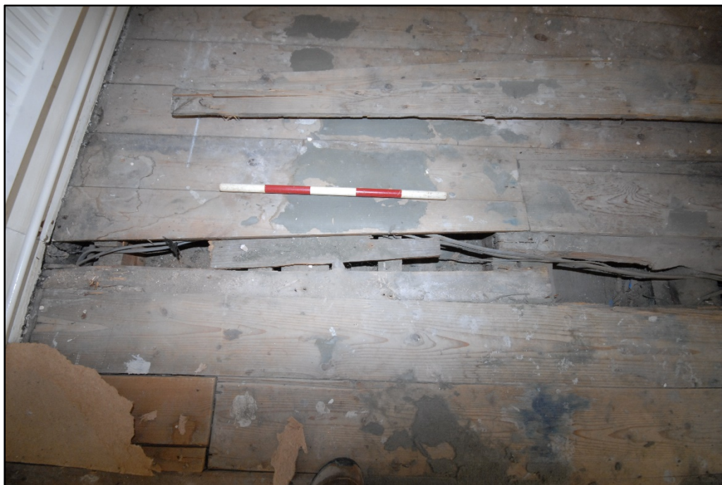
The newer joists, looking north Fig 15
