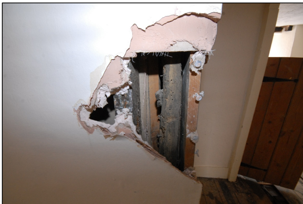
Modern plasterboard wall Fig 13
