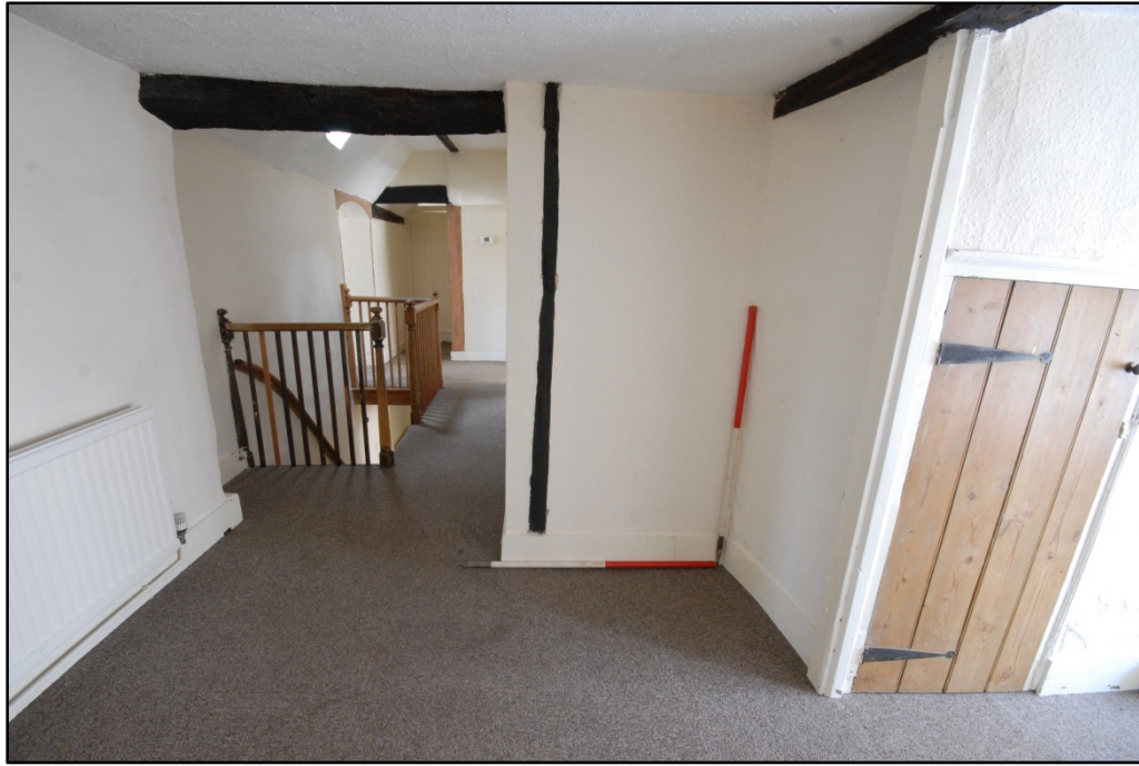
The investigation area, looking north Fig 8
