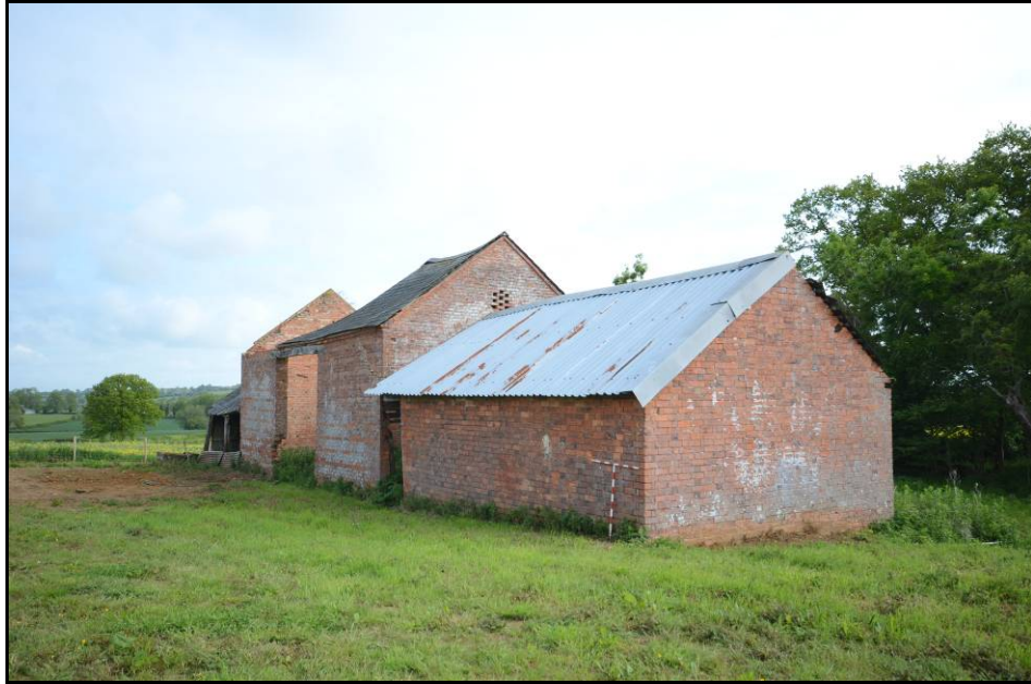
General view of the Stable, looking north-east Fig 22
