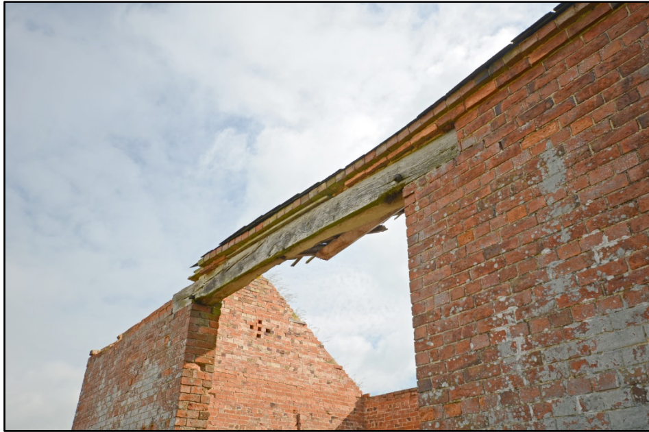
The Barn, detail of timber lintel Fig 16
