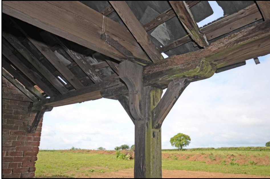
Cart shed, detail of post with decorative supports Fig 12
