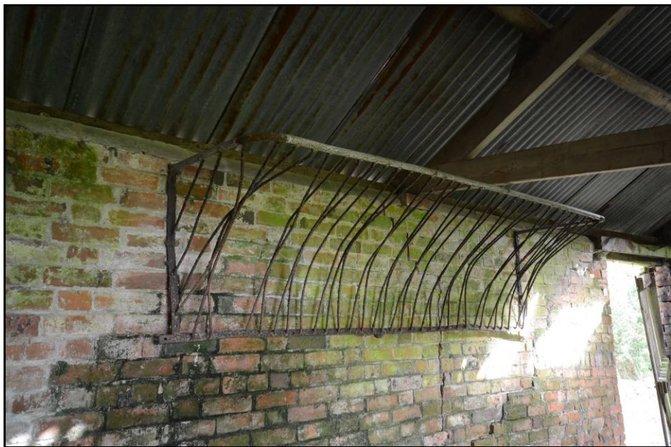
The Cow shed, detail of manger Fig 37
