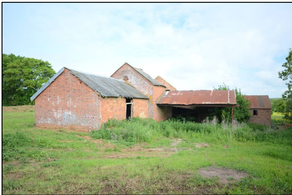
General view of the buildings, looking north-west Fig 29
