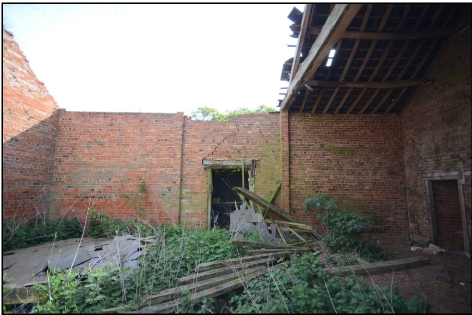
The Barn, interior, looking north-east Fig 17
