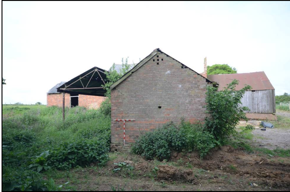
The Cow shed, the east elevation, looking south-west Fig 32
