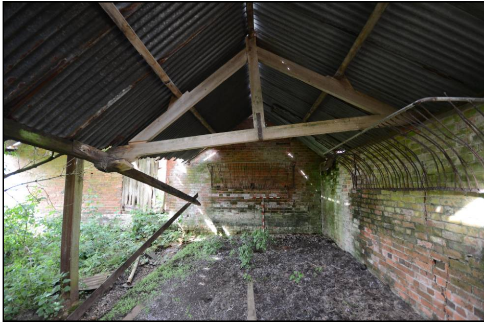
The Cow shed, interior, looking west Fig 36
