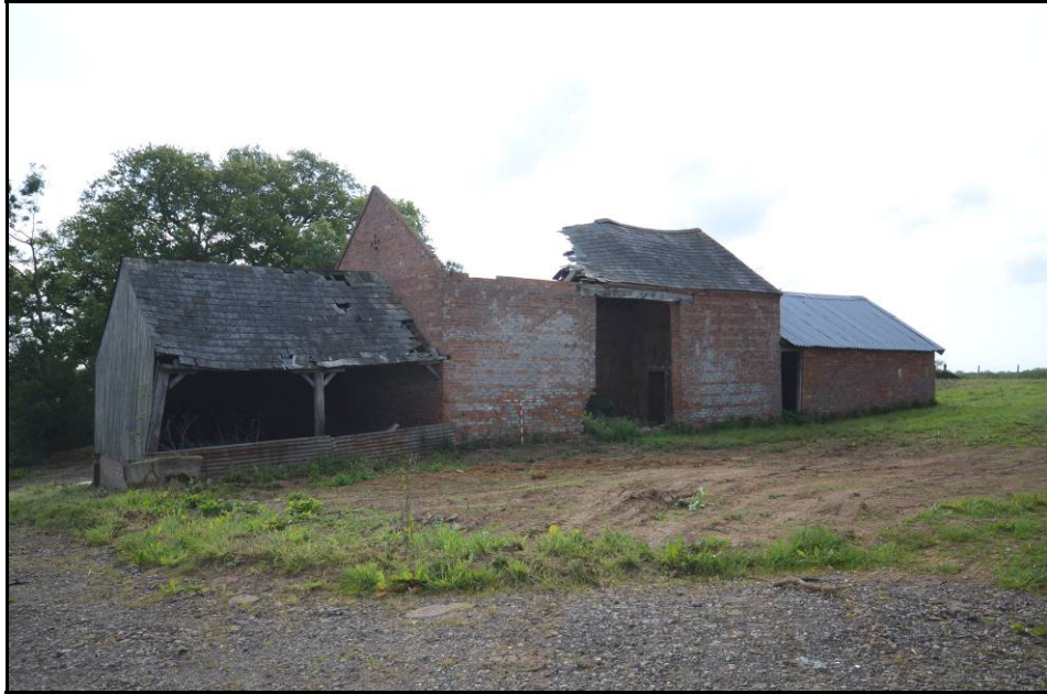
General view of the buildings, looking south-east Fig 8
