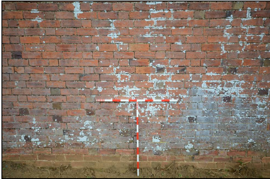
The Stable, detail of the building's construction Fig 28
