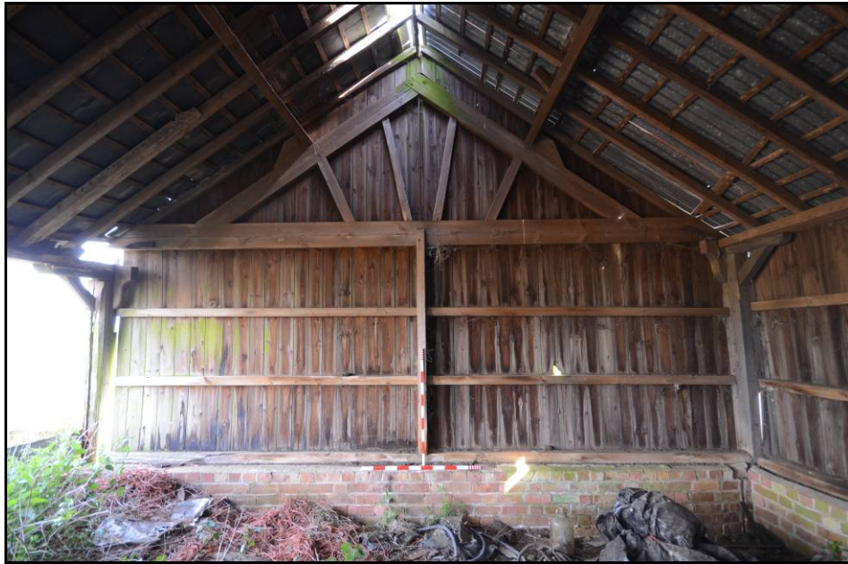
Cart shed, the interior, looking north Fig 14
