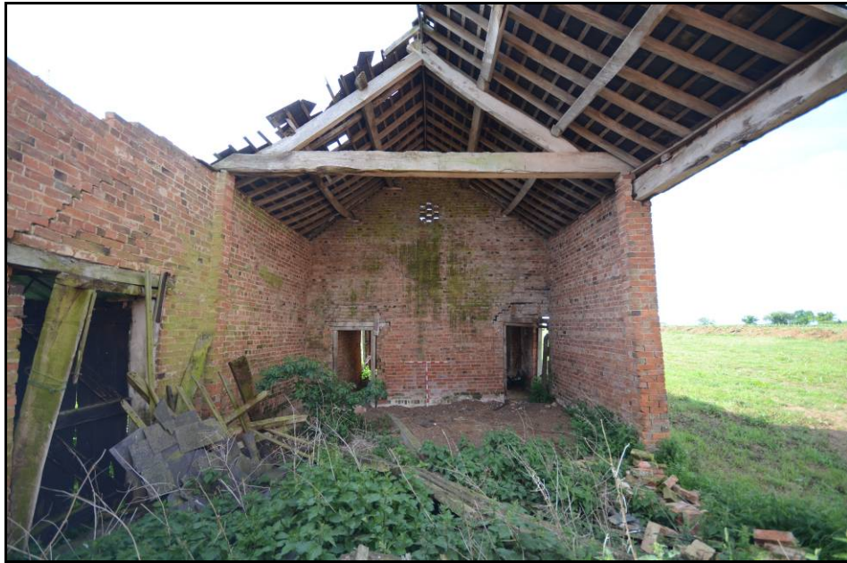
The Barn, interior, looking south Fig 18
