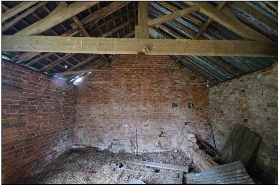
The Stable, interior, looking south Fig 26
