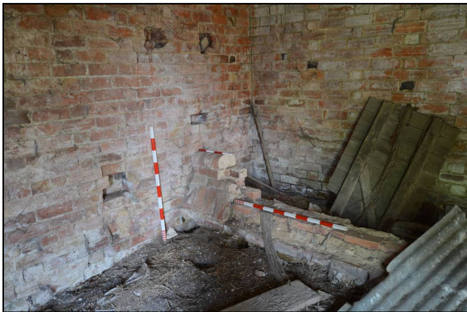
The Stable, detail of brick trough Fig 27
