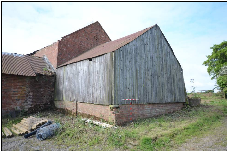
The Cart shed, looking south-west Fig 11
