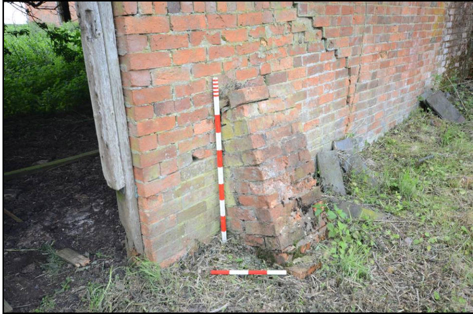
The Cow shed, detail of buttress adjacent to door Fig 34
