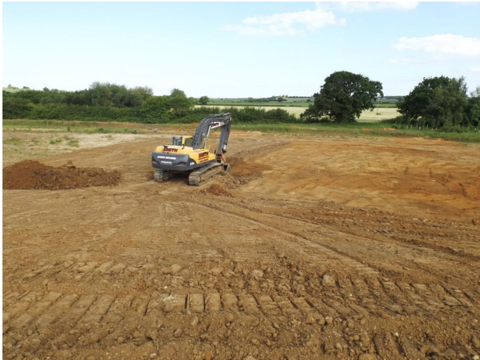
The western side of the stripped area, looking north-west Fig 3
