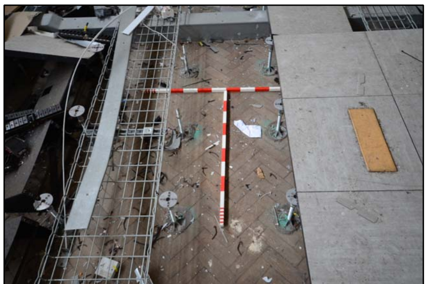
Transmitter Hall 2, detail of modern and original floors Fig 4.3.28
