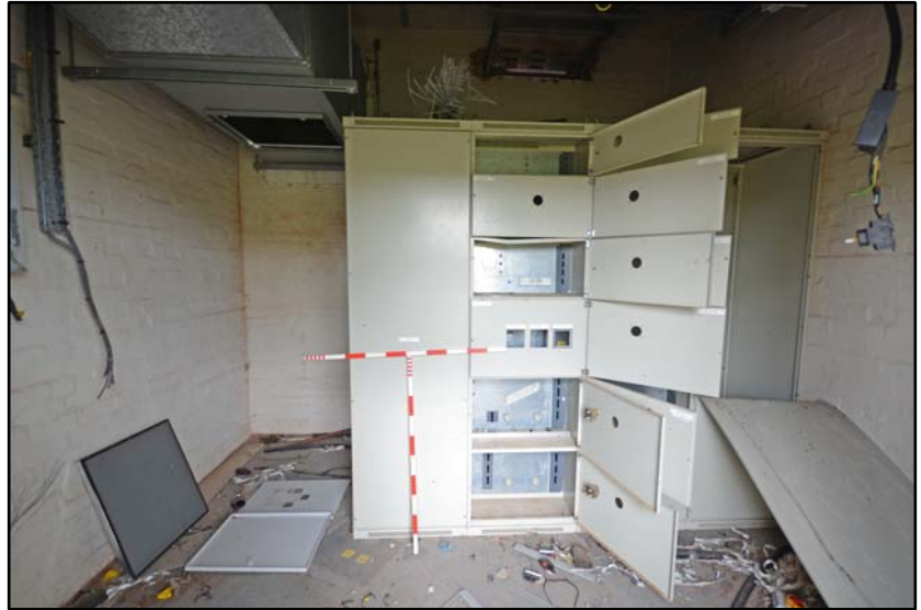
Transformer 2, mounting cabinets within the east rooms Fig 4.6.11
