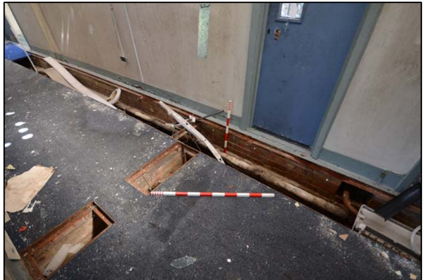
Administration, detail of pipe trench in central corridor Fig 4.4.12
