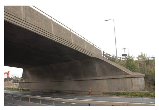
Detail of the inclined tapering haunches, looking north-east (digital ref no 0211) Fig 9
