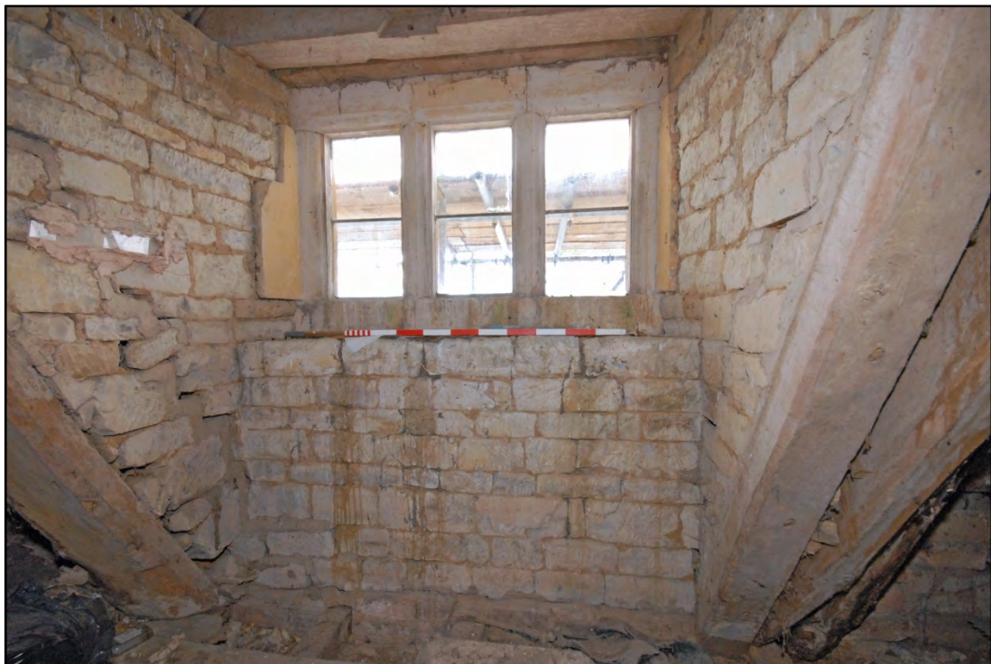
Dormer 1, interior view Fig 19
