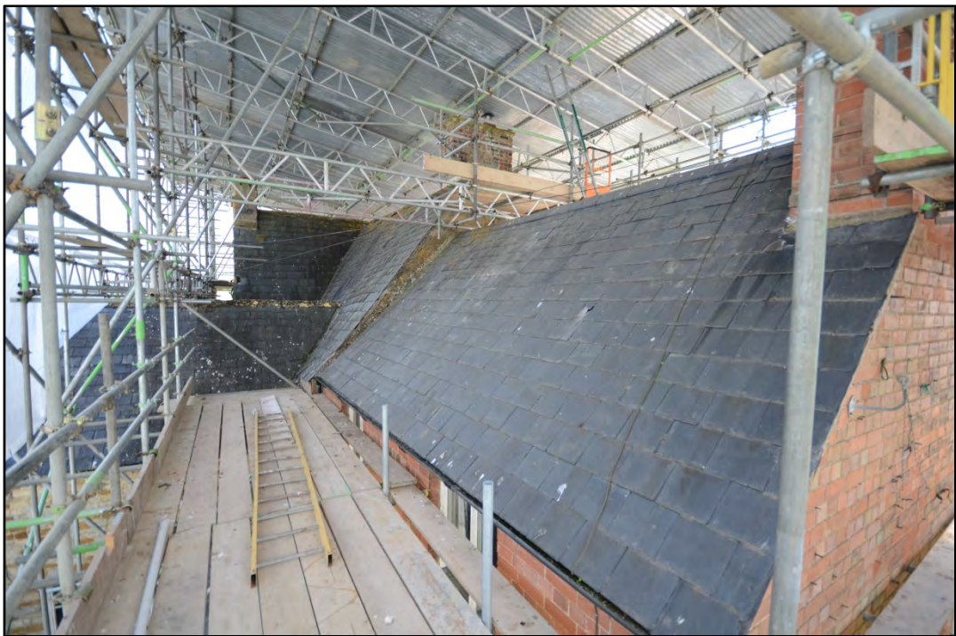
General view of the roof, looking east Fig 3
