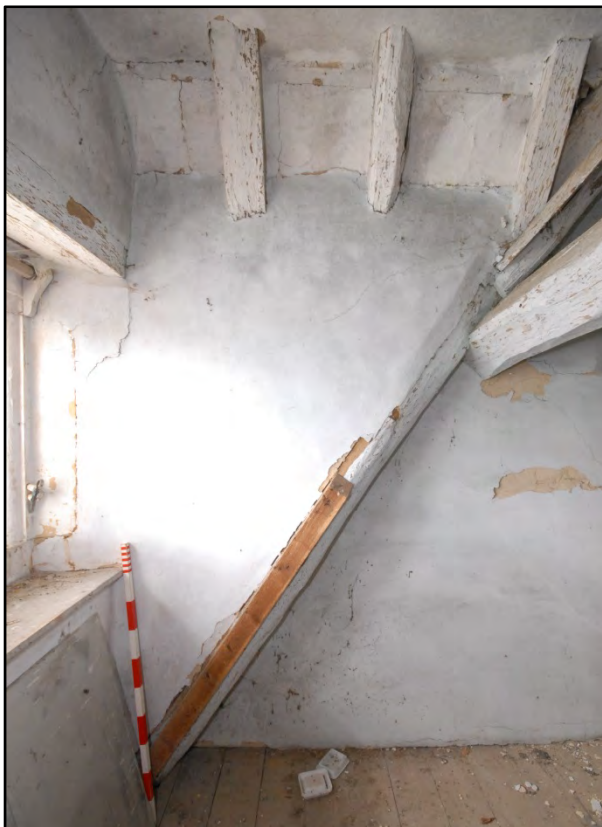
The interior face of the west elevation of Dormer 2 Fig 28
