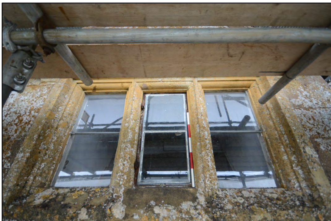
Dormer 2, detail of the window Fig 26
