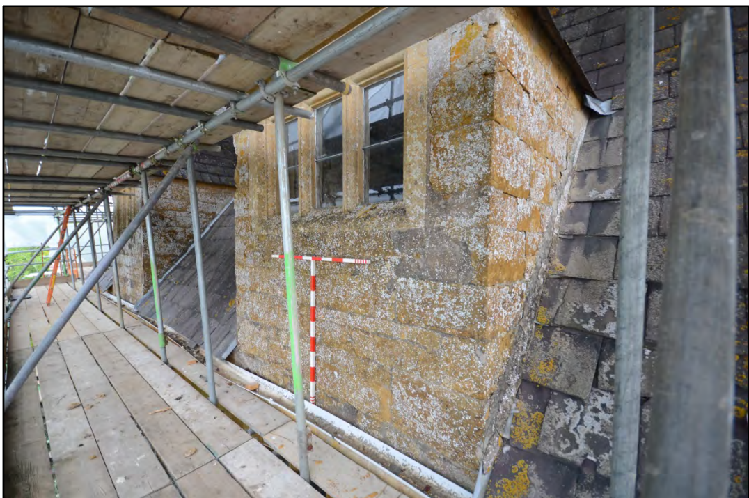
Dormer 1, looking north-west Fig 15
