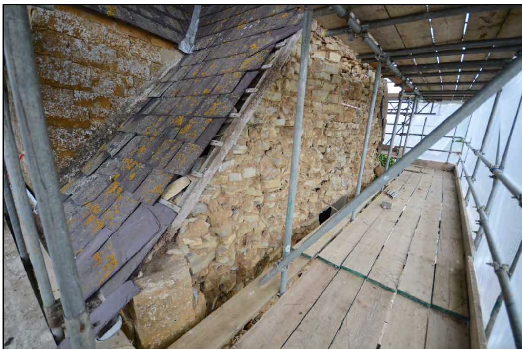
The external face of the south-east gable, looking north Fig 8
