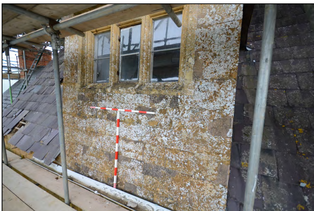
The lower extent of Dormer 2 Fig 23
