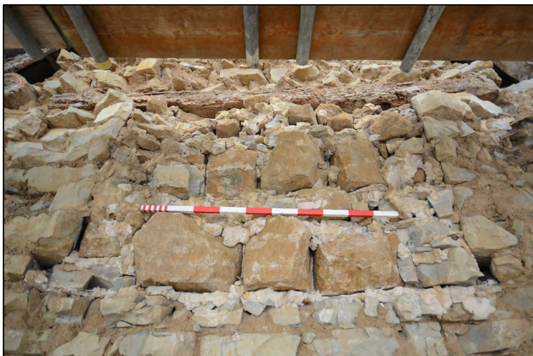
Blocked window in the south-east gable Fig 10
