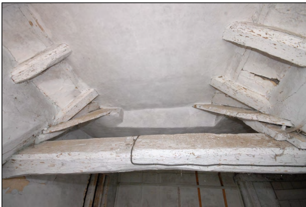
The roof structure of Dormer 2 Fig 30
