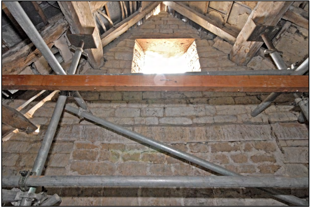
Interior face of the south-east gable Fig 12
