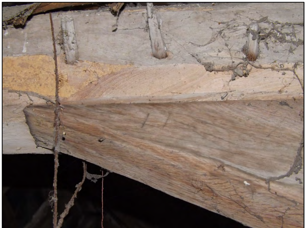
Detail of joinery, with a carpenter's mark central to the image Fig 35
