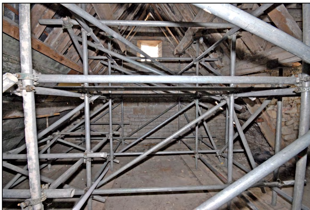
The attic space, looking east to the south-east gable Fig 11
