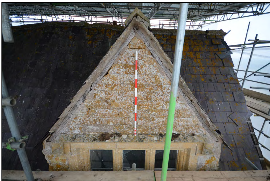
Upper extent of Dormer 1, looking north Fig 16
