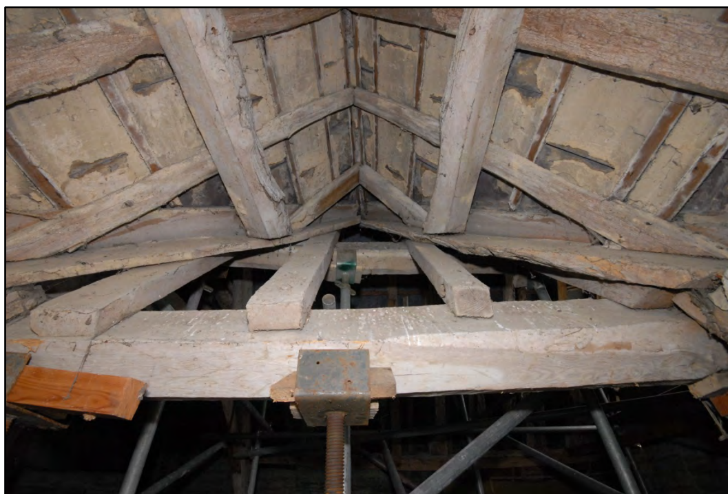
Detail of the Dormer roof structure Fig 21
