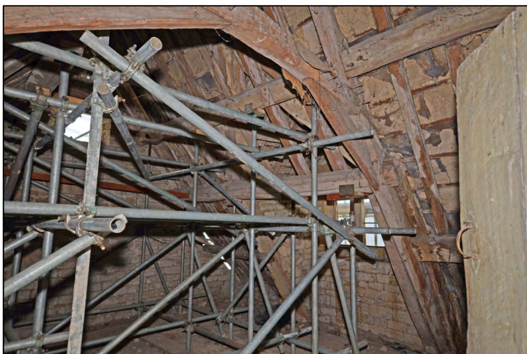
The lower extent of the cruck truss Fig 31
