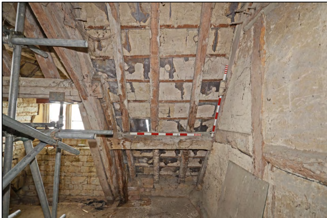
The interior face of the slatework adjacent to Dormer 1, showing remnants of daub on the underside of the slates Fig 6
