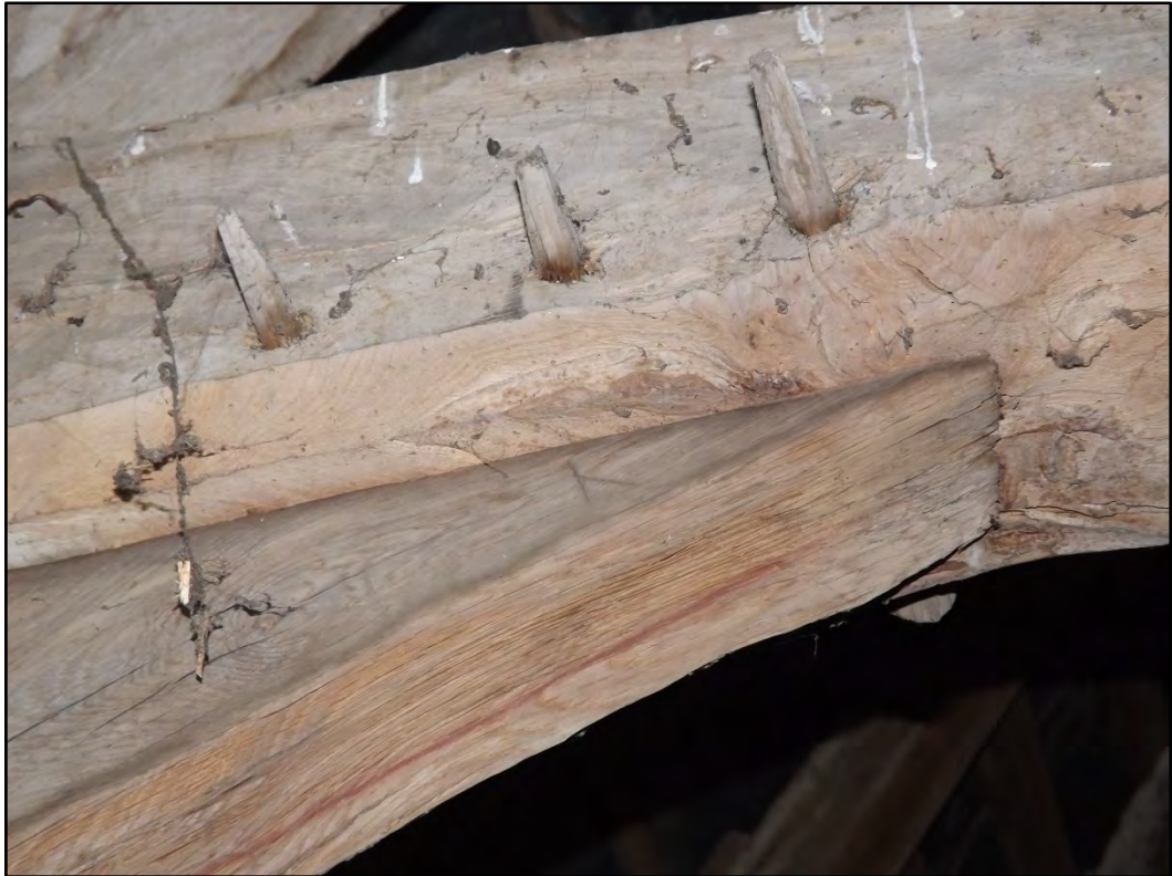
Detail of joinery, with a carpenter's mark central to the image Fig 34
