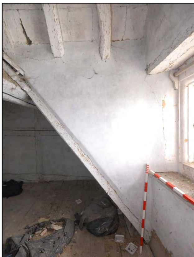
The interior face of the east elevation of Dormer 2 Fig 29
