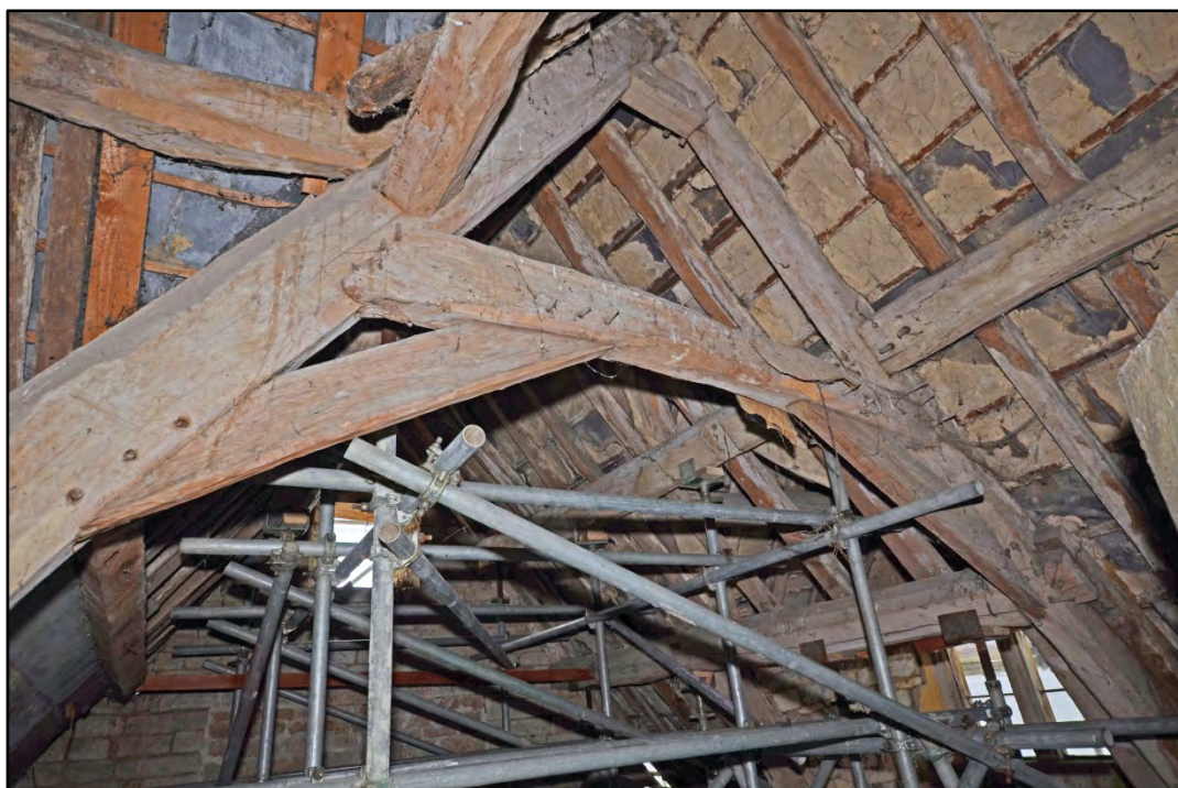
The upper extent of the cruck truss Fig 32
