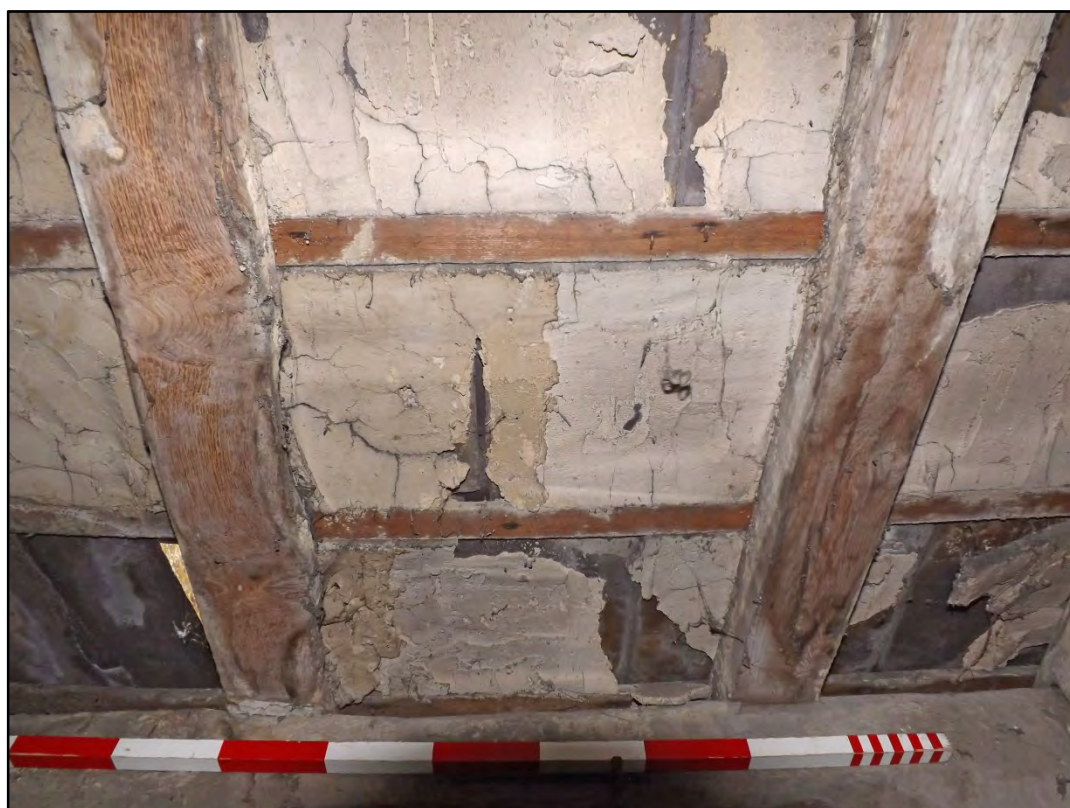
Detail of daub on the underside of the roof slates Fig 7
