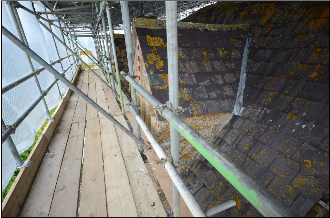
General view of the Dormer windows, looking west Fig 14
