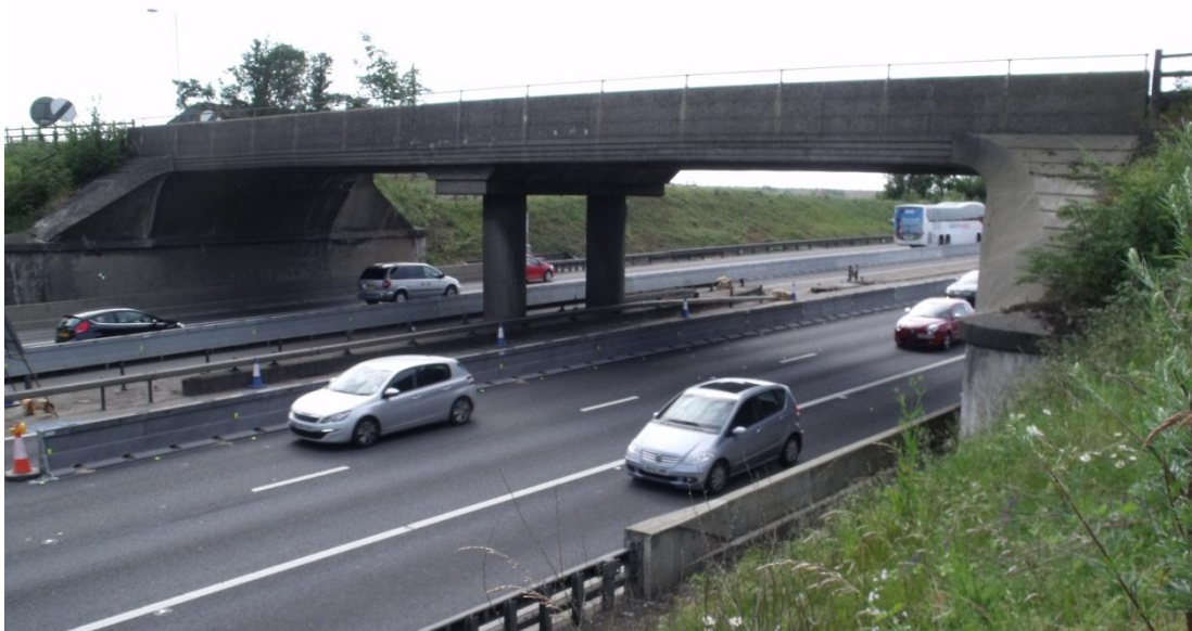
Houghton overbridge, M1 motorway, looking east Fig 34
