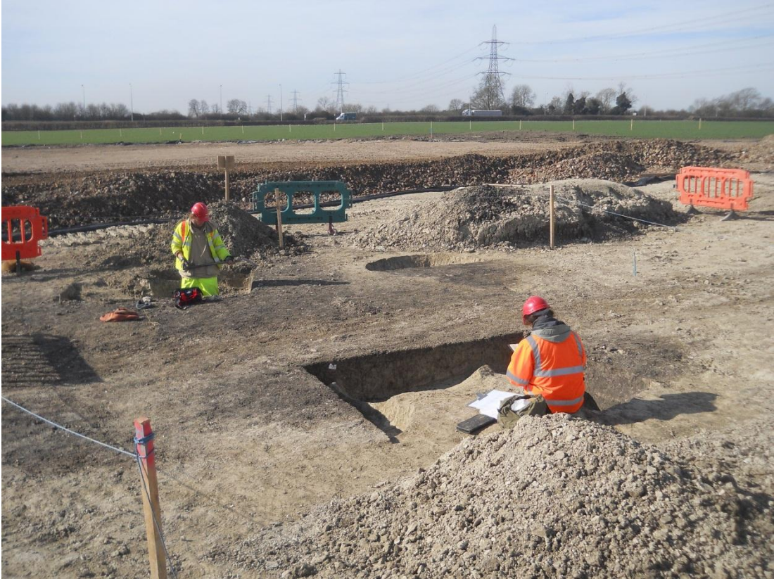
Investigation of an intersecting pit cluster, north of Thorn Road, looking west Fig 6
