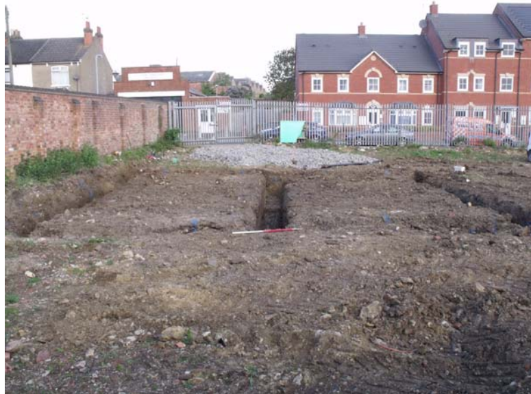
Overview of the foundation footings for plots 1 and 2, looking north-west Fig 6
