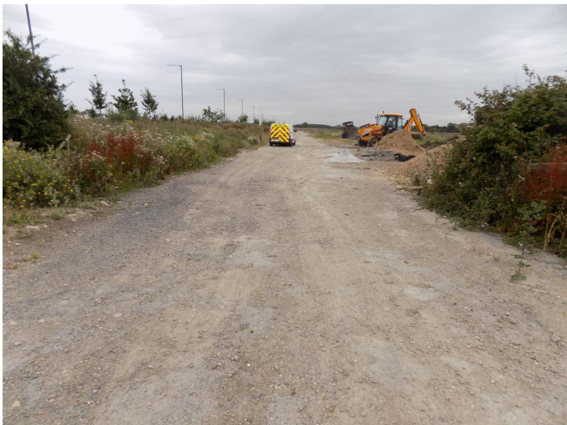
Concrete road way across southern edge of site, looking south-west Fig 4
