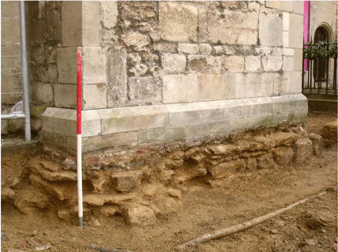
Foundation of the south turret of the 14th-century West Gate, partially disturbed by early 20th-century services, looking south-east Fig 3.5
