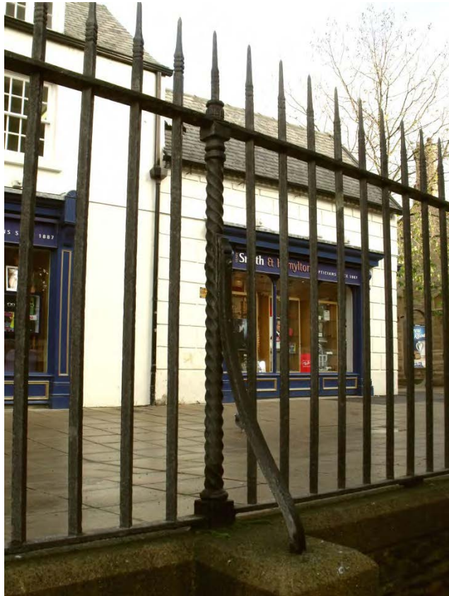
Churchyard railings on the north side of the church Fig 3.41
