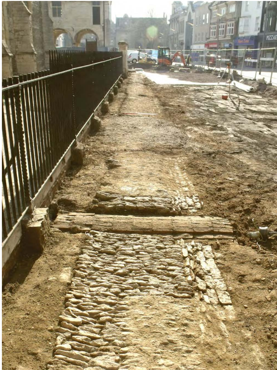
Pitched-stone pavement with an open gutter along its outer edge, to the south of the church, cut by a Victorian brick culvert, looking east Fig 3.30
