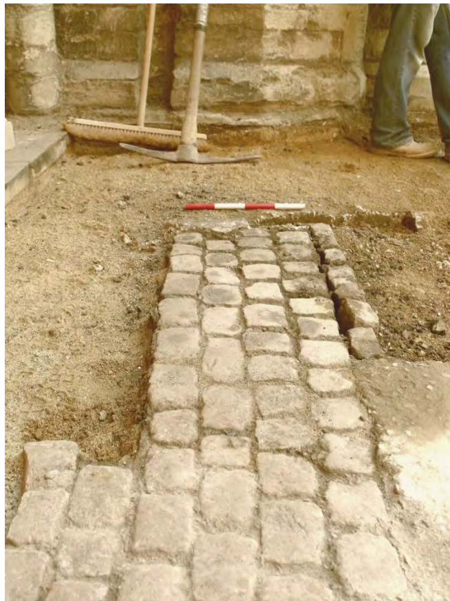
Remnant of late 19th to early 20th-century granite setts under the Cathedral West Gate, looking south Fig 3.45
