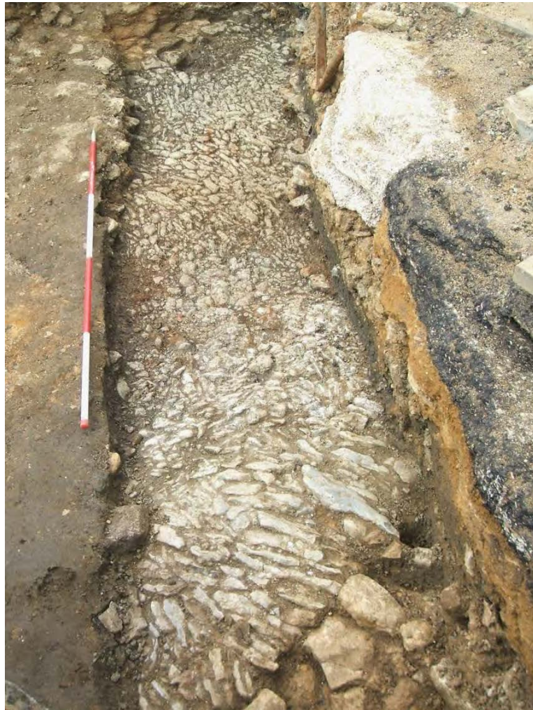
Pavement and street surface on the west side of Building 3 Fig 3.19
