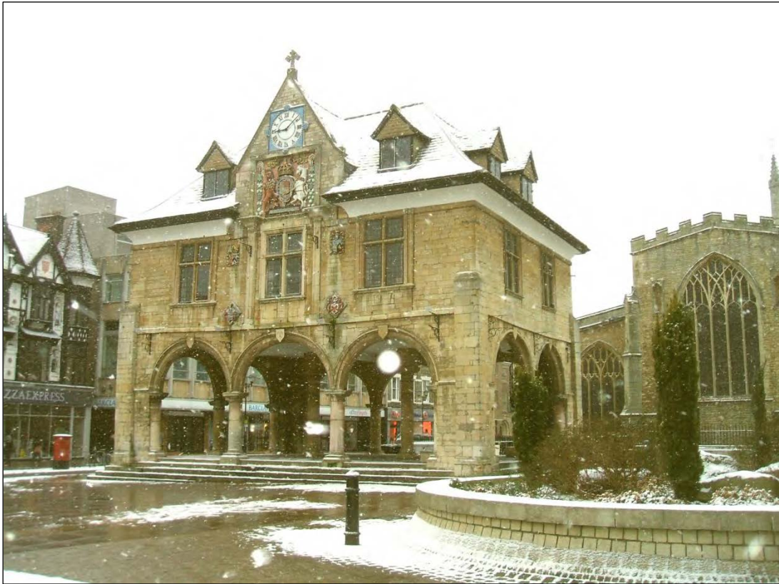
The Guildhall, built in 1671, looking south-west Fig 2.4
