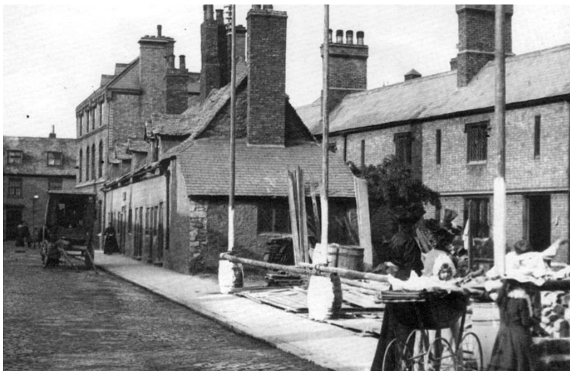
Demolition of the almshouses in 1903, looking north-east Fig A7.5
