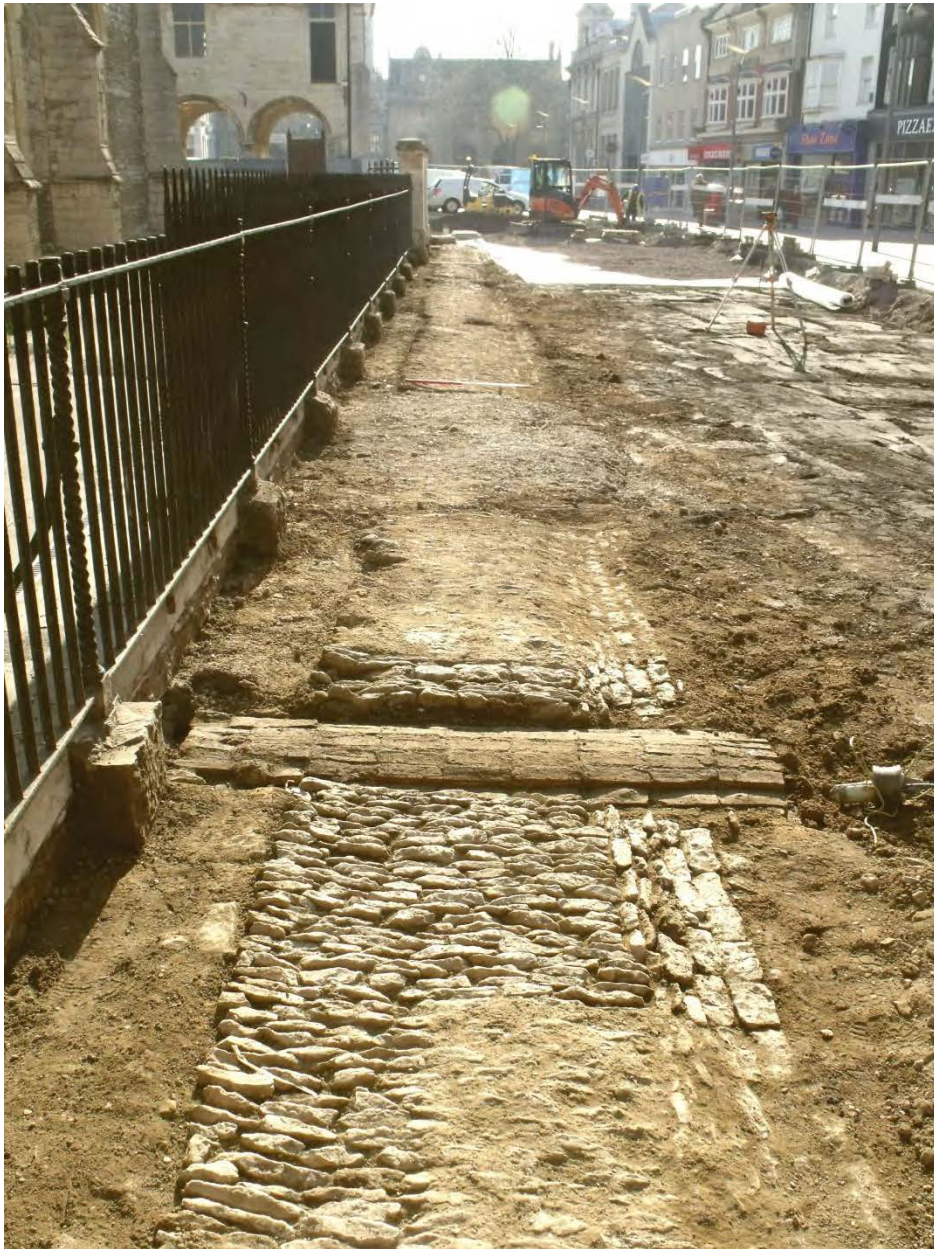
18th-century pitched-stone surface cut by brick culvert, looking east
