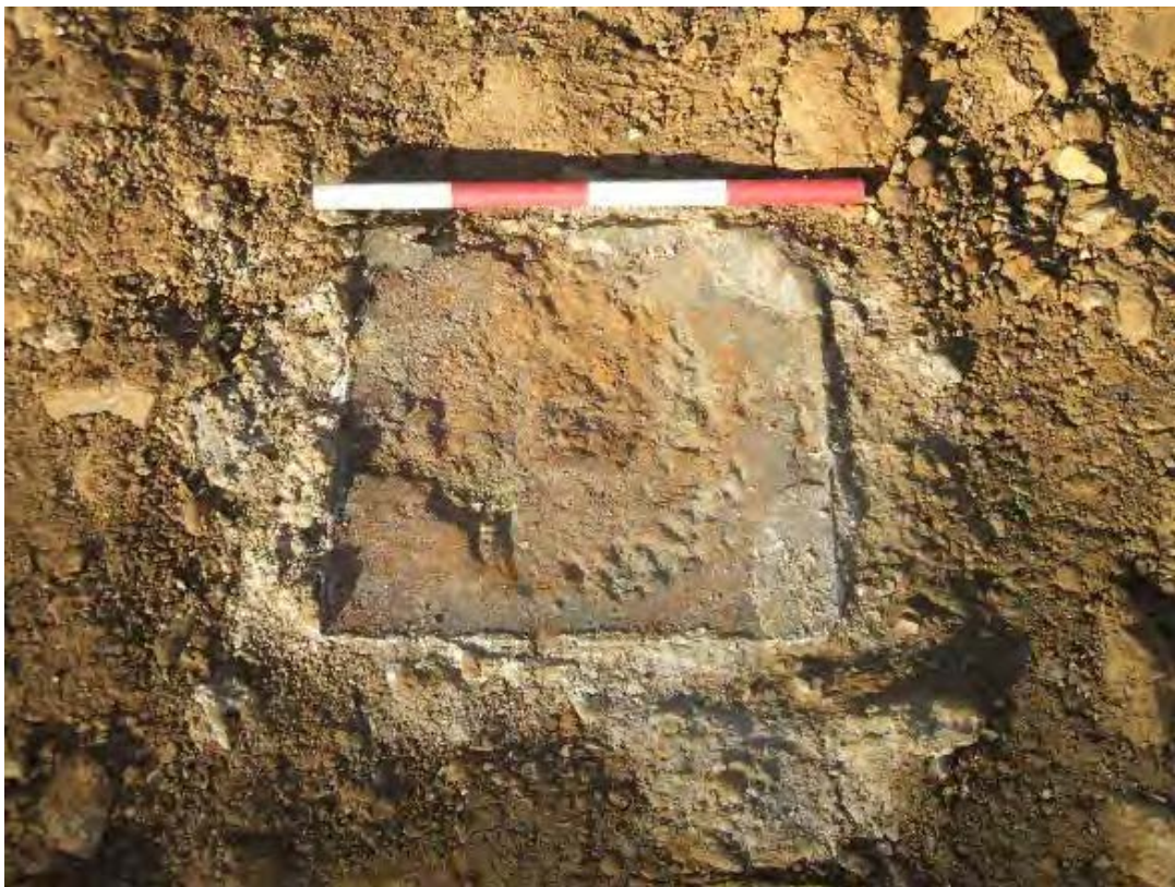
One of the ten square bollard bases forming a line adjacent to the east side of the Guildhall, probably dating to the early 20th century and set in 18th to 19th-century make-up deposits Fig A2.48
