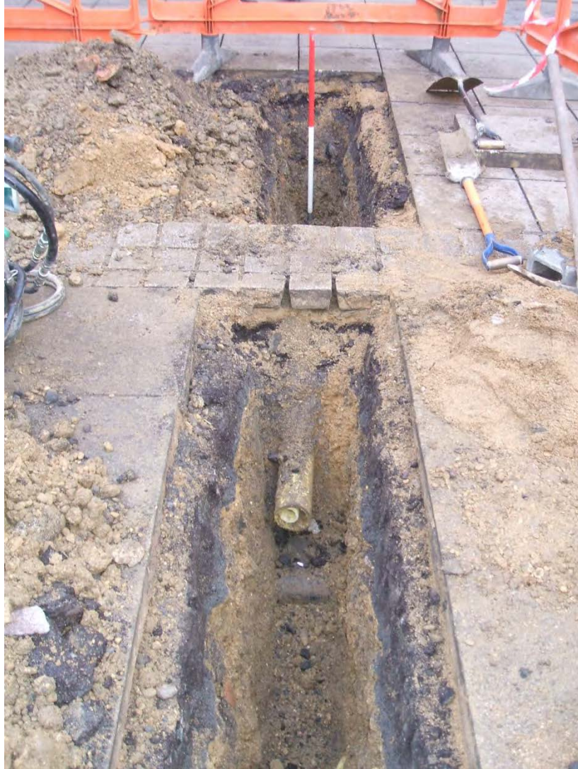
Services and dark fuel ash layer, Trench 13
