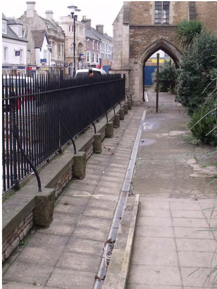
A view of the churchyard on the south side of the church, displaying the 1980s replacement churchyard wall [1516], with the limestone plinths supporting the 19th-century iron railings, looking west Fig A5.19
