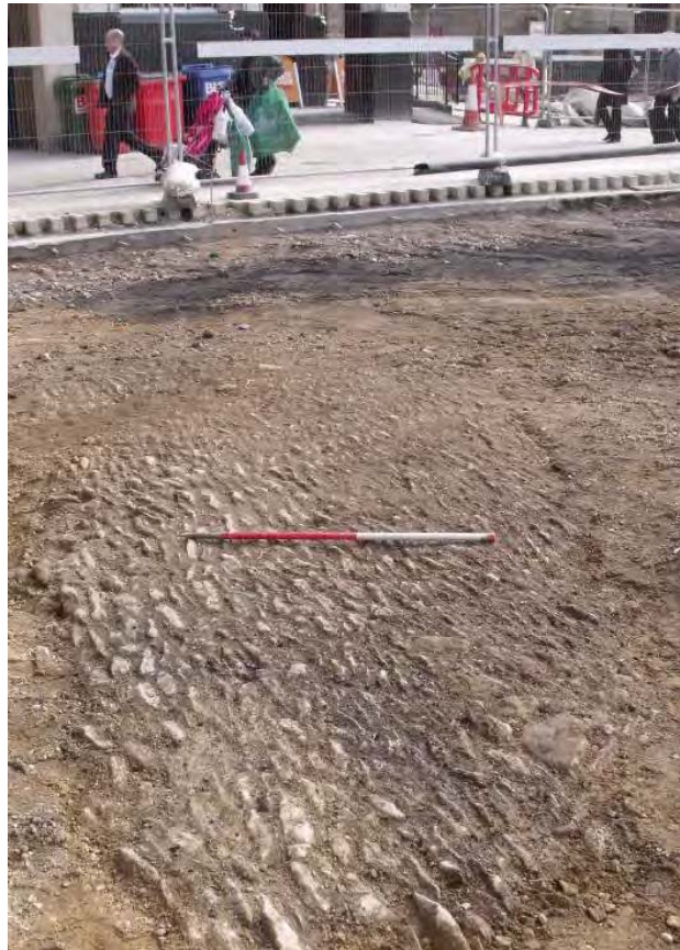
Late 18th- to early 19th-century pitched-stone surface, east side of Cathedral Square, looking east Fig A1.10
