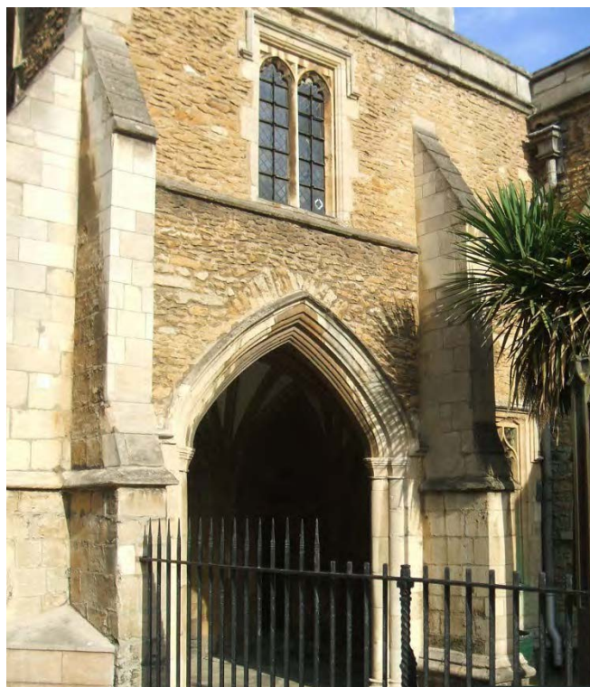
The 15th-century church porch, with the 19th-century buttresses at the south-east corner, looking south-east Fig A4.9
