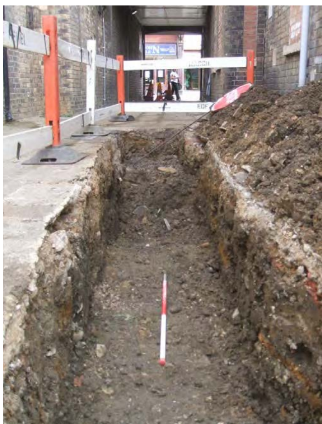
The alleyway trench looking north towards Cowgate, with the covered frontage in the background Fig A10.1
