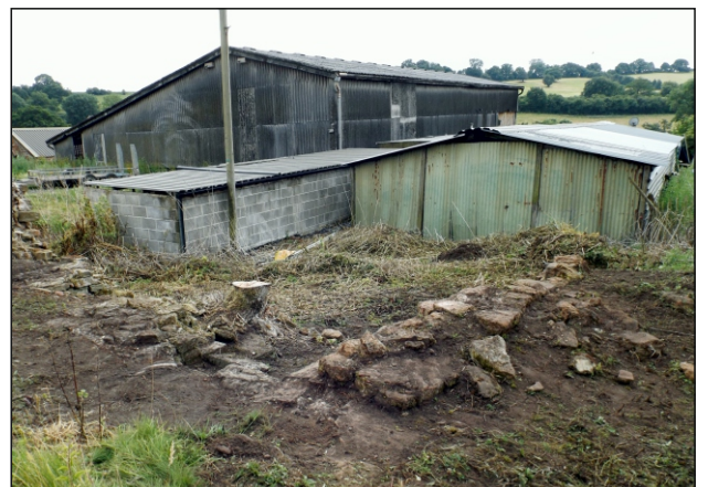
(d) Area B, after clearance of surface rubble, looking south-east
