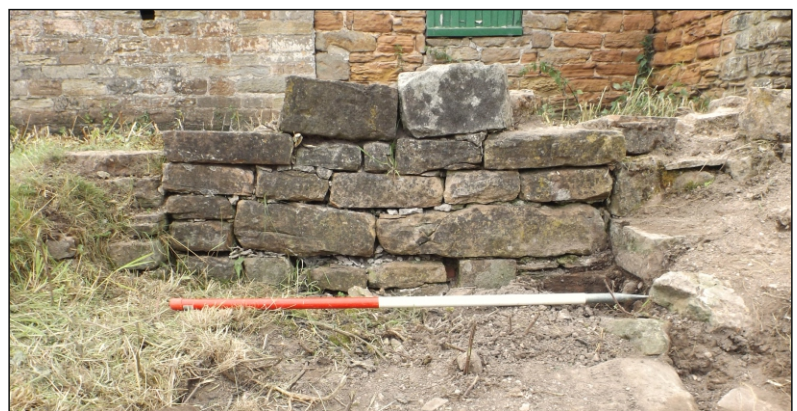
(e) The blocked doorway 107, looking west
