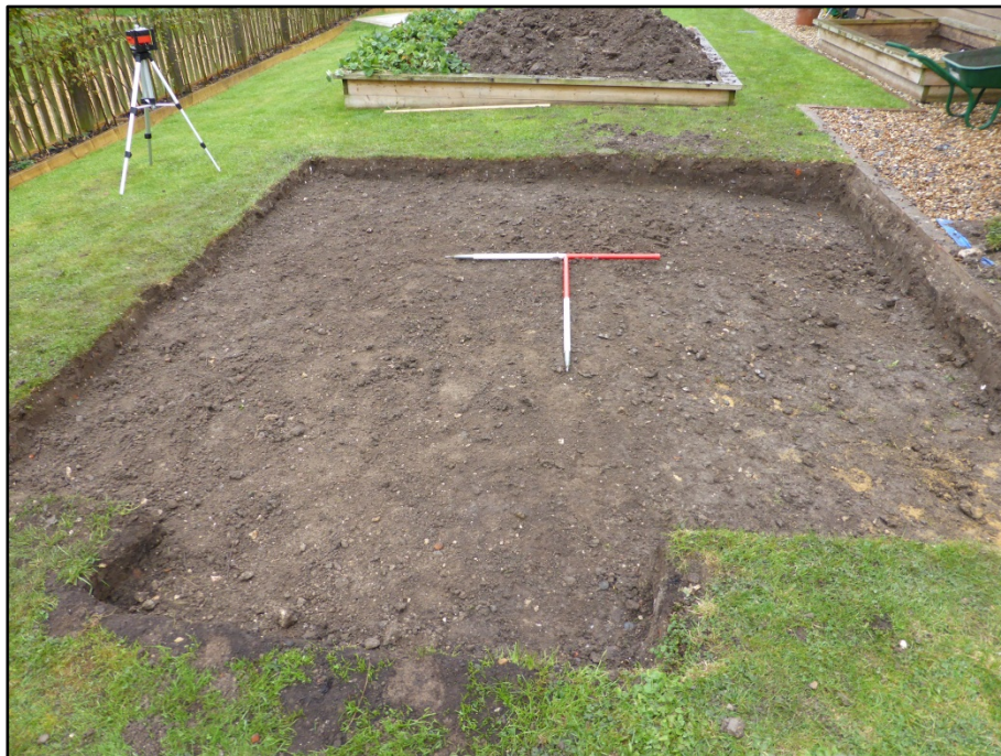
The completed stripped area, looking south Fig 5
