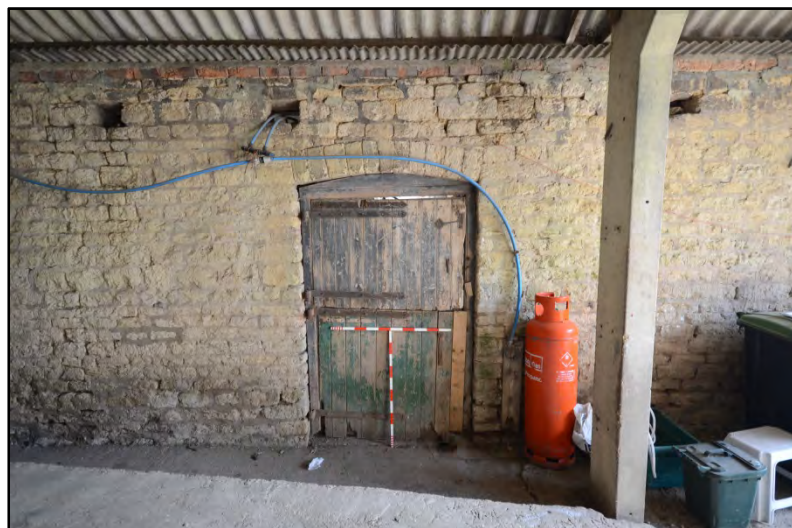
Room 7, detail of doorway Fig 49
