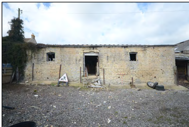
The south elevation of Room 7 / Barn B Fig 18
