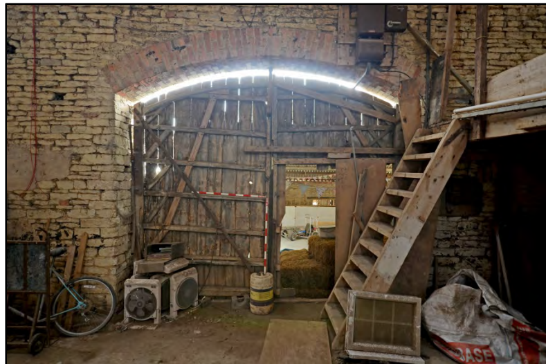
Room 2, detail of south doorway Fig 27
