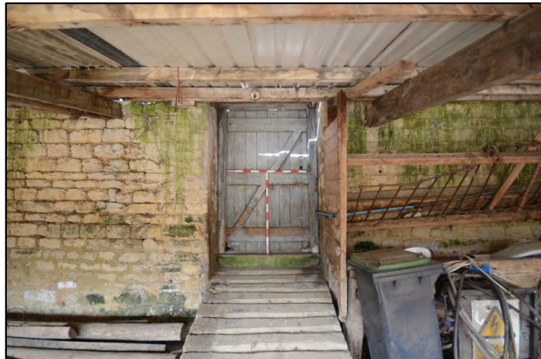
Door and concrete ramp to room 6, the Chicken Shed Fig 41
