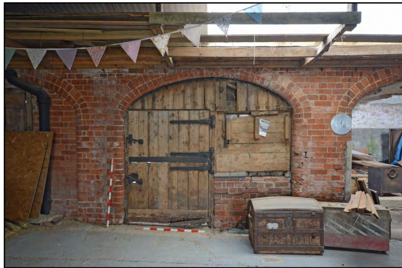
Room 3, former arched opening with timber and brick infill Fig 36
