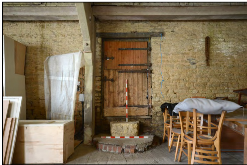
Door to Room 1 Fig 21
