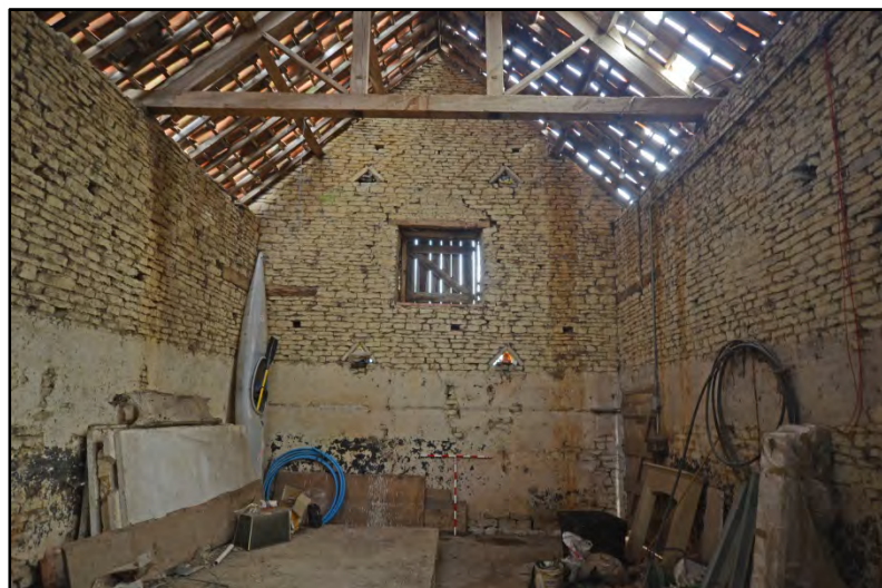
Room 2, looking north-east Fig 25
