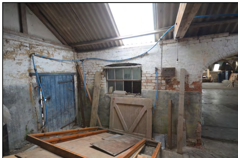
Room 3, former arched opening with brick infill Fig 37
