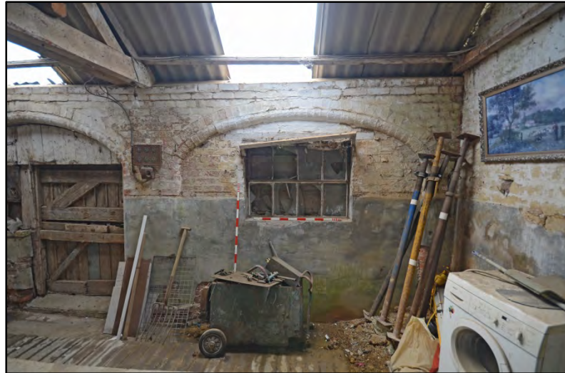
Room 3, former arched opening with brick infill Fig 35
