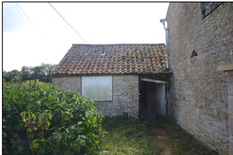
Room 4, the Milk Room, looking south-east Fig 13
