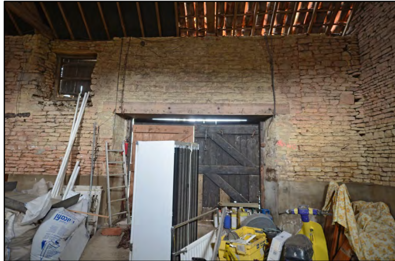
Room 1, detail of the north doorway Fig 23
