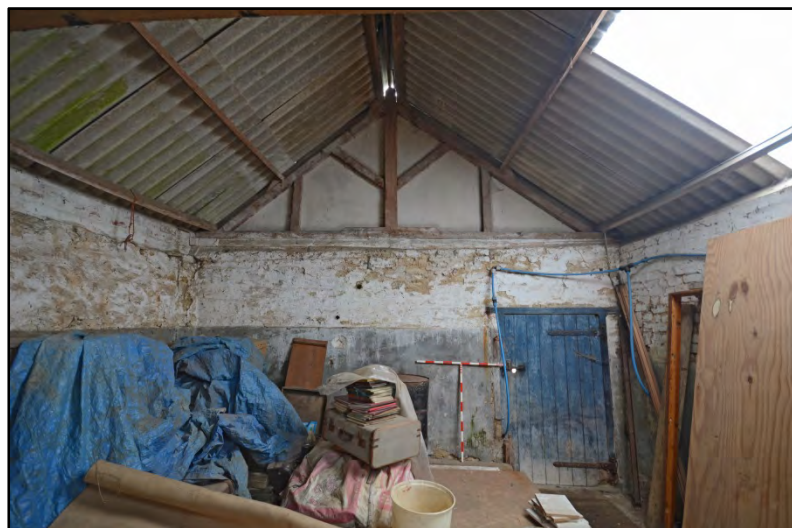
Room 3, detail of the south internal elevation Fig 31
