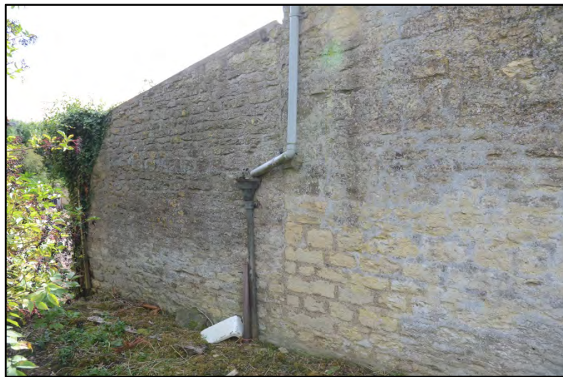
Vertical joint between the east range and the Chicken Shed Fig 15
