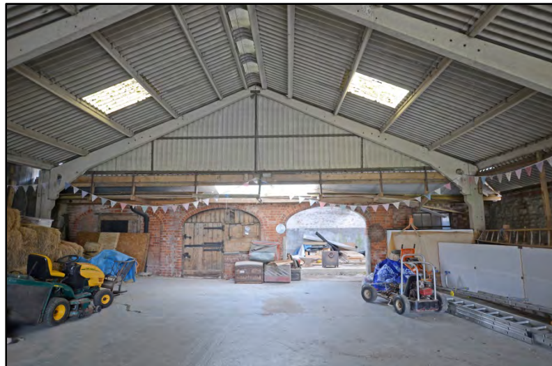
The west elevation of Room 3 Fig 34
