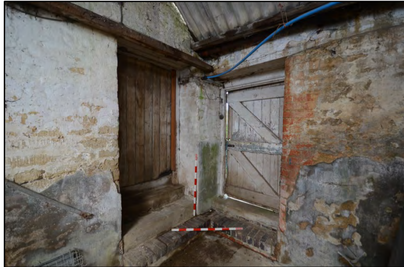
Doorways between the north and east ranges and Rooms 4 and 5 Fig 29
