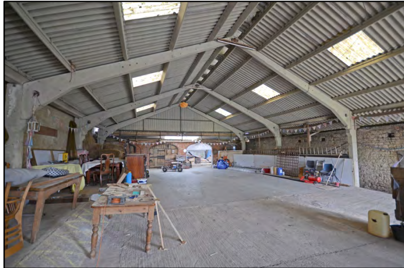
The modern central shed Fig 20
