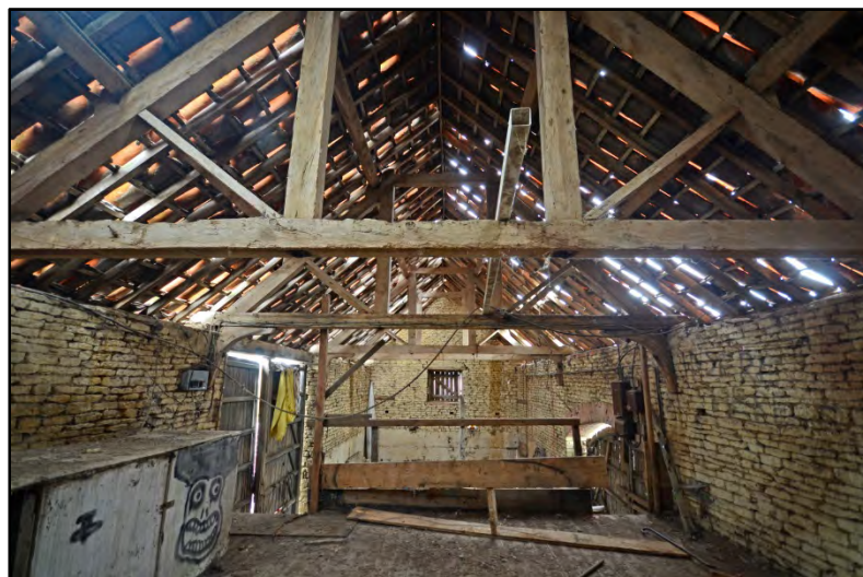
Room 2, detail of roof from the platform Fig 28
