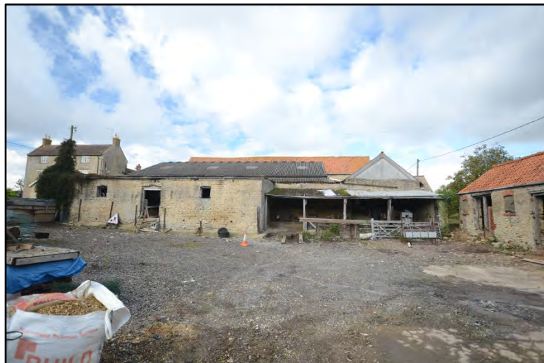
General view of the south range and yard Fig 16
