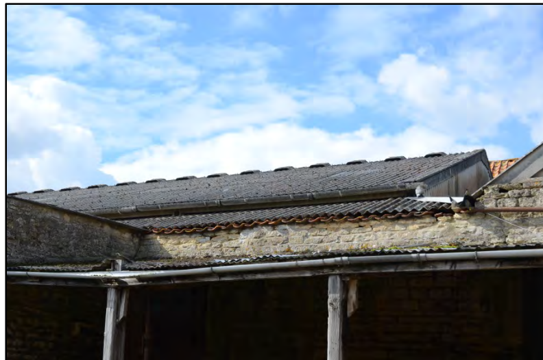
Capping pantiles over the south wall Fig 45
