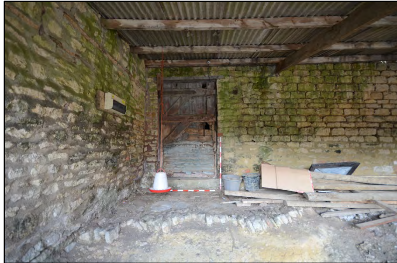
Remains of cobbled floor surface Fig 44
