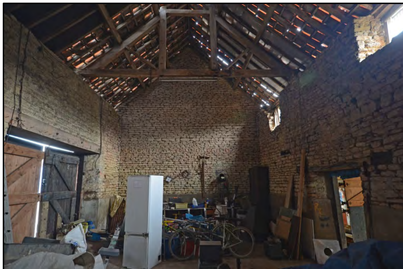
Room 1, looking north-east Fig 22
