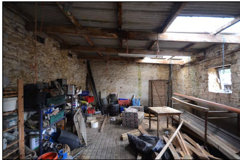
Room 7, looking north-east Fig 48
